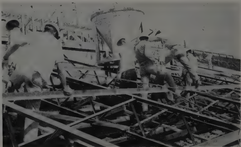
CREW operated on an obstacle course during the pour. Tops of the steps were hand finished, but the risers were produced directly by the form which is 48 x 30 ft. in area.
