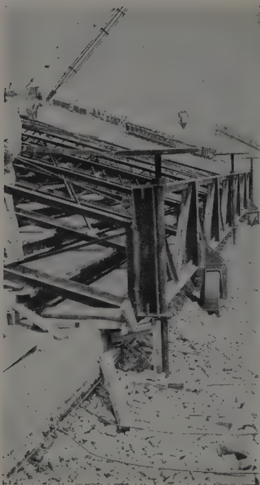
DETAILS of the solid-rubber wheels and jacks. For making a move the jacks raise the lower edge of the form and the two wheels are bolted on. After the form is rolled forward the jacks again raise the form so the wheels can be removed and the form lowered.
