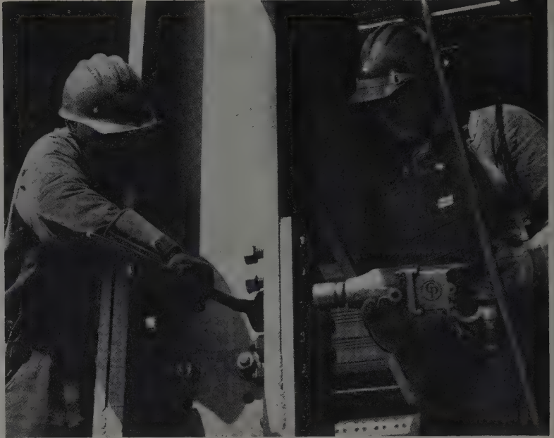
TURNING THE HEAD instead of the nut is a satisfactory way to tighten high strength bolts. This is sometimes necessary to avoid having long bolt ends interfere with fireproofing. The modified turn of the nut method is being used which allows the nuts to be run up snug and then tightened one half turn. Filler plates, not visible, have been welded to upper column flanges.
