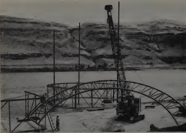
TEMPLATES 60 to 70 ft. in diameter are being assembled on the north shore in preparation for driving sheet piling. The resulting cofferdam will enclose a work area for the navigation lock, spillway, fish ladder facilities and non-overflow section.
