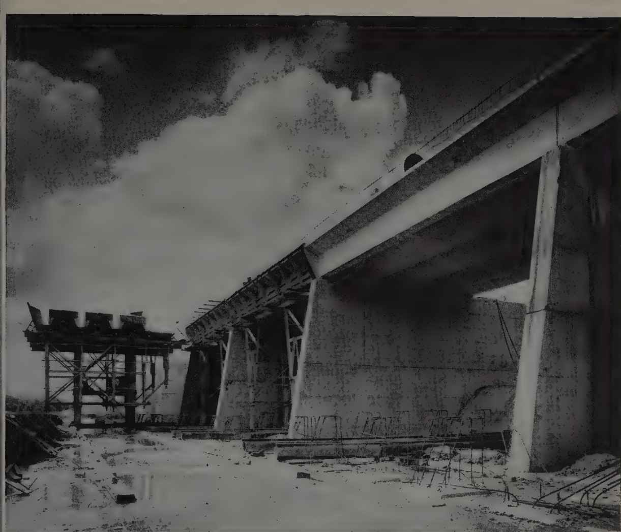
Ten-ton Blaw-Knox bridge deck form moves on traveler to new position. Steel chains for fir gates are cast integrally with girders. Old River Control Project is a $47 million job designed to preserve Mississippi's flow into its lower basin.
