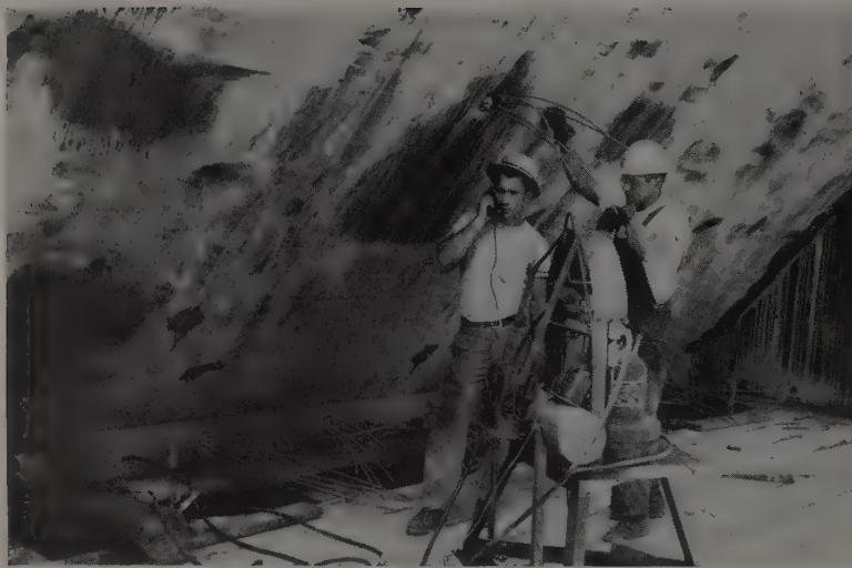
PRESTRESSING CREW keeps in touch by telephone with men at other end of pontoon so jacking can proceed simultaneously. Hydraulic jack is operating at lower left.
