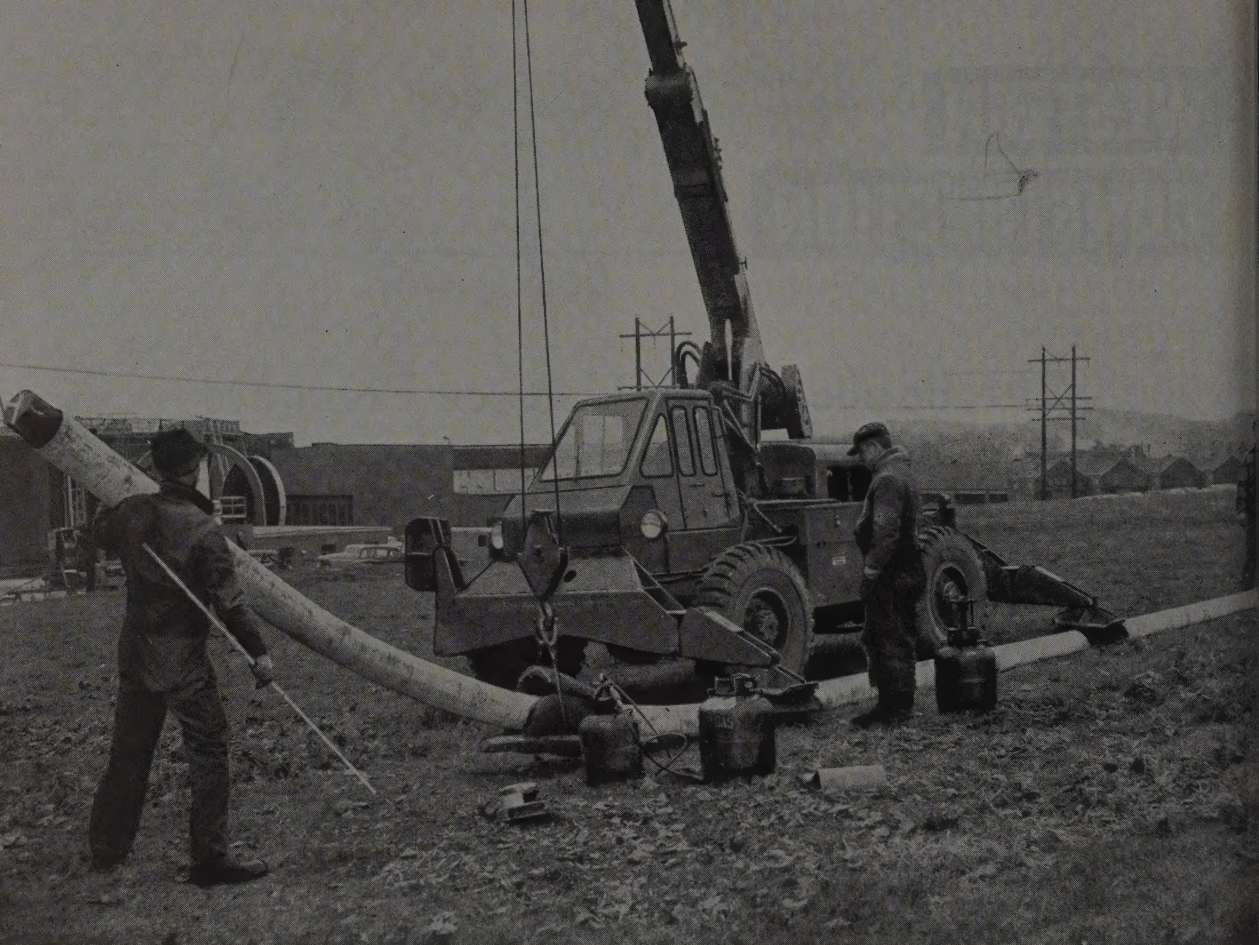
A-W Hydraulic Crane shown bending pipe-type cable at Wright-Patterson Air Force Base, Dayton, Ohio. Two hydraulic outriggers on the sides of the crane hold the pipe while the boom pulls it up into the desired curve.
