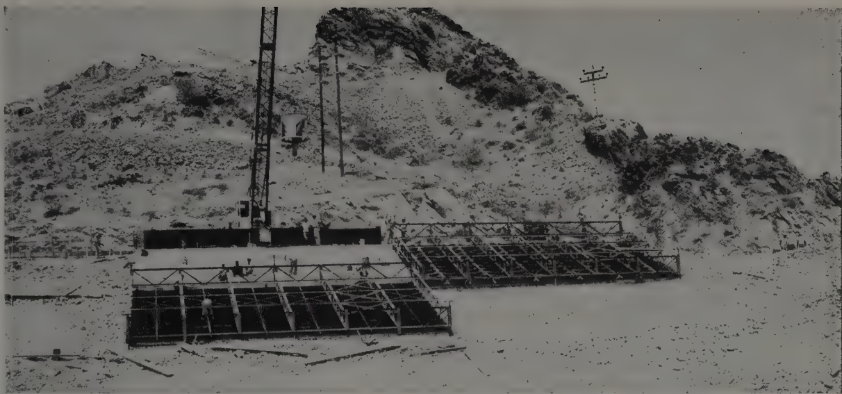
TEMPE BUTTE provides the background for this construction scene at the new stadium. The form at the right has just been rolled into a
