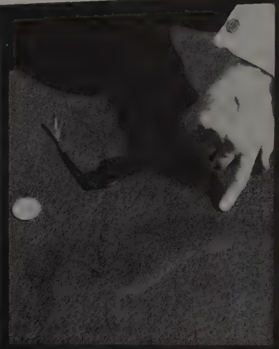
These photos tell the "before and after" story of Bitumuls Slurry Sealing. Notice in the photo, right, how the large crack in foreground has been filled and sealed.
