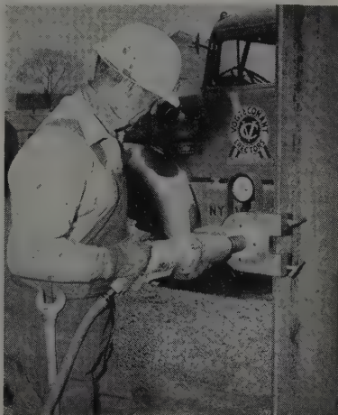
WRENCH CALIBRATOR, manufactured by Skidmor-Wilhelm, measures tension in the bolt by hydraulic pressure shown on dial gage.
