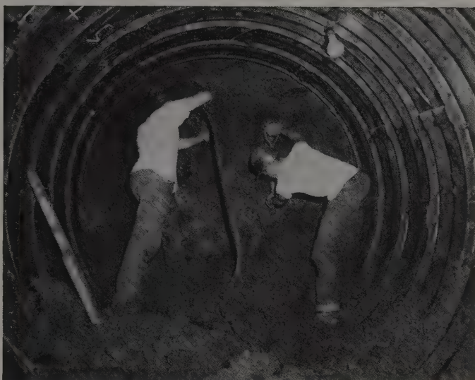
Tunneling under railroad tracks for new sewer in Topeka, Kansas. The Armco Construction Department installed Armco Liner Plate on a subcontract for the general contractor.
