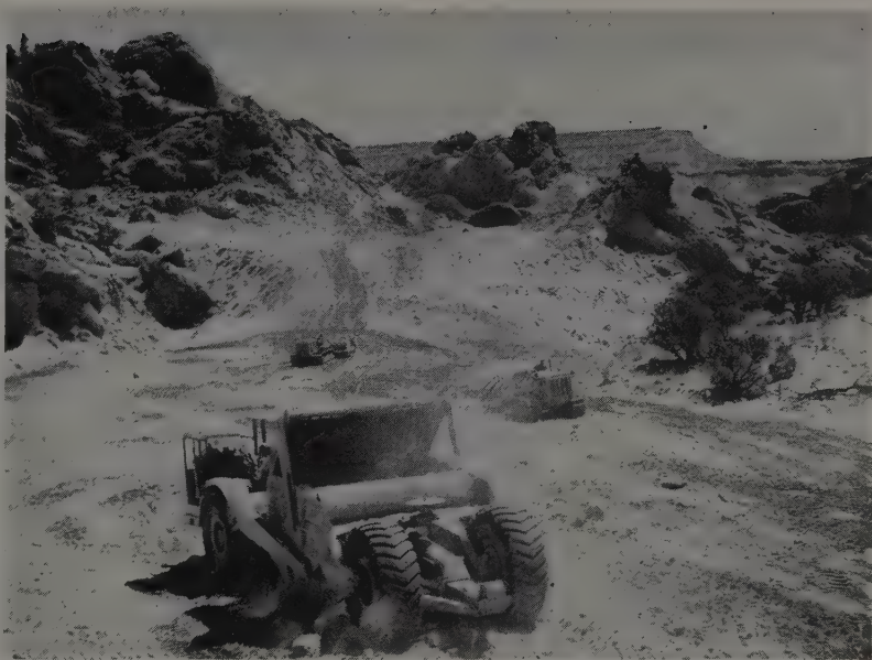
UNLOADING part of the 1,000,000 cu. yd. of material which was moved is a Cat DW21. In the background, compaction is carried out by sheepfoot rollers and D8's.
