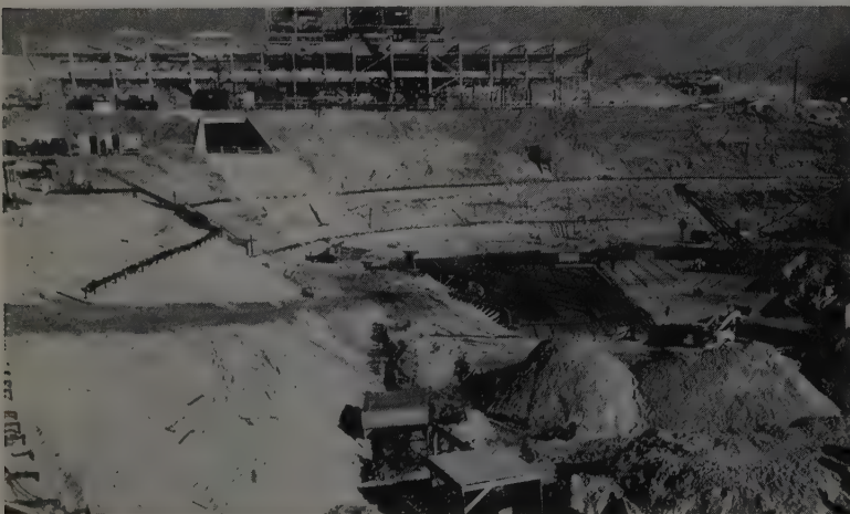
AT THE SITE of a large steam power station in Southern California, this multi-level installation was used to pull down the water level about 30 ft. and hold it there for several months.
