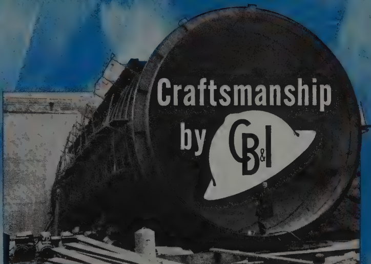
Penstocks for Mountain Home—CB&I built three, 22-ft. diam. penstocks for the Idaho Power Co.
