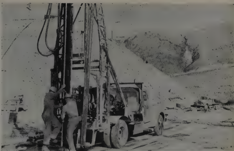
CASINGS are placed in the holes drilled through the clay layer. The rig shown can quickly be converted from percussion to rotary drilling, a contractor idea.
