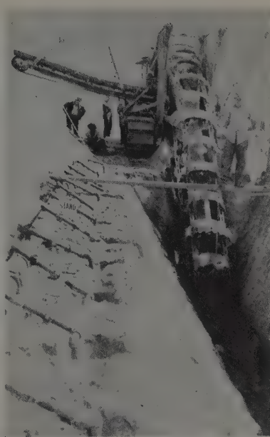
DEWATERING OF trench excavations is frequently done with wellpoints, as shown in these two examples. Usually a line on one side of the trench is sufficient. The practical limit of water lowering below the header is 15 to 18 ft., but altitude of the job has to be considered.
