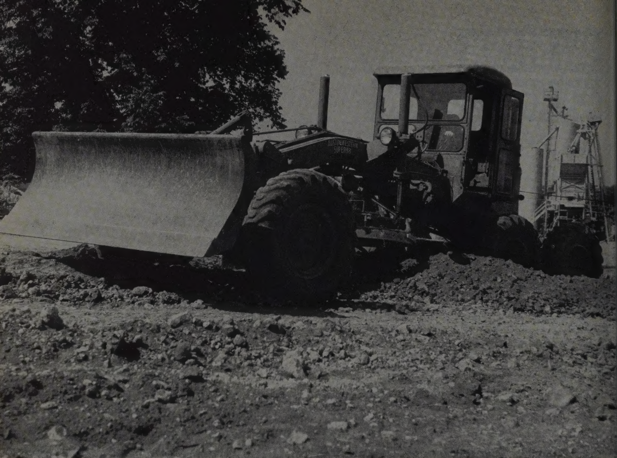
Powerful 6-wheel Austin-Western tandem grader prepares bedrock surface for construction of a cloverleaf, part of the giant New York thruway project. Rear wheels are offset to compensate for sidethrust of fully loaded blade.
