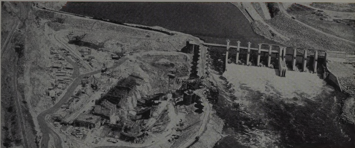
COFFERDAM swings out from west side of Columbia River to protect powerhouse work at Rocky Reach Dam. Concrete batch plant
