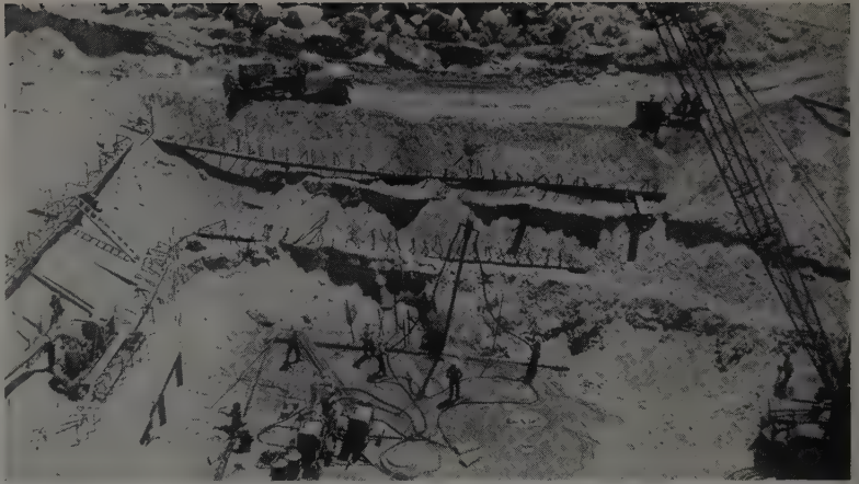
WITH THE AID of a truck crane workmen at the Mammoth Pool Dam project jet into place wellpoints at 2-ft. spacing for a pit to test foundation materials. Located upstream from the cut-off excavation this system intercepted the majority of the seepage, simplifying excavation.
