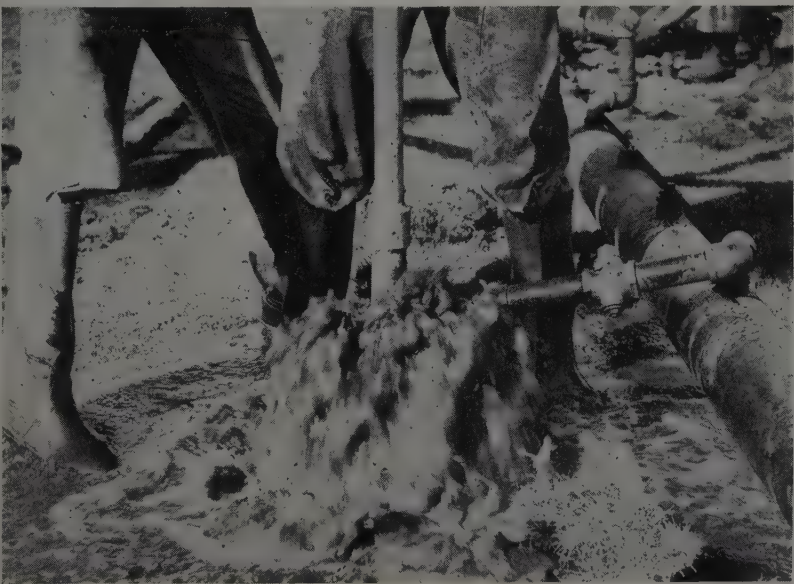
JETTING ACTION used to sink a wellpoint. In properly graded material, no sand envelope is required. Note the stop-cock on the line that will connect the wellpoint to the header. This cock can be used to control the volume of air coming in through the wellpoint.
