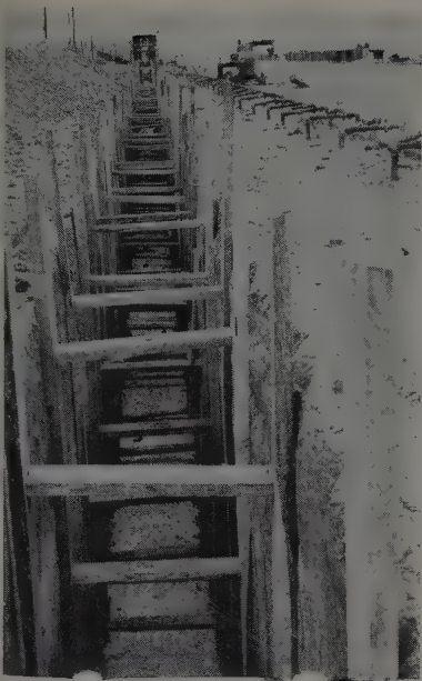
DEWATERING OF trench excavations is frequently done with wellpoints, as shown in these two examples. Usually a line on one side of the trench is sufficient. The practical limit of water lowering below the header is 15 to 18 ft., but altitude of the job has to be considered.
