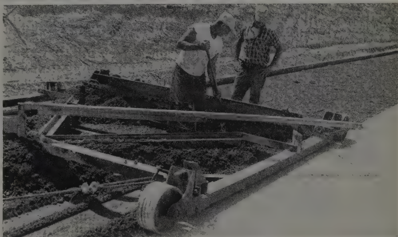
PAVING TRAIN includes two pieces of contractor-built equipment. Both are pulled by tractors and run on solid rubber wheels. In top photo is a windrower; in the bottom photo is a spreader for base material. Spreader has long-handled rudder to direct material.
