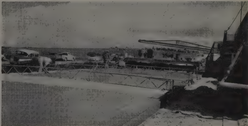
FIG. 3—Feature of the attachment is the runners extending from the front of the sled back into the concrete. The fabric rides down these rails and into the concrete at the specified depth 2 in. below the surface. The timbers under the corner wheel are to lift the front edge of sled to pass over the dowel bars.
