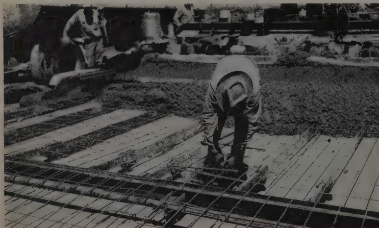
FIG. 1—Spread out in front of slip-form paver is the 6 x 12-in. welded wire fabric with provision for sawn joints at 106 ft. 6-in. spacing.
