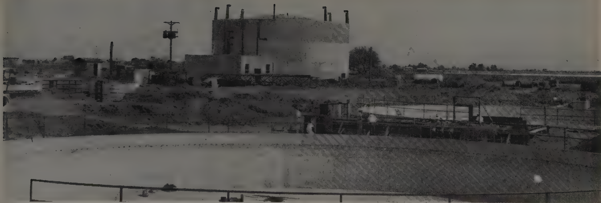
THIRTY-FOOT wall of digester in the background was formed with Symons panels, using small filler strips to secure circular pattern.
