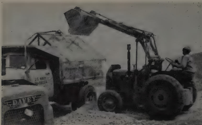
NAVY FORCES developed this system for screening clay to minus \frac{1}{2} in. Powered by air a regular concrete vibrator was mounted on the sloping screen which was fastened to the truck. Loads were tail-gate spread on the floor of the test ponds.
