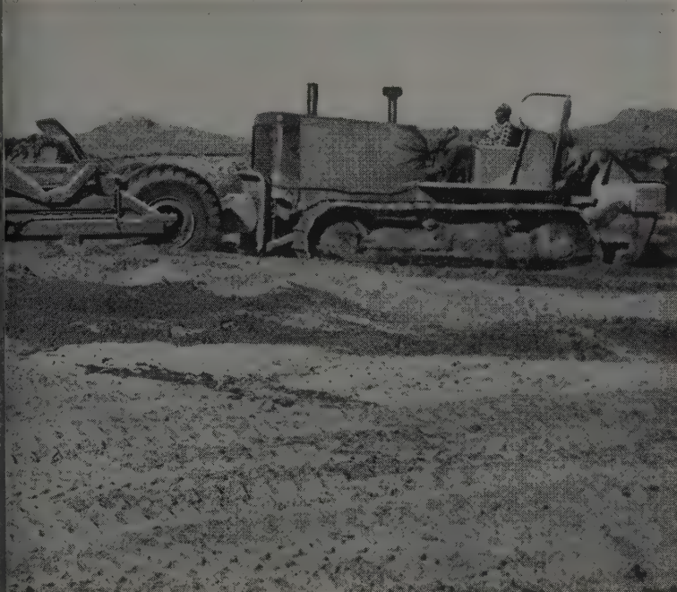
Compacting scraper-hauled fill, big HD-21 crawler tractor tows four-gang sheepfoot roller.
