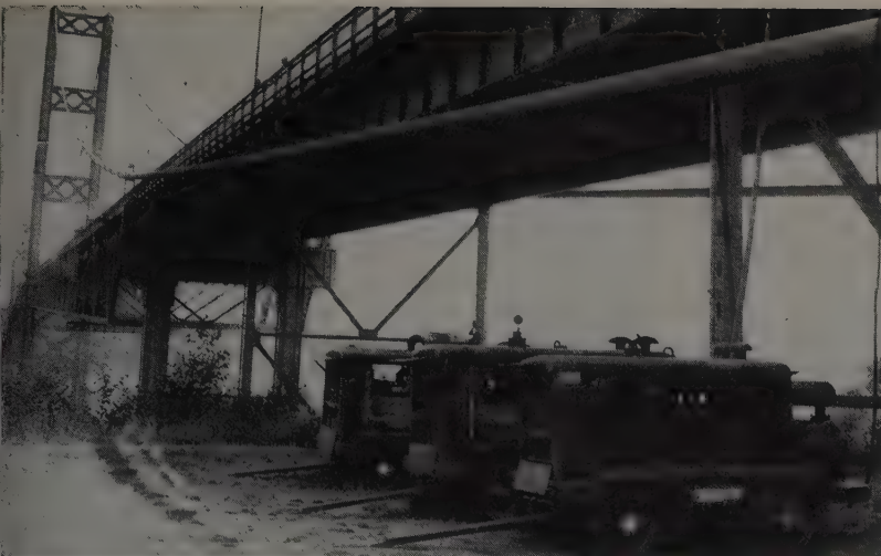
1565 CFM OF 110 LB. AIR FOR BRIDGE CLEANING: Runnels Industries used these 3 Jaeger rotary compressors (two 600's and a 365), connected to a 3" air line, to supply twelve 5/16" sandblasting nozzles spread out over a mile along
