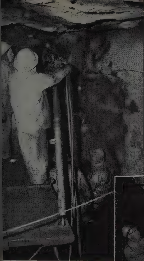
of the Ingersoll-Rand JR-38B Universal drills at work on the tunnel face. Each took 2 to 3 hours, and from 50 to 60 of rock were removed at each blast.
