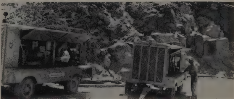
COMPRESSED AIR for the project is supplied by portable teams of Gardner-Denver compressors like the two 900's shown here. Job includes 1½ mi. of aluminum pipe with Wade couplings.
