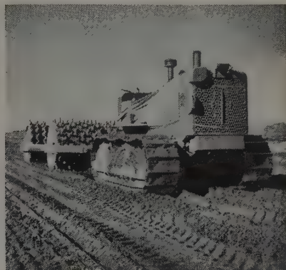
Compacting scraper-hauled fill, big HD-21 crawler tractor tows four-gang sheepfoot roller.
