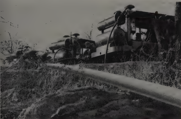
3 COST-SAVING IDEAS ON ONE JOB: This job, by Rambore, Inc., drilling specialists, was 280,000 cu. yds. of rock, mostly granite, in depths to 40', on Massachusetts' Southeast Expressway. One of their good ideas was to hook up their drills and compressors through 1500' of easily portable 5" aluminum pipe. This saved frequent moving of
