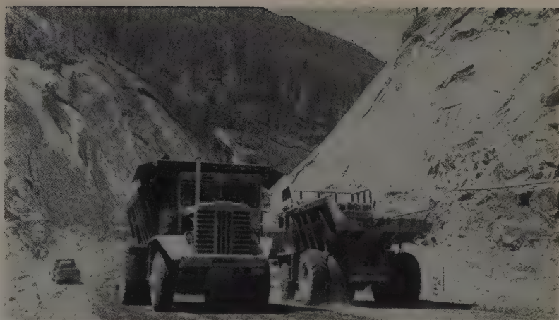
STEADY SHUTTLING of big rigs permits difficult excavation to progress at the rate of more than 5,500 cu. yd. per day. Note smooth granite cliffs which form dam abutments.
