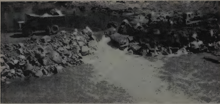
COFFERDAM CLOSURE took 12 hr. and was accomplished smoothly despite high flows. In photo a Payhauler backs in with a load of boulders which will close the final gap.
