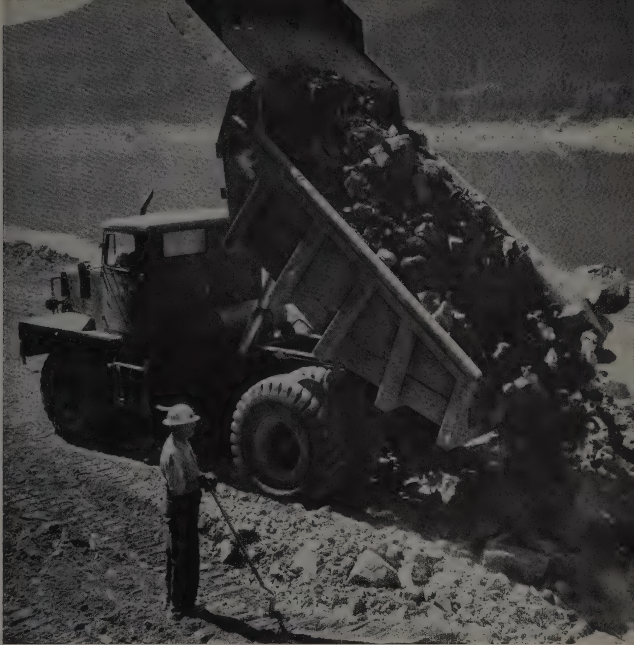
Dumping rock on a road-widening operation on Highway #10 in Washington's Cascade Mountains. Prior to this road job, Goodfellow's 22½ ton Macks were used in the 3,000,000 yd. excavation and backfill for the Rocky Reach Dam near Wenatchee, Washington.
