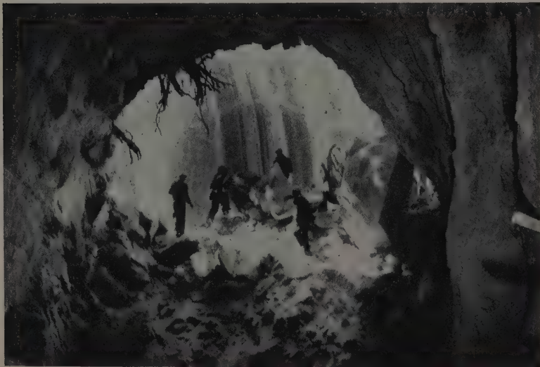
HOLING THROUGH the diversion tunnel came far ahead of schedule, another successful job for Morrison-Knudsen veteran P. "Whitey" Lee. Note waterfall on cliff opposite outlet.
