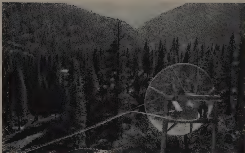
MICROWAVE relay dish located near camp sends signals to station atop peak. Project is thereby tied in to Southern California Edison's microwave communications network.
