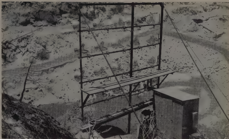
FLOODLIGHT TOWERS were spotted on almost inaccessible locations overlooking dam site. The towers hold twenty 1,000-watt mercury vapor lamps, are made of 3 x 3 x \frac{1}{4} steel angles.
