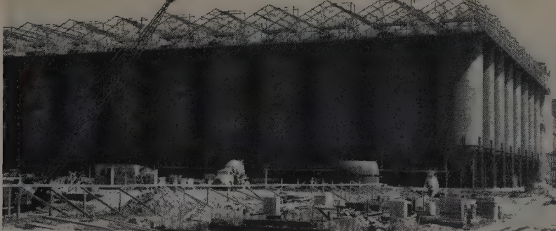
Part of the 144 cone bottom precipitators fabricated and erected for Alcoa by PDM. The units, each 24' diameter x 60' shell height, represent 8500 tons of plate-work, with another 3100 tons of structural steel on top.
