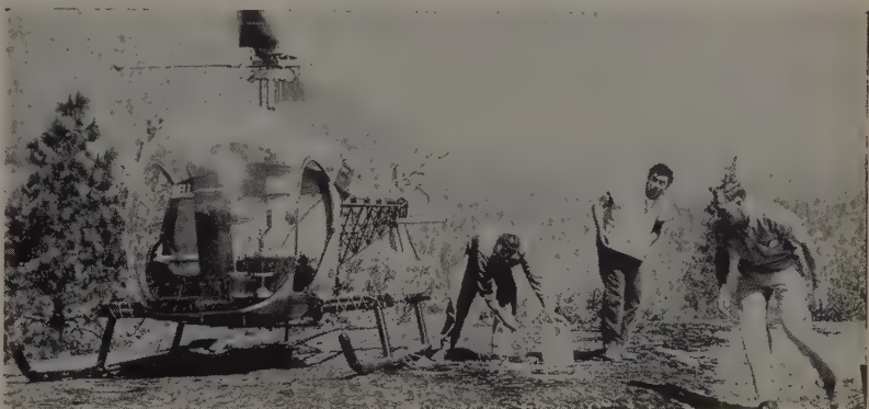
FLOODLIGHT TOWERS on dam abutments were erected with a Bell G-2 helicopter, which has a maximum load capacity of about 500 lb. Pole placement was done with larger Sikorsky rig.
