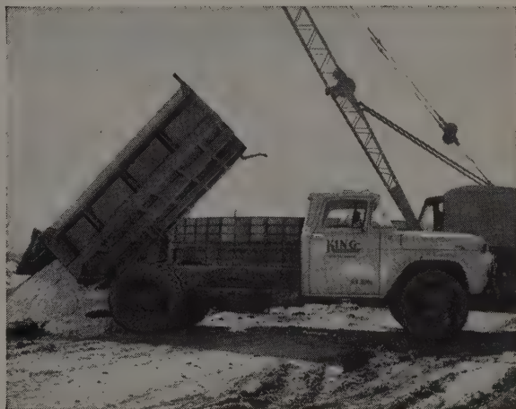
Carrying 5 to 6 yards of sand or rock , this Ford dump truck hauls many loads daily from nearby production sites.
