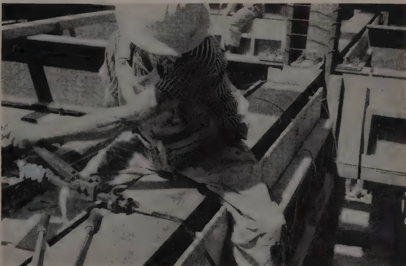
TENSION is applied to strap by movement of lever on tensioning tool. Final step is use of sealing tool, handles of which can be seen. Procedure is fast, easy to learn.
