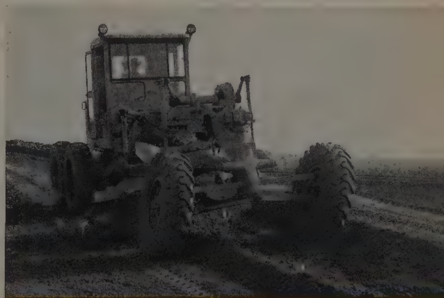
No. 12 Motor Graders, workhorses of highway construction, maintained haul roads and graded to fine tolerances. Grading was carried out in blocks 500 to 800 feet long.
