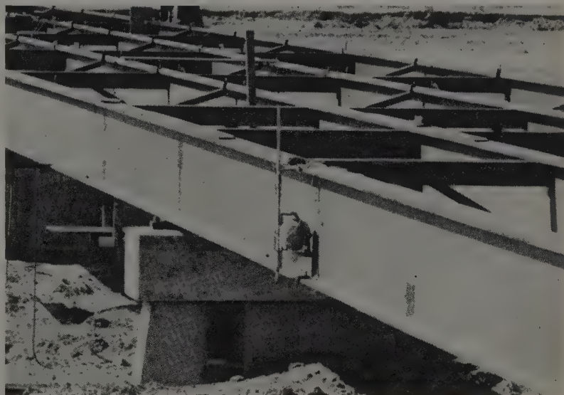
CLOSE-UP of projector in position at the butt splice. The film is in the lightproof holder on the opposite side of the weld. After warning all people and setting barricades, the operator throws the switch on the remote control box to make the exposure.
