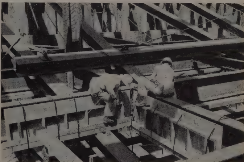
PRE-CUT STRAPS are spaced along beam at left. One man inserts straps through slots in side forms, drawing them underneath beam with aid of long wire. Man at right follows with tensioning and sealing tools. One man can do job alone, drawing strap from reel.
