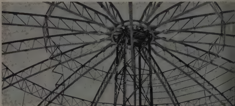
LOOKING UPWARD, photo shows center falsework tower supporting the compression ring, sixteen radial arch trusses, and the innermost circular bracing truss, nearing completion.
