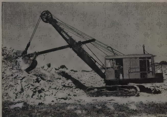
A Cat D337 Engine powers this Lorain shovel feeding rock to Pioneer portable crushing plant — part of the W. J. Menefee Construction Company's big Missouri Freeway linkage project.
