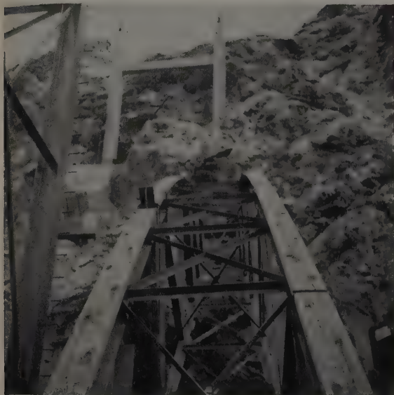
STEEL FALSEWORK on the ground ready for lifting into position shows the 3 x 12-in. planks bolted to the top flange. Planking 14 ft. long was placed transversely and then covered with 5/8-in. plywood to form the soffit of the concrete arch rib. The planking was made up with a railing to provide a prefabricated walkway for the form crew. Two ribs and the falsework weighed 1,600 tons. Arch has a rise of 65 ft.
