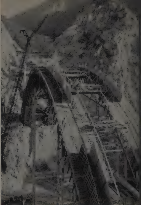
STEEL TRUSSES were supported on two steel towers. Fabricated in pairs, they were centered under the arch rib. This falsework design was selected to reduce hazard from brush fires and keep the channel open for floods. Pacific Iron & Steel Co. supplied falsework.
