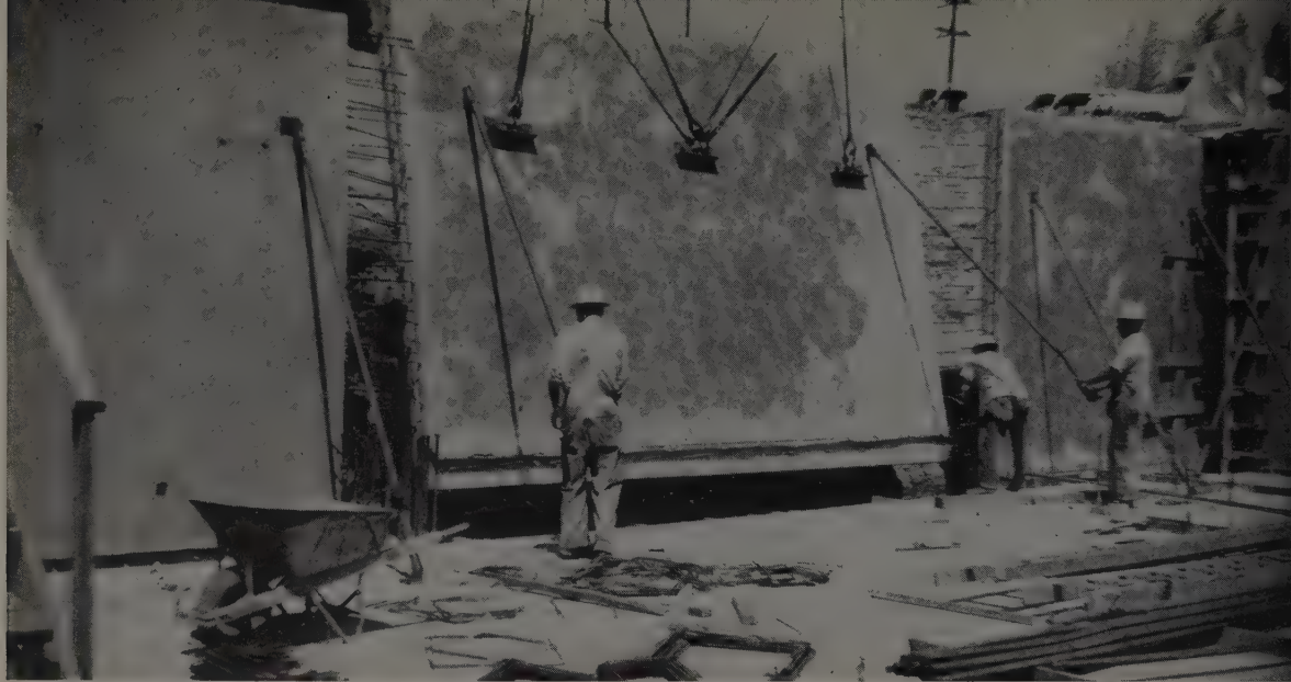
BASEMENT WALL PANELS were lowered into place after being cast on adjacent parking lot. Pipe supports held them in position temporarily while 2-ft. 2-in. spaces between panels were cast in place.
