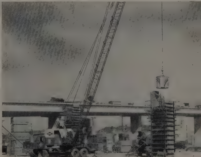
Lima Type 44-T Truck Crane pouring concrete into bridge pier form on the West Coast's largest freeway at Oakland, California.
