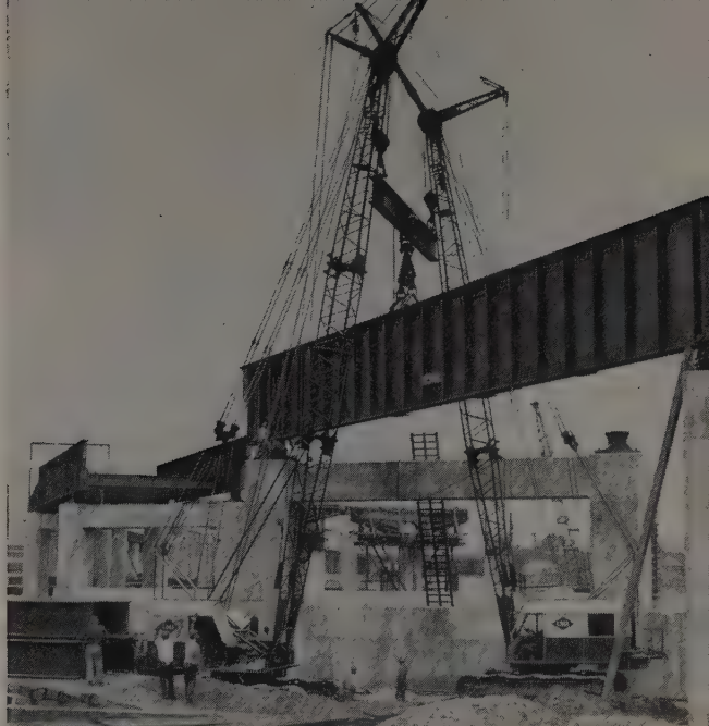
Two Lima Type 703-SC Cranes, equipped with 70' booms and 20' jibs, hoisting 110' long steel girder weighing 76 tons on the construction of a bridge over the Calumet River.
