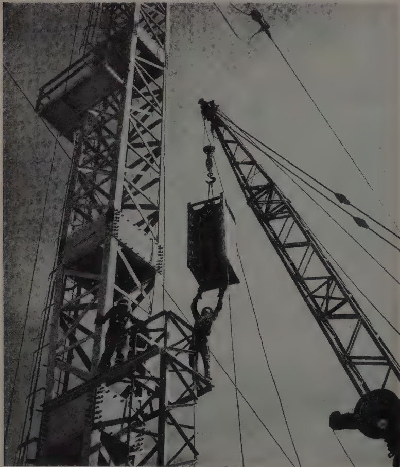
UNDER CONSTRUCTION—A Lorain Moto-Crane lowers a 6-ton counterweight into place at the base of the tilting headtower of the main cableway. The weight is composed of steel punchings.
