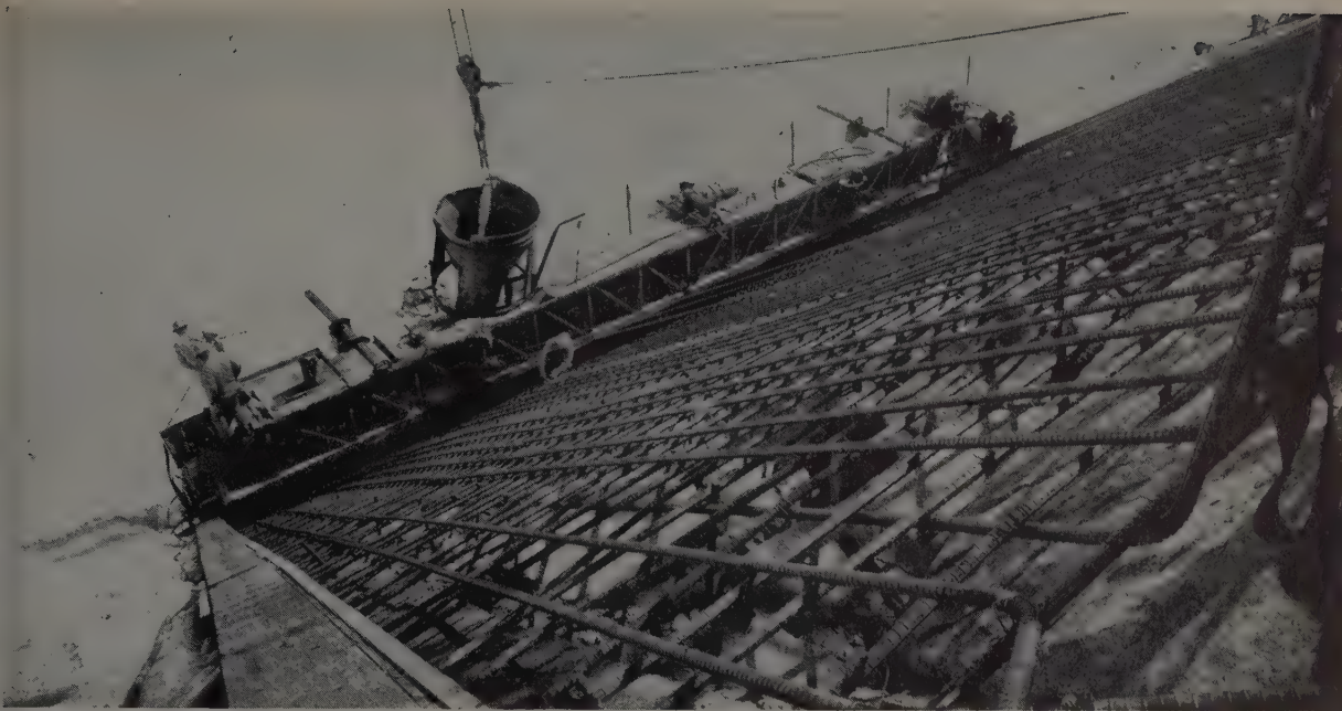
SLIPFORM is sharply outlined against the snow in this view from the dam's crest. The rig rolls on rubber wheels, is pulled up slope by
