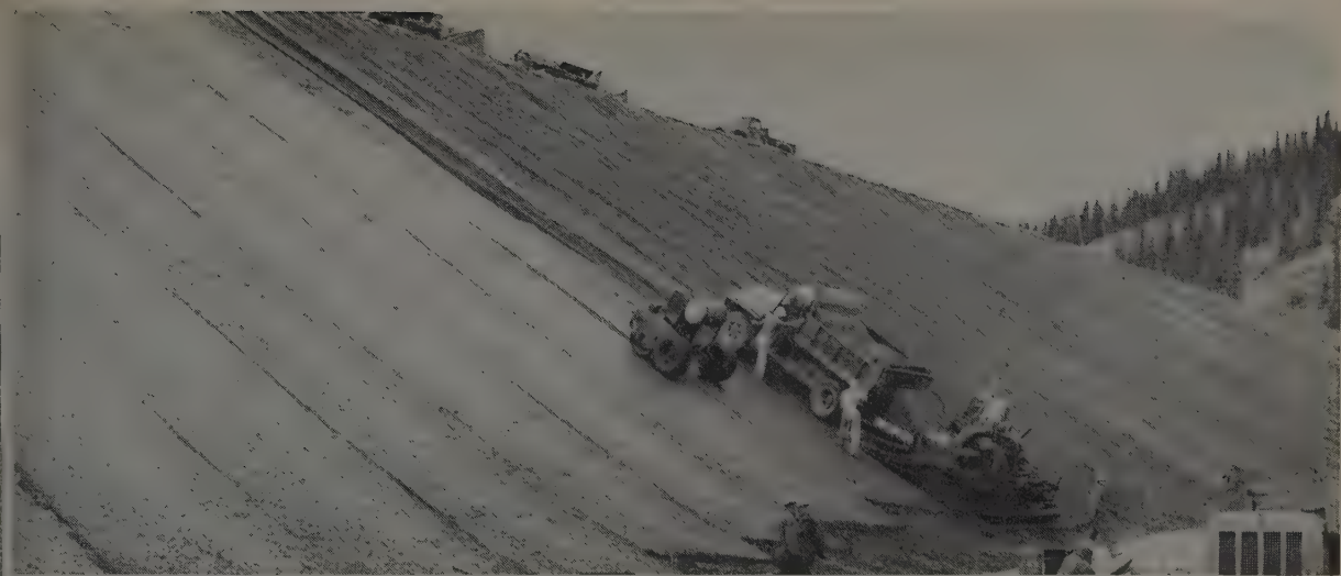
This Barber-Greene Finisher paves the upstream face of the dam. Bulletin showing many other jobs available on request.
