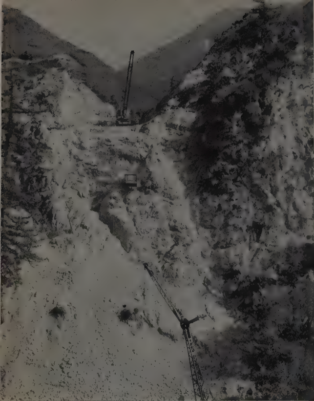
CHARLES MacCLOSKEY CO. is building a 270-ft. concrete arch bridge for Los Angeles County to close the final gap in the new Angeles Crest Highway. With the deck 150 ft. above the canyon floor, the falsework system was the key to the contractor's construction plan.
