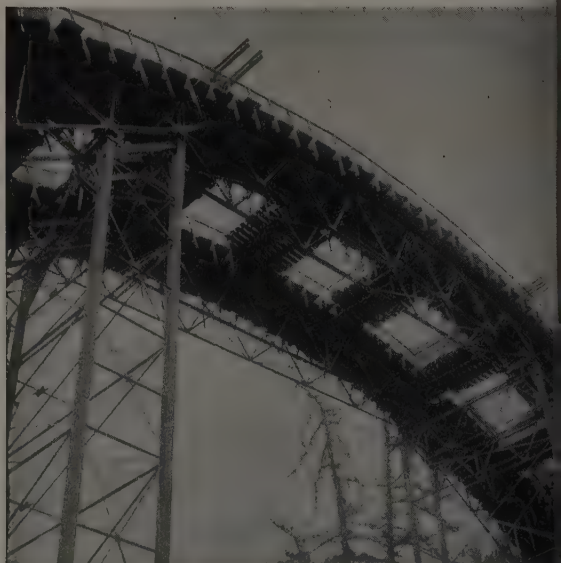
IN POSITION the steel truss falsework was supported on jacks because the contract required the decentering to be simultaneous. At the ends the falsework thrust was carried through the jacks to steel beams directly into the rock of the canyon. A vertical steel plate at the ends of each steel truss was separated from the concrete skew back by 1-in. steel rods to prevent wedging during decentering.
