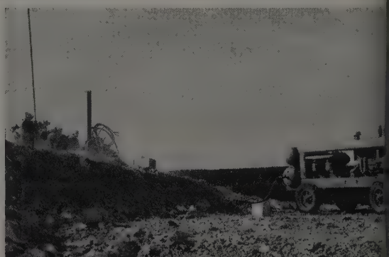
Cat Diesel drives a pneumatic compressor drilling blast holes in rock quarry for materials used on the Freeway job.
