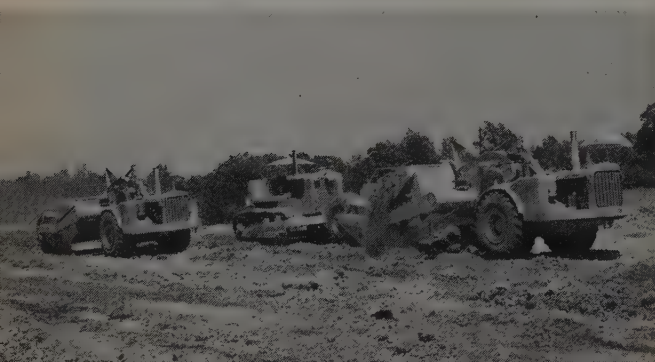
Cat DW21 Wheel Tractors pushloaded by a big D9 work in tough chert conglomerate on Menefee's Freeway job.
