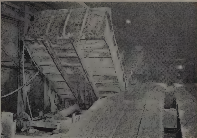
DUMP-TRUCK BED was installed in the tunnel to feed conveyor belt leading 30 ft. to Rex Pumpcrete machine. Dump bed is fed by transit mix trucks from ramp at right.
