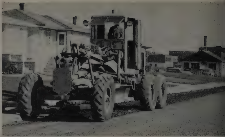
STEP 1—Motor grader rips up the next-to-curb lanes of base material placed a few years before. These parking lanes will be mixed-in-place; the center of the street will be surfaced with 2½ in. of plant mix. The base is crushed and screened gravel. This work was at Regina.
