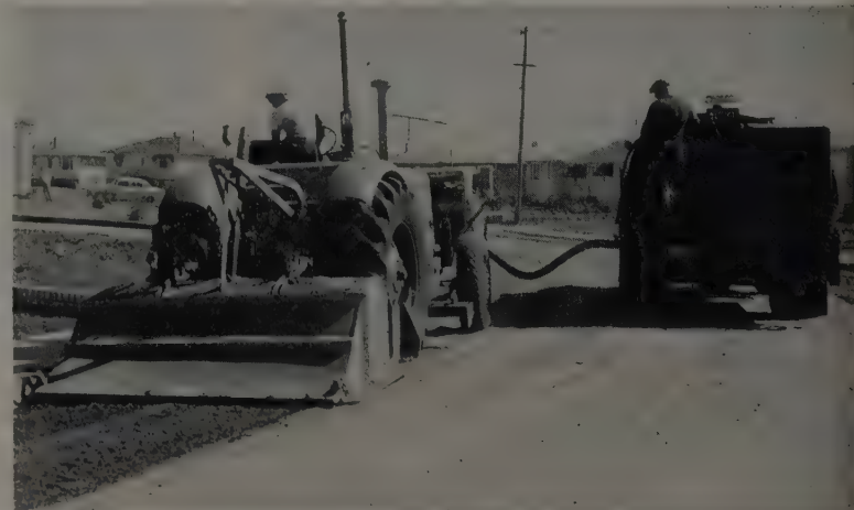
STEP 3—Asphalt emulsion from the distributor is metered by the pump on the Trav-L-Plant. Cost of street work was $128 per 50-ft. lot. Initial mixing takes place when the asphalt is injected into the material under the hood. The asphalt is Type 55-1.
