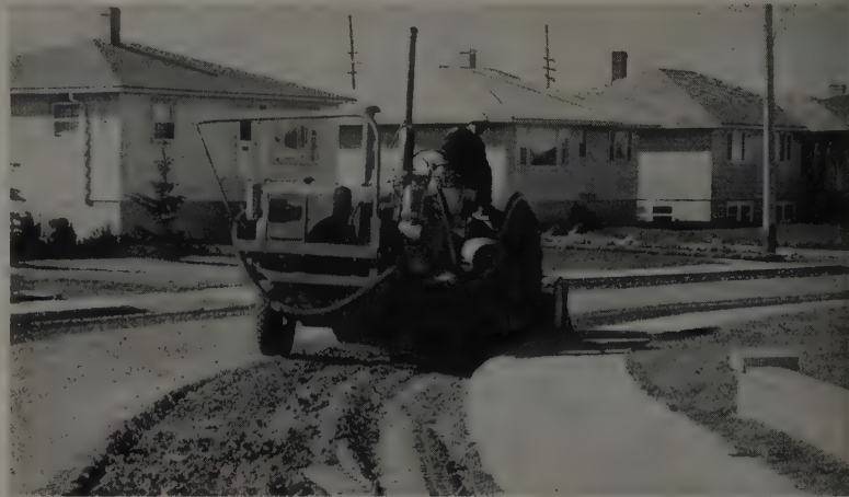
STEP 2—The Seaman-Andwall Trav-L-Plant is making a dry run through the scarified material to break it down and pulverize it prior to adding the oil. This base material had received an oil palliative treatment when placed, a few years before, as a first stage.
