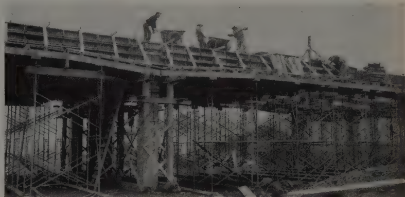
Bridge Forming . . . By using Symons high strength forms, contractor was able to reduce pouring time, use fewer men and cut 100 days off bridge forming job.
