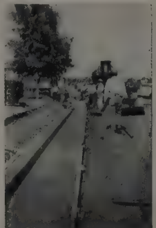
Dotmar paves curb and gutter, over 8' per minute. Total job 14 miles long.
