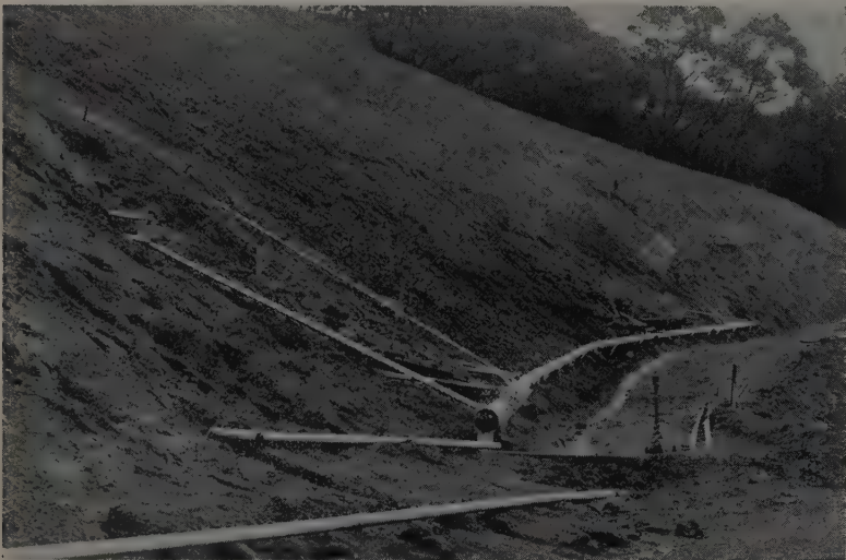
A SYSTEM of horizontal drains flow into an 8-in. collector line which empties into a drop inlet. The 2-in. drain pipe is perforated along 3 of the 4 quarter points.
