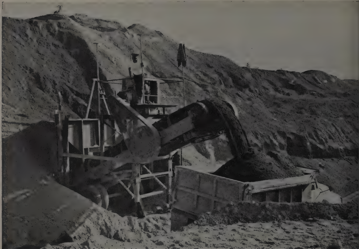
THIS ALBINA 48-in. x 24-ft. G.E. 3-71 diesel-operated Trap-loader fills 12-yd. trucks in 45 sec. The unit is owned and operated by the Donald M. Drake Co. on the Spokane Freeway project and was built under specifications of Donald G. Drake and Ernie Hill of the firm. Albina Engine & Machine Works
