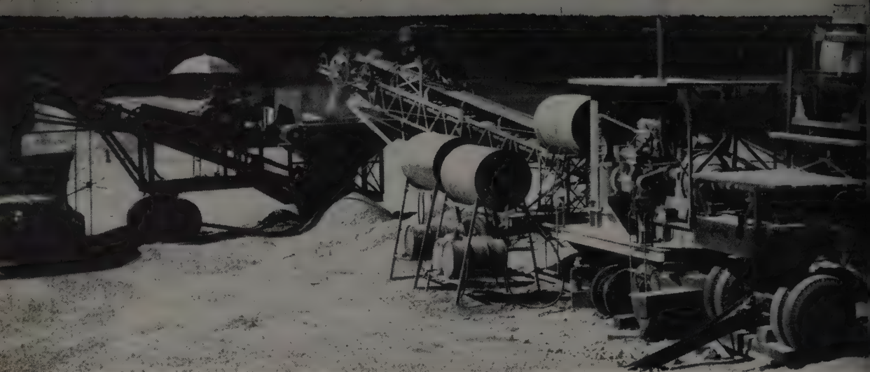
On this portable crushing operation, producing materials for use on a grading and drainage contract for the Missouri Freeway
