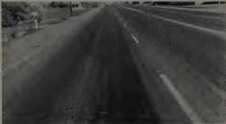
CONSTRUCTION MEN should be aware of the many factors that make up good seal coating practice. On the road shown, use of 200-300 penetration paving asphalt during cool weather resulted in loss of seal coat screenings in the traffic wheel tracks.
