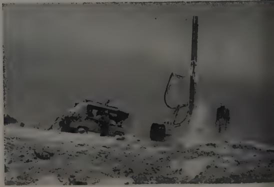
A Dalon wagon drill prepares a shot in a rocky stretch of terrain. The job site included many areas of heavy rock and earth mixtures.
