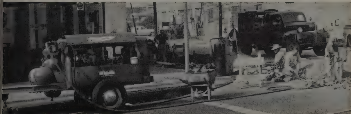
Constant full pressure behind breakers, tampers and other tools keeps them operating at top efficiency, speeds job progress.
