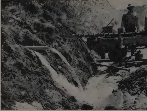
HORIZONTAL DRAIN flowing at a rate of 500,000 gal. per day. An auger flight rig is shown at work in the background.
