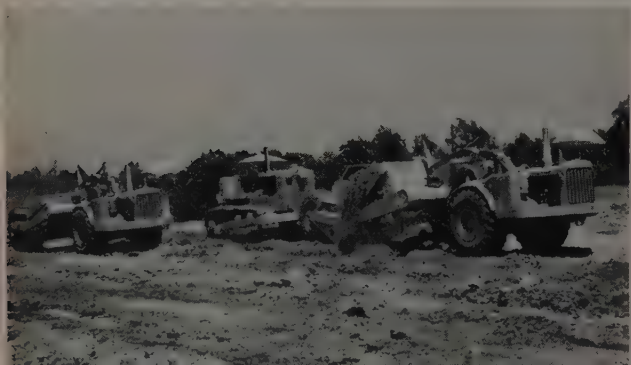
Cat DW21 Wheel Tractors pushloaded by a big D9 work in tough chert conglomerate on Menefee's Freeway job.
