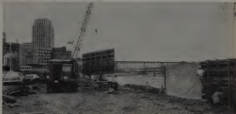
Retaining Wall Forming . . . Symons wide panel forms made up in sections of 10' x 24' and 15' x 24' used to pour 2,400 foot long retaining wall.
