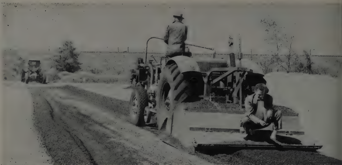
IN Missoula, Mont., when a small amount of mix was needed it was prepared on this off-street mixing table. Hot bitumen was added to
