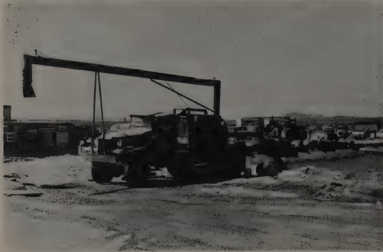
WATER TRUCKS were loaded from truck-mounted pumps capable of discharging 3,000 gpm. Temporary reservoirs fed by pipeline were spaced every 2 mi. along length of project.
