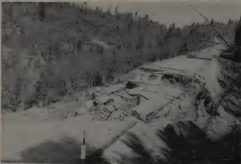
SLIPOUT OF a highway fill in Trinity County. The corrective treatment to be applied will include the installation of a system of horizontal drains.
