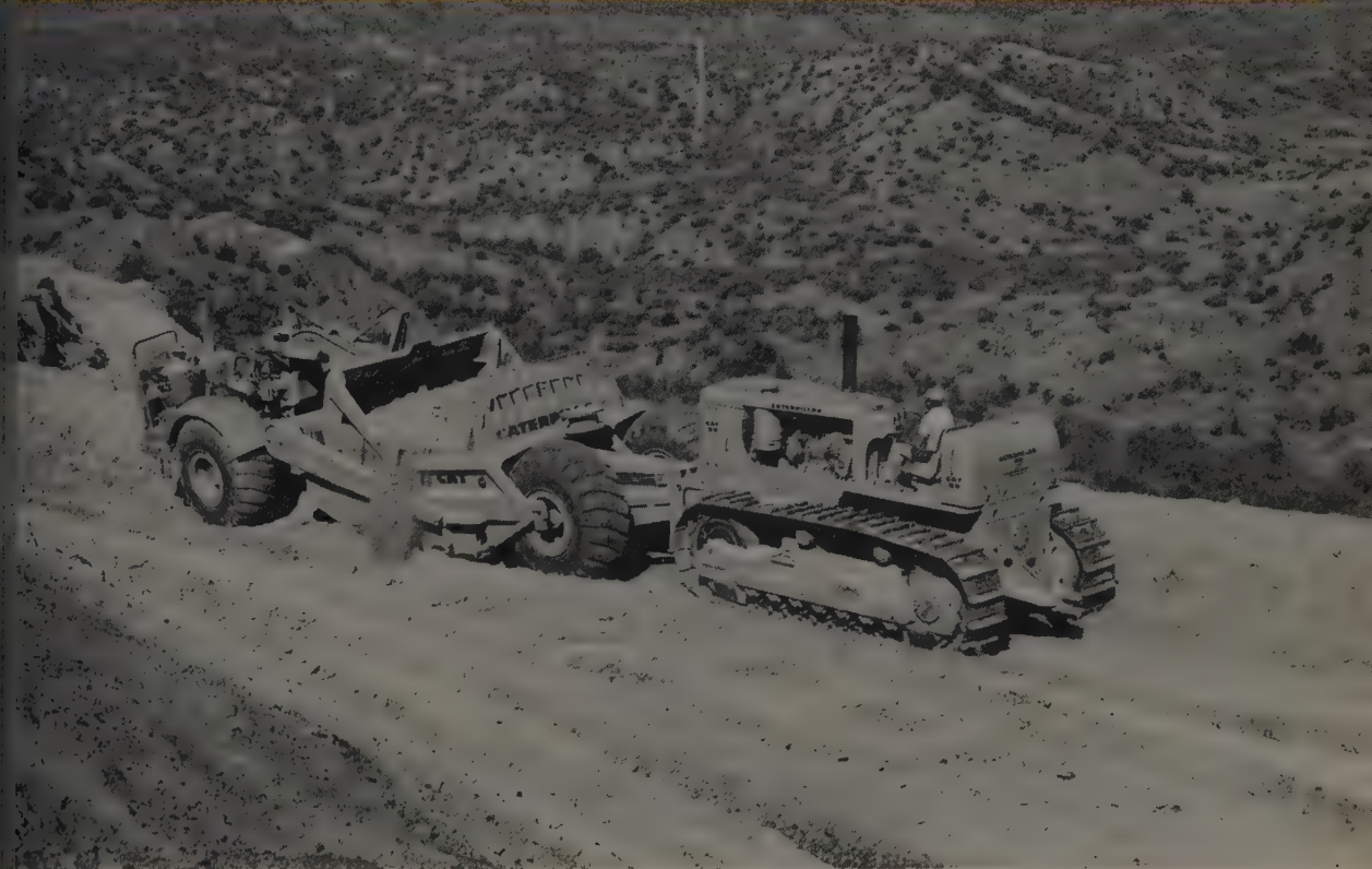
Unbeatable road building team by Caterpillar: DW21 Tractor with No. 470 LOW/BOWL Scraper is pushloaded by D9 Tractor
