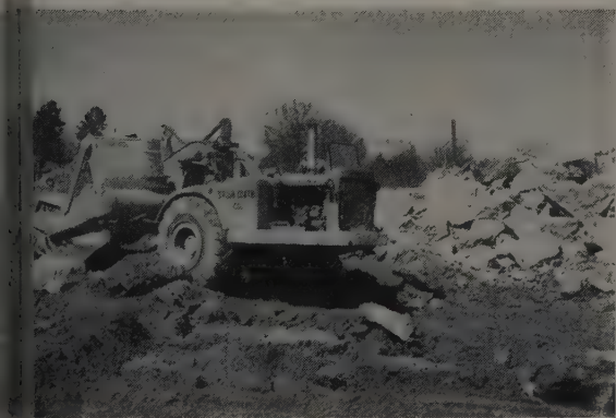
Let a Cat DW21 team up with a model 470 scraper to clear a rocky patch of ground.
