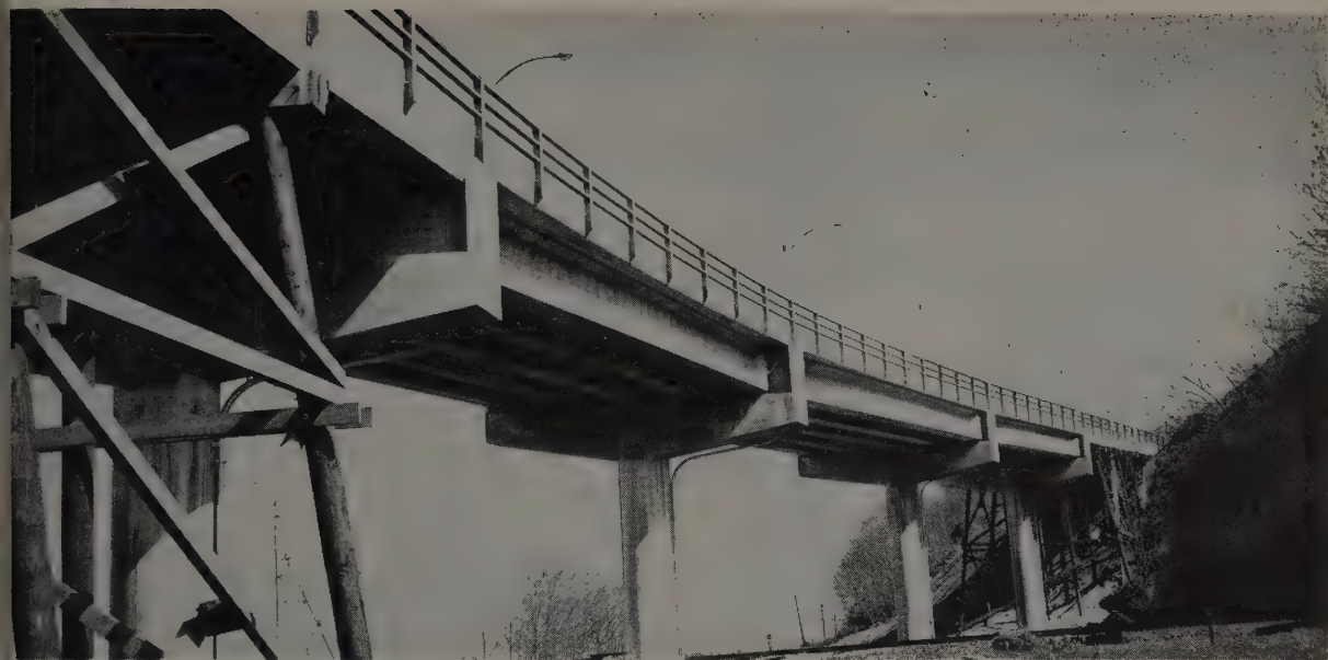
SUPPORTED ON 5-ft. diameter column shafts the three main spans are 80-100-80 ft. Center span crosses present and future railroad
