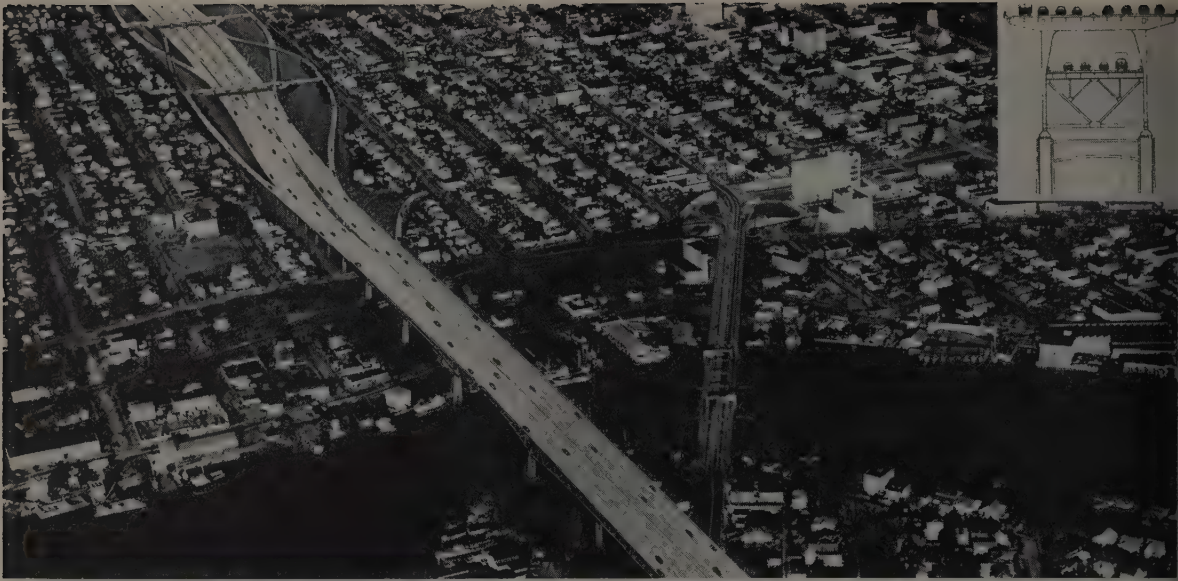
SKETCH OF THE proposed bridge to carry the Seattle Freeway over the Lake Washington Ship Canal. The two-deck design (see upper right) will accommodate 12 lanes, with the 4 lanes of the lower deck
