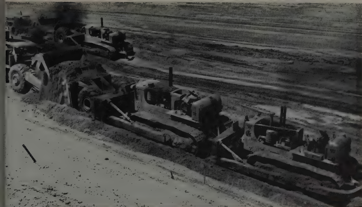
TANDEM PUSHING was done whenever possible to keep loading time at a minimum. In photo a D9 and D8 quickly give a Euc scraper
