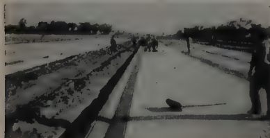
Dotmar Paver with extensions paves integral gutter, curb and sidewalk.
