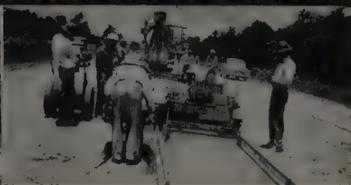
Dotmar with extensions paves state highway median strip.
