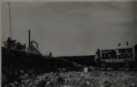
Cat Diesel drives a pneumatic compressor drilling blast holes in rock quarry for materials used on the Freeway job.
