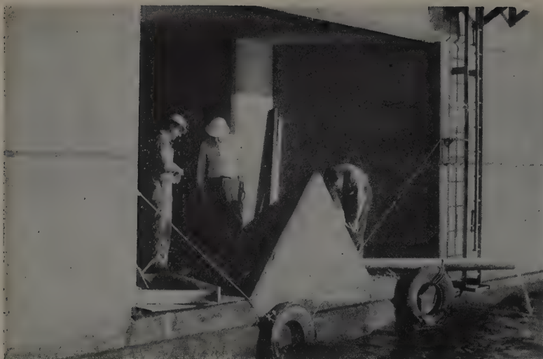
SPLITTER BLOCKS at the discharge end of the lower conduits deflect the water and throw it up and away from the toe of the dam. The blocks are subjected to great impact and abrasion. Epoxy adhesive was brushed on both upstream faces.
