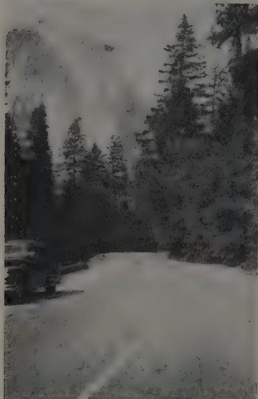
1933—Heavy-duty pavements of Bitumuls Penetration Macadam.
