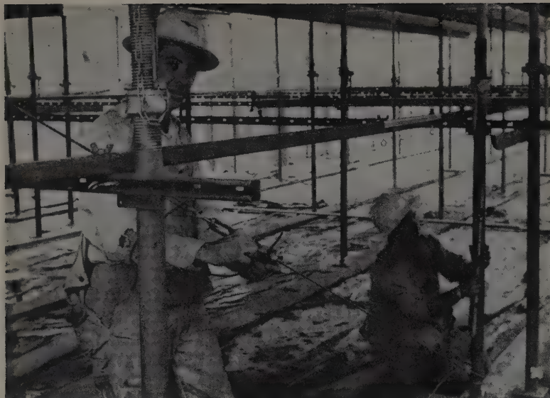
DIAGONAL WIRE with turnbuckle is added about every 30 ft. to provide sway bracing. At right, shore is checked with level for plumbness as turnbuckle is tightened.
