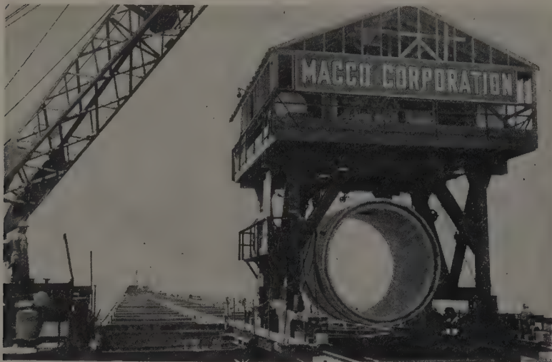
GANTRY CRANE ON tracks was used by Macco Corp. to place precast concrete pipe sections on ocean floor for submarine cooling water lines. Temporary timber trestle was 2,000 ft. long.
