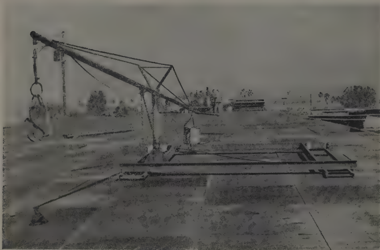
HOME-MADE RIG which runs on two sections of conveyor rollers is used by contractor to handle purlins and panels on the roof. Roof is erected entirely from the top.
