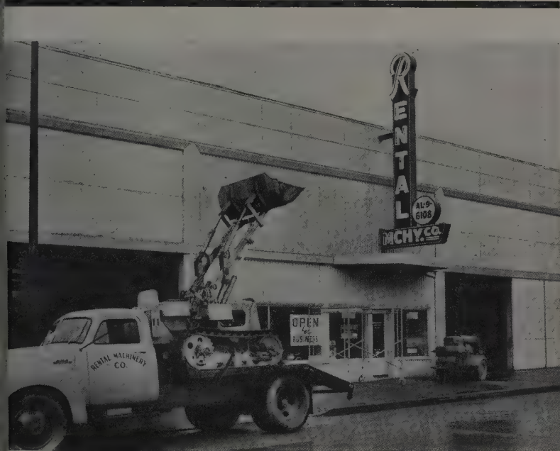
NEW BRANCH office and plant recently opened at 2411 Hewitt Ave., Everett, Wash., by Rental Machinery Co., a division of A. H. Cox & Co., of Seattle. Under the management of William R. "Bill" Snyder, the new outlet is set up to handle both equipment rentals and new equipment sales.
