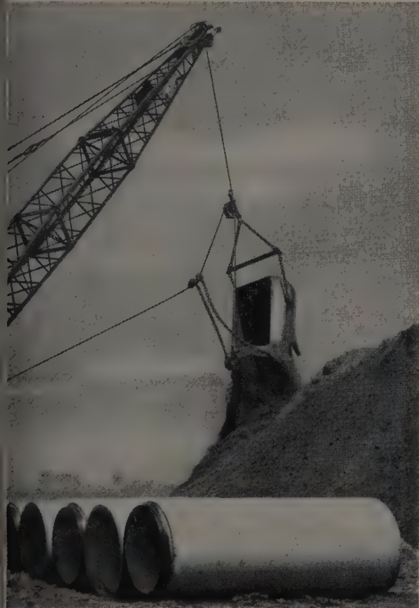
This Bucyrus-Erie 1 1/4-cu. yd. medium-duty bucket is on a 30-B dragline excavating for a 30-in. sewer line.
