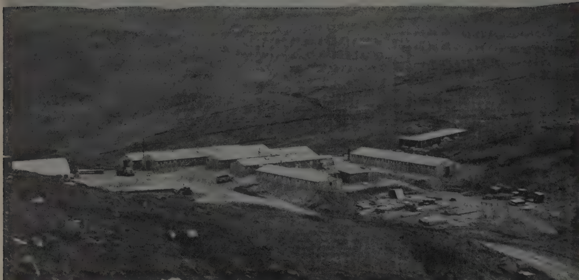
CAMP SITE was located behind the hills in an effort to escape some of the fury of the winds. In spite of buildings designed to cope with
