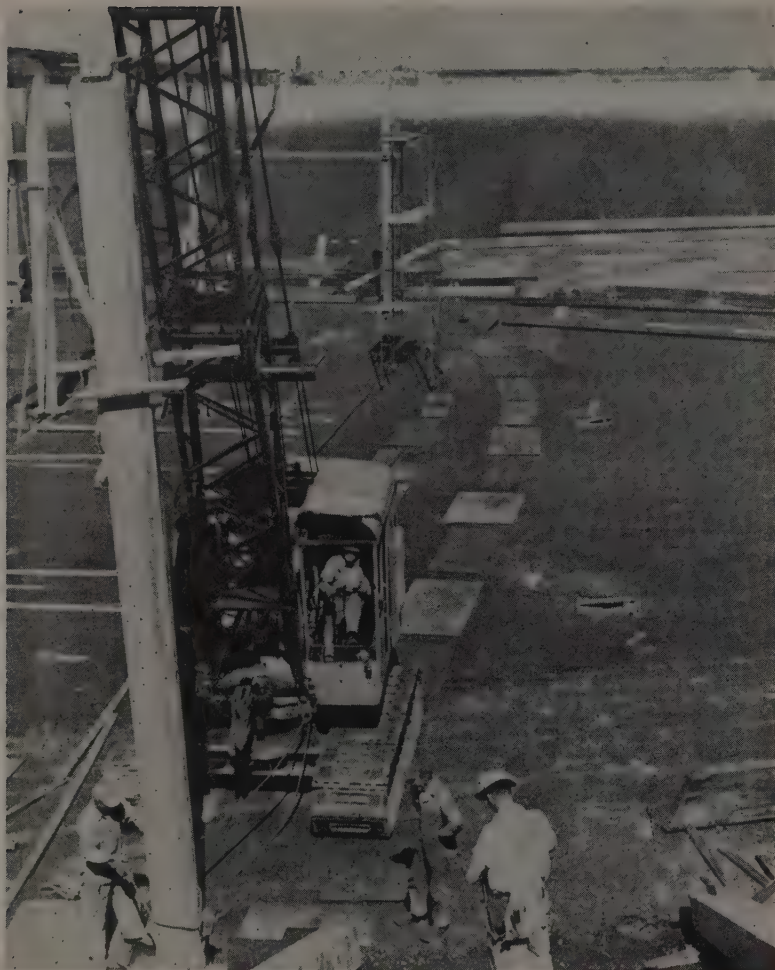
PRECAST COLUMNS are set in place before prefab asphalt panels are laid. Notice how crane moves over porous asphalt layer on plywood without causing damage.
