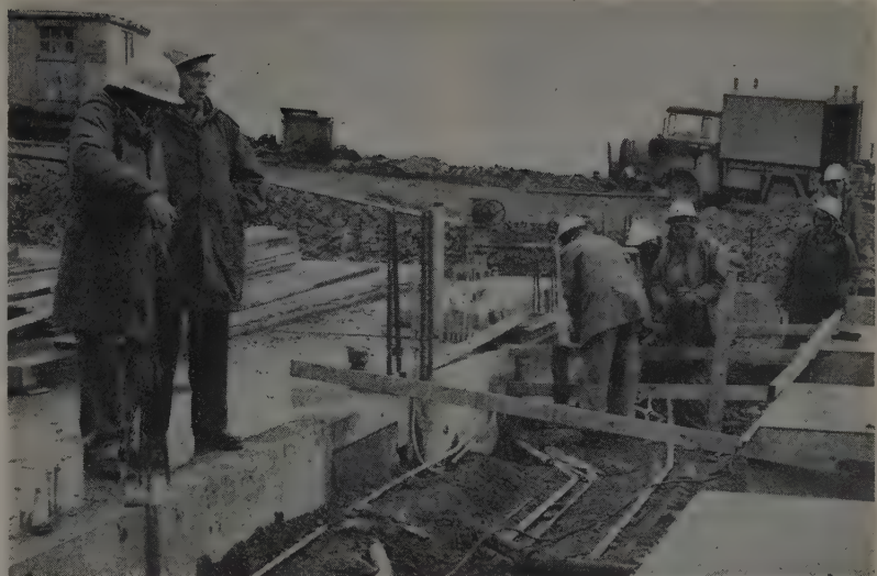
WHEN WIND AND weather were at least reasonable, the actual construction operations were not particularly difficult. Crew is building foundation for generators.
