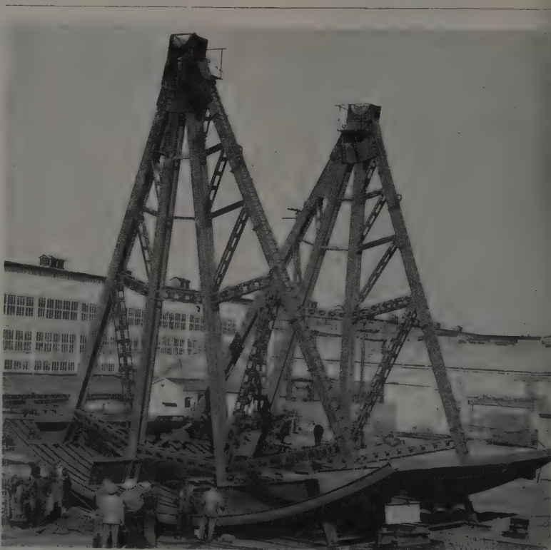
GATES PRE-ASSEMBLED FOR BROWNLEE DAM
