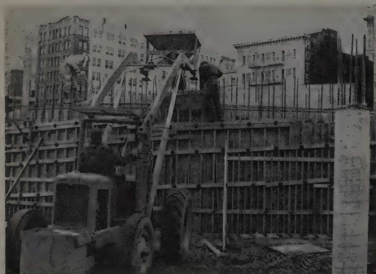
AN ECONMOBILE with concrete bucket attachment is used to carry concrete from transit trucks to walls and columns. Wall shown is curved, ruling out prefab forms. Column at right is one of 408 to be formed by Sonotubes 8 ft. high.
