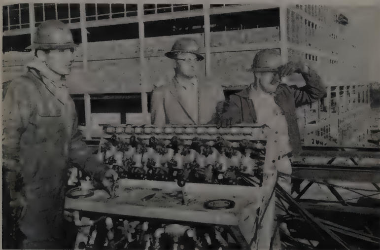
SUPERVISING the unusual lift are (l. to r.) Otto Nass, Vagtborg hoisting engineer operating the console, Carl Fornstrom, Vagtborg vice president, and Louis Hack, American Bridge superintendent.
