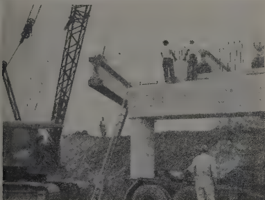
Illinois Toll Highway
