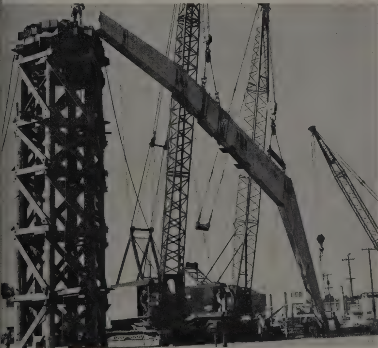
LIFTING required careful teamwork by three crane operators to compensate for the shifting weight as the arches were rotated upward from the ground to final position.
