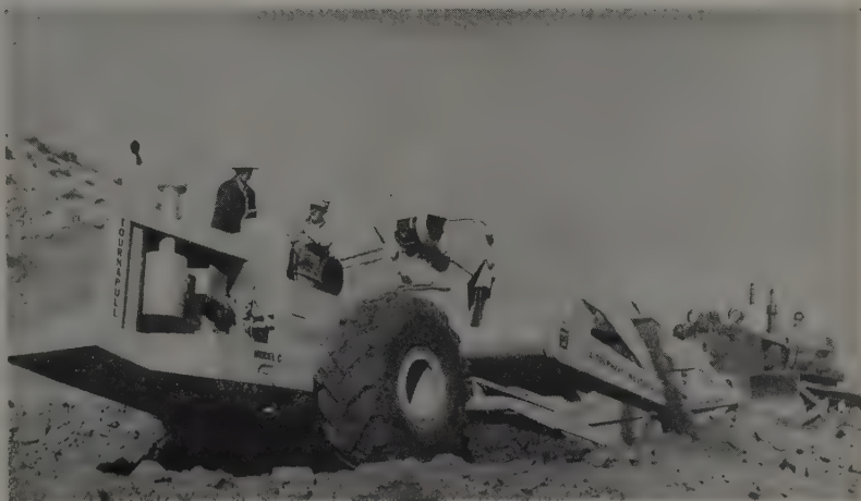
TEAMWORK ON pusher-loading is practiced by two students under the watchful eye of the instructor. Safety practices are emphasized on operations, and Red Cross training is given.
