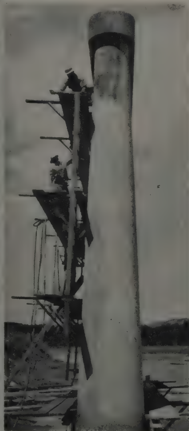
CONCRETE FOR the piers was handled in buckets by Lorain and Northwest cranes. Plywood forms were built on the job.
