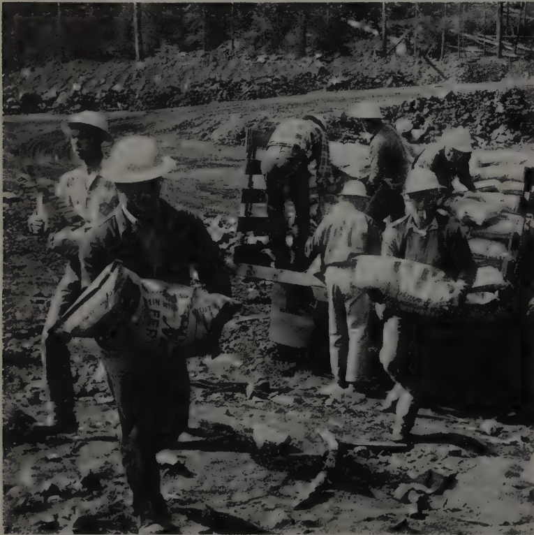
HANDLING NITRATE requires no costly safety precautions. The hazard from sparks or cigarettes is almost nonexistent and the danger from shock is eliminated. Shipping rates are low. It can be stored in any dry place—no bulletproof magazines needed.
