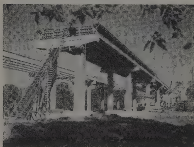
Illinois Toll Highway
