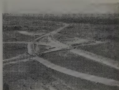
Illinois Toll Highway
