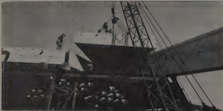
ROOF PANELS are lifted at three points. The lower two connections are made through chain hoists which are operated by a man riding on the panel to give it the proper pitch.
