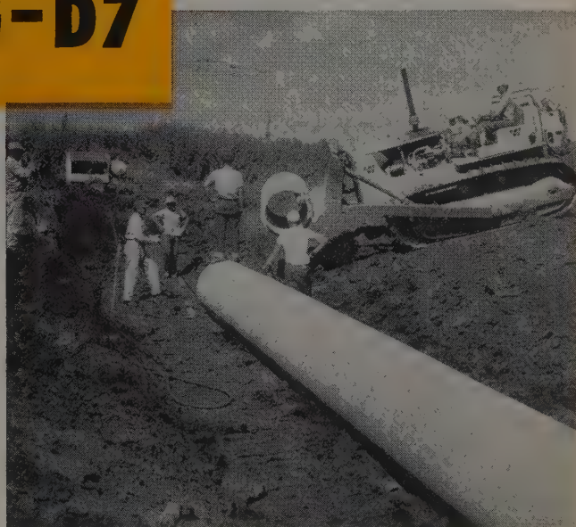
Final step, before covering and cleaning up, is laying the concrete pipe itself.
