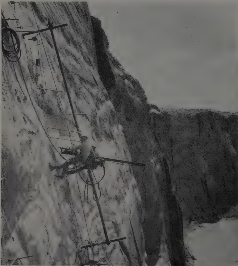
SPECIAL METHODS were devised for rock drilling on the face of the cliff during abutment excavation for the steel arch bridge. A Thor drill was mounted on a vertical bar.
