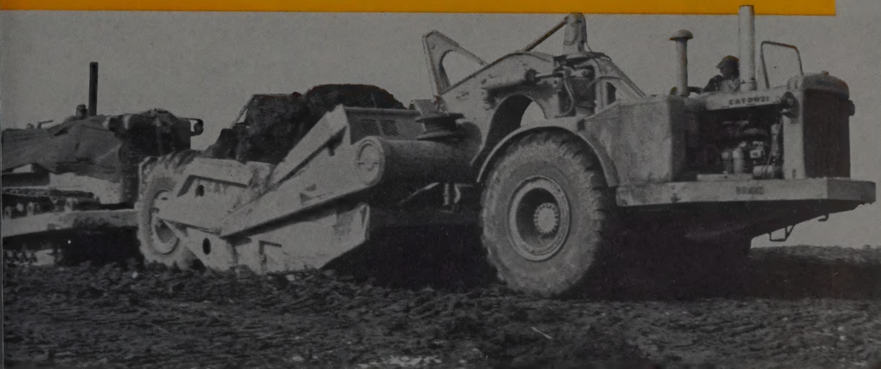
DW21, owned by McCarthy, Mass, Dillon, is pushloaded by a D9 on a section of the Illinois Toll Highway near Elgin. LOWBOWL design, fast cycle time make DW21-No. 470 rig a favorite on this project.
