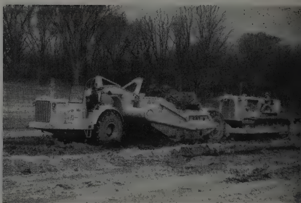
material. In the same, a D9, with more hp. and more weight easily tops off a capacity load to increase the productivity of the haul unit.
