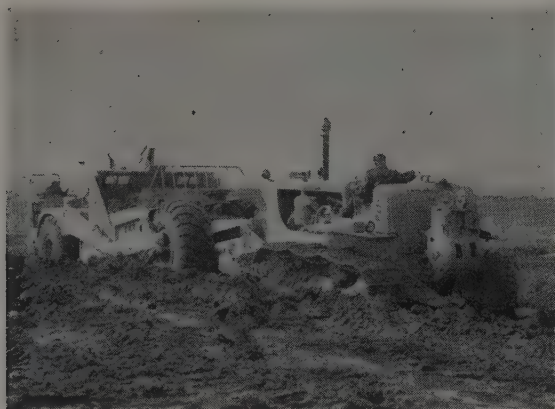
THE "STANDARD work-horse," a Caterpillar D8 tractor, labors to load the DW21—No. 470 (18 cu. yd. struck capacity) in extremely heavy
