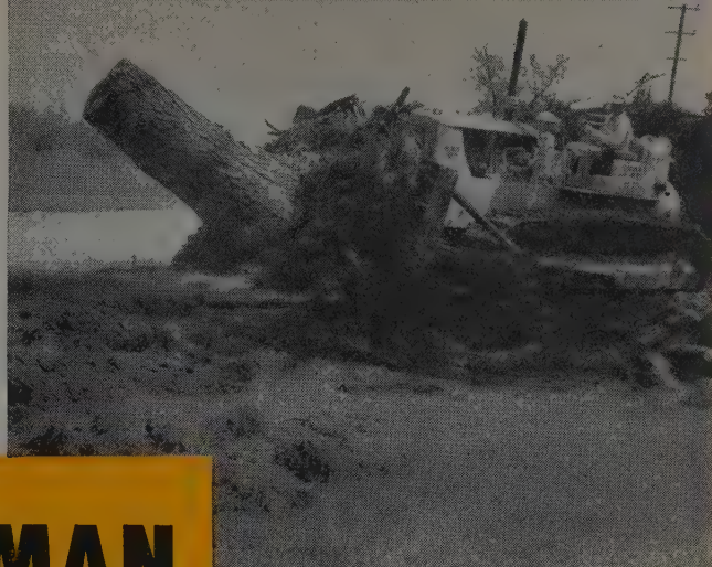
Along highway's right of way, heavy stump with extensive root formation is 'dozed out.
