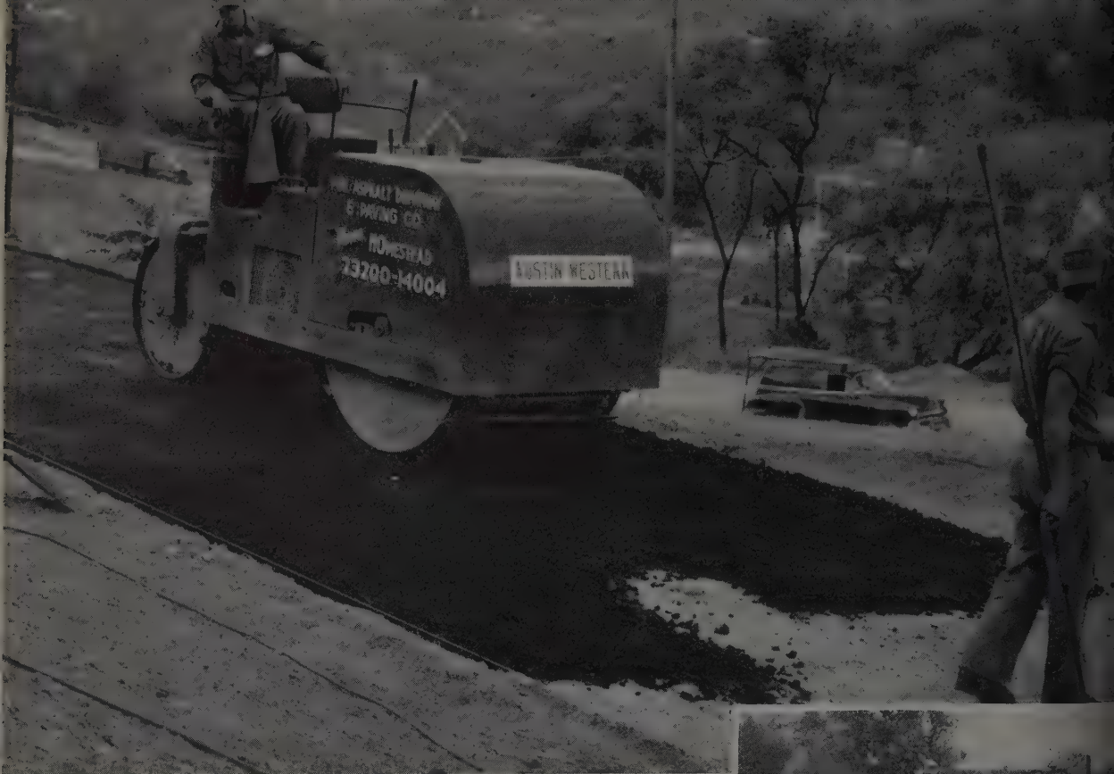
A-W portable tandem roller, owned by Pittsburgh Asphalt Driveway & Paving Co., rolling binder layer of asphalt.
