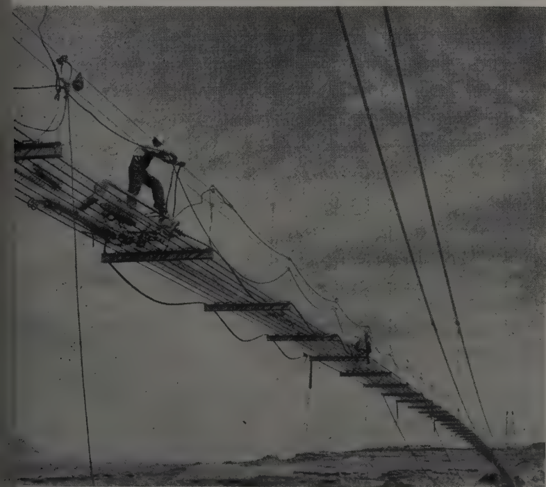
RE MESH footbridge is located 1,500 ft. upstream from the dam. The bridge is 1,280 ft. long and 700 ft. above the water, hung between two 100-ft. high steel towers.
