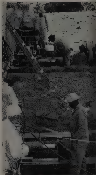
RAMS were mounted on each of the four tracks. The total 400-ton rated capacity of the jacks moved the building at a rate of 5 ft. per hour. Rams pushed against cleats clamped to the track beams.
