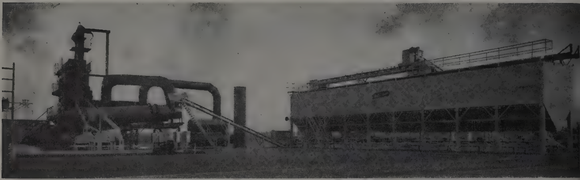
For an asphalt plant to function properly, the crew and inspector must be fully aware of the factors affecting each component.
