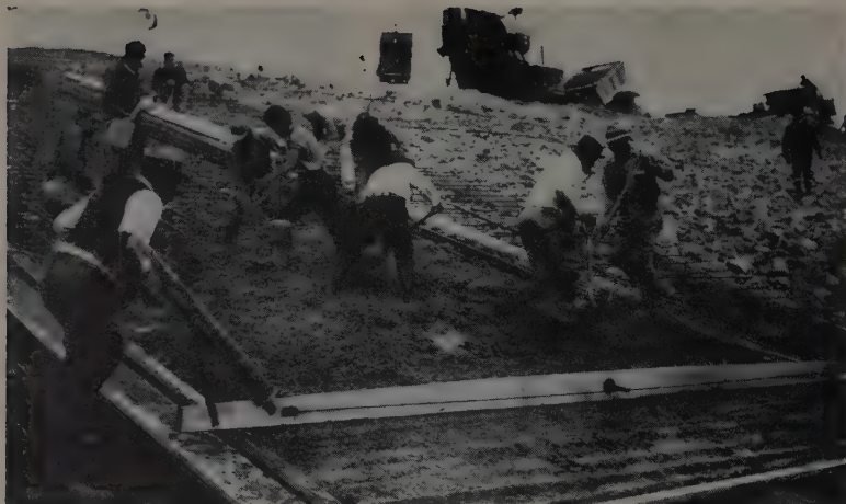
1938 Hand labor was used twenty years ago to spread, screed, and finish concrete on the slope. Griffith Construction Co. won the first contract.
