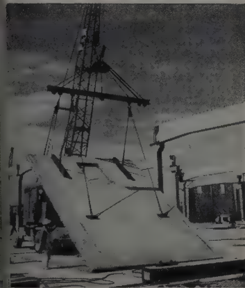
C—LOAD STILL IN TENSION. Superior's System provides necessary strength and saves omission of reinforcing steel which is used only for stresses which occur at time of lift.
