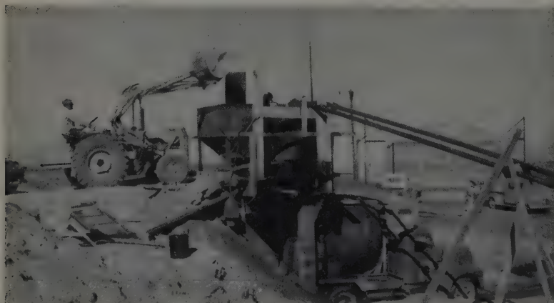
BATCHING HOPPER is being filled, and the mixer truck is taking its load. Lines from the right deliver the emulsion. To the 6,000-lb. charge of aggregate was added 150 gal. of SS-1 and 110 gal. of water.
