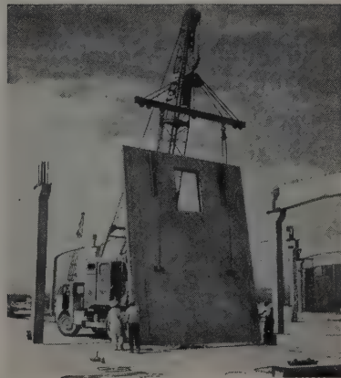
D—AS LOAD TRANSFERS TO SHEAR, Superior Pick Up Inserts, Bolts and Stress Equalizer Beams resist the forces which occur at this time.
