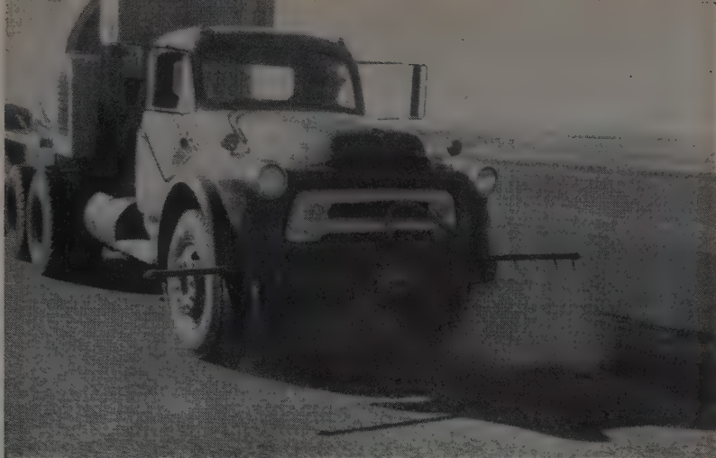
MOISTENING the old surface ahead of the spreader represents a good example of contractor ingenuity. The water tank on the truck was connected to a spray bar with weed sprayer type nozzles mounted on the front bumper. This fogged the surface at exactly the right place and time.
