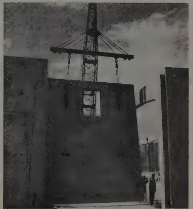
E—CRANE MOVES PANEL towards final position. Simplified pickup speeds up crane operation considerably and provides faster and safer control.
