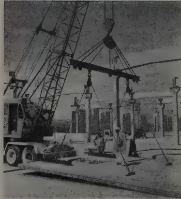
A—START OF LIFTING OPERATION. Note Superior Stress Equalizer Beams at top position and regular Superior Lifting Angles at bottom.
