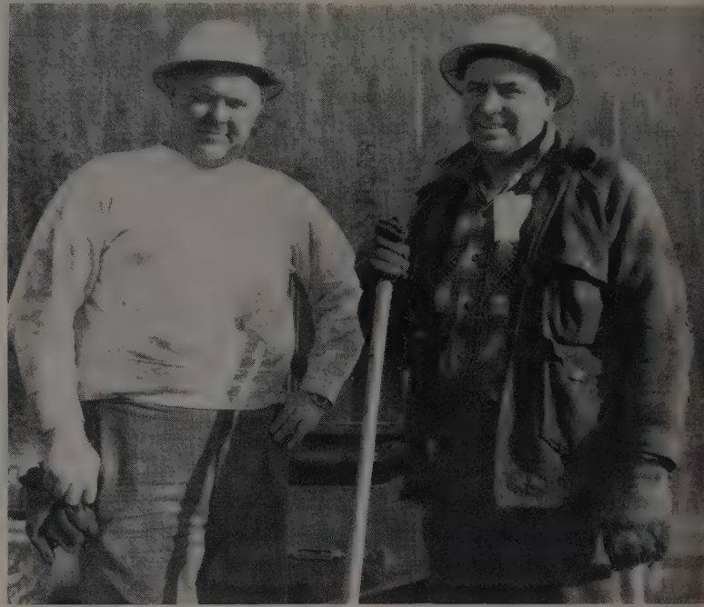
KEY MEN on Washington Asphalt Co.'s paving job at Snoqualmie Pass near Seattle, Wash., Dick Jackson, paving foreman, and Glen Howard, plant foreman, took full advantage of unusually good late fall weather at that altitude to get in some extra work before winter close-down.
