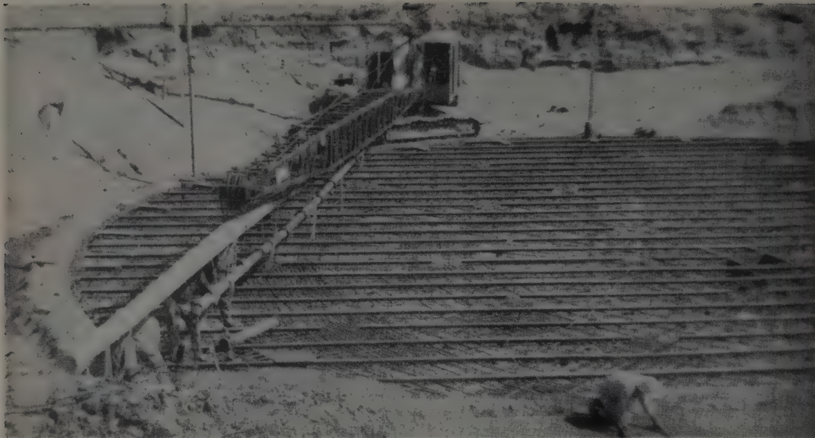
THIS "RUBE GOLDBERG" arrangement was improvised by Macri Construction Co. to place concrete over a 100-ft. diameter area. The pole extended the Link-Belt boom and the Pumpcrete line was shortened
