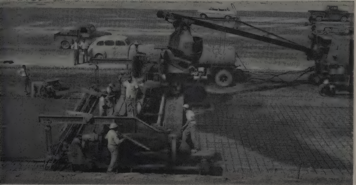
THE FIRST slip-form concrete paver to be mounted on crawlers, a Giffith & Zimmerman machine, enabled Griffith Co., the contractor,
