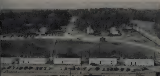
These 16- by 60-foot Armco Buildings in the foreground have been dismantled, moved and re-erected twice. First time they were moved 90 miles; the second time it was 140 miles.
