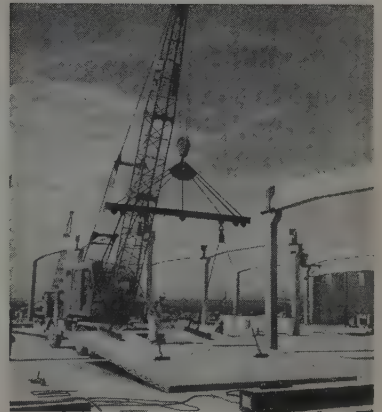
B—SIMPLIFIED RIGGING is an important advantage of Superior System as only two running lines are needed. The 27 1/2' high panel shows virtually no deflection during pickup.
