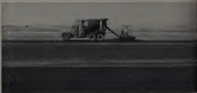
WIDTH of slurry sealing operations on an airport runway, as compared to a road job, is shown by the distance to the mixer truck and spreader. This seal will face a severe test during the Montana winter and spring seasons.
