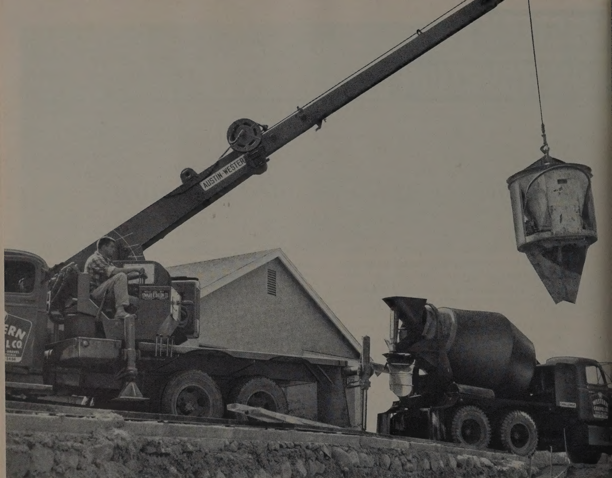
Truck-mounted A-W Hydraulic Crane Equipped with ½-yd. concrete bucket shown working on job for Western Gravel Co.
