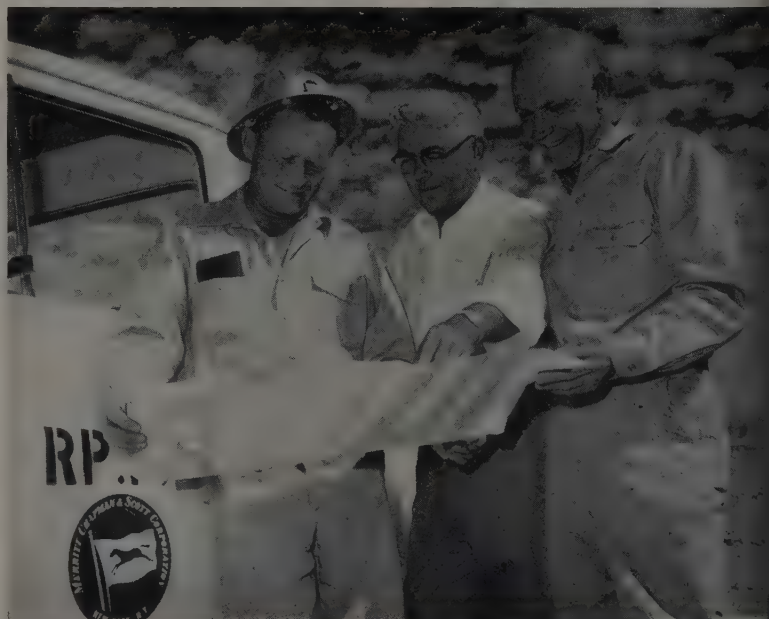
FORREST JONES , GENERAL SUPERINTENDENT for Merritt-Chapman & Scott Corp. , prime contractor for construction of Glen Canyon Dam , goes over plans with Glen Roper (right), rigging superintendent, and Donovan "Whitey" Candaux , carpenter superintendent. A key structure of the Colorado River Storage Project Glen Canyon will be the second highest dam in the United States.
