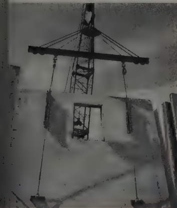
C—LOAD STILL IN TENSION. Superior's System provides necessary strength and saves omission of reinforcing steel which is used only for stresses which occur at time of lift.
