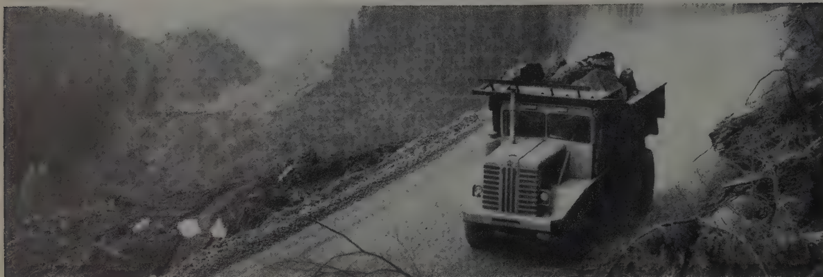
RUGGED TERRAIN of Western mountains means tough hauling when a railroad has to be moved out of a dam site. Slate and Hall of Portland have a 6-mi. contract for part of the relocation of the Northern Pacific at the Eagle Gorge Dam. They are using a fleet of six International Harvester Model 95 Payhaulers on a hazardous 2 1/2-mi. haul
