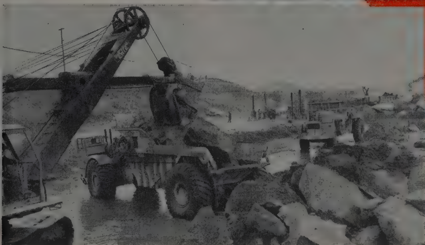
Two 32-ton Yuba Movalls replaced five conventional heavy-duty end dumps on a 5 mile section of Massachusetts Turnpike involving movement of 2,725,000 yards of rock and earth. These are powered by Cat DW-21s.
