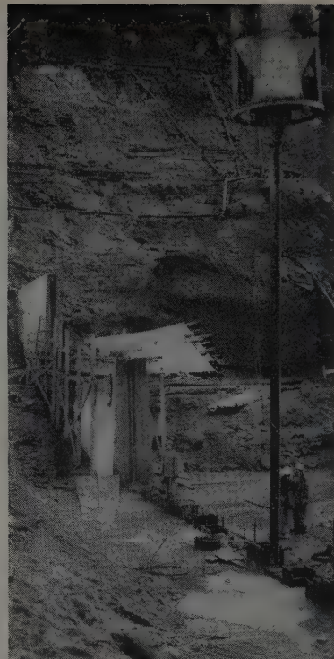
H-BEAMS driven to bedrock interlock to form cutoff wall, which was filled with concrete by bucket with long spout, as shown. A concrete wall about 30 ft. high extends this cutoff into the impervious fill.
