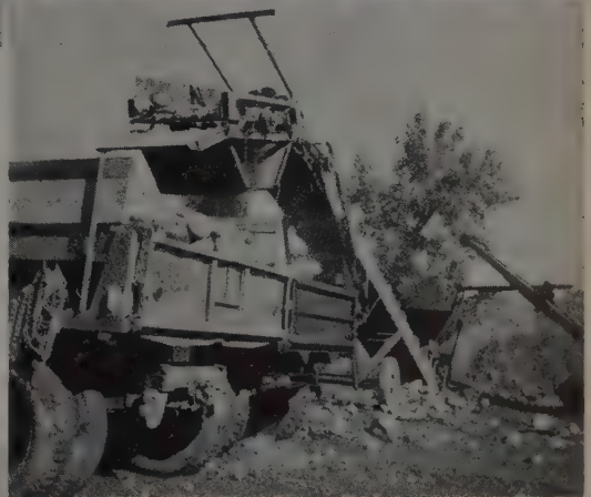
(Above) Shovel loads hopper on this 40'x24" Model 202 Conveyor with 7'x42" screen on scalping job in Jefferson County, Colorado.
