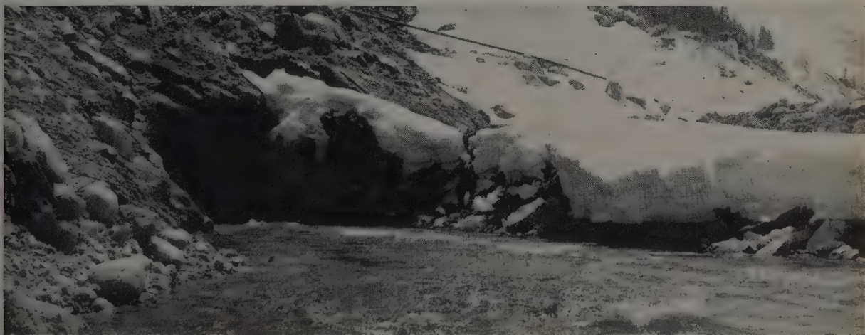
1100-ft. long diversion tunnel for Courtright Dam. This was driven with two Gardner-Denver SF93 drifters and one DH123 drill mounted on an aluminum guide.
