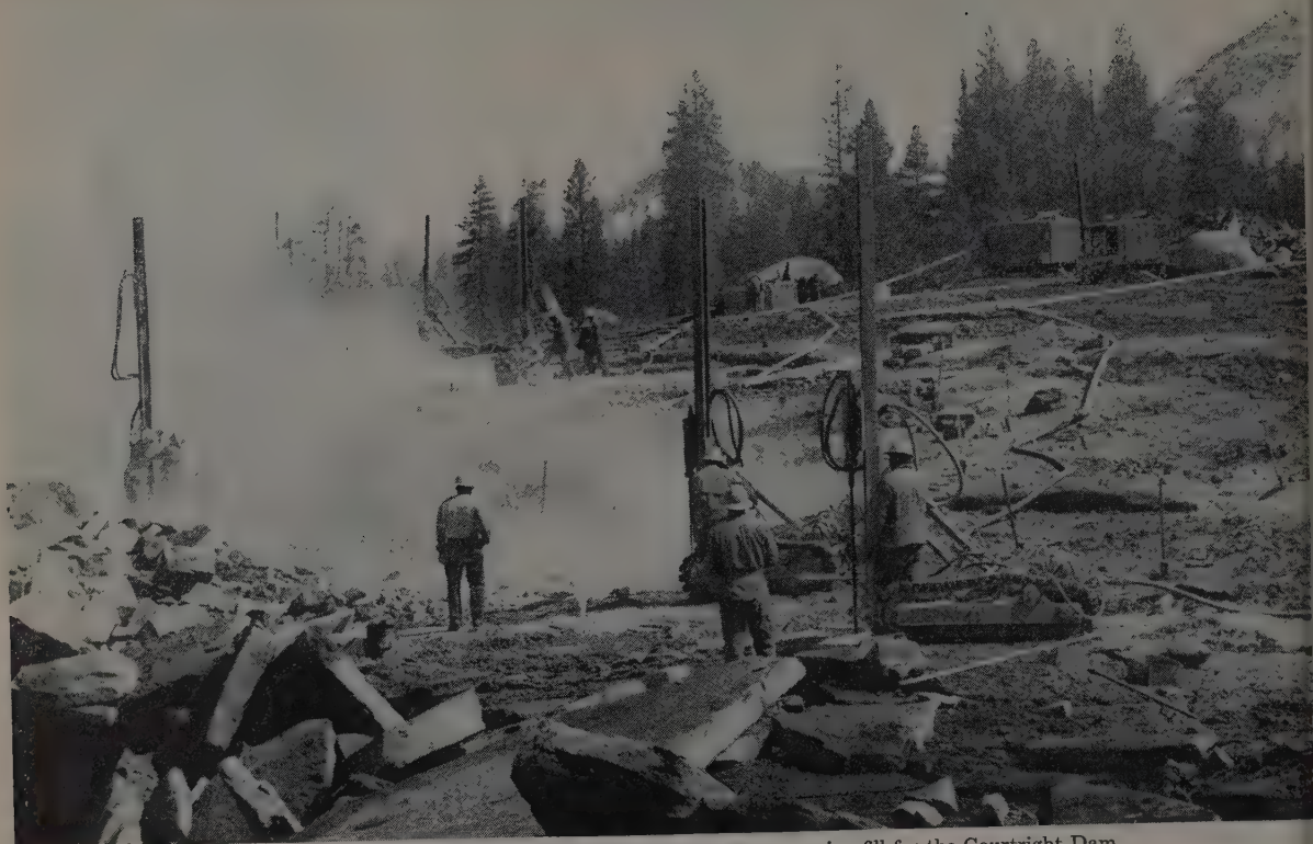
Gardner-Denver "Air Trac" drills and portable compressors quarrying fill for the Courtright Dam.
