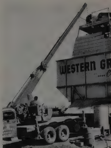
HERE'S A SHOT of an Austin-Western hydraulic crane owned by Western Gravel Co. of Campbell, Calif. The rig has an 18-ft. extensible boom and a 17-ft. manual extension. The machine's versatility enables it to perform a great number of tasks around the firm's gravel plant and two batch plants. On one chore, changing the screen in the gravel plant, saved 75 % of the manhours.
