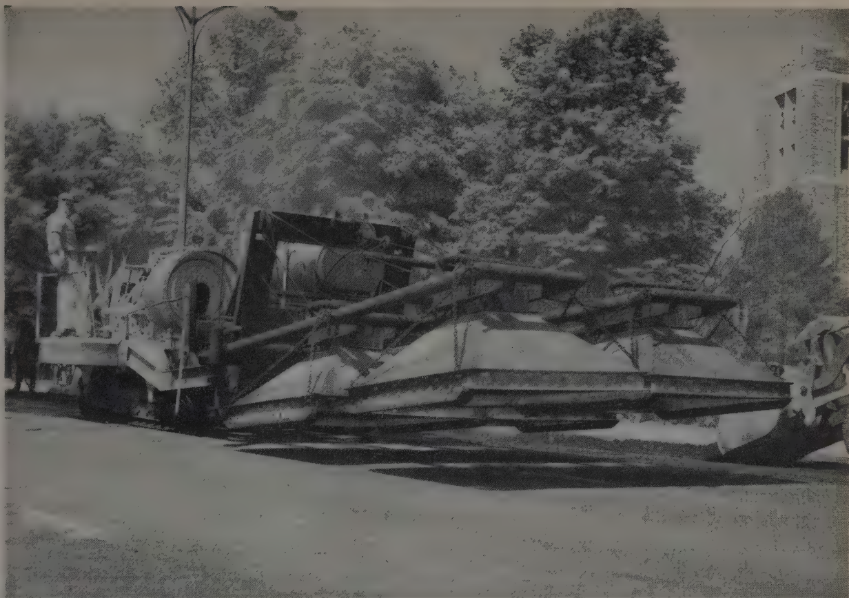
Giant Spears Heater-Planer burns off approximately 1,000 square feet of asphalt per hour.
