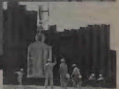
Gar-Bro Concrete Bucket is lowered to dumping position. Note: Crane Hook is absolutely safe; cannot open under load.
