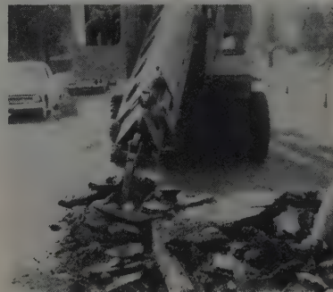
PEOPLE are still thinking of new ways to use the Gradall, Warner & Swasey's versatile rig. The one shown is being used by McRae Bros. of Seattle to break up pavement around old streetcar rails. The end of the telescopic boom is fitted with a ripper tooth. Gradall distributor in the Northwest is Columbia Equipment Co.
