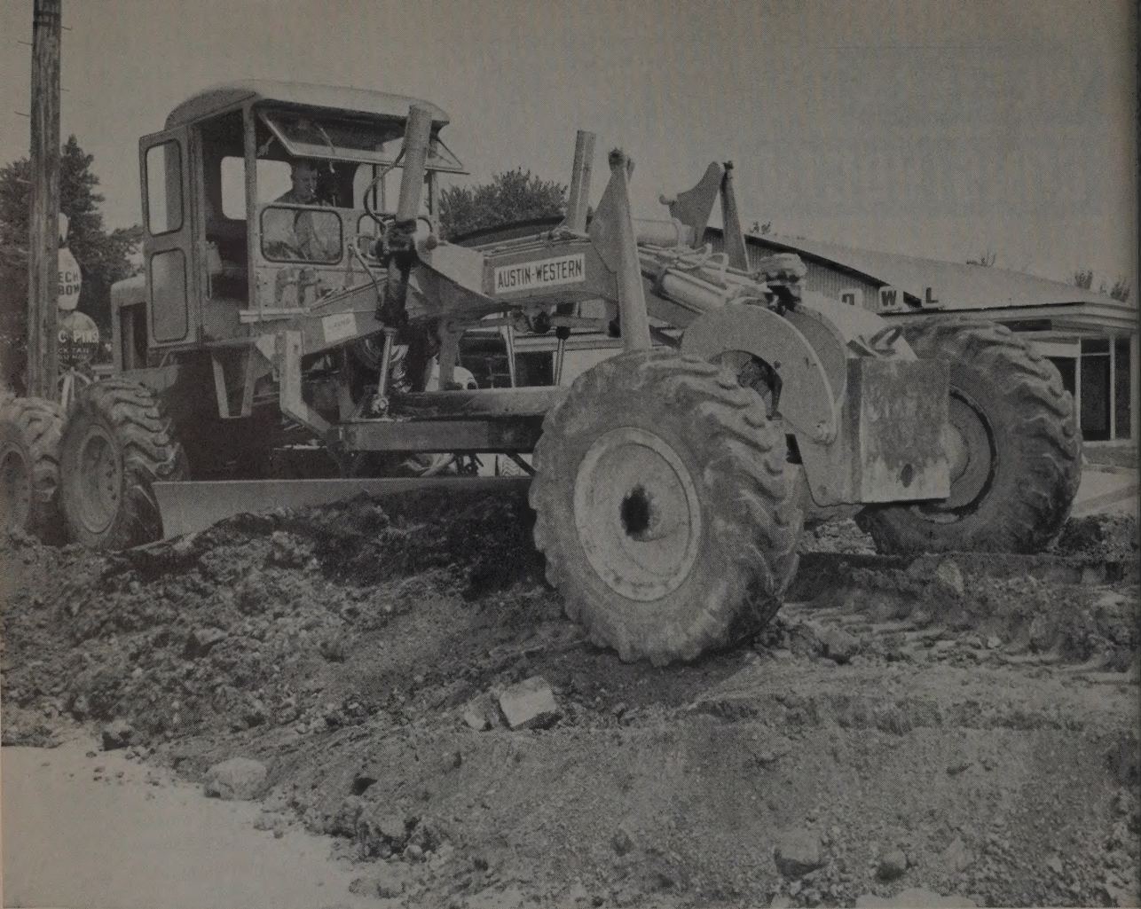
Vernon (Stub) Faber doing a rough grading operation on a highway widening project inside the city limits of Milwaukee, Wis. The machine is an Austin-Western Super 99 with 6-wheel drive and 6-wheel steer.
