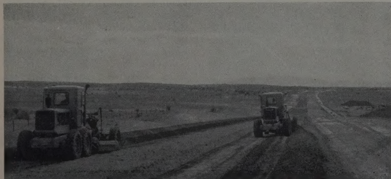
CRUSHED ROCK is low in fines, and is blended with sand by two graders. Moisture is added to bring the material up to the 8% optimum. Specifications call for compacting with 50-ton pneumatics.
