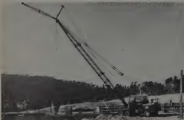
A MARION Type 35-M 25-ton truck crane was used with advantage by Stolte, Inc., on a project for Corps of Engineers near Monterey, Calif. It is shown with a 60-ft. boom and 20-ft. jib. A 1-cu. yd. clamshell was used for sand.
