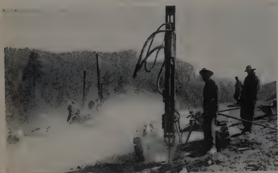
Two Gardner-Denver "Air Tracs" drill out rock at the Wishon Dam site.
