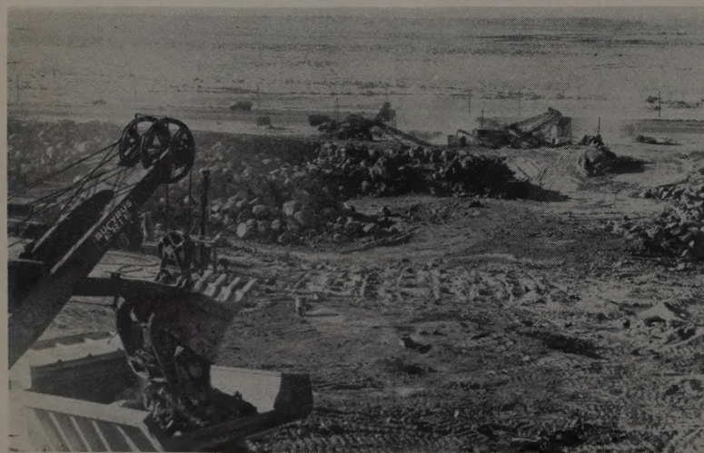
LOADING AT the quarry, the blasted rock is hauled to the primary unit of the plant in the back-ground. The rock feeds into a Pioneer 153-PRL with the jaw crusher set at 7 in.
