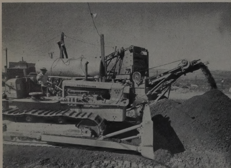
PROCESSED MATERIAL was dumped directly on the roadway in the rear, and kept shaped up by D-8 Caterpillar. About 28,000 tons of material came out of one 25-ft. cut, and 42,000 tons out of a second. The rock was lava and used for base and shoulders.
