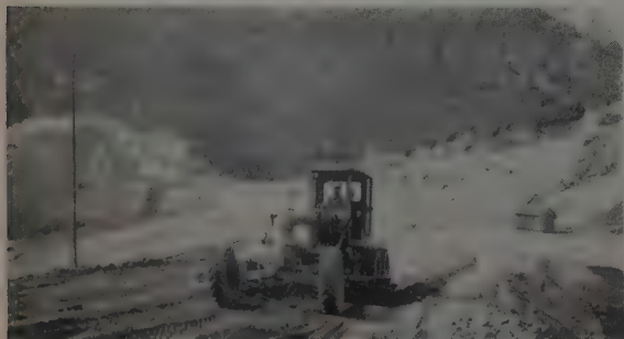
UTILITY units on the fill and on the hauling roads are the Allis-Chalmers Model 45 motor graders. The A-C equipment was supplied by the Wood Tractor Co. of Portland.
