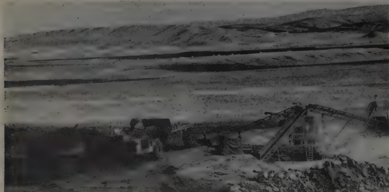
ACCURATE spot dumping over the edge of an embankment into a crusher hopper is easy for these two Movalls, working for Morrison-Knudsen near Rawlins, Wyoming.
