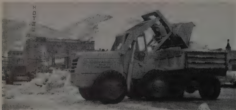
A MICHIGAN model 125A tractor-shovel is kept mighty busy by the City of Missoula, Mont. It is shown loading windrowed snow into an 8-cu. yd. truck. It does this job in 1½ min., just half the time required by the previously used elevating grader. Another way the unit saves time is by the speed with which attachments can be changed. One man needs only 10 min. to change over to a 2-yd. dirt bucket, straight, V, or blower plow. High travel speed along the city's streets helps, too. The machine even works at night, picking up gutter rubbish.
