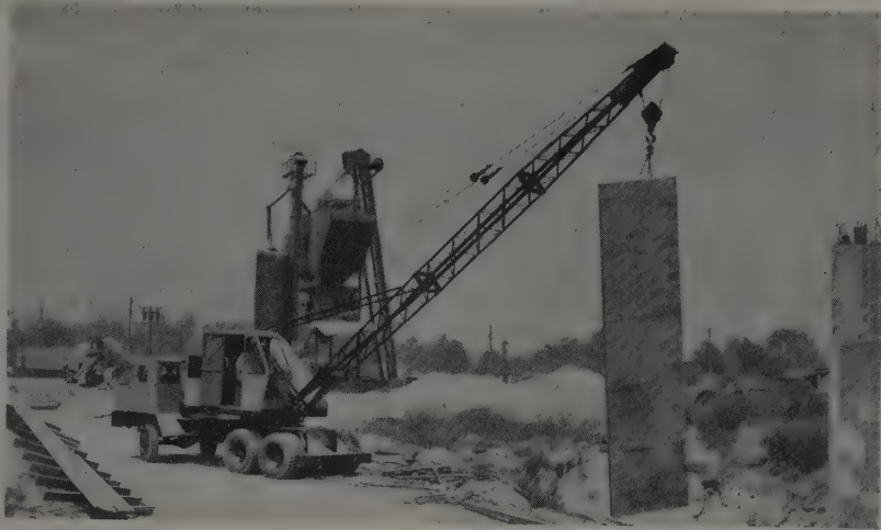
MOUNTED ON rubber, this Schield Bantam T-35 is used by Vinnell Construction Co. of Los Angeles for a wide variety of scattered jobs on the Golden State Freeway job. Traveling from location to location, the mobile rig lifts and handles concrete forms and other heavy or bulky materials as the work moves along.
