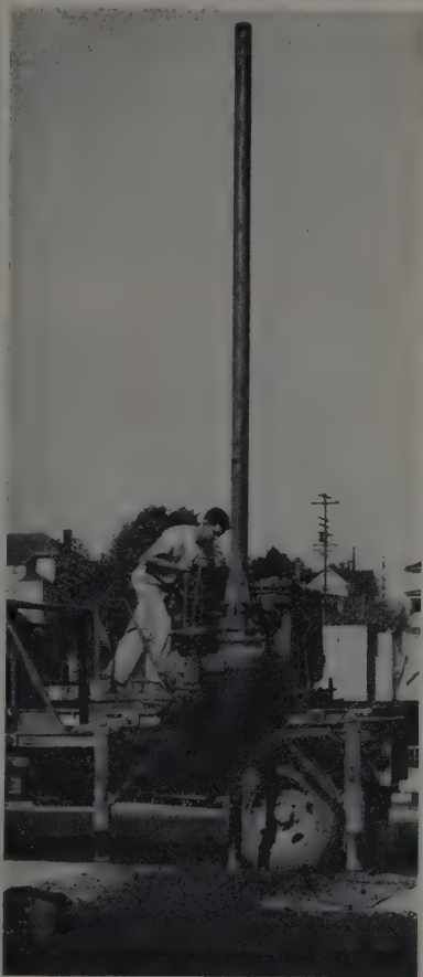
THE J. C. DENTON & SONS CO., Oregon, have just completed a guard rail contract for the Seattle District Corps of Army Engineers at Cottonwood, Idaho. Contract called for 2,060 lin. ft. of guard rail using 164 posts, each post hole to be 4 ft. 2 in. deep. Engineers estimated 25 days for the job. Using the Highway Swing Base Earth Boring Machine all holes were drilled in 3½ working days, instead of the engineers' estimated 10, and the total job completed in 9 days.
