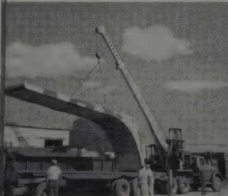
H-5 Hydrocrane makes good use of big capacity and precision control as it lifts this arch for a commercial structure from a railroad car.
