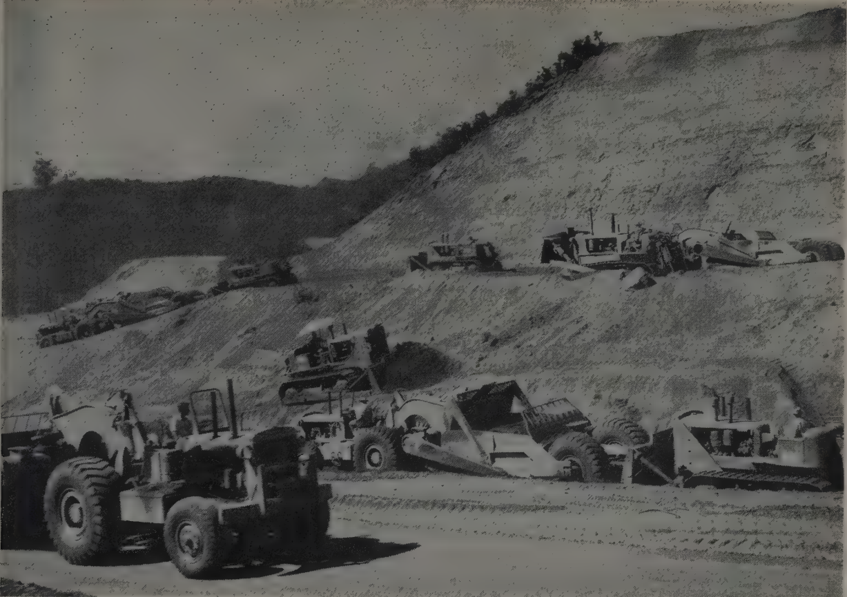
Preparing a mountain top development site in Beverly Hills
