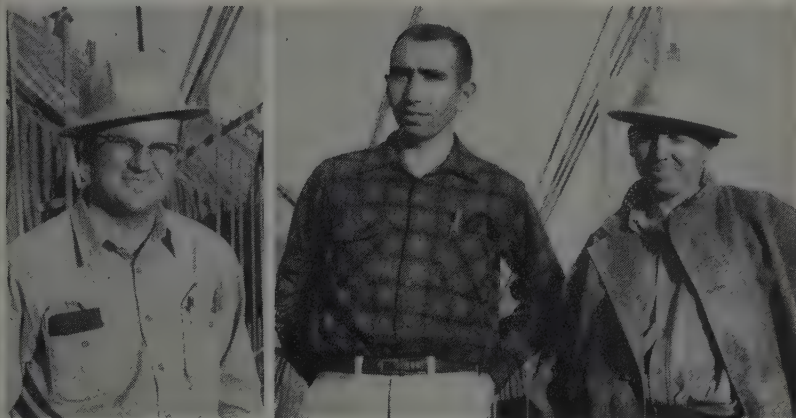
W. D. HUGHES (left), engineer on the Pacific Highway undercrossing at Portland now under construction by Gibbons & Reed Co. Shown with him are Edward L. Hardt (center), resident bridge engineer, and Don Callaher, assistant resident for Oregon State Highway Department. This job is described on page 50 of this issue.
