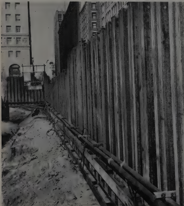
TWIN 6-in. steel pipes encircle site to carry water for eduction pumping system. Note neoprene hoses every 27 ft. which bring water up from 45 ft. below.
