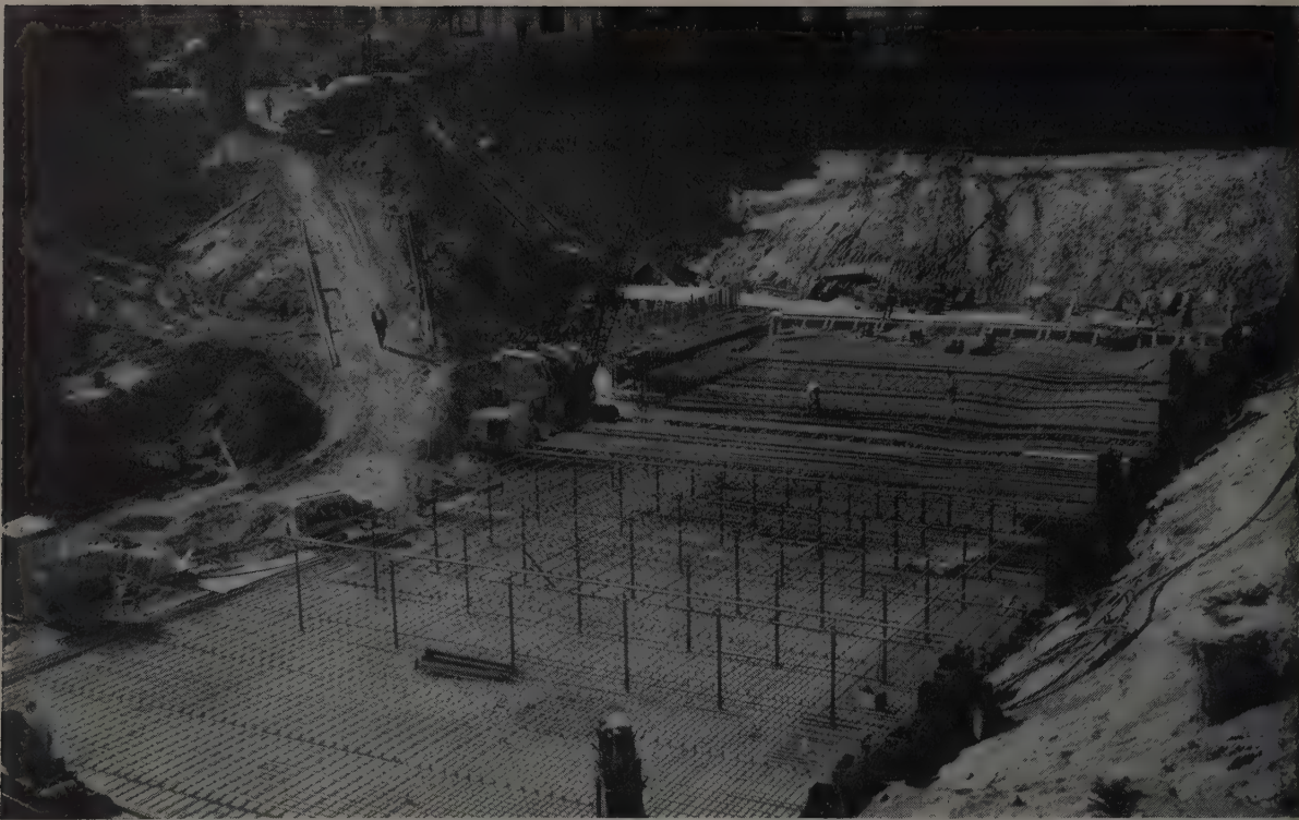
OVERALL VIEW shows steel going into place for the 8-ft. thick main foundation mat. Re-bars up to 2 1/8 in. in diameter are being used in
