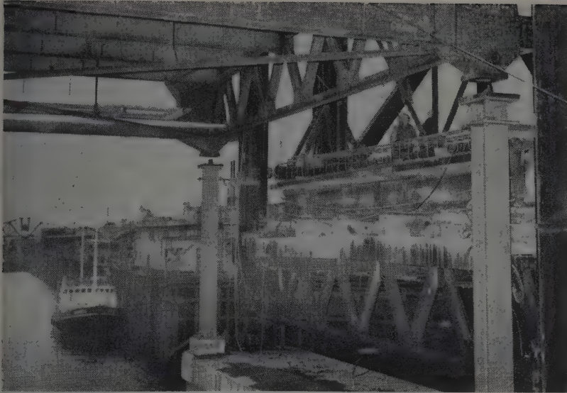
SLOWING LOWERING , as the tide ebbs, the span is approaching final seating with pintles on the pedestals about to engage. Clearance was only 1½ in. at each end.
