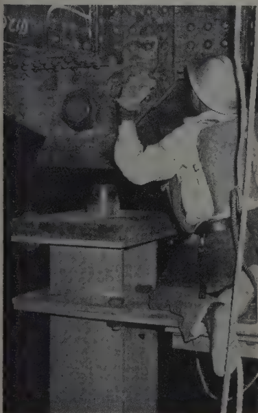
FINAL POSITIONING approaches as one corner of the 426-ton span is kept under close observation. Jockeying into position and lowering was accomplished from 4 to 7 a.m.
