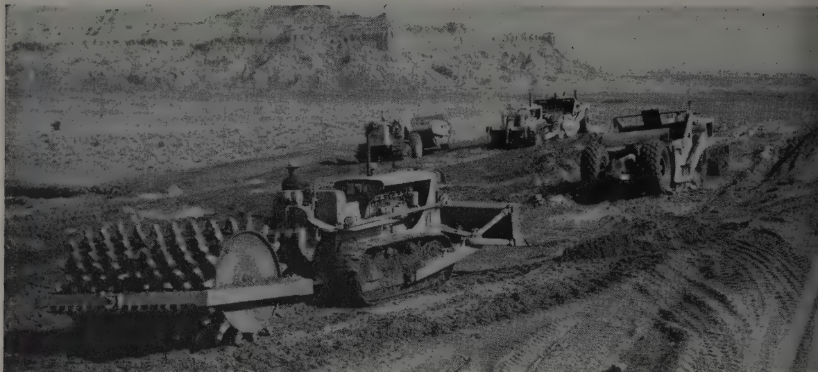
GRADING AND COMPACTION equipment at work on the 8 1/2-mi. section near the Utah-Arizona border. Here, as elsewhere, lack of water
