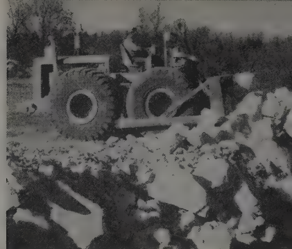
Tournatractor's wide, low-pressure tires flex easily over sharp rocks without cutting... end age-old problem of rocks, sand, and dust clogging up track assembly.
