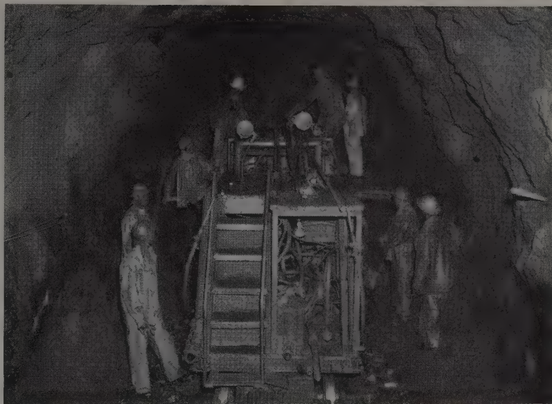
TUNNEL DRILLING is done with 6 Gardner-Denver drifters mounted on a job-built two-deck jumbo. Bits are Sandvik Coromant and Brunner & Lay. Blasting pattern involves about 64 holes divided into 10 groups with 25 millisecond delays between most of the groups.
