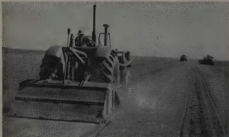
MIXING was done by a Seaman-Andwall Pulvi-Mixer, starting as soon as two lanes of cement had been applied. Mixing was to full depth. Cement content was 7.2% by volume.
