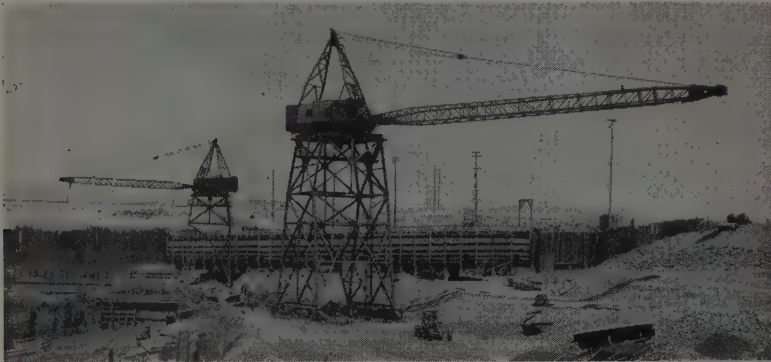
THREE WHIRLEY gantry cranes, 85 ft. high, handle concrete placement. Schedule calls for 80,000 cu. yd. of concrete to be placed each month. Completion date is Aug. 1958.
