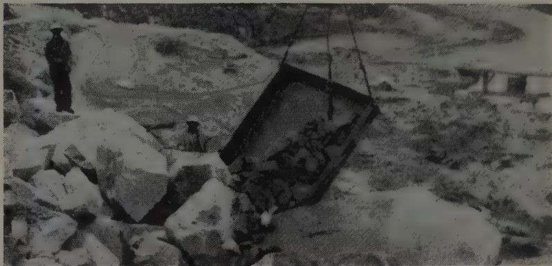
FILLING THE VOIDS between the large rock are small chink rock (minimum: 2 in.) which is placed by this 6 x 6 x 1-ft. pan. Michigan loader fills the pan at the top of the embankment.
