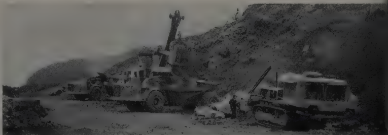
ROCK FOR THE underwater fills was drilled by Ingersoll-Rand unit on Caterpillar D8 providing stability with mobility. The Koehring 3-yd. shovel loads into Cat DW21-Athey PR21s. Steeply timbered bank which made the fill location economical is shown in the picture at top of page.
