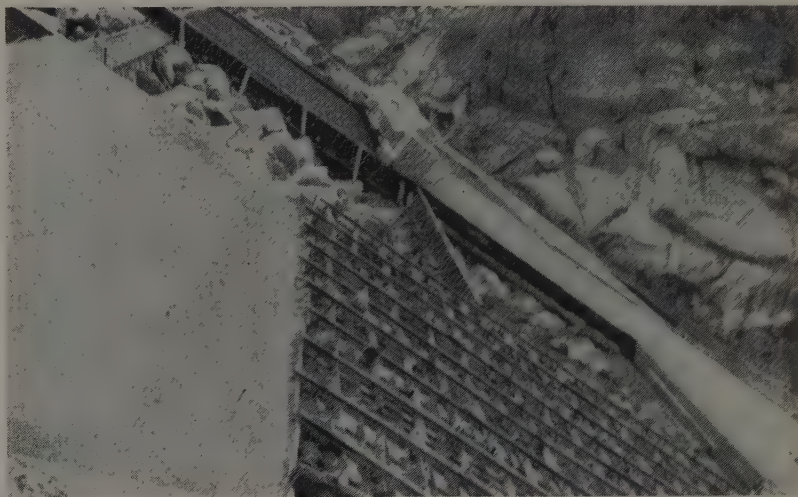
TWO METHODS of forming the concrete face at Courtright were tried. In the foreground are prefabricated panels backed by strongbacks, and in the background is the slip-form screed. Experience at Wishon showed that the screed worked best.
