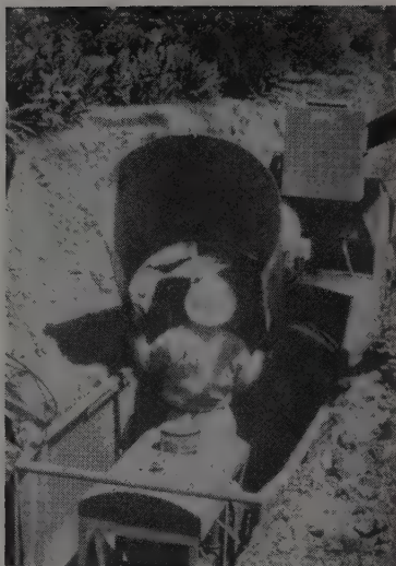
INSIDE forms for sides and top of pipe are handed to operator in 4-ft. lengths, as shown, and hook onto the preceding section. No outside top-form is required. Interior shape is maintained by struts placed inside the form. From 2 to 4 hr. later the struts are removed, forms collapsed and pulled forward.
