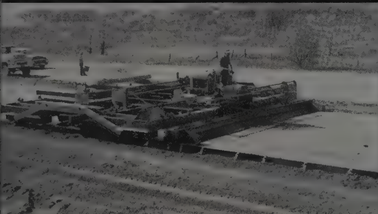
S. ROUTE 12—Kalamazoo, Mich.: Bypass is worked Carl Goodwin & Sons. Contractors generally report substantial savings over previous finishing methods.
