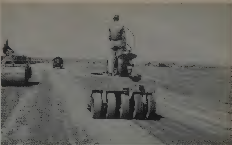
INITIAL COMPACTION was by rubber-tired rollers working on the mixed material while it was still very damp. Steel-wheel rollers followed. A smooth, tight finish was secured.
