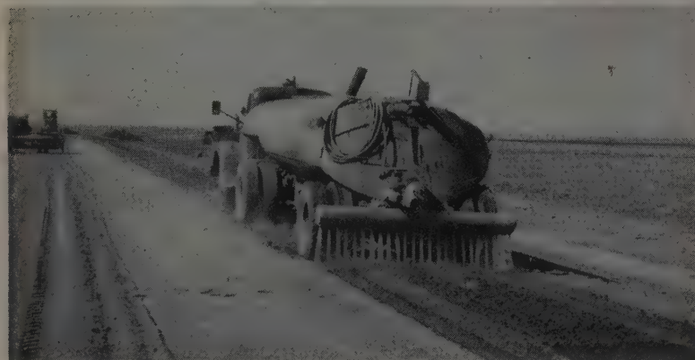
THREE tank trucks, hauling from a coulee 7 mi. from the job, added water during moist mixing. The contractor handled the processing work in 1,000-ft. sections.
