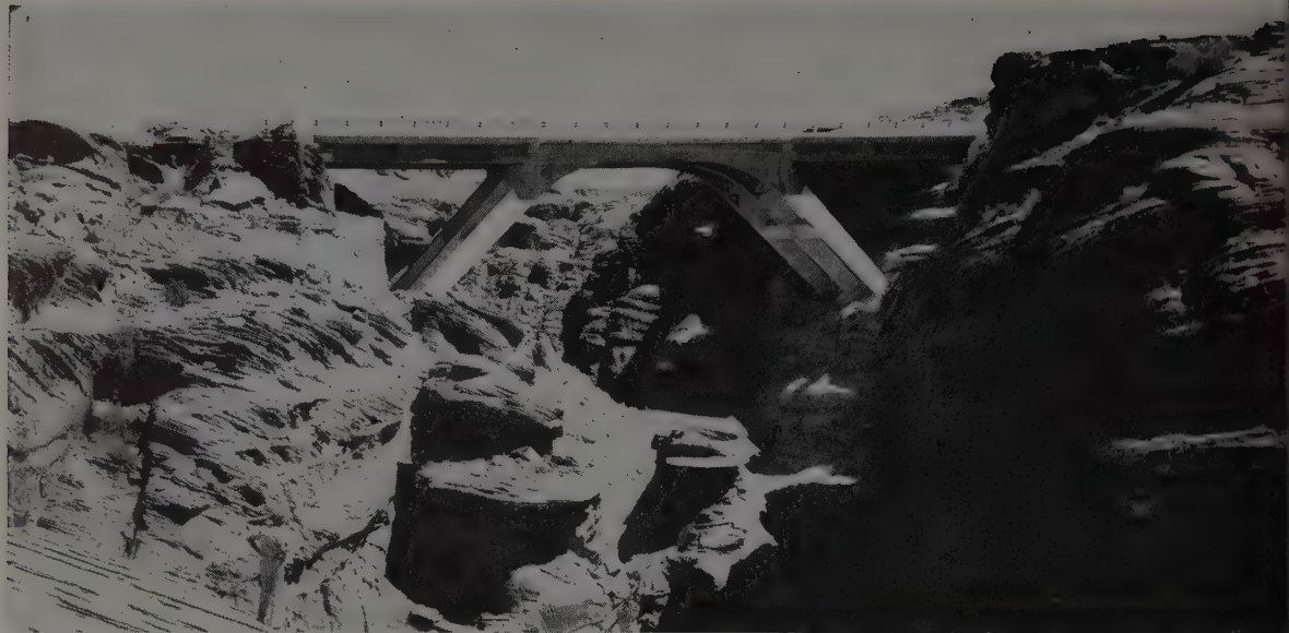
WATERHOLES BRIDGE has been completed. The narrow canyon was the only obstacle in the 20-mi. access road contract being carried out
