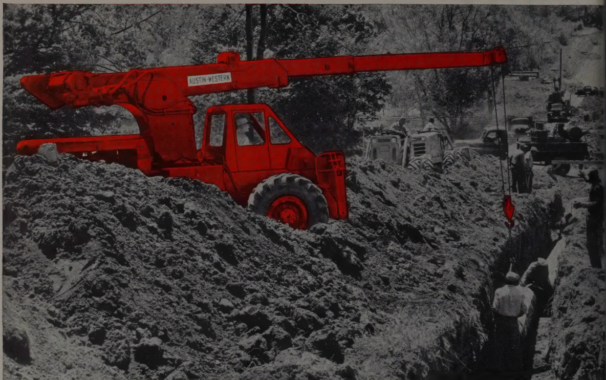
A-W hydraulic crane setting 24 in. x 20 ft. drain pipe on highway job near Philadelphia
