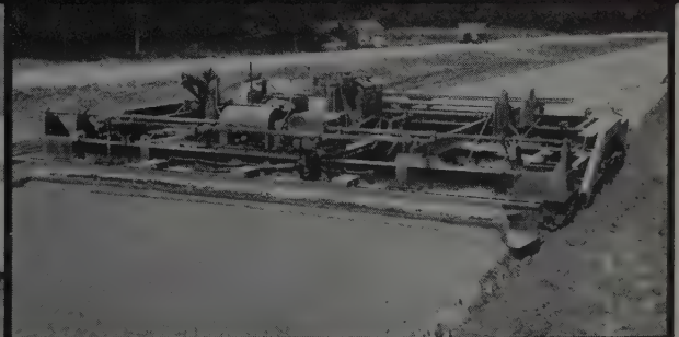
U. S. ROUTE 23—Combination Machine owned by Denton Construction Company keeps up with three dual drum pavers south of Brighton, Michigan.
