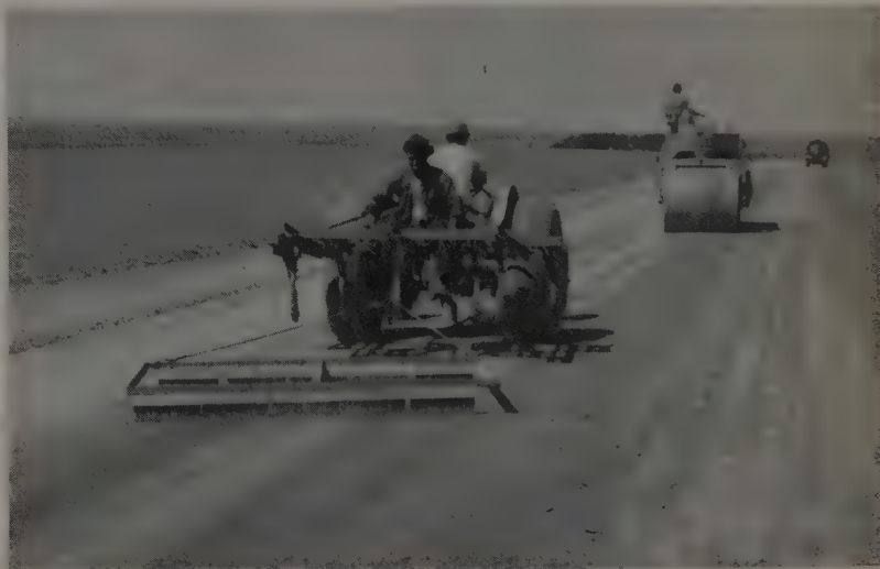
GRAVEL COVER was pressed into the unhydrated soil-cement to provide a firm bond between surface and base. Later, a second bituminous shot was applied, and covered with small chips. A broom drag removed small irregularities before final rolling.
