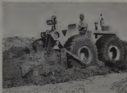
One of many spare-time jobs handled by Tournatractor is building new haul road. Operator takes overburden dirt, drifts it on down to bottom, building up road grade.
