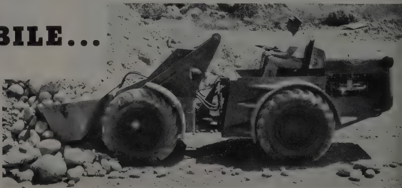
LD-5 Scoopmobile loading boulders for fill.
