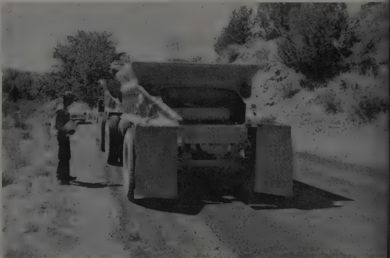
LOADS WERE dumped directly into a windrow sizing box. As the truck moved forward it dragged the box and placed the windrow, which was picked up by the paver.
