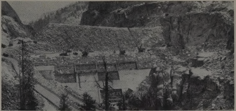
OVERALL VIEW of Courtright Dam shows three operations proceeding at once, the concrete facing at the bottom, the crane-placed rock, in the center, and the dumped rock at top.
