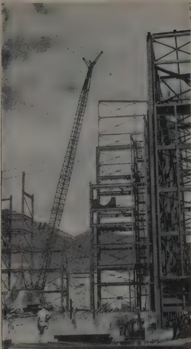
AT a guided-missile plant near Littleton, Colo., this Manitowoc 3,900 crane with a 170-ft. boom sets high steel in the assembly building. Contract is held by Shurtleff & Andrews Co. of Salt Lake.
