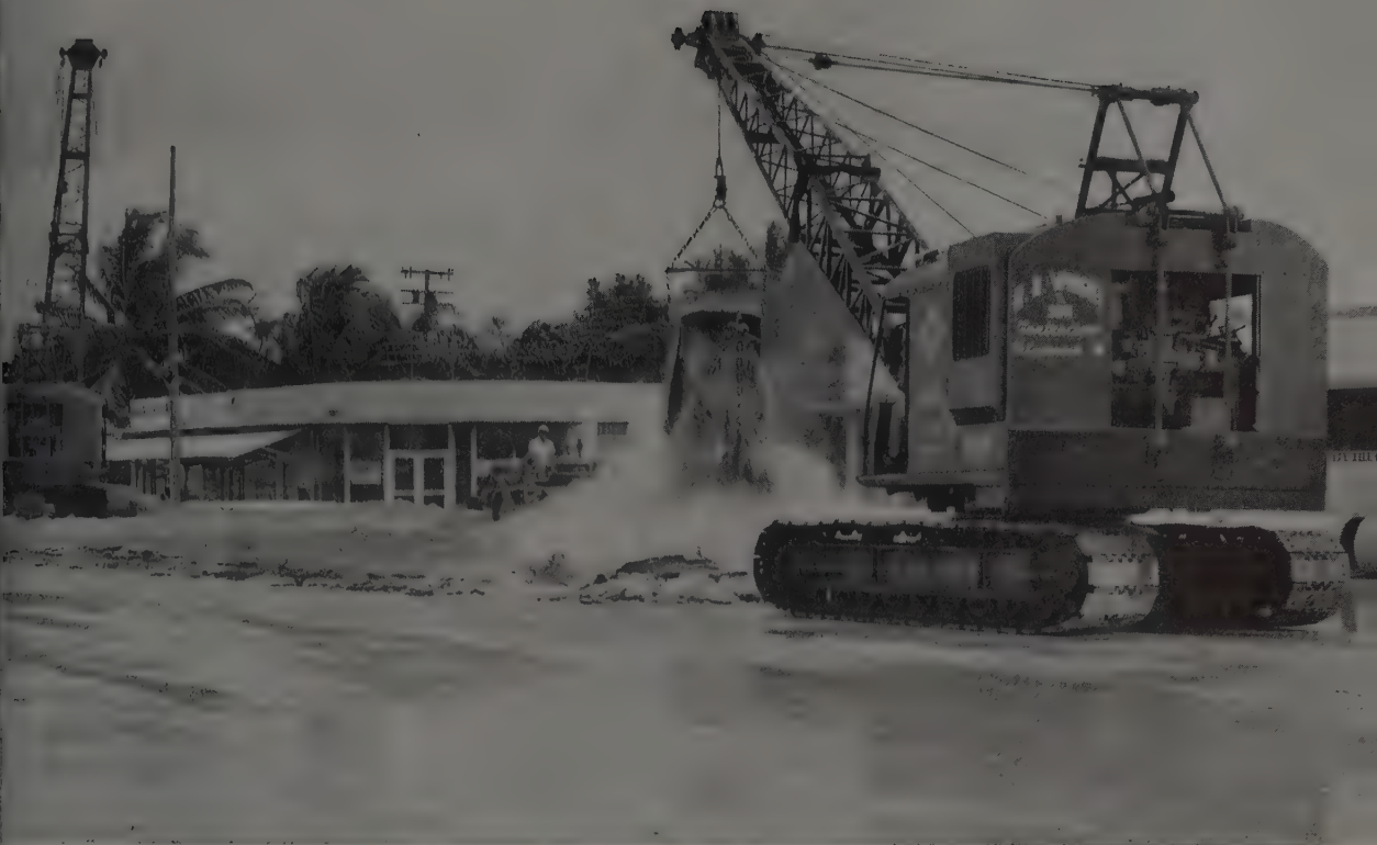
Lima Type 604 Dragline excavating trench for storm sewer pipe in Miami, Florida. This machine and the other Lima Type 604 in the background are owned and operated by R. H. Wright & Son of Fort Lauderdale and are both equipped with 45-ft. booms.
