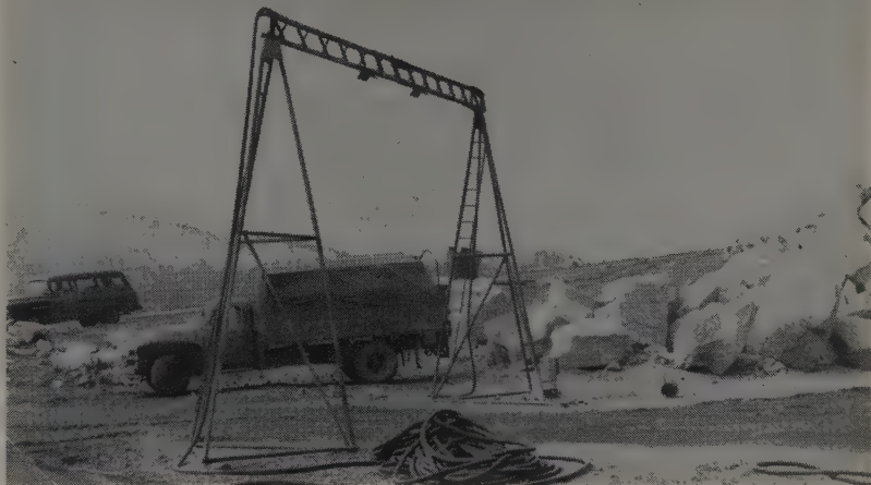
CABLE TOWERS which carry electric shovel cables over truck path are fitted with brackets on the cross-piece which enable truck to lift them and carry them away on upraised dumps.
