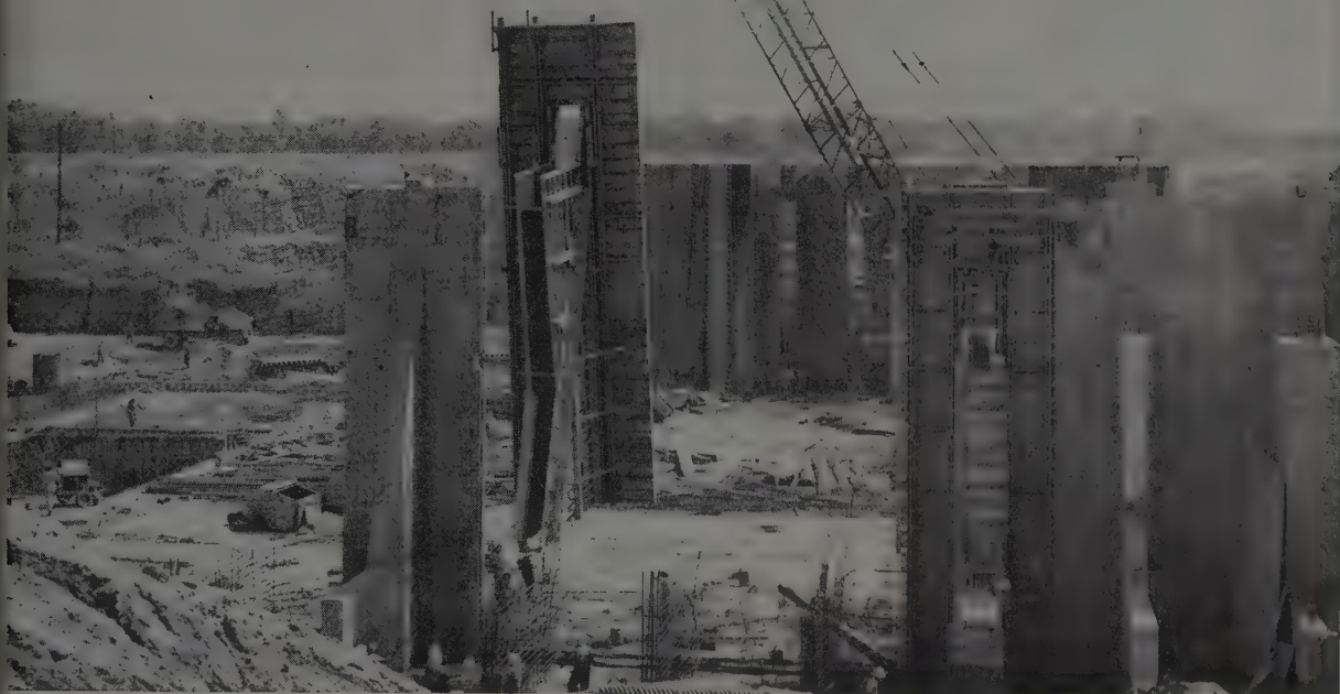
Backwall and counterfort form being placed. Handling time is cut to the bone by special form design. Form at right is ready for stripping and re-setting at new location.
