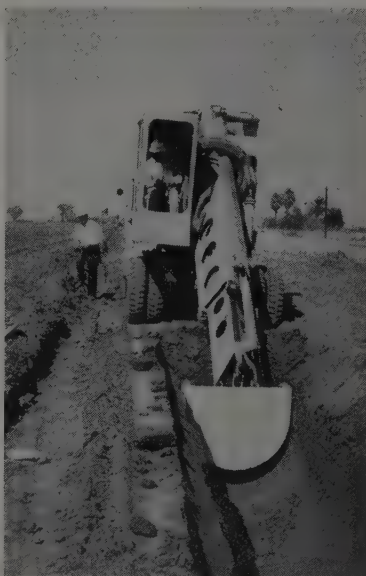
SPECIAL shaping bucket designed by Dick Juetten, of the project engineering staff, enables the Gradall to prepare the ditch to proper shape for pipe casting.
