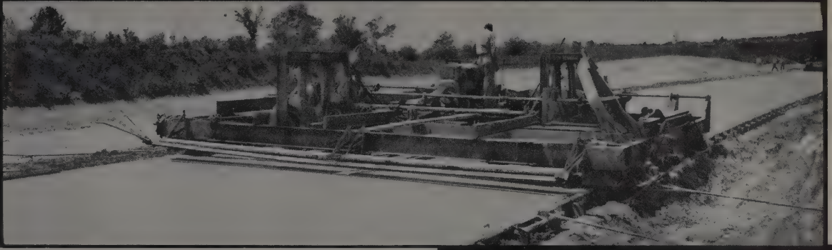
U. S. ROUTE 30 — J. A. Jones Construction Company uses combination on straightaway paving — Flexplane self-widener on interchanges near Mansfield, Ohio.
