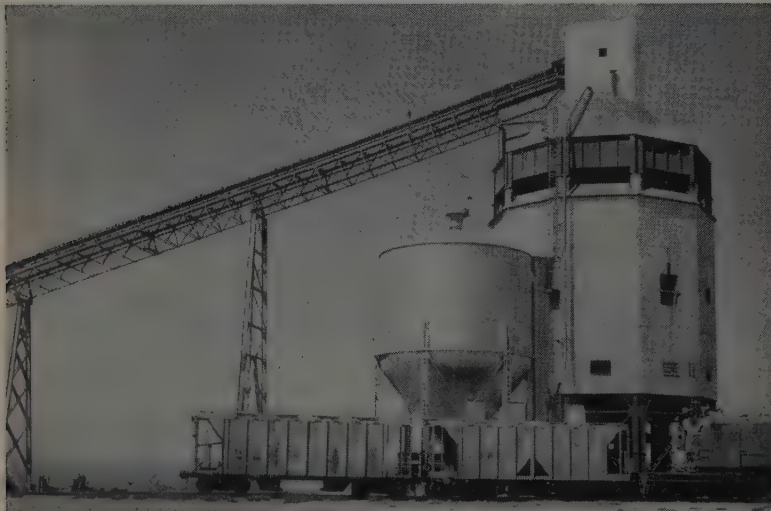
BATCH PLANT used for Montana's Hungry Horse Dam is now at work at Ice Harbor turning out 300 cu. yd. per hr. Plant was built originally for California's Shasta Dam.
