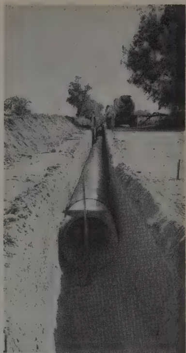
COMPLETED section of No-Joint pipe, with casting machine at work in the background. A day's pour of 30-in. pipe is usually about 500 ft., completed in 2 to 2½ hr.
