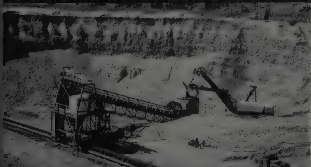
PIT HOPPER FEEDER, PENDULUM CONVEYOR, CRUSHER CAR AND FIELD CONVEYOR
