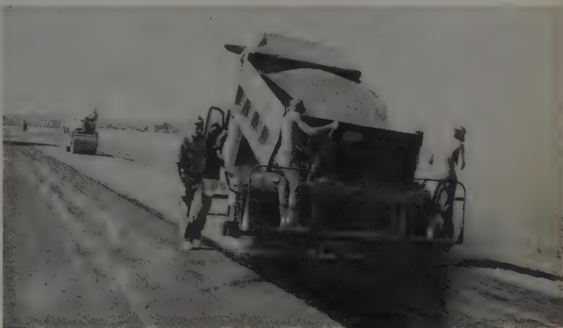
SURFACE treatment was an application of RC-2 bituminous material placed immediately as a cure and covered with \frac{1}{2} in. of crushed gravel.
