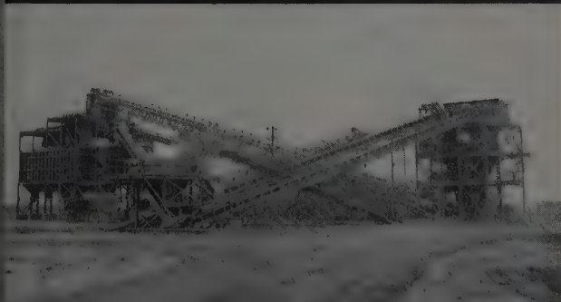
HARTMAN CONCRETE MATERIALS CO., SAN EMIDIO PLANT, BAKERSFIELD, CALIF.
