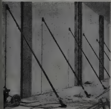
SUPERIOR ADJUSTABLE BRACES with exclusive pivoting action, permit quick and easy alignment of panels.
