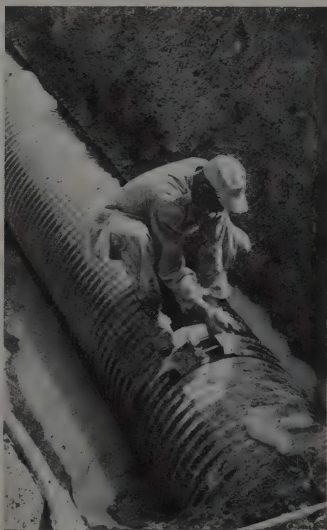
Joints can be made quickly and easily. Here one man tightens the two bolts on a connecting band with a hand wrench.
