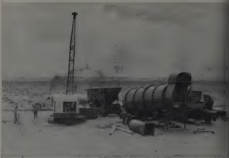
AS THE UNITS of the asphalt plant arrive on the job a Lorain crane begins assembling them. The 9 x 12-ft. rotary dryer on the right is the largest made. The barrenness of the countryside in the background indicates the remoteness of the project site.
