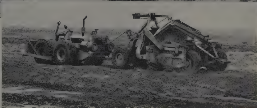
R. Brown's Tournatractor, with cable-operated scraper, self-loads about 8 loose yards of taxi-strip excavation at Farmington, N. M., Municipal Airport.
