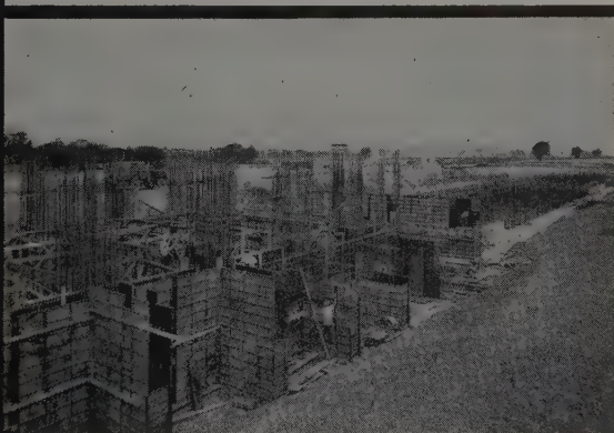
Heavy Industrial Foundations
