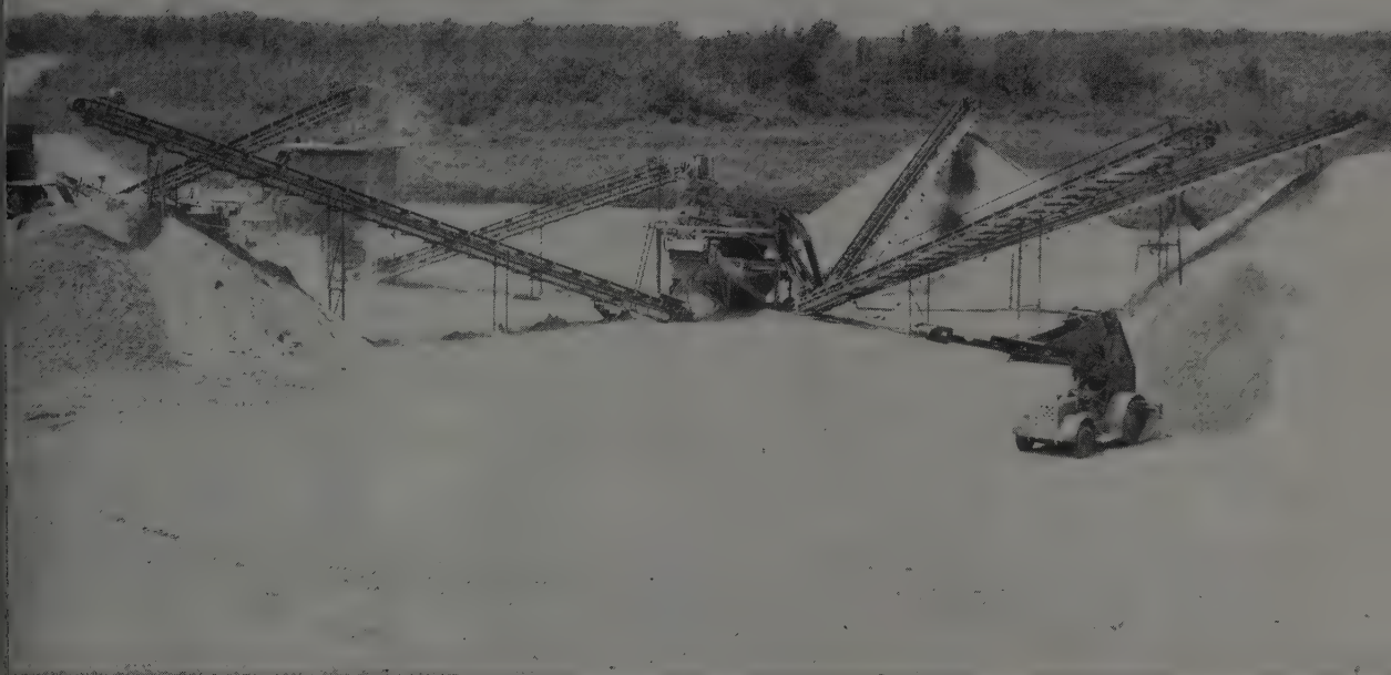
A-W Crushing Plant of J. J. Cronin Co., showing primary crusher at extreme left. Washer is in center of photo. Washed sand is delivered by the conveyor on left of washer, specification material by the three stock-piling conveyors at the right.
