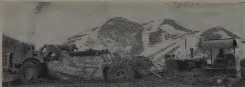
WITH A background of rugged Alaskan scenery, excavation was a problem for both access road and structures. Rock was porous and the ice melted as the surface was uncovered. This water collected in all excavated areas, and heavy rains were common.
