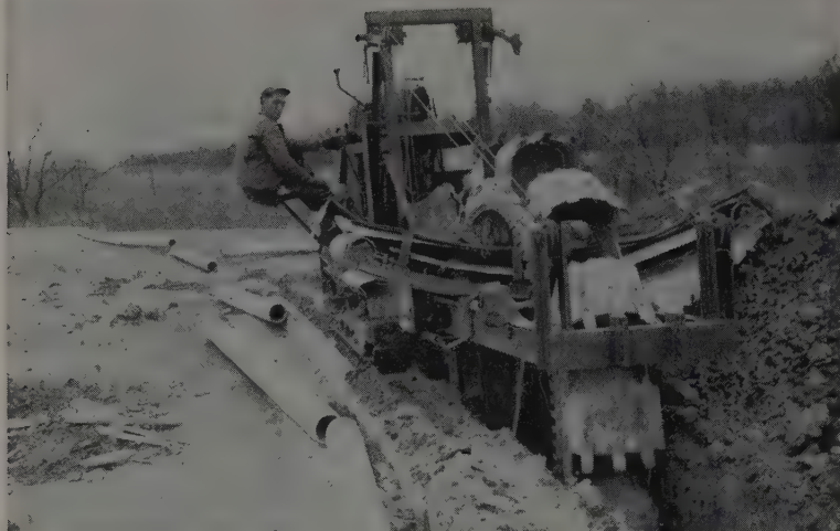
Veteran operator Delbert Corman "at ease" while his Cleveland is digging gas and water lines for a Lexington, Ky. subdivision
