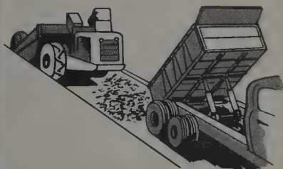
2. "D" spread pit-run gravel dumped in trench by trucks.
