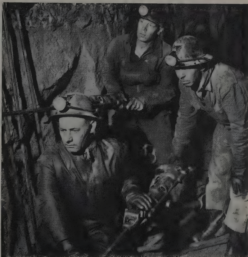
DRILLING CREWS used Atlas Copco airleg rock drills with Sandvik Coromant drill steels. Left to right are Carl Saueruiem, Billy D. Moore, and Charles H. Moore starting a round.
