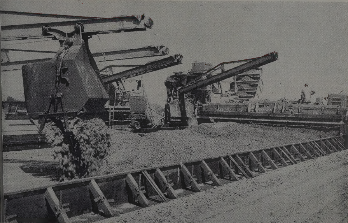
R KOEHRING 34E pavers team up to pour 6 cu. yd. of concrete 42 sec. for a B-52 runway at Beale Air Force Base near Marys-
