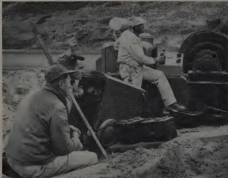
THE HOLD-BACK winch on the shore and the pulling barge at sea were coordinated by two-way radio communication. The pipe-pulling technique was described in the July issue.
