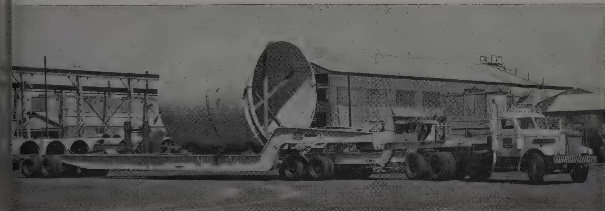
TRAILER WITH 11 AXLES AND 42 TIRES HAULS LARGEST CONCRETE PIPE
