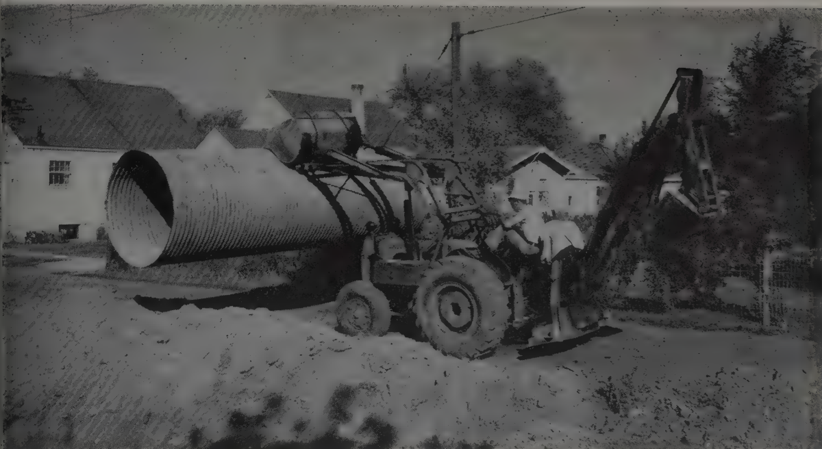
No special lifting equipment needed. The machine that dug the trench for this job was also used as a hoist in laying the pipe.
