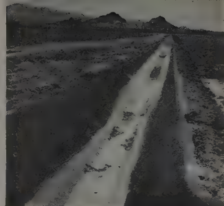
Completed concrete-lined irrigation ditch — like that under construction at Wing Low Ranch, 25 miles northwest of Tucson.
