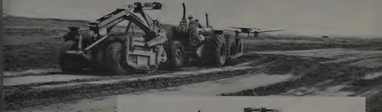
R. Brown's Tournatractor, with cable-operated scraper, self-loads about 8 loose yards of taxi-strip excavation at Farmington, N. M., Municipal Airport.
