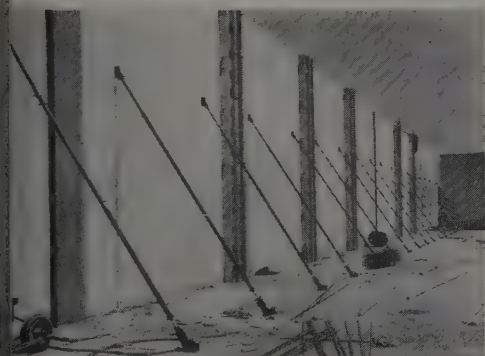
ADJUSTABLE BRACES used for quick and easy alignment of panels
