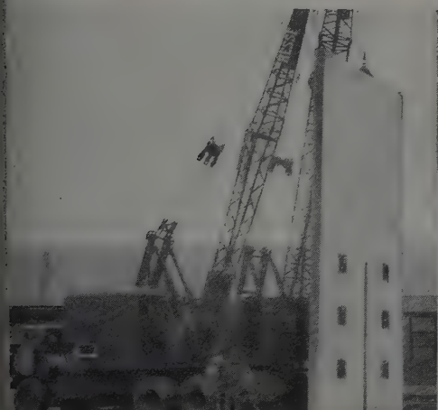
57 TON SLAB being positioned
