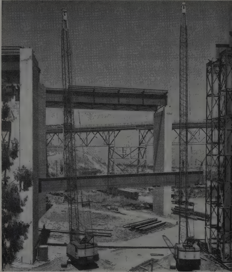
WITH HAMMER-HEAD booms 130 ft. and 140 ft. long these two cranes picked up and placed this 105-ft. 22-ton girder section at a height of 120 ft. One of the cranes was positioned on a pile of dirt placed on an existing highway, and the other occupied an area leveled by bulldozers.
