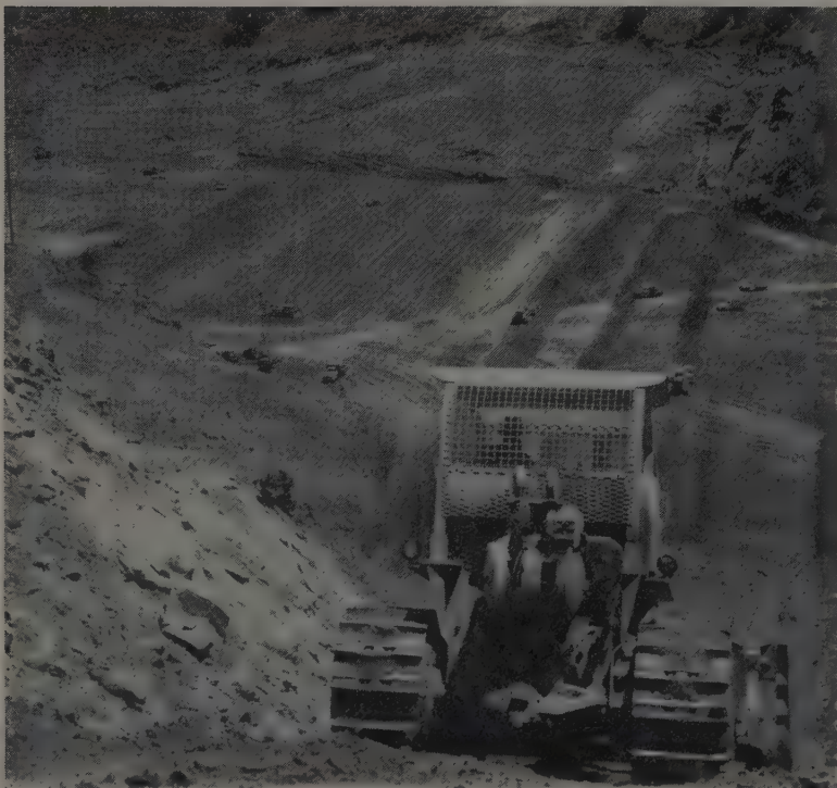
A CRAWLER TRACTOR dozes down a steep slope high above the steadily growing Casitas Dam. Located on Coyote Creek above Ventura River, the dam will be 275 ft. high, 2000 ft. long.
