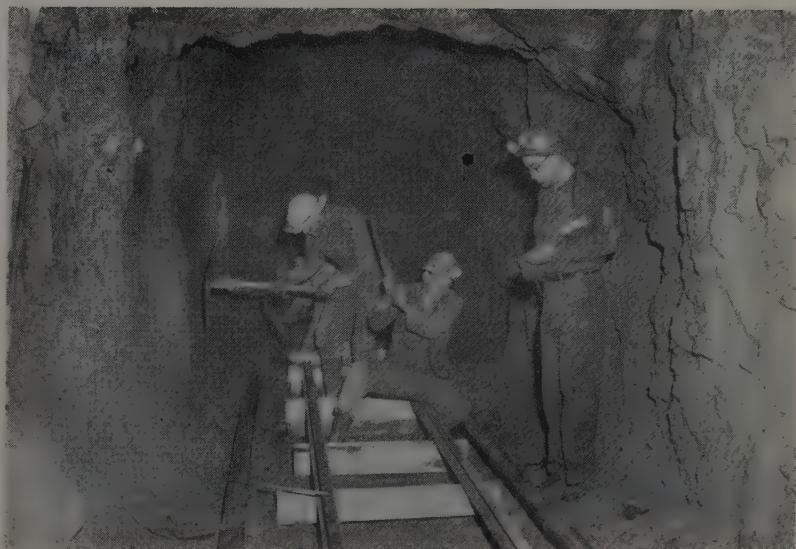
CREWS lay shuttle car line under supervision of tunnel foreman Jess Bingel, right. The 4-ton shuttle car was homemade. Mucking was done with an I-R slusher.
