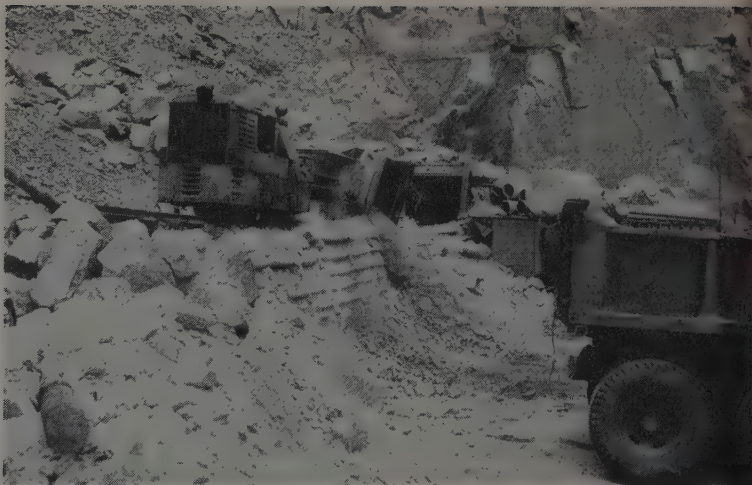
PLYMOUTH diesel engine has pulled two rocker dump cars into position for dumping out west portal. Rock is then reloaded into trucks and hauled to waste site.
