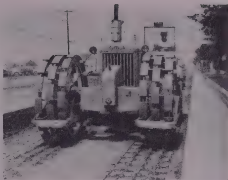
Here, the K-45 Kompactor works up close—eliminates hand tamping on this California job.
