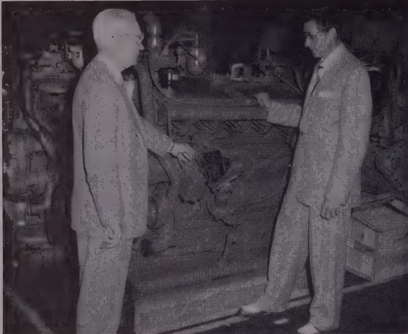
JOHNNY BULLA has joined the sales staff of Cummins Diesel of Arizona. Here he appears at the Cummins plant in Columbus, Ind., with Paul J. Every (left), general sales manager. The engine is a 600-hp. VT-12-1 used in the construction industry, a sales field in which Bulla will specialize. He will serve as a sales representative for Paul Miller , Cummins distributor in Phoenix, Ariz.
