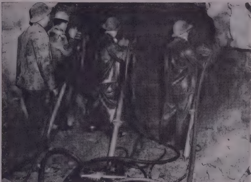
Three Ingersoll-Rand JR-38B Jackdrills with 1½" Carset Jackbits, drilling through hard sandstone in the 8' diameter Oswego Water Tunnel. Thirty holes were drilled for each round, and two rounds were drilled, blasted and mucked per shift.
