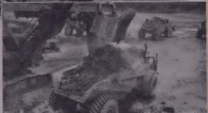
B Rear-Dumps, working on St. Lawrence Seaway lock at Côte Ste. Catherine, carry 33 to 38 tons of shot rock. In earth overburden weighed loads averaged 34.4 tons.
