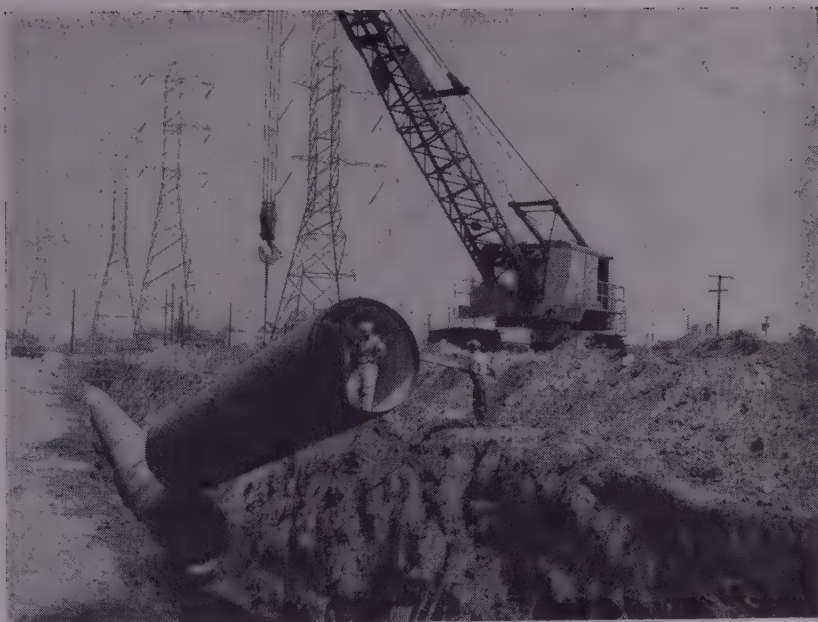
LOWERING A 79-IN. WELDED STEEL PIPE NEAR SOUTH GATE
