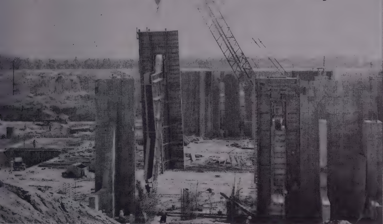
Backwall and counterfort form being placed. Handling time is cut to the bone by special form design. Form at right is ready for stripping and re-setting at new location.
