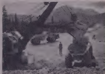
Three to four passes by 2-yd. shovel fill 11-ton Rear-Dumps to heaped capacity. Low rear entry and wide bowl provide easy target for shovel operator... allow fast swing-out of shovel dipper, let shovel operator heap maximum yardage with minimum spillage.
