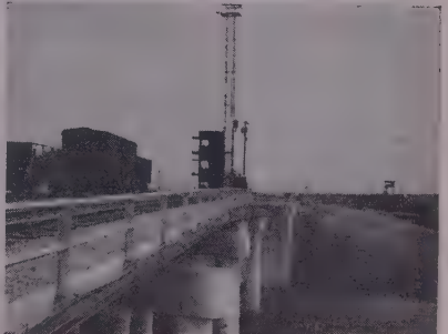
Bridge Wing Walls?
