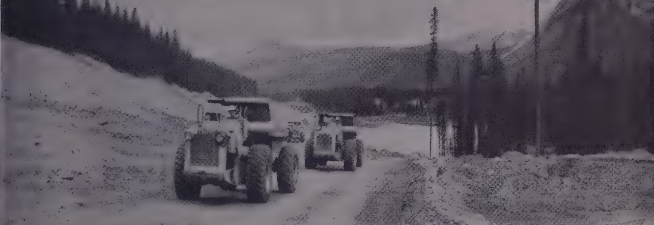
Photo shows Rear-Dumps on return portion of cycle, climbing grades to 12%. This new section of Trans-Canada Highway will eliminate narrow twisting roads with many hairpin turns.
