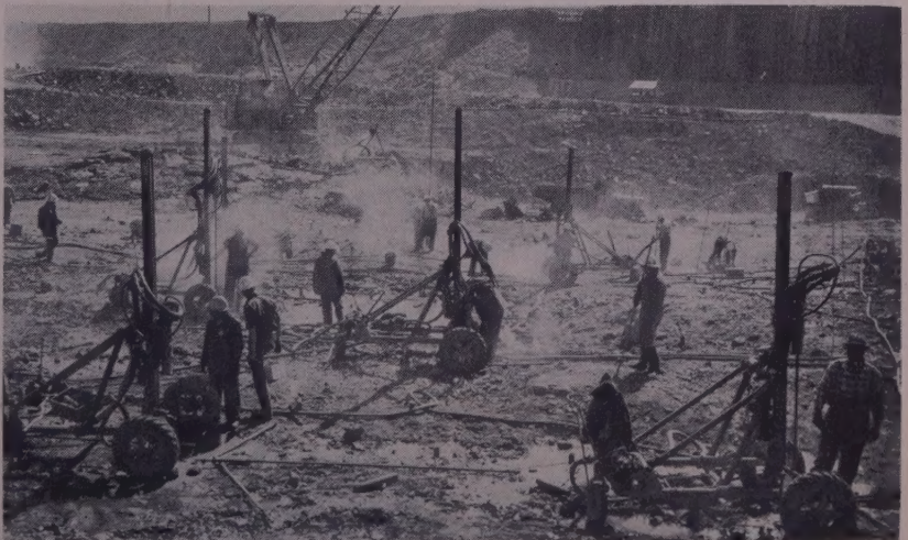
DRILL RIGS go to work sinking blast holes into the bedrock as the powerhouse excavation gets underway. The powerhouse will be 1,025 ft. long, with a base width of 197 ft.
