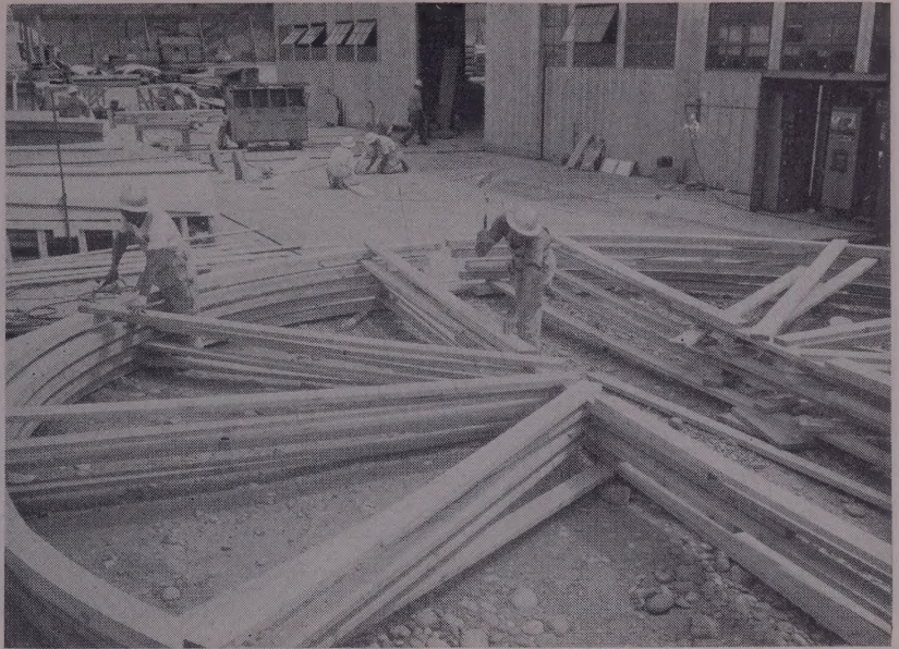
CARPENTERS WORK on a 28-ft. wooden form that will be used in building draft tubes below the turbines. Entire job will require 85 acres of wooden forms for concrete work.
