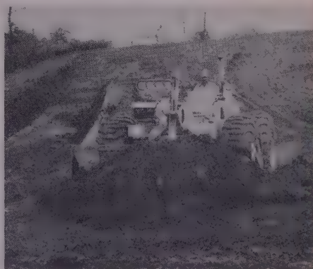
Speedy Tournatractor kept Tournapull production high. It push-loaded "D's" to capacity in soft, uncertain footing... dozed on fill between times. Like the 'Pulls, this 210 hp unit goes anywhere fast, under its own power.
