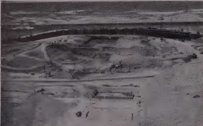
FIRST STEP COFFERDAM has been completed by Guy F. Atkinson Co., and foundation work has started by joint venturers Montag-Halvorson-Austin, holders of a $30,000,000 contract.
