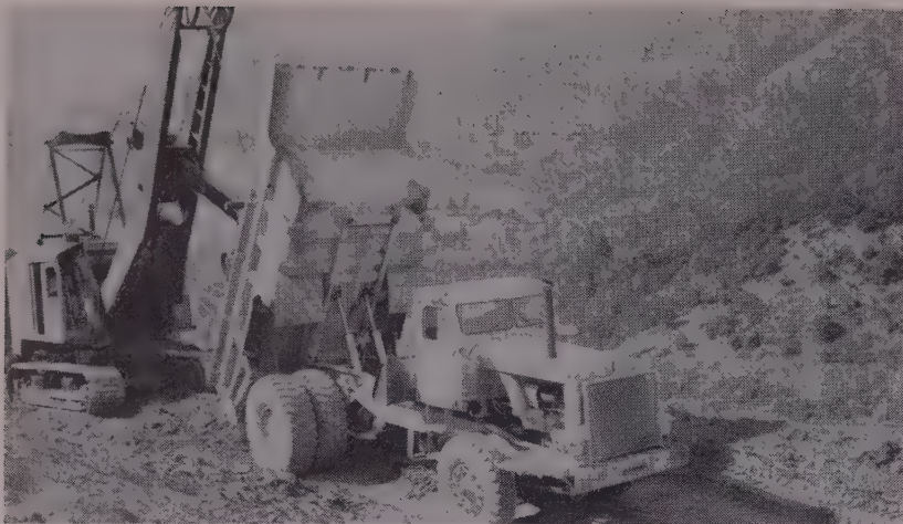
YOU SCRATCH MY BACK, ETC. A Northwest 80D scrapes off an accumulation of mud from the bed of a Euclid. Mud was troublesome in the wet spring months.
