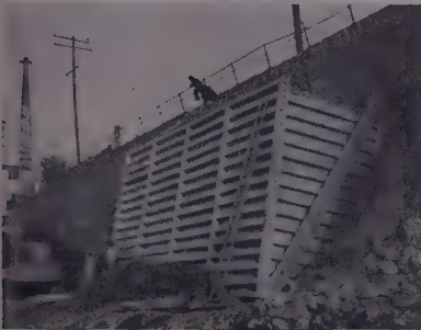
Replacing Existing Wall?
