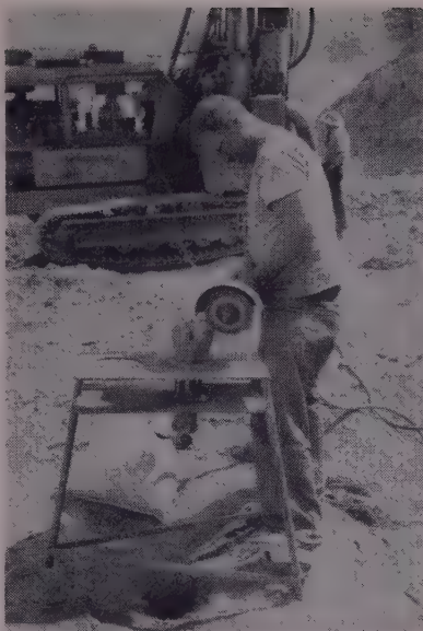
AN INGERSOLL-RAND Rockmaster, visible in the background, is being used by subcontractor Gibson & Roberts on the C. R. O'Neil contracts. Bits are sharpened every 30 ft.
