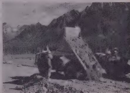
Building a 10-ft. lookout point between grade of Trans-Canada Highway and Bow River, D Rear-Dump spreads its load in about 18 seconds. Electric controls respond instantly for positive, controlled dumping.
