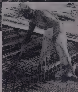
Above: Pouring section of first floor of new 5-story Herman Miller Bldg., Dayton, Ohio. Right: Close-up of operator using a Master "1-Man" vibrator between closely spaced reinforcing rods.
