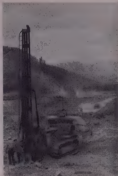
DRILLING on the Kuckenber contract is being done with a rig assembled in the contractor's shops. It's a 500 Joy drill mounted on a Cat D8 and powered by an I-R Air Flow Compressor.
