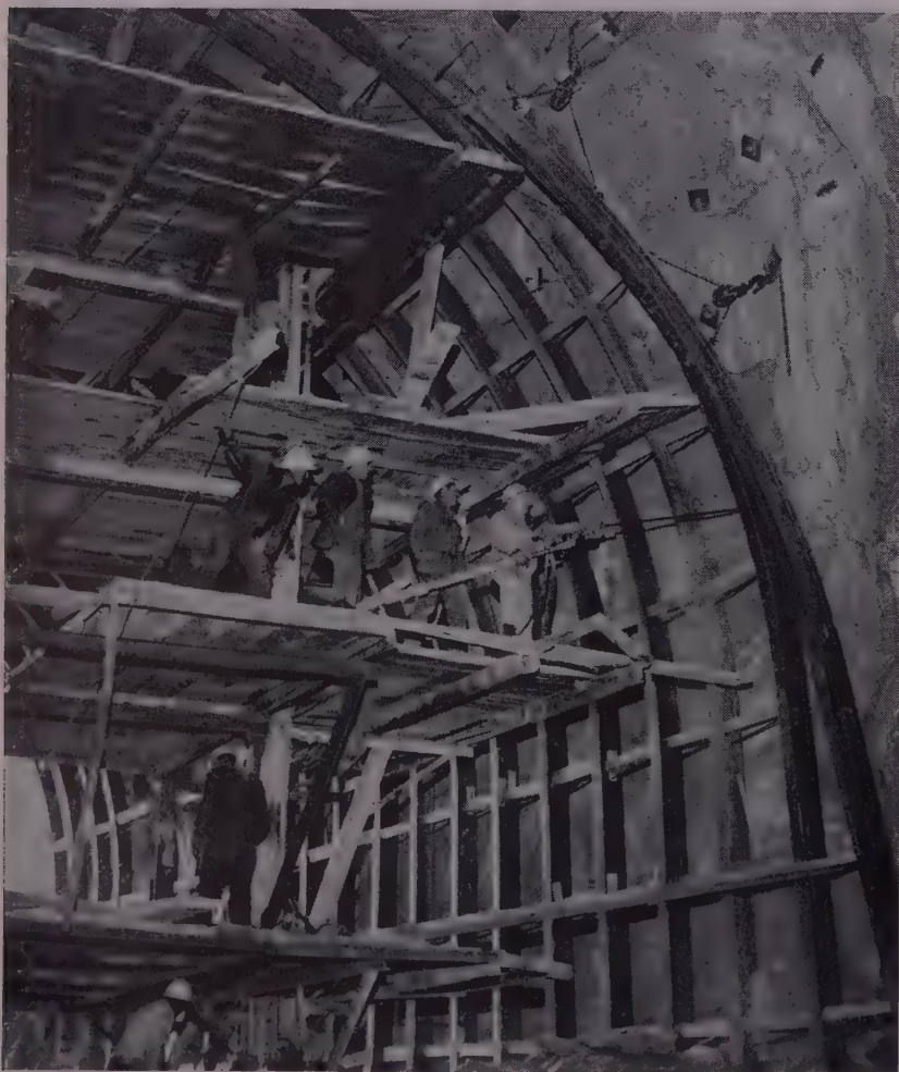
STEEL SUPPORTS were set near the tunnel portal. Drilling is to trim rock back to the line for the rib. Note plates showing installation of rock bolts at upper right.
