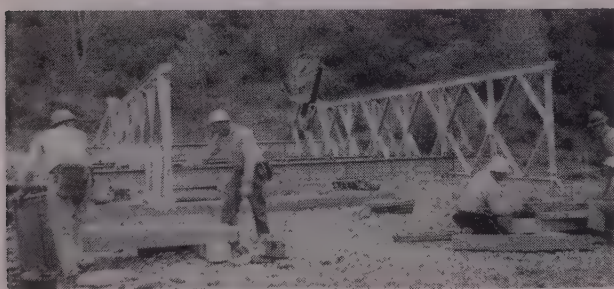
1½ HOURS: Assembling launching nose on rollers.
