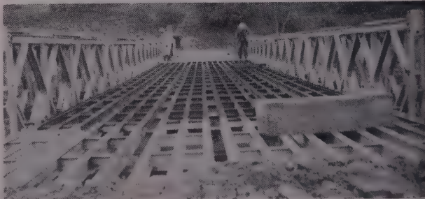
26 HOURS: Ramps and fills completed. Deck and curbs going in.
