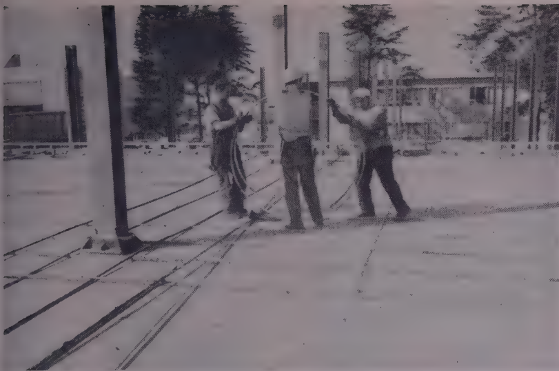
PRESTRESSING CABLE is rolled into place. After utilities are also in place concrete is poured, cables are stressed, and the slab is raised to correct elevation by jacks on top of columns.
