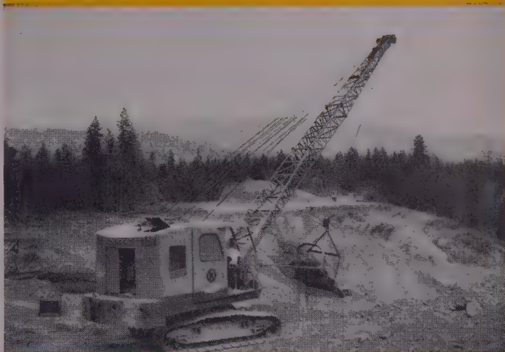
▲ The Koehring dragline, with 1-yard bucket, is powered by a Cat D318 Engine.
