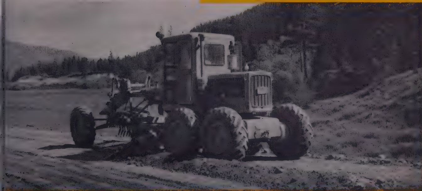
A Caterpillar No. 112 Motor Grader scarifies and grades road surface before asphalt mix is laid.
