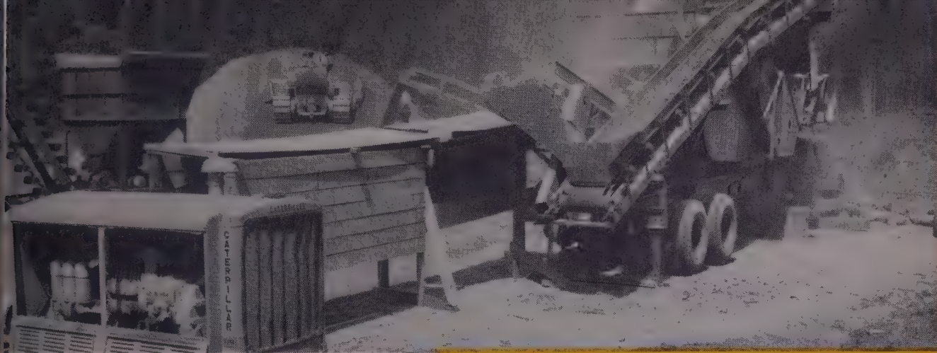
▲ This D342 Engine drives the Pioneer portable crusher. In background, working on the gravel stockpile, is a Caterpillar D6 Tractor.
