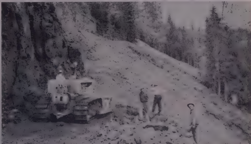
NEW LANES are now being excavated at the base of the bluff at the top of the talus slope. This phase corresponds to diagram three in the sequence drawing presented on page 52.
