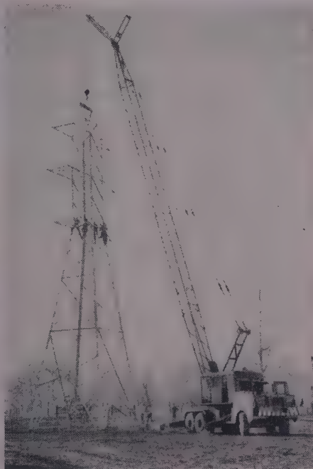
COLORADO Erecting transmission towers
