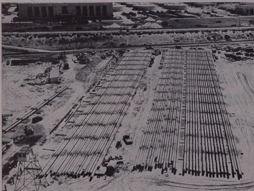
AERIAL VIEW shows 7 mi. of pipe stored on the beach before the pulling operation. Pipes arrived in 40-ft. lengths, were welded into 600-ft. sections. Hyperion treatment plant in background.
