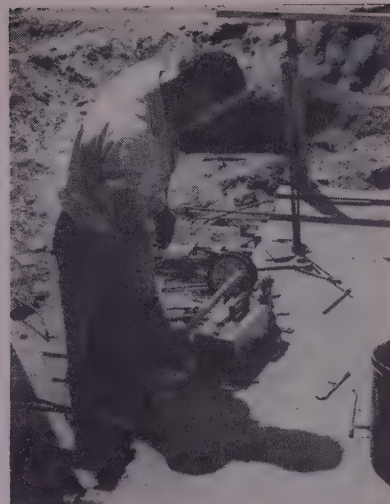
STRESSING is done manually with hydraulic jack from one end on short cables, from both ends at once on long cables. Job called for about 1,500 stressing cables.
