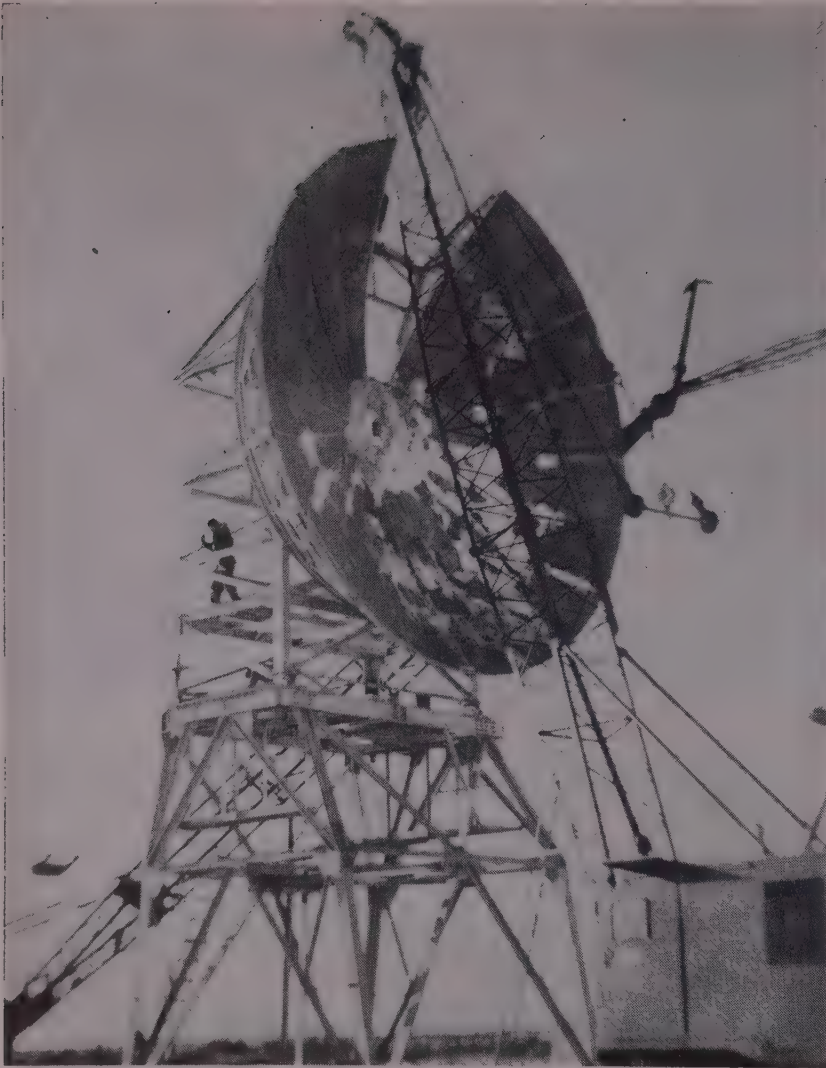
GALE WINDS and sub-zero weather gave erection crews a tough fight. After the lower part of the tower was in place, two cranes were used. One lifted 30-ft. pieces of the antenna and held it in place while the second filled in the supporting structure behind it.
