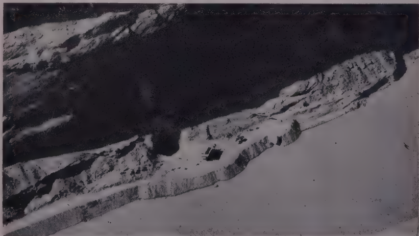
PORTAL of the diversion tunnel in the sheer canyon wall shows access difficulty, with muck used to build a working area at the river's edge.
