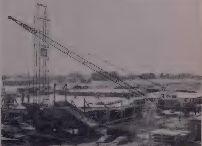
Lima Type 44-T truck crane, equipped with a 90' boom, placing concrete on a new junior high school building, Dallas, Texas.
