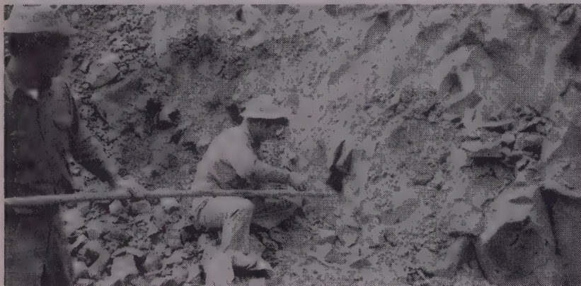
BLASTING CREW loads holes with sticks of dynamite. Crevices in the diced basalt make loading difficult. So far the material has averaged about \frac{1}{2} lb. of powder per cu. yd.
