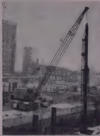
NEW YORK Pile driving
