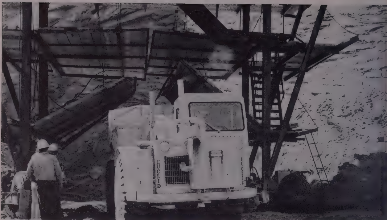
THROUGH the jumbo, with its lowest platform pulled up, comes the 12-yd. Euclid with a load of muck. The jumbo is mounted on rubber tires. Bur. of Recl. photo
