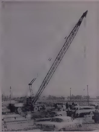
VIRGINIA Handling precast beams
