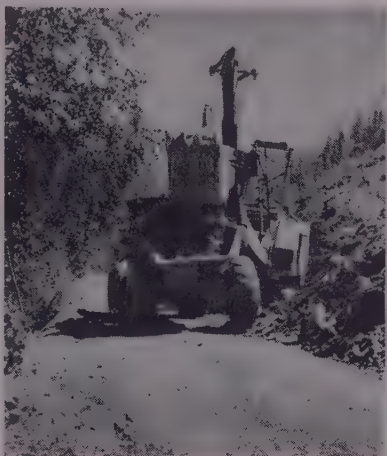
On this narrow ledge, 2 of Marrazzo's C Rear-Dumps and 2 competitive dump trucks were each loaded with five 2½-yd. buckets of blast-rock. Restrictive terrain temporarily made it necessary for loaded haulers to back up to 40' wide turn-around before starting haul.
