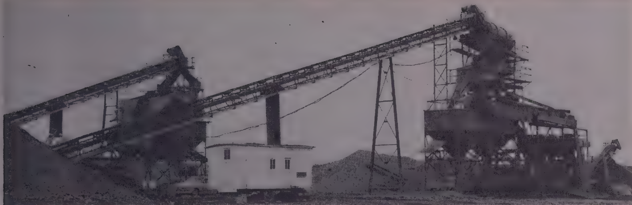
WASHING and screening set-up with Pioneer 405-W washing plant at the right topped by its 6x13-ft. scrubber. The Pioneer screening plant in the left background was used to size base material.
