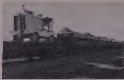
Lucin Cutoff —G-D Rotary 600 supplies air for dumping fill in Great Salt Lake.
