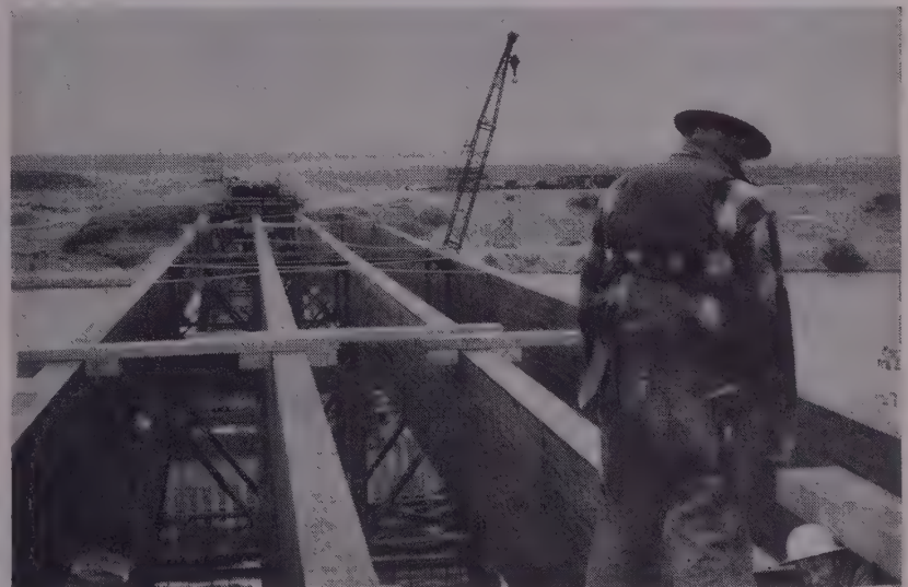
EACH of the fifteen 100-ft. spans consists of four glulam girders to carry the 24-ft. roadway. The structure will provide ready access to both sides of the Columbia River.
