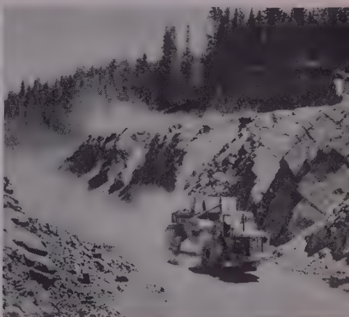
Hauling thru cuts previously carved-out, loaded Tournapulls attained speeds to nearly 30 mph, averaged 7.08 mph from start to stop on 1470' trip to the fill. Haul road presented a continuous succession of grades varying from 18% favorable to 10% unfavorable on the haul.
