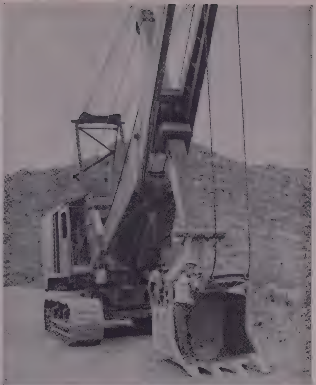
They are using two Gardner-Denver and two Ingersoll-Rand drilling rigs. At the right the Northwest 80D gets an oiling during lunch period.
