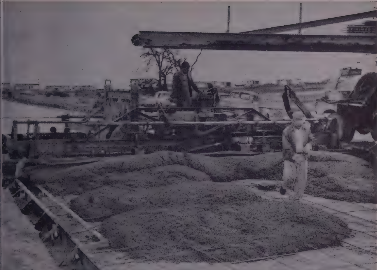
TEXAS CITY STREETS Contractor reported highest pouring ever. Credits Flex-Plane. Note amount of concrete in front of screed here.
