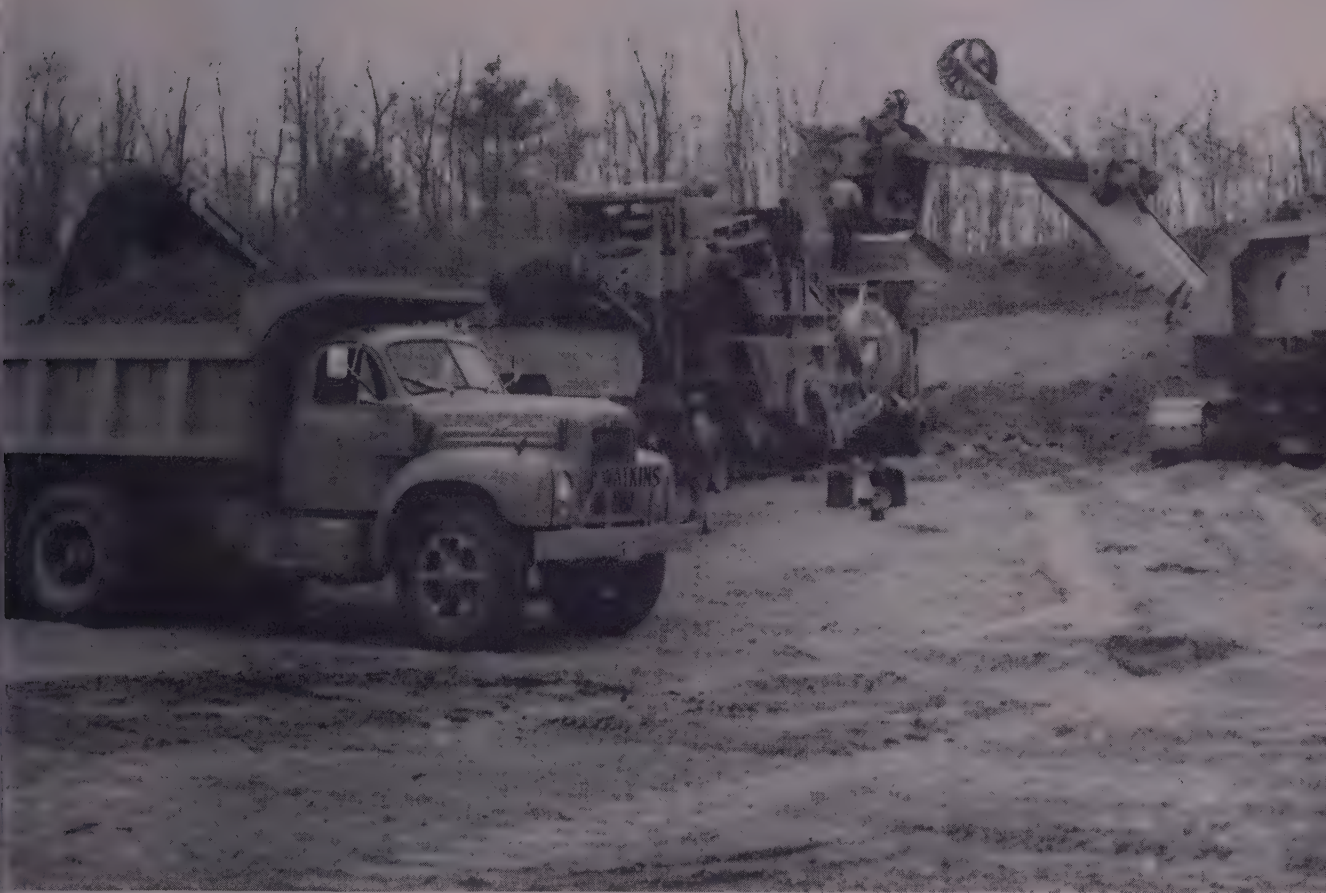
One of Watkins' 26 Macks receiving a load of crushed gravel from a crusher fed by a 1¾-yard shovel.
