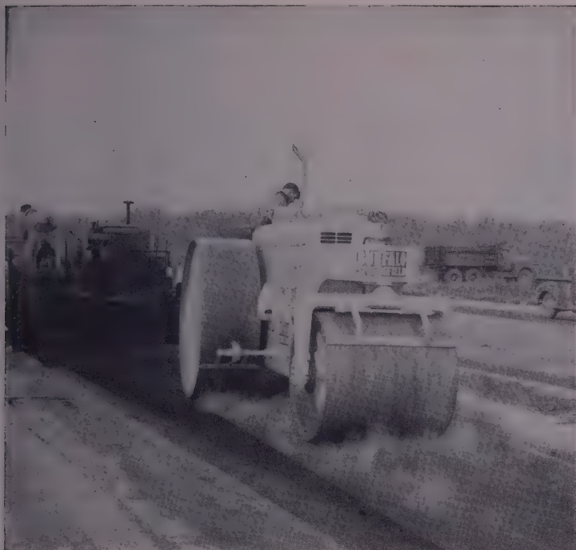
Buffalo-Springfield 3-Wheel Roller on a widening and bituminous resurfacing job.
