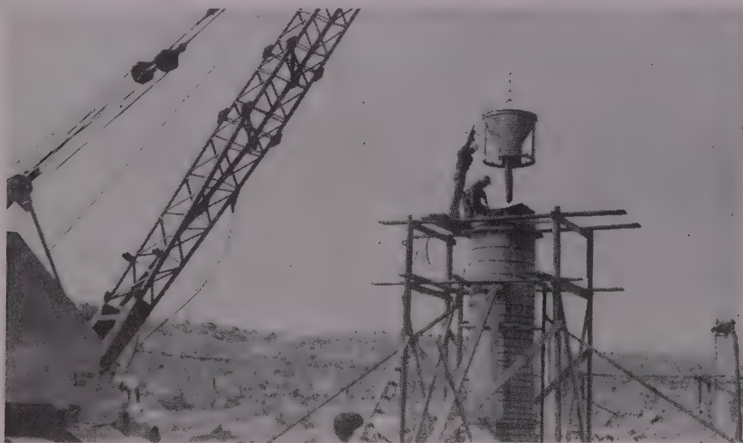
CONCRETE is dumped from a one-yard bucket into 48-in. cylindrical pier form for overcrossing structure. Forms are made of wooden barrel staves and steel banding.
