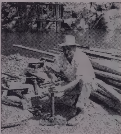
GEORGE BOROVICH checks one of the jacks which will be used to support forms at the top of falsework on the O'Bryne Bridge. Borovich is superintendent for Thomas Construction Co. See article on page 57.
