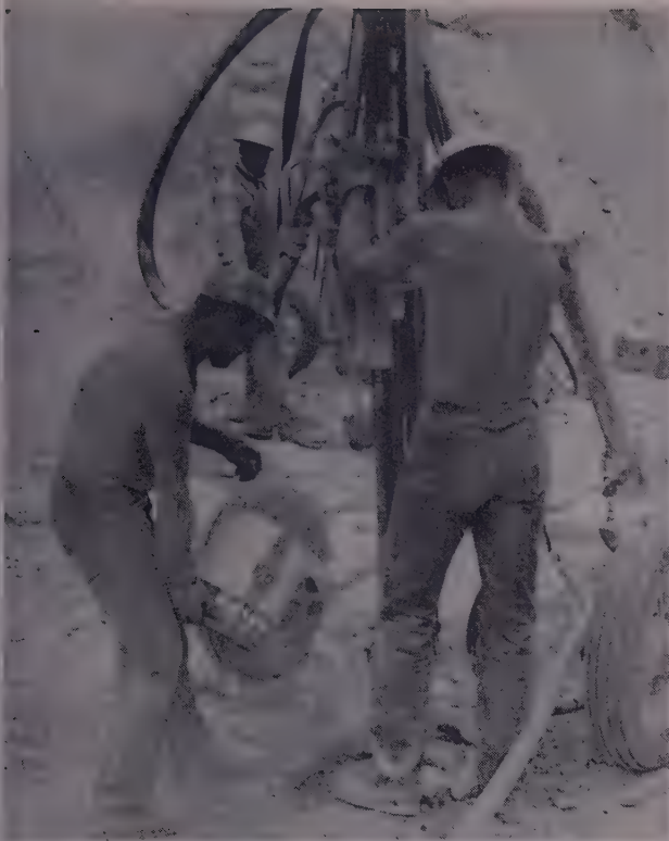
CONTRACTOR Wallace and Wallace has what many consider to be the finest drilling and blasting crew in Arizona at work on this job.
