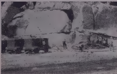
Wishon Dam—G-D rotaries power "Air Trac" and heavy-duty G-D 5 1/2" drill.
