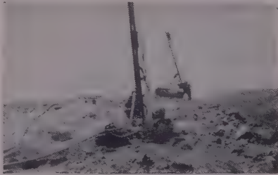
Dalles Dam —G-D "Air Trac" drills maneuver readily over rough terrain.
