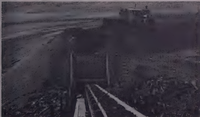
RAW GRAVEL with its tight coat of plastic clay is being moved by Cat and U-dozer into the feeding hopper to be moved up to the scrubber at the top of the washing plant. Note the hand-picked pile of wood and debris indicating the condition of the raw gravel.
