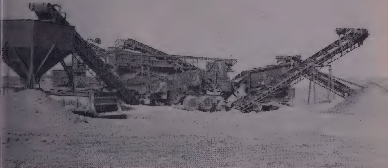
Portable A-W plant producing base material for large state highway job near Los Banos, California.
