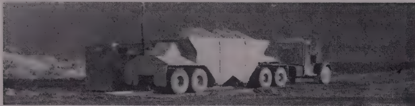
HERE is the two-hopper belly dump wagon manufactured by the contractor being weighed after leaving the crusher. The big rigs were capable of hauling over 36 tons.
