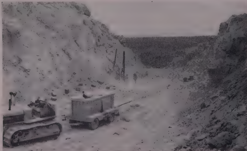
SOLID ROCK was encountered in some sections. The rock is very hard, very abrasive. Carbide drill bits required sharpening about every 35 ft. The deepest cut on the job is about 127 ft.
