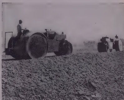
Buffalo-Springfield 3-Wheel Rollers speed compaction on fill consisting primarily of slate refuse from a coal mine.
