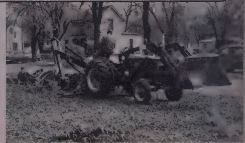
Mr. Reinhardt's HENRY BACKHOE digs a ditch for a sewer line in a Pontiac residential district. Though soil is laced with tree roots, digging goes ahead smoothly.
