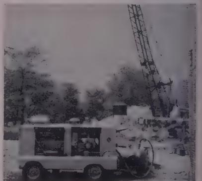
Chicago Filtration Plant —G-D rotary compressor sinks shaft to water tunnel level.
