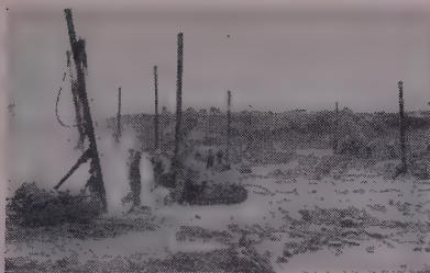
Beauharnois Canal and Lock—G-D "Air Trac"® drills on St. Lawrence Seaway.
