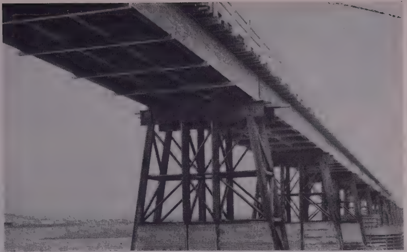
PIERS of welded I-beam design are supported on concrete footings. Concrete curtains protect the steel on the sides and the upstream edge. Fast dismantling and high reclaim value were important factors in selecting the glulam design.
