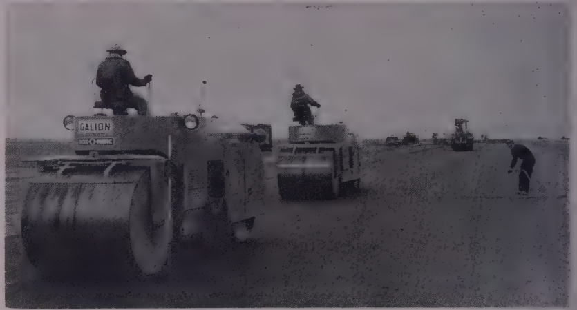
TEAM of Galion rollers compacting asphaltic concrete paving on the runway. Inspector is checking with a straight-edge. The 4-in. surface has a 45-in. base depth.
