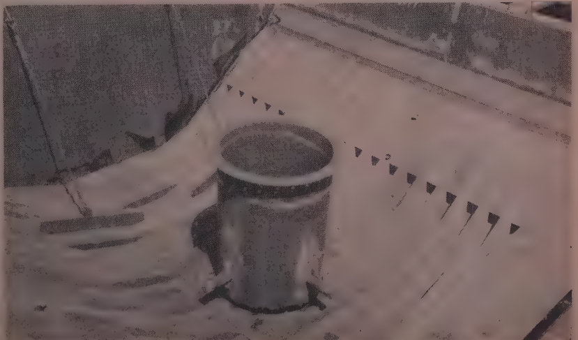
WOODEN FALSE bottoms in each cell kept water out. Jetting and pumping were done through a 30-in. pipe leading to top of caisson. Bottoms were knocked out when clamshells were needed.
