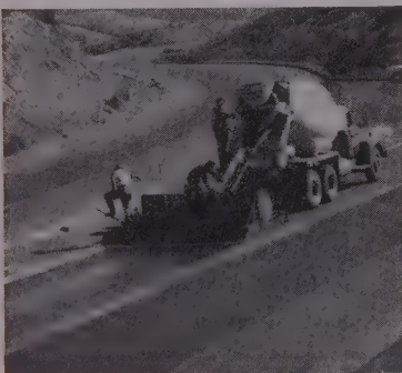
Applying Bitumuls Slurry Seal to existing bituminous pavement ahead of resurfacing.
