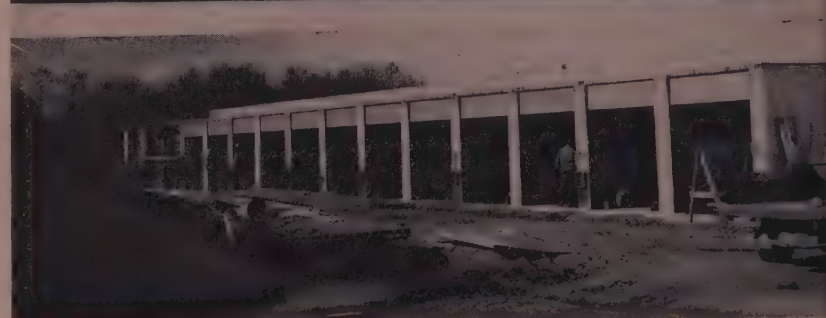
FOUR VIEWS of construction of one ammunition storage building are shown above in chronological order from top to bottom. Four men set forms in 3 days, strip them in ½ day.
