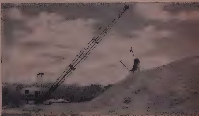
Lima Type 1201 dragline equipped with an 85-ft. boom, dredging channel into Biscayne Bay at Ojus, Fla. Approximately 250,000 cu. yds. of sand and coral rock will be moved to complete this job
