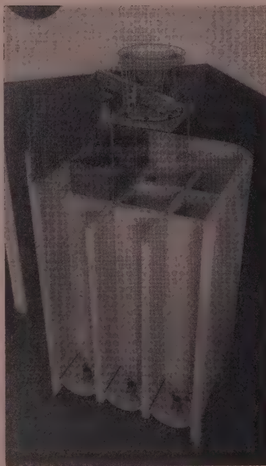
CUT-AWAY MODEL shows wooden false bottoms but without the dredging pipes leading to the top. Although each false bottom was fitted with a 30-in. dredge well opening, jetting and pumping was done only from the four interior cells to minimize sloughing of material from outside the caisson. The rotating concrete distributor has an extendable horizontal conveyor, was designed by contractor, built by Noble Co.
