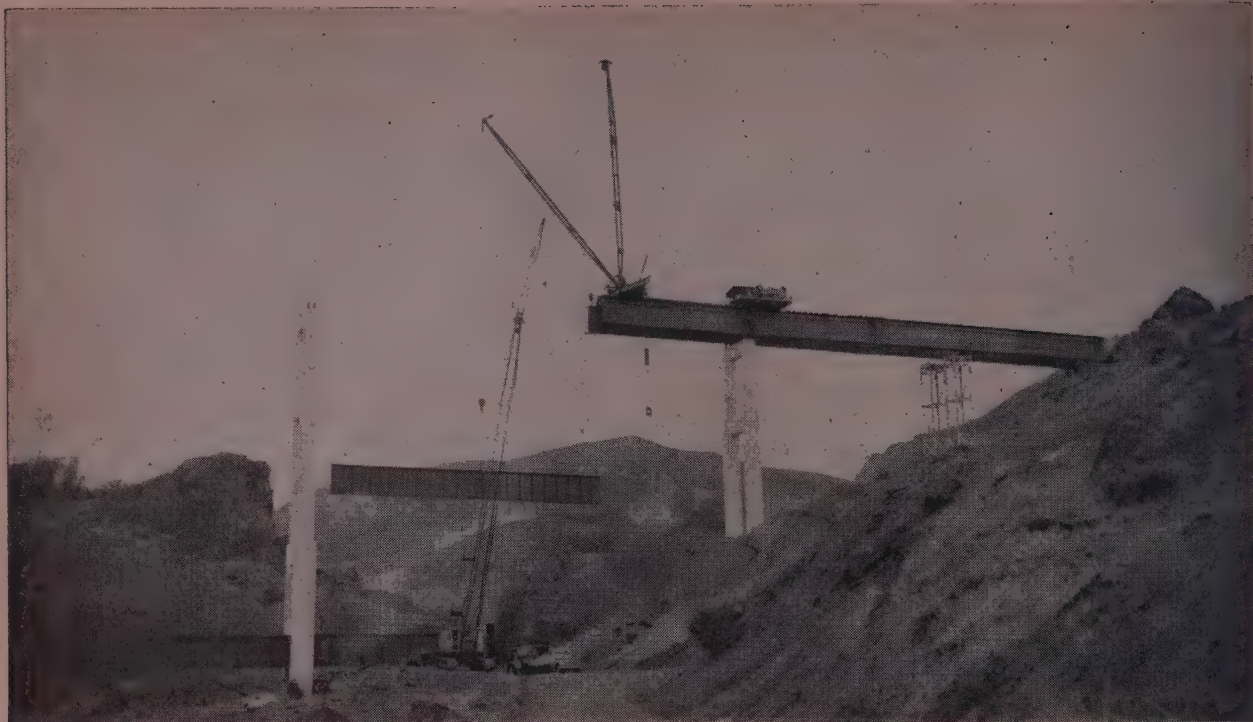
PLATE GIRDER weighing 34 tons is being raised into place by derrick poised on end of temporary cantilever. When girder is in place and the
