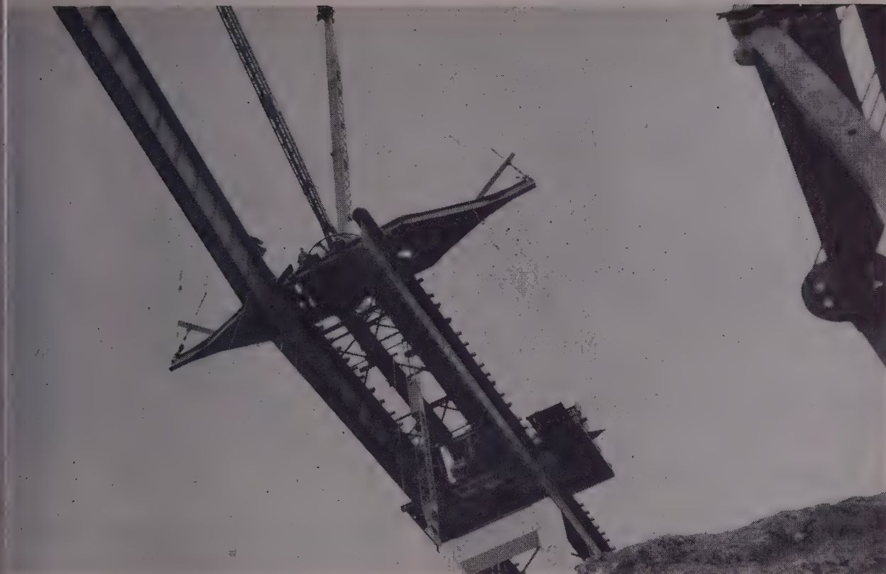
JEHLHEM PACIFIC steelworkers prepare to bolt a splice as girder is swung into position. Derrick platform extends to each side of cantilever
