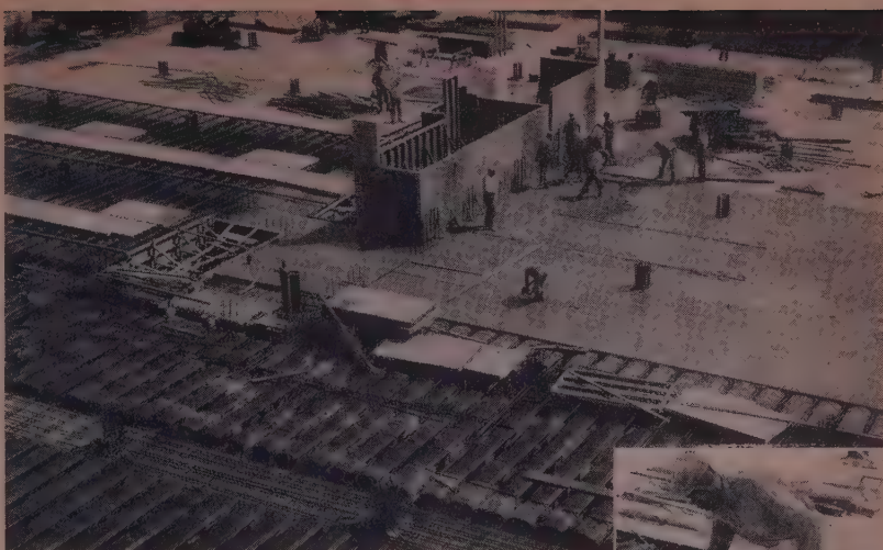
Above: Pouring section of first floor of new 5-story Herman Miller Bldg., Dayton, Ohio. Right: Close-up of operator using a Master "1-Man" vibrator between closely spaced reinforcing rods.
