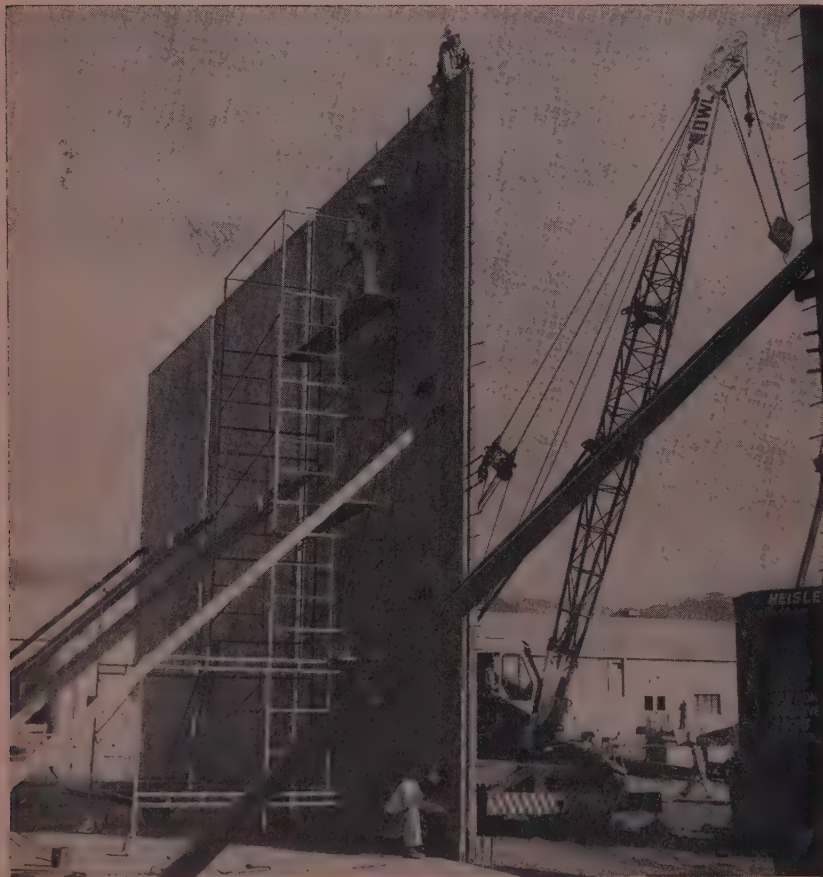
WORKMEN on rolling scaffold remove steel angles from the pickup points. Slabs were cast in stacks 5 units deep. Slab weights ran as high as 33 tons.
