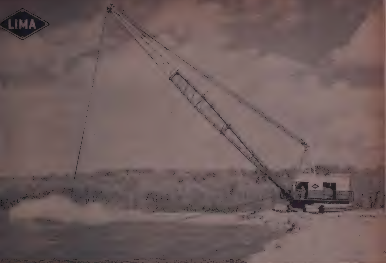
Lima Type 1201 dragline equipped with an 85-ft. boom, dredging channel into Biscayne Bay at Ojus, Fla. Approximately 250,000 cu. yds. of sand and coral rock will be moved to complete this job
