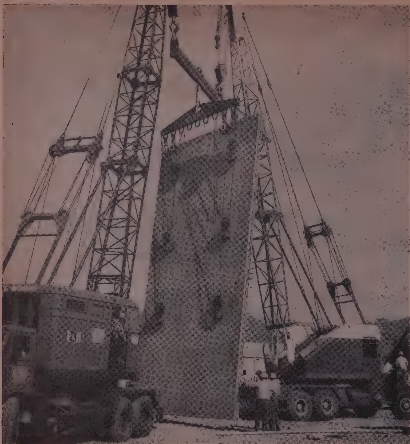
SELECTION of pickup points must arrive at a layout that will keep erection stresses within allowable limits. Next, inserts must be designed to provide satisfactory anchorage and to allow easy cable attachments to the panel (see diagram at right).
