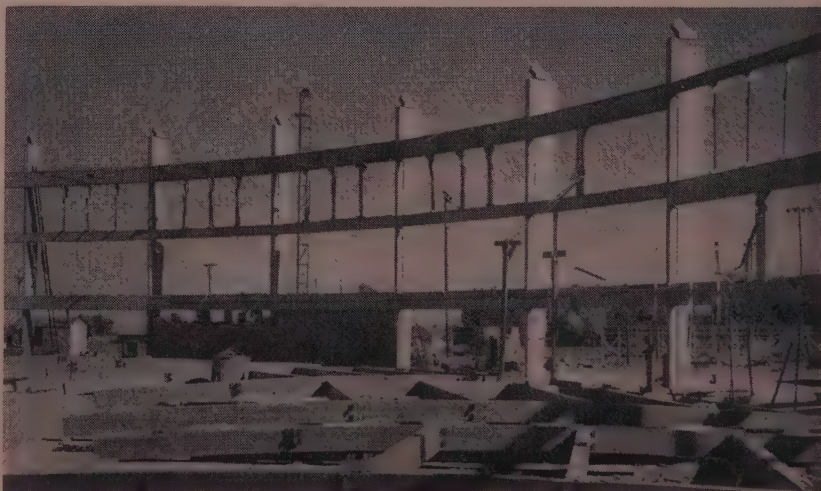
A RING of concrete columns 39 ft. high provides support for the ribs of the dome. The steel tension ring (not yet in place) connects the bearing shoes at the top of the columns.
