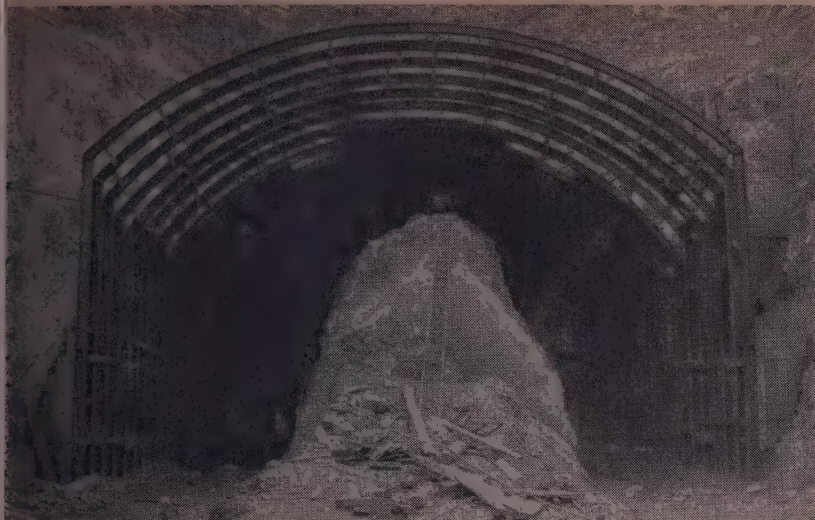
PORTAL diameter of 50 ft. tapering to 34 ft. called for two separate headings in the tapered section 50 ft. long. This procedure permitted early placement of steel. It also eliminated the need for special drill platforms, since the jumbo was designed for the 34-ft. diameter.
