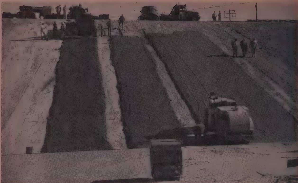
THREE TEST STRIPS are shown during construction on the side slopes of newly-excavated North reservoir. Bigge Drayage Co. winch trucks
