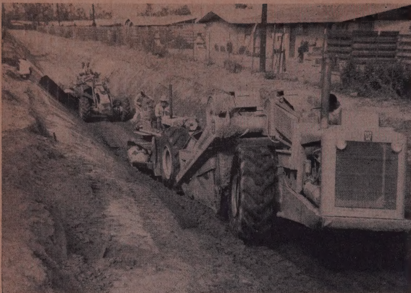
A LeTOURNEAU-WESTINGHOUSE scraper gets a boost during the excavation of the \frac{3}{4} -mi. channel while a motor grader rough grades the sides. Right-of-way was only 35 ft.
