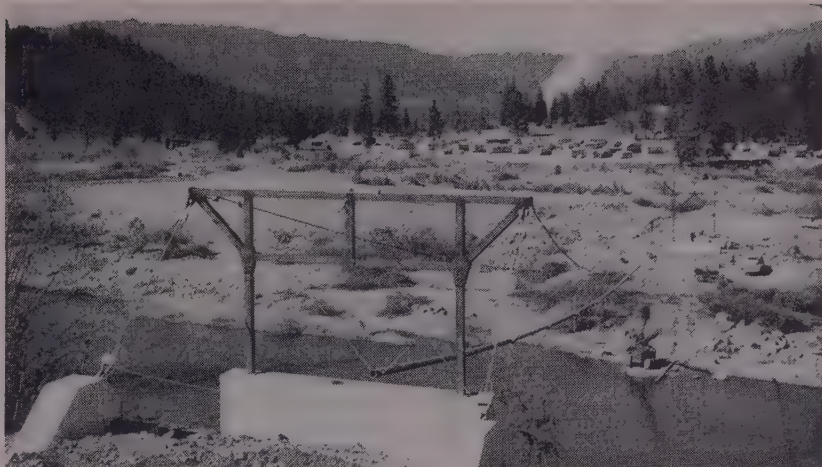
CAMP SITE type of area in the Trinity River valley, now occupied by trailers housing employees on some of the preliminary contracts. Pipe on suspension span is sewer outfall.
