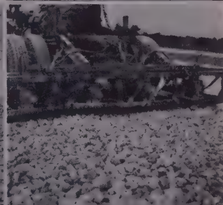
4 COMPACTING UNITS just fit this widening job. Change required only a few minutes.
