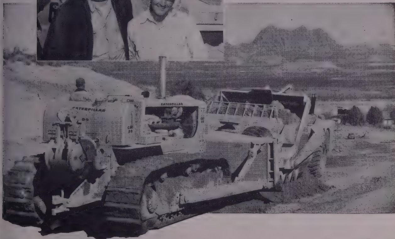
Close-up view of the Cat D9 push-loading a DW21 and scraper near Globe, Ariz. Twin Disc Torque Converter components are standard in the torque converter version of the powerful D9 and D8. Inset (left) shows Roy E. Hale, Superintendent, and Link L. Colvin, Co-owner of Copper State Construction Co.
