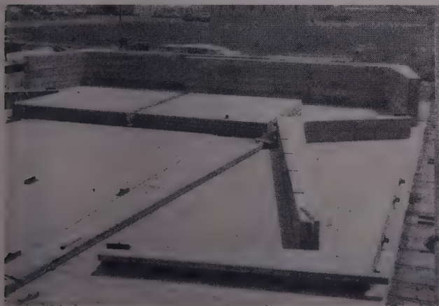
ARCHES of precast concrete of three-hinge design span 75 ft. to provide a clean floor area. The second floor is a 55 x 28-ft. slab 7 in. thick poured on the ground and raised on pipe columns.
