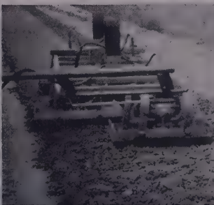
3 COMPACTING UNITS in tandem and staggered. One of many hook-ups to exactly suit conditions.
