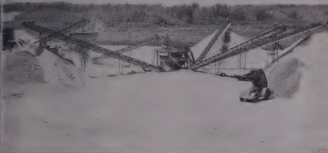
A-W Crushing Plant of J. J. Cronin Co., showing primary crusher at extreme left. Washer is in center of photo. Washed sand is delivered by the conveyor on left of washer, specification material by the three stock-piling conveyors at the right.
