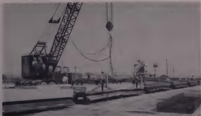
SPECIAL FORM-STRIPPING RIG was able to strip a panel and move on to the next within 3 min. Panels are left in forms 48 hr., then stripped and treated with Hunt's Process.
