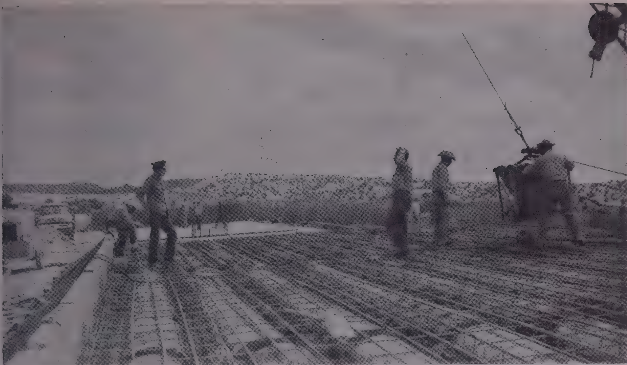
SONOVOIDS were used to lighten deadload. Contractor solved problem of resisting the flotation tendency with straps, No. 9 wire, reinforcing steel, and U-bolts. Earth fill made access easy. When fill had been
