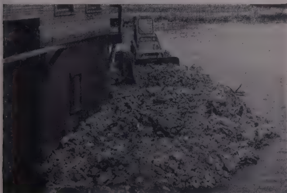
Rip-rap — old brickbats and concrete dozed into river to protect building.
