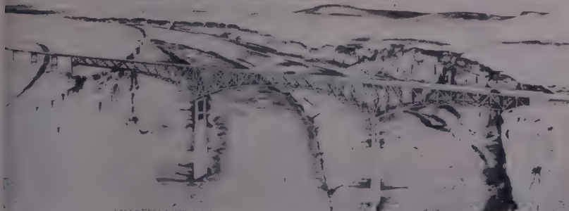
TEXAS HIGHWAY DEPARTMENT sketch of 1,310' long bridge on Highway 90, near Langtry, Texas. The 3-span continuous deck truss cantilever structure runs from rim to rim across top of the canyon—272' above the traditionally treacherous Pecos River.
