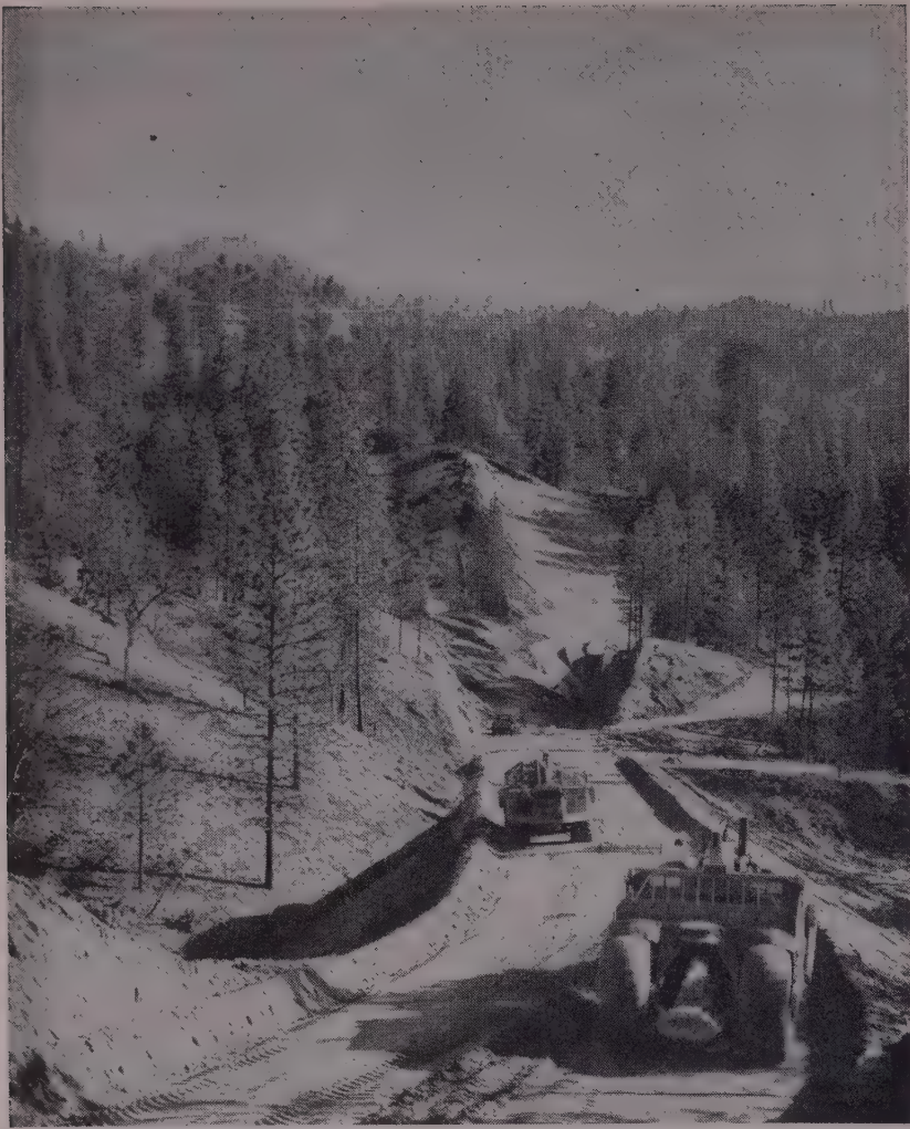
ACCESS ROAD is pushed through mountain areas to reach site of Trinity Dam. Nearest railroad facilities are 40 mi. away. Road will connect with U.S. 299.
