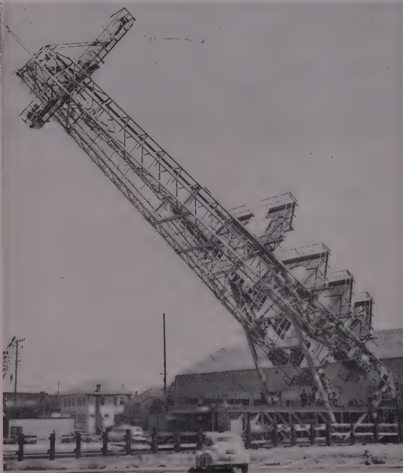
RISING into position, this 120-ft. tower can transport, tilt upright and provide servicing platforms for various types of guided missiles. Self-contained power units move the tower on two parallel sets of standard railroad rails.
