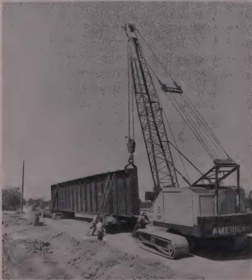
THE CRANE also escorted the truck to the site in order to move the rear dolly to the outside of sharp curves in the road. Three cranes lifted girders onto the bridge piers.
