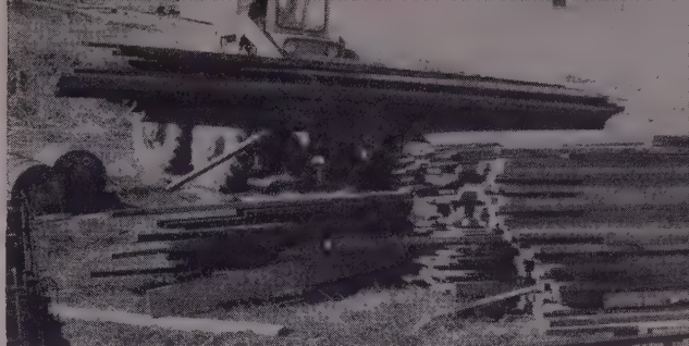
Lumber — as much as \frac{3}{4} of a truck load (3500 to 4000 lbs) unloaded at once, stockpiled, later carried to hoist.
