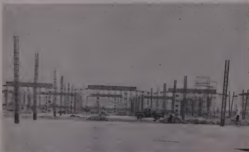
EARLY CONSTRUCTION view shows reinforcing steel for the continuous framing. Re-steel is being supplied by F. A. Klinger Co. of Stockton, Calif. An estimated 126,400 bbls. of cement is being trucked to site from San Andreas plant of Calaveras Cement Co.
