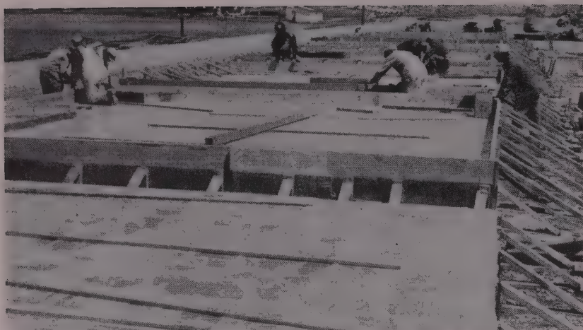
TILT-UP contractors can use polyethylene film as a bond breaker between slabs cast on top of each other. Film can be used the same way in lift-slab construction.
