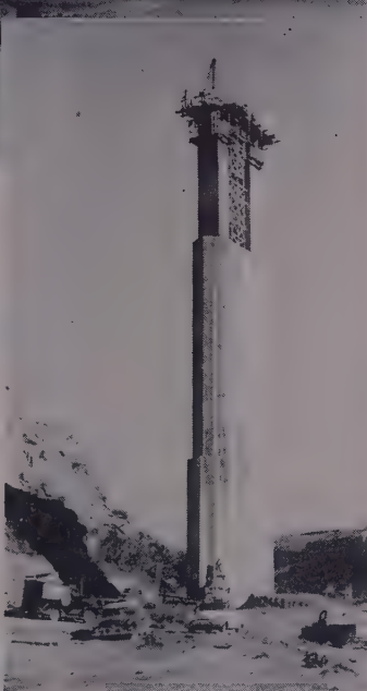
BOTH RECTANGULAR COLUMN LEGS of upper tier were poured simultaneously. In about 90% of the pier elevation, alignment is within 1/16".
