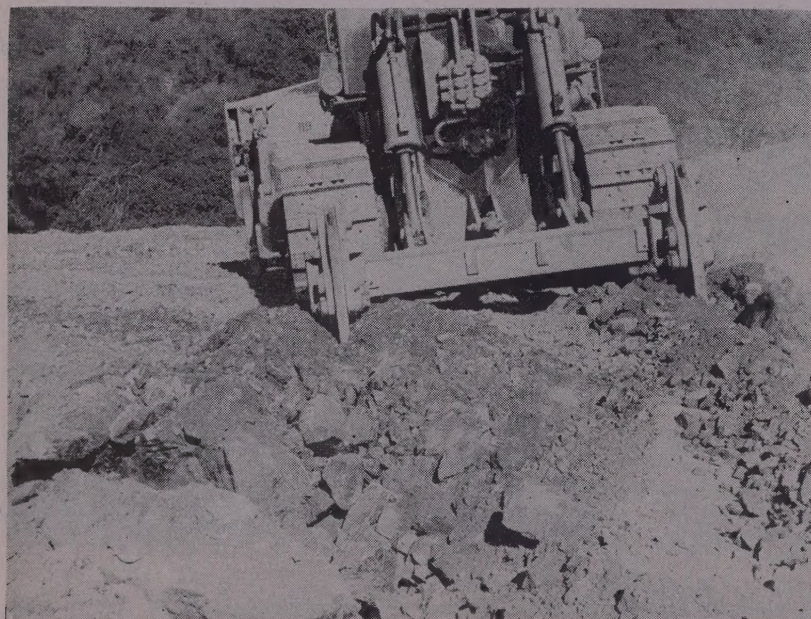
RIPPING through tough granitic soil with soil breakers is much smoother since flat horizontal plate holds tooth and shank in ground at full depth. Note great width of disturbed soil. Shank is knife-edged to facilitate rock fracturing. Breakers were developed in 1955 for agricultural use.
