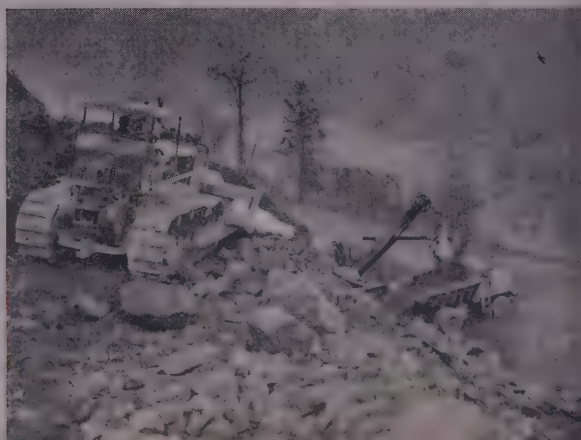
International TD-24 dozes shot-rock down the slope to 1½ cu yd shovel and easy-loading International "65" Payhauler. 250,000 pounds of dynamite were used...about a pound to every 3 yds of rock!
