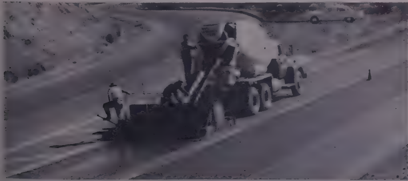
BITUMULS SLURRY SEALING ahead of resurfacing on the existing bituminous roadway.
