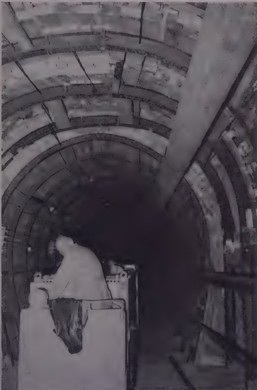
AT THIS POINT the contractor changed from conventional pile driving to the partial shield. Section in foreground was made several feet larger to permit assembly of shield. Note that portion driven with shield is very uniform, shows efficient use of lagging.
