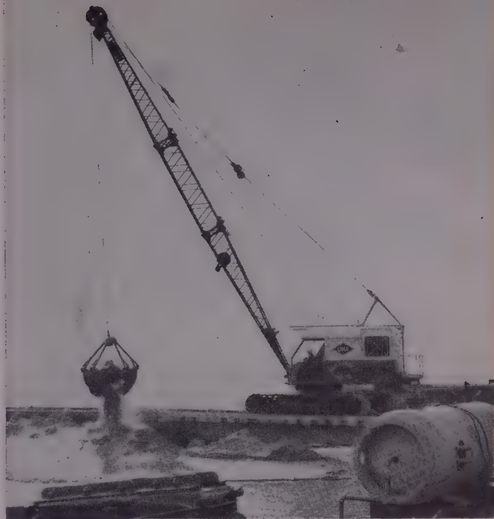
Lima Type 604 dredging sand from single-cell cofferdam prior to driving piling.
