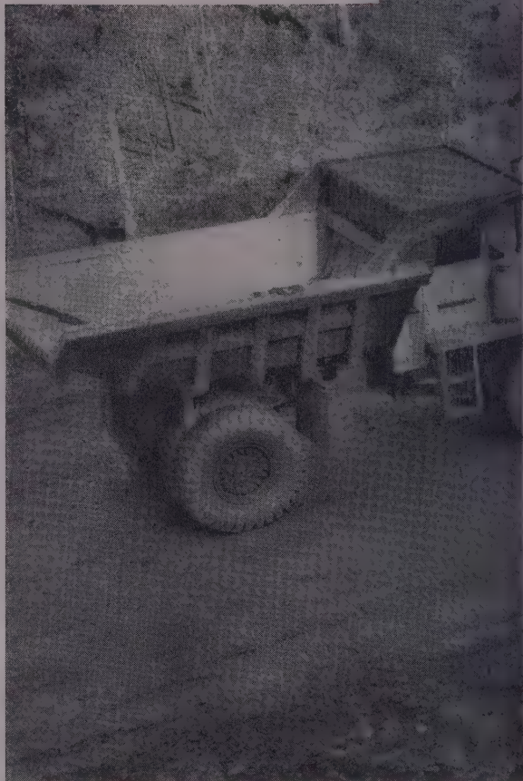
International TD-24 dozes shot-rock down the slope to 1½ cu yd shovel and easy-loading International "65" Payhauler. 250,000 pounds of dynamite were used...about a pound to every 3 yds of rock!
