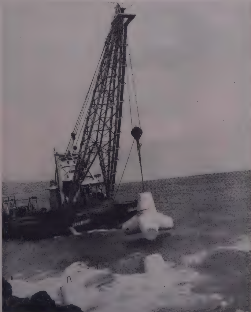
PLACED by derrick barge, the pods go into water up to 40-ft. depth and extend 13 ft. above low tide level. Rounded surfaces and interlocking action are two special design features.
