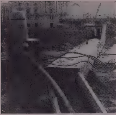
BERKELEY TURBINE pumps are handling from 100 to 300 gpm. Water passes through settling trough so that sand will not be delivered into the city's storm sewer system.
