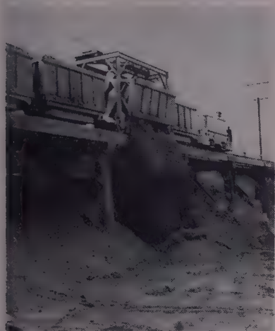
EXCAVATED MATERIAL is dumped from cars, then loaded into trucks by front-end loader. Madsen cars, Goodman locomotives are used.
