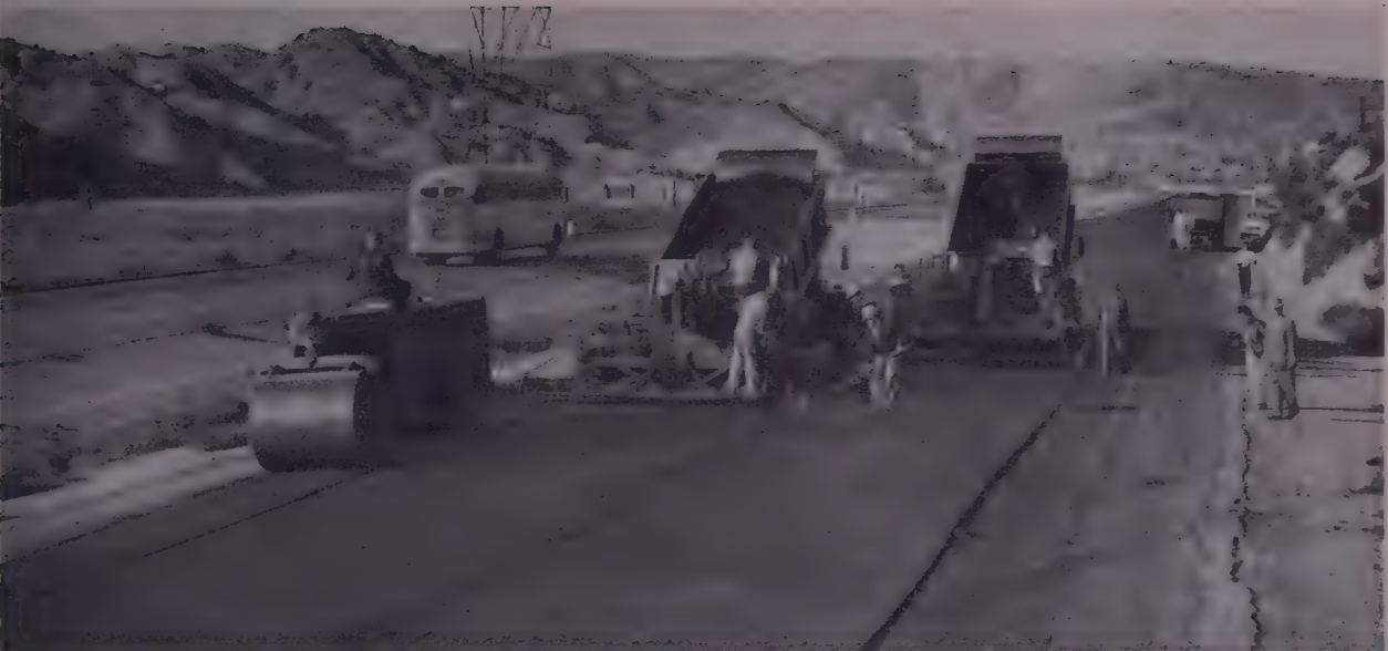
TANDEM SPREADING of the Asphaltic Concrete speeded the resurfacing work as . . .
