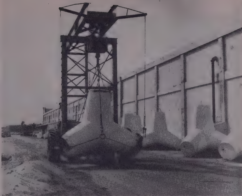
FROM casting bed to storage yard, the pods were handled by Tournacrine. This same machine also moved the units from yard to the loading dock. Note the special lifting harness.
