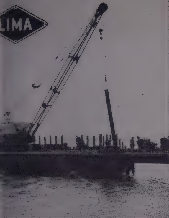
Lima Type 604 lowering pile into position on the Manahawken Bay Bridge, Ocean County, N. J.
