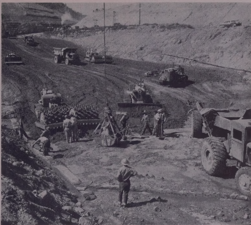
LOOKING TOWARD right abutment during placement of impervious core materials following clean-up of the cutoff trench. Dam volume is 2,650,000 cu. yd.
