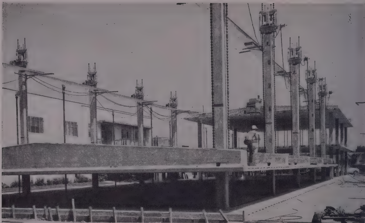
TWO STAGES of lifting in progress with final position shown in the background. Being raised by the ten jacks of Western Concrete Struc-
