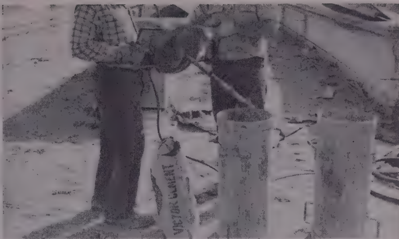
GROUT HOMOGENIZER has a one horsepower electric motor turning a 30-in. long shaft which mounts three 4 1/2-in. blades. The can is one foot in diameter and 30 in. long.
