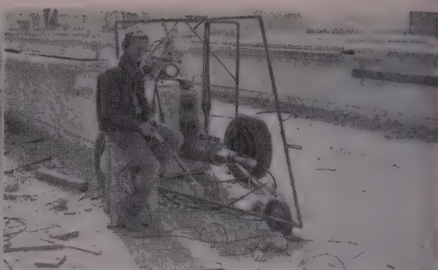
electric hydraulic pumps and are carried with a portable rig made out of reinforcing bars. The BBR system of stressing was used.
