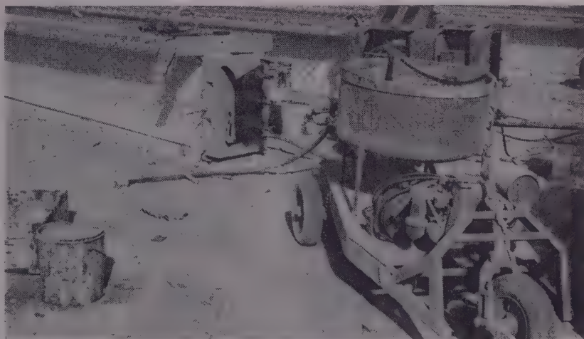
GROUT is returned to hopper on portable grout pump through rubber hose from far end of girder. There is no spillage and constant motion prevents it from stiffening.
