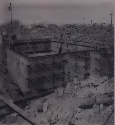
FOUNDATION —Erects fast . . . two men only on inside; no liners on outside.
