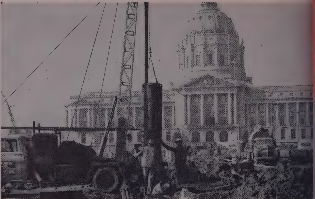
RUBBLE from pre-1906 earthquake buildings held up excavation on construction of underground exhibit hall. Drilling subcontractor found
