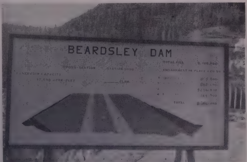
SIGN overlooking dam is kept up-to-date to show visitors the amount of fill remaining to be placed. Above picture was taken in late fall when 600,000 cu. yd. were left to place and compact.
