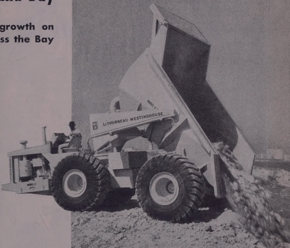
Tournapull dumps a load of rocky spoil blasted from the tunnel. Across the Bay can be seen the tall commercial buildings of downtown Havana.
