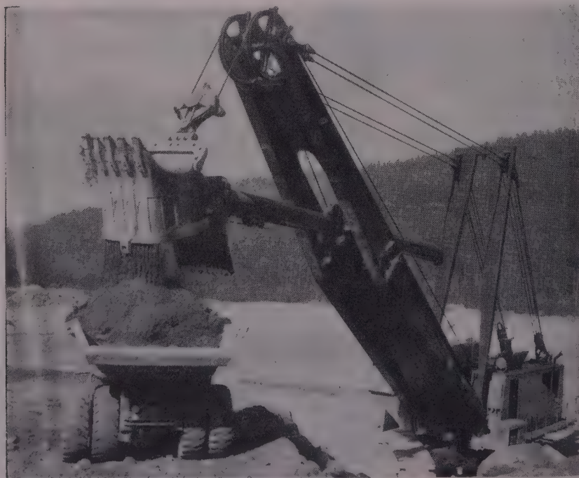
LOADING pervious zone material this Maniotowoc handled a 5½-yd. bucket. During peak operations fill in all zones was placed at a rate of more than 100,000 cu. yd. per week.
