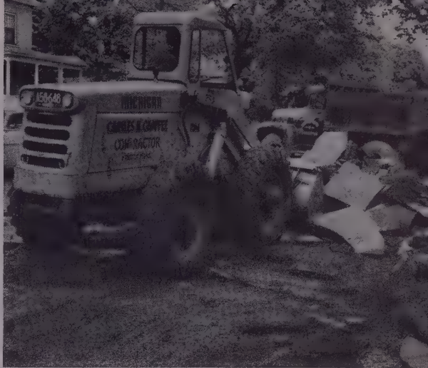
Breaks, loads asphalt —Before resurfacing street in Worcester, Mass., Contractor Charles Chaffee uses 1 1/4 yd Michigan to strip old asphalt. No "ramming" is required—powerful breakout quickly shatters paving.
