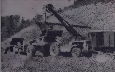
The Athey PR15-Cat DW15. Hauls 22 tons of rock or other material at speed to 31.3 MPH.
