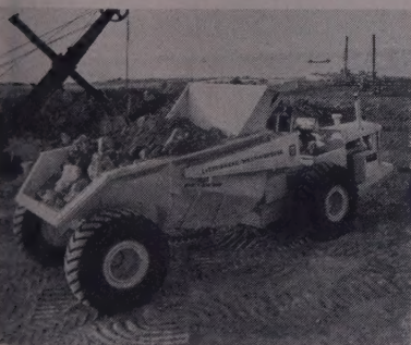
Tournapull Rear-Dump is shovel-loaded with 15 cu. yds. of blasted rock, excavated for the eastern approach to the "Tunnel of Havana". Tournapulls traveled around the Bay from the dock in the city, to this work site at tunnel entrance, under their own power. The 8-mile trip took about an hour.
