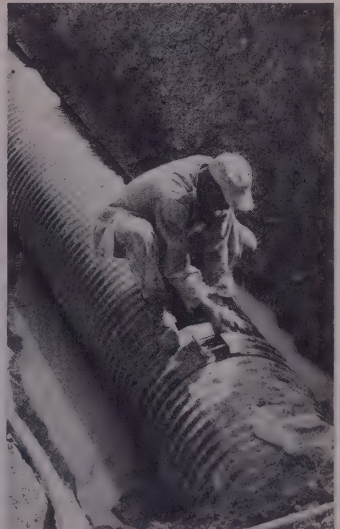
Joints can be made quickly and easily. Here one man tightens the two bolts on a connecting band with a hand wrench.
