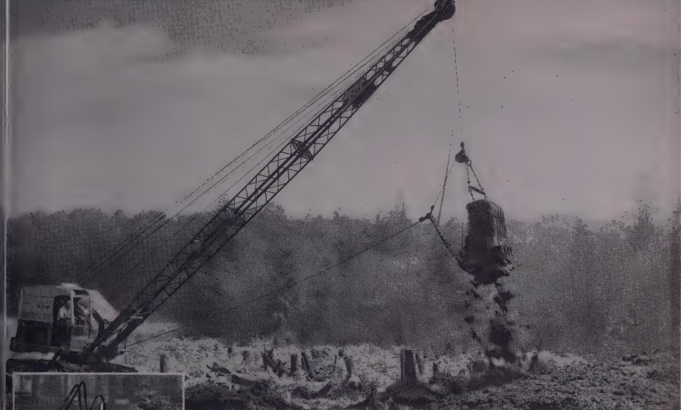
Cutting a new highway through a peat bog, 15 feet deep in spots, is this \frac{3}{4} -yd. Bucyrus-Erie 22-B dragline owned by K. L. Goulter & Son, Seattle. The job was located between Lake Stevens and Everett, Wash.
