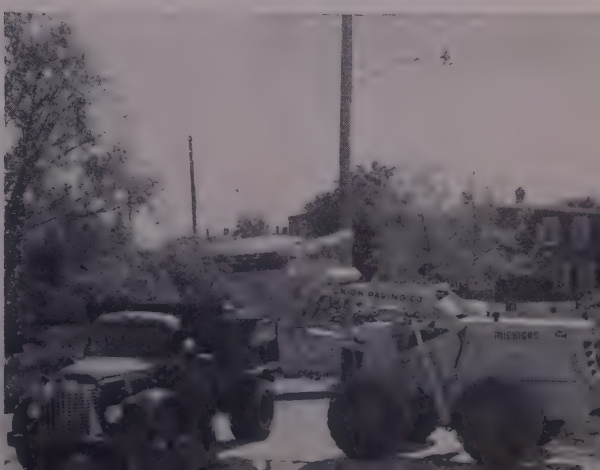
Breaks, loads concrete —On Philadelphia city street repaving job, Union Paving Co. breaks and loads 4 to 6-inch concrete slab with this 2 yard Michigan Model 125A.
