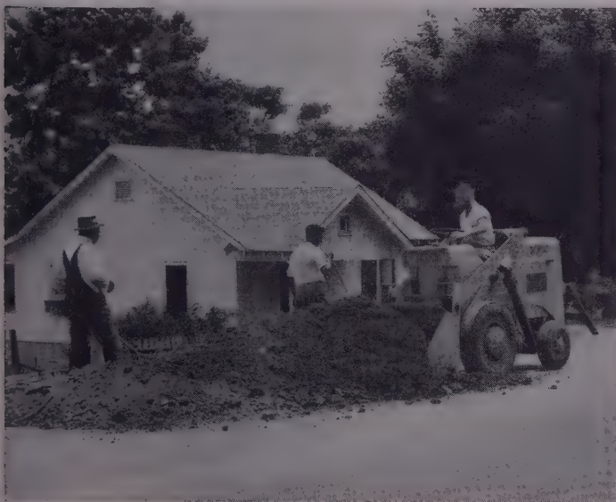
Cleans pavement —Highway must stay open said Nashville officials, so Wright & Lopez do cleanup with small, agile 16 cu ft Michigan. Only 4'2" wide, 10'8" long, unit works rapidly, doesn't block traffic, doesn't damage newly-set pavement.
