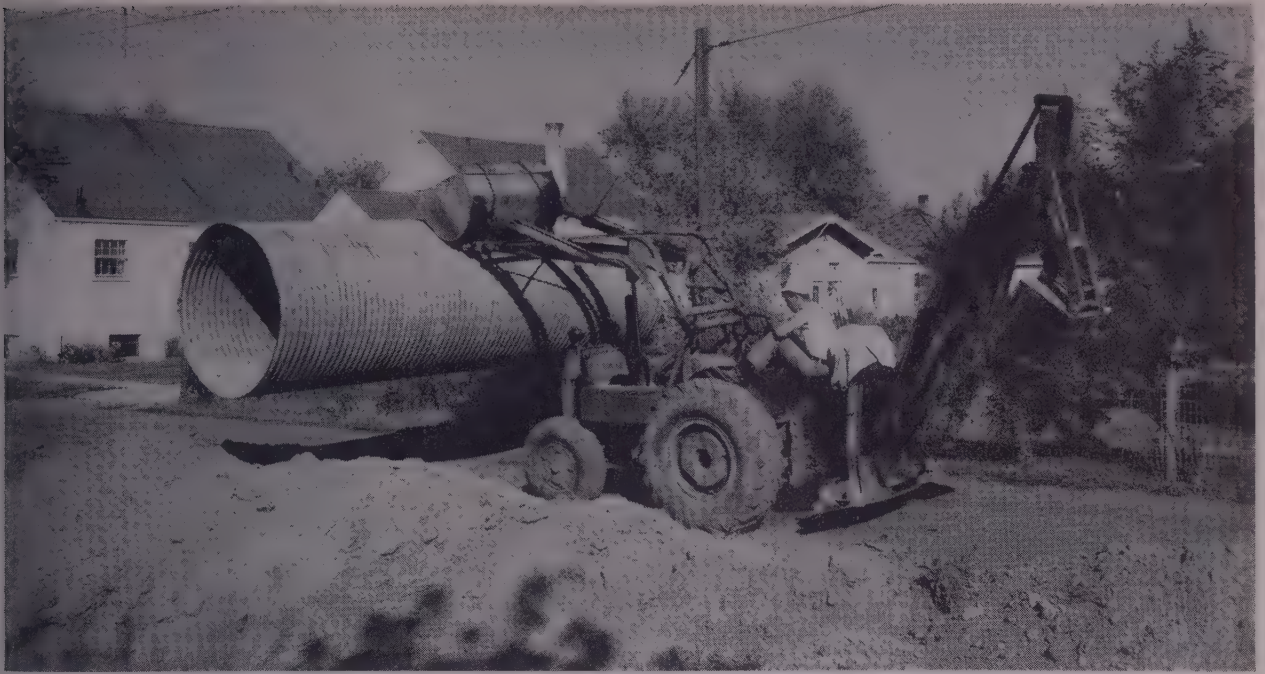
No special lifting equipment needed. The machine that dug the trench for this job was also used as a hoist in laying the pipe.
