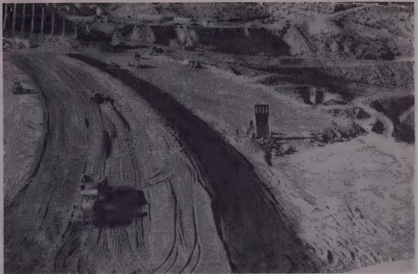
ZONES are clearly visible in this view of the top of the embankment. Beardsley contains rolled earth, sand, gravel and cobbles, with dumped rock on the upstream and downstream slopes.
