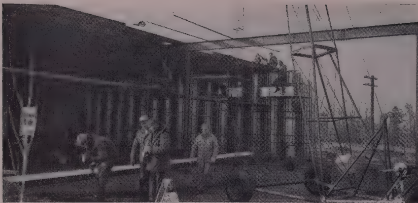
FAST AND SIMPLE erection procedure builds walls and roof. The crew is applying adhesive for the neoprene joint strip before the panel is lifted to position on the roof.
