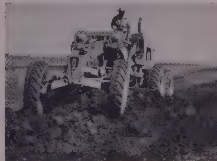
Amis Construction Co., of Oklahoma City, Okla., uses one of its 6 Adams 150 hp 660 graders to spread fill on Kansas Turnpike.
