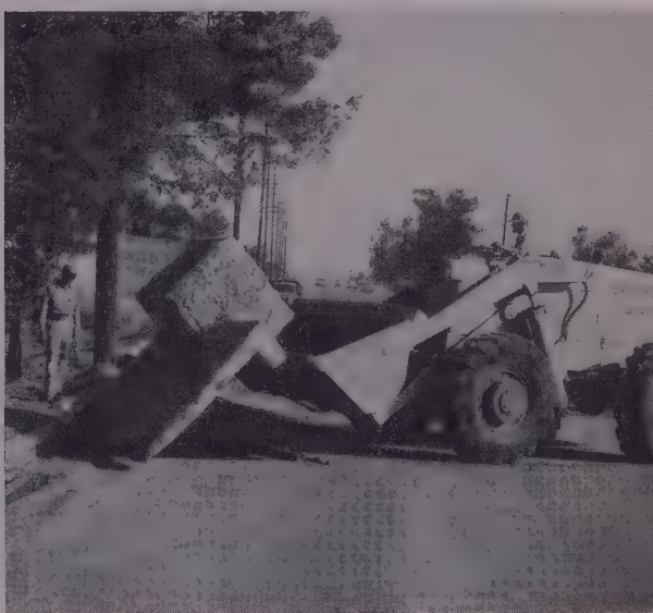
Removes sewer cover —When other big loaders failed, Kirby-Erwood's 133 hp Michigan succeeded in prying off this 2-ton concrete cover. Assignment was part of cleanup before widening Los Angeles freeway.
