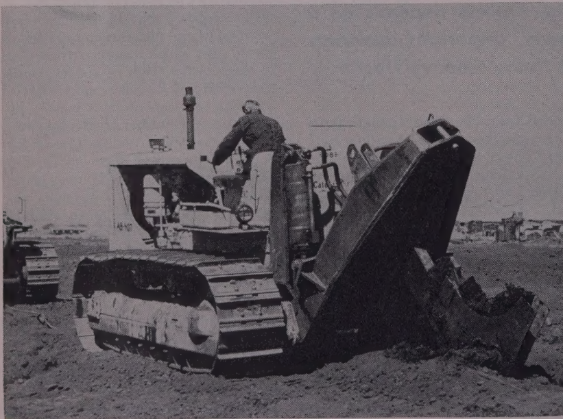
ADAPTED from early rippers is this cable-plough which buries telephone or power lines. The cable is fed through the hollow tooth as the plough is pulled forward.
