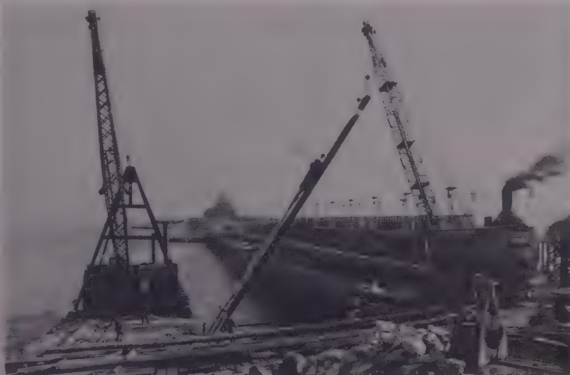
A DOUBLE-ACTING hammer shown driving batter piles using an H-beam spud. The hammer is fastened by grapples on the flange of the beam and slides along it. Maneuverability is a feature.
