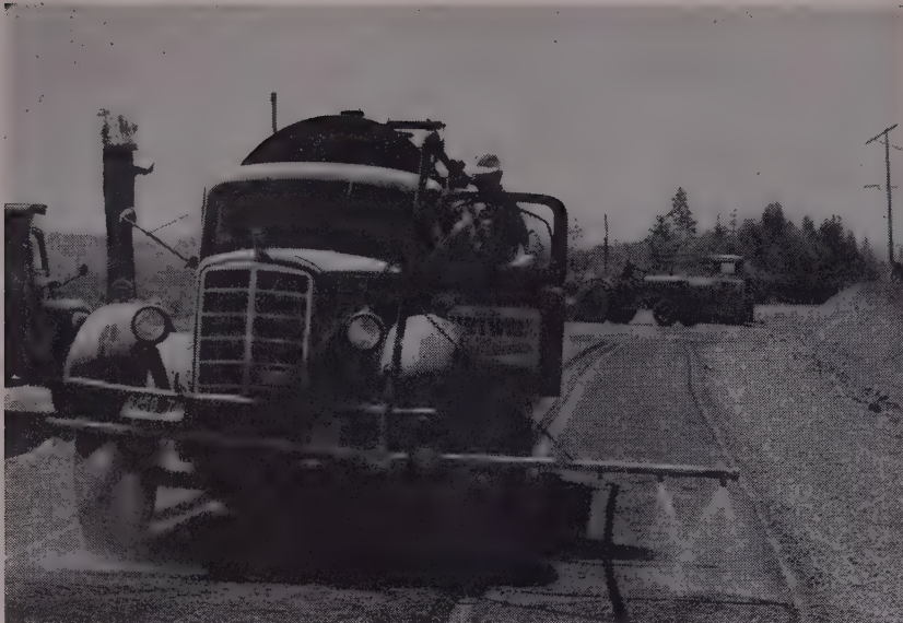
MOISTURE of the surface was maintained during final rolling by applying a mist spray. After the final pass of a steel roller the surface was sealed with asphalt emulsion.
