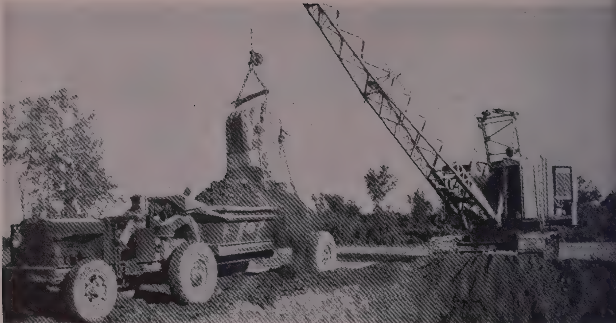
AN EARLY model bottom-dump tractor trailer unit on truck tires. Pneumatic tires introduced the modern age of earth-moving equipment. The
