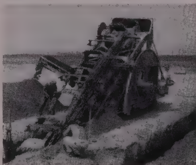
Here's a ladder-type Trenchliner worth looking into. This general-purpose 250 digs 16 to 42 in. wide, 12½ ft. deep. When equipped with dual booms, it digs 5 ft. wide, 8 ft. deep. Parsons line offers all sizes, types, on crawlers or rubber — also "big-inch" and "middle-inch" wheel-type Trenchliners.
