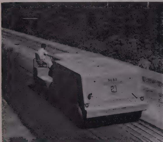
THREE passes of the Sta-Bilt Compactor were enough to secure the 95 % compaction on the 5-in. lift of stabilized base.
