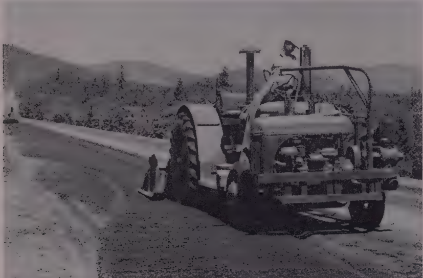
FINAL mixing and blending operation of the two Seaman-Andwall Trav-L-Plants was done in a "figure-8" pattern which aided in reducing all inequalities in the mixture.
