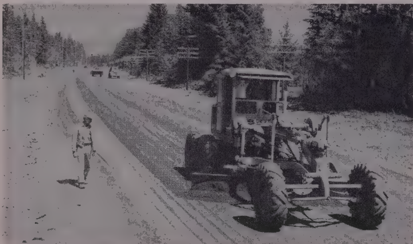
SURFACE of the soil-cement left by the mixing machines required only a small amount of grader work. This No. 12 Caterpillar is doing final blading behind the pneumatic compressor.
