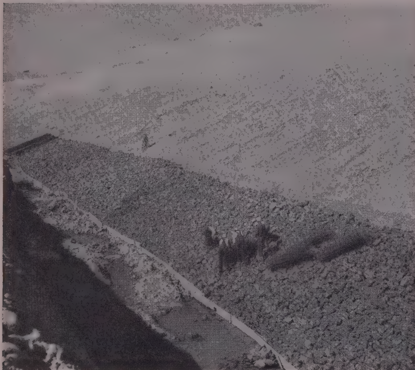
WORKMEN place covering layer of 6x6-in. steel mesh over 2-ft. layer of dumped rock. Rock blanket is slush grouted for lower 15 ft. at toe of slope for greater strength.
