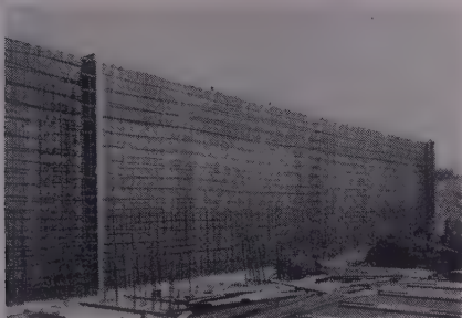
FLUSH DESIGN —Simplifies stacking the forms at job site. All Ply's weigh less than 5 psf.
