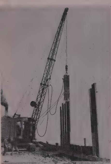
HAMMER with "pants" driving interlocking steel sheet piling. The pants align the suspended hammer over the pile, unaffected by any release of the load line.
