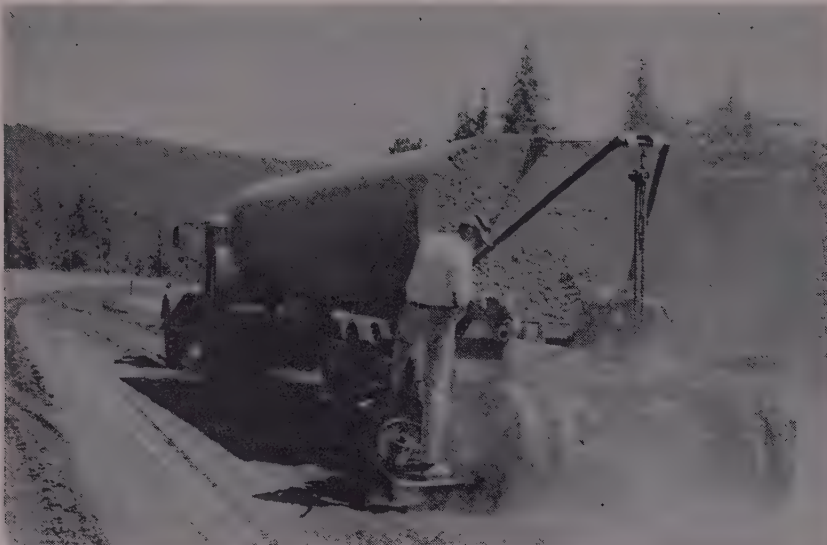
PROPORTIONED at 4½ % by volume, bulk cement was added through a Hercules spreader. Frequently, the spreader was hooked directly to the transport truck, bypassing the job storage silo.
