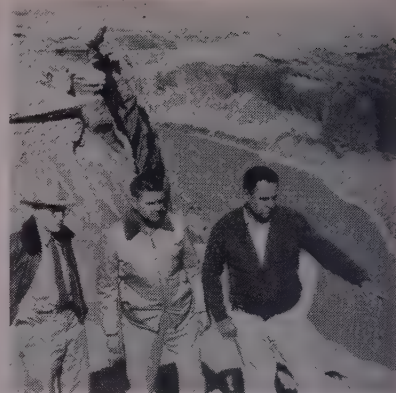
Directing the tunnel contract are (left to right): E. M. Cooper, project manager; C. E. Thompson, project engineer; and F. C. Jackson, company general superintendent. E. C. Steph is project superintendent; Clyde H. Jackson, purchasing and contracting officer.
