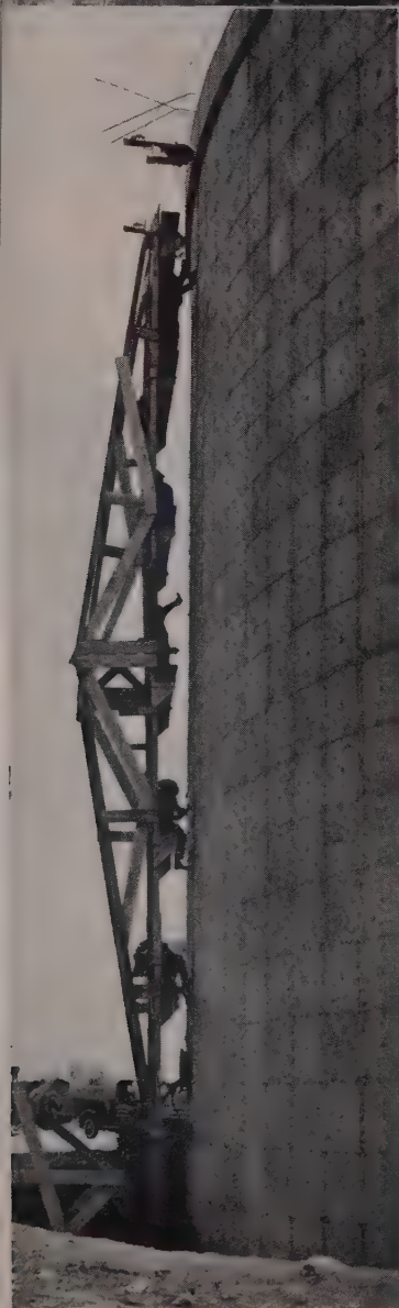
5 MEN ON ROLLING TRUSS removed form ties before prestressing operation.
