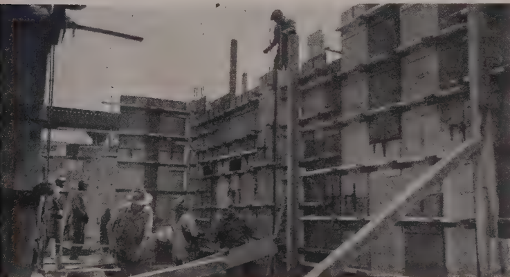
$3 Million ELEMENTARY SCHOOL —Plywood face and rigid locking of forms by Combination Clamp insure clean, true surfaces.
