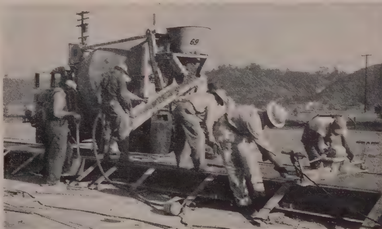
VIBRATING SCREED and internal vibrators used in pouring the channels to secure uniform density for the 5,000-psi. concrete. Maximum aggregate was \frac{3}{4} in. and slump 2 in. The top slab of the channel is only 1\frac{1}{2} in. thick. High early strength cement was used.
