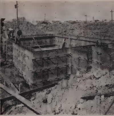
RESIDENCE FOUNDATION —Erects fast . . . two liners only on inside; no liners on outside.
