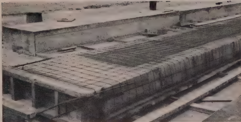
CHANNELS were poured around concrete blocks, seen in background, with two pretensioned strands in each rib (flange). Feature of the tensioning was the hold-down device that depressed the top strand 7 in. at mid-point, requiring a force of about 1,000 lb.
