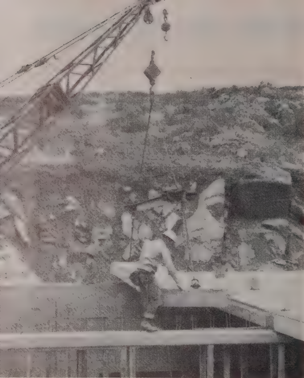
SETTING 33 x 4-ft. pretensioned channels with a 12-in. space for the poured-in-place closure. This closure, properly dowelled and keyed, provided a composite beam action of 19 in. for both the dead and live loads.
