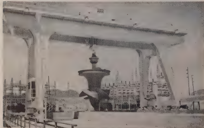
PLACING RUNNER assembly of turbine in pit took place last July. Size of crane can be estimated by noting men at lower right. Completion date for project: Dec. 23, 1956.
