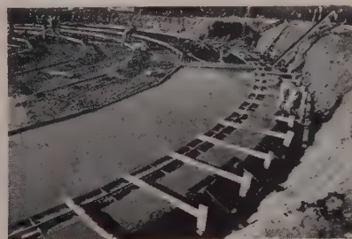
CONTINUOUS POUR of 125' dia. foundations and floors (540 cu. yds. per tank) avoided joints.
