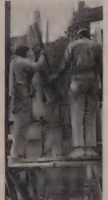
ALL PLY PANELS come in 3 standard sizes: 2 x 4, 2 x 6 and 2 x 8 ft.
