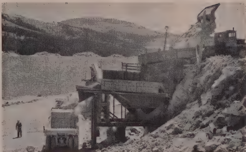
MATERIAL was dumped directly onto the Wobbler (note size of rock being ejected at left). Revolving bars in Wobbler are made of manganese steel to withstand heavy beating.
