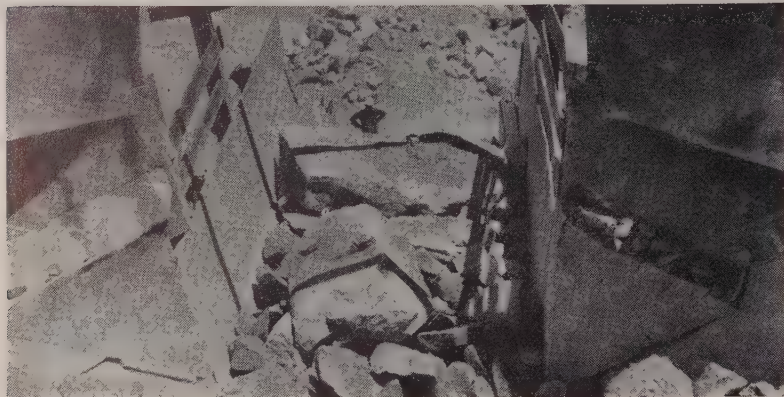
Scalper-feeder saves the day for Fisher Contracting Co. when rock source turns bad at Montgomery Dam in Colorado.
