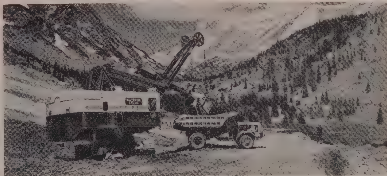
HIGH ELEVATION , 10,800 ft., caused machine efficiency to drop off (30% for gasoline engines). This is the highest dam in elevation in the nation, first with asphalt face.
