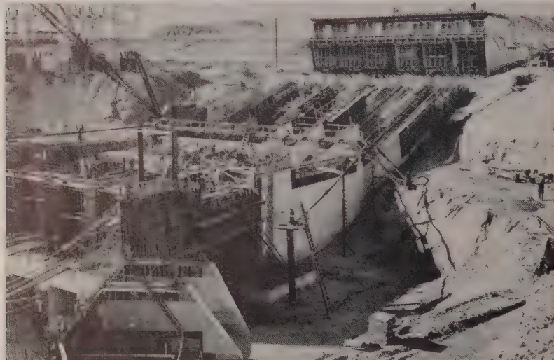
POWERHOUSE has advanced to the roof of the scrollcase. In the background are the six penstocks and the intake structure. Note deep well pump in center foreground.
