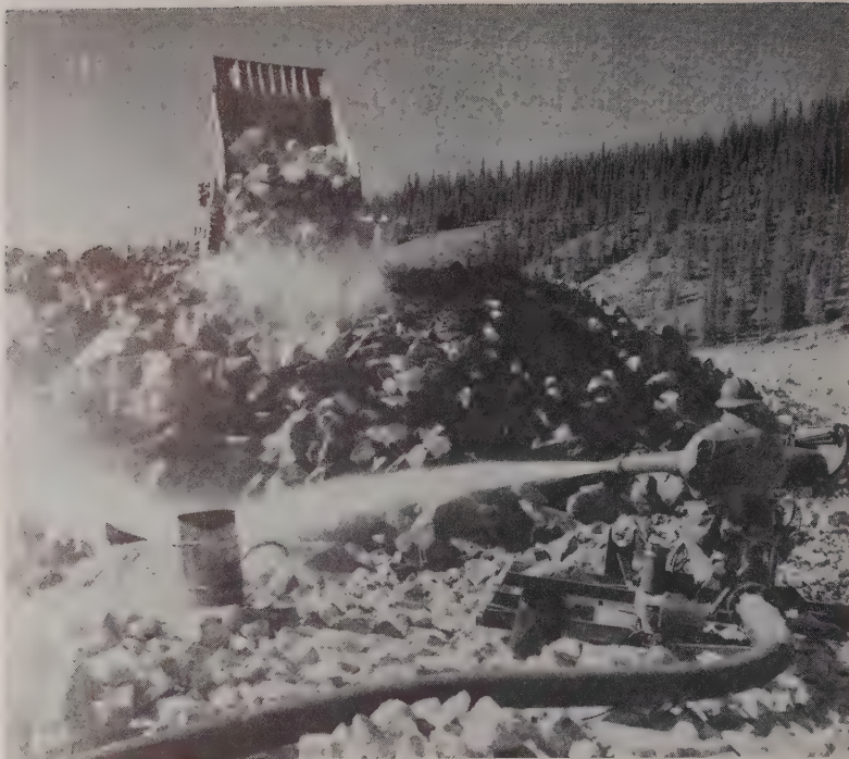
JETS wash rock as it is placed to prevent pockets of fines from forming supporting pads to permit excessive future settlement. Lifts were up to 30 ft. in height in main zone of dam.
