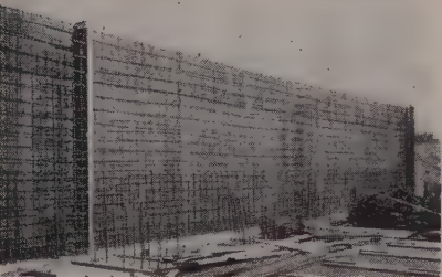
FLUSH DESIGN —Simplifies stacking the forms at job site. All Ply's weigh less than 5 psf.
