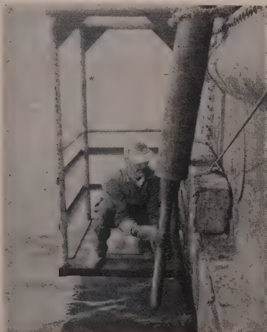
BLASTING (left) for the rock trench was done with unusual bomb which exploded upon impact. Average charge was 5 lb. of 60% powder. DERRICK WINCH (right) is modified Skagit model 140. Front drum is divided to operate topping lifts. Back drums operate two load lines separately.
