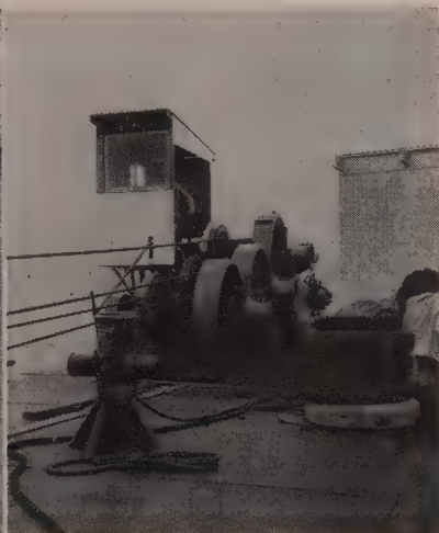
BLASTING (left) for the rock trench was done with unusual bomb which exploded upon impact. Average charge was 5 lb. of 60% powder. DERRICK WINCH (right) is modified Skagit model 140. Front drum is divided to operate topping lifts. Back drums operate two load lines separately.
