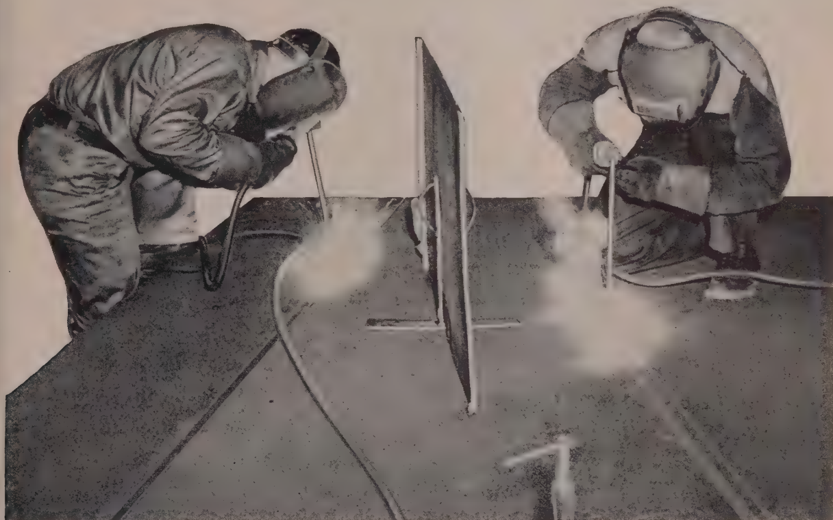
Fabricating ½-inch wrought iron pier plates with "Easyarc 12" electrodes. Powdered metal electrode coating actually becomes part of the weld deposit.
