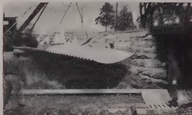
Truck hoist is used to place individual plates into position.
