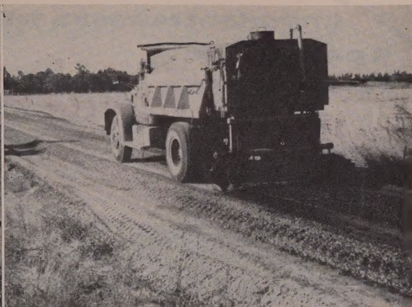
Fig. 4—Emulsified asphalt is applied from water tank mounted in truck. Rate is 0.7 gal. per sq. yd. for the 2-in. depth of material. Emulsion is undiluted.
