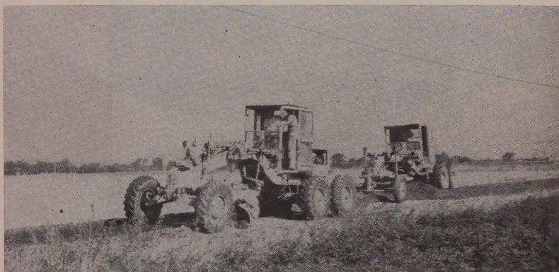
Fig. 5—Mixing is the usual process, and is shown being carried out by motor graders working in tandem. If mixing becomes difficult more water is added, if the mix is wet it is allowed to dry out.
