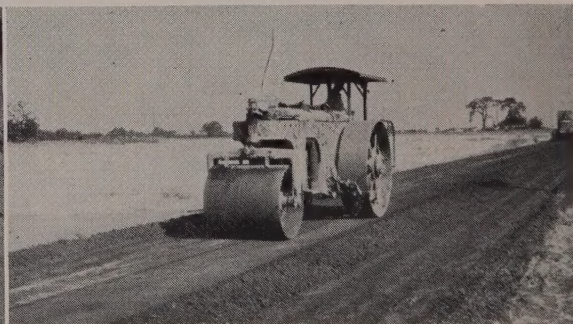
Fig. 2—After breaking up the existing mat with a Hyster Grid roller, it was rolled to secure compaction. All equipment is the type normally owned by counties and county engineers work with what they have.
