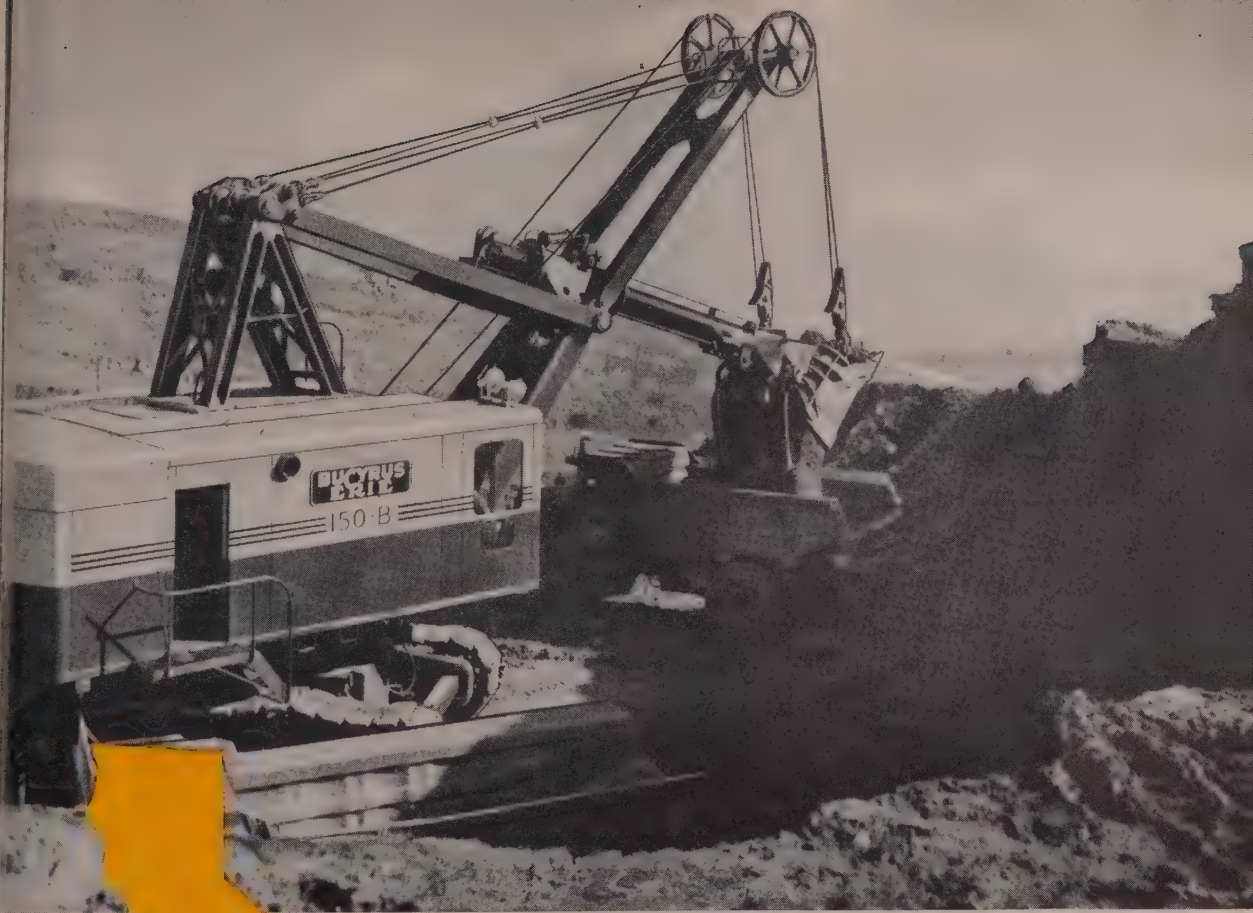
Near Candlestick Point, outside of San Francisco, a 6-yd. 150-B loads borrow to help build a new freeway.
