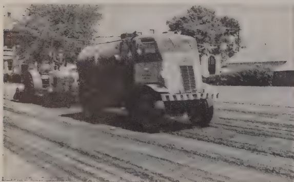
Distributor and "Pulvimixer" apply and mix Bitumuls to stabilize old pavement that has been scarified and bladed.
