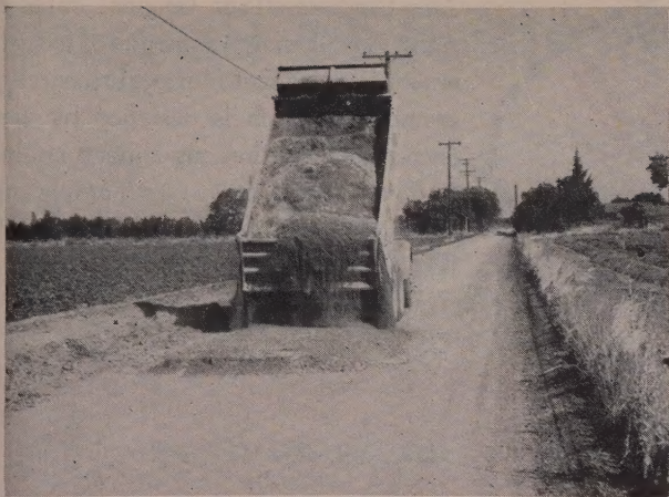
Fig. 3—Gravel of a type normally considered sub-standard, but available and cheap, is deposited. Again, note how the problem is complicated by irrigated fields.
