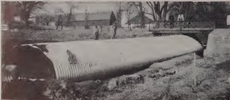
Finishing up assembly of Armco MULTI-PLATE Pipe-Arch structure to replace old bridge in background.
