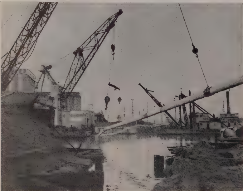
WATER CROSSINGS are always tough. This shot was taken when Engineers Pipeline Co., Ltd. crossed W. Waterway of the Duwamish River on a lateral for Seattle Gas Co.
