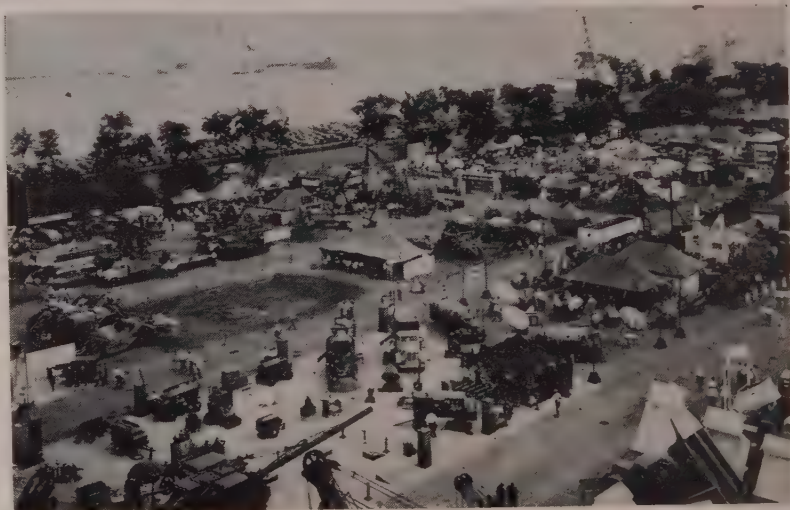
1948—"The World's Fair of the Construction Industry" as it was called was held in the summer outdoors. The 1957 show will again be indoors in Chicago's International Amphitheatre.
