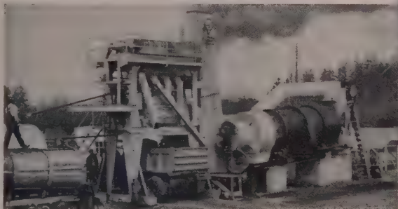
MADSEN 2000-lb. SPECIAL Asphalt Plant... ideal for the not-too-large contractor, the municipality, and the large contractor who wants a small type of operation for producing approximately 480 tons per 8-hour day. (Ask for Catalog No. 20-S.)
