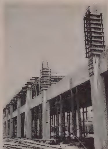
COLUMN FORMS consist of 2x12s faced with 1/4-in. plywood backed with a welded steel frame.
