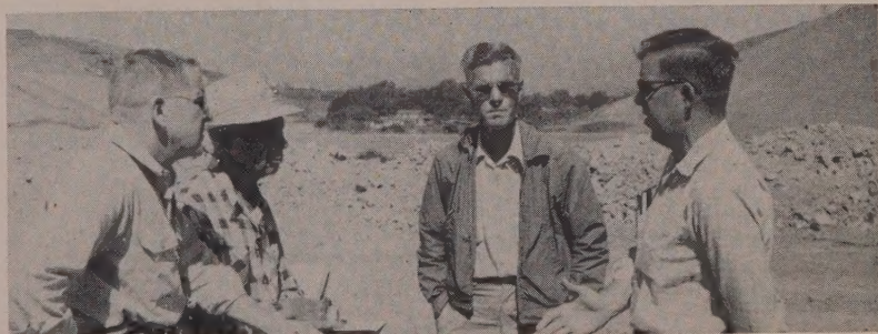
MEN IN CHARGE —Left to right are: Charles Sweet, resident engineer; R. Philbert, superintendent for contractor Ferry and Crow; H. Tunks, assistant resident engineer; G. Kelly, chief of surveys. See end of article for other personnel.
