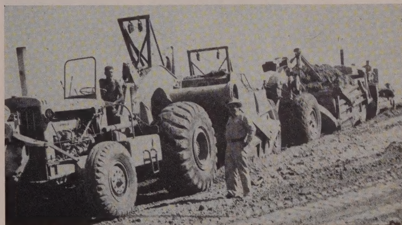
LOADING is watched by grade foreman Obie Hall. Note front power take-off and cables passing through pulleys on A-frames to rear scraper. Operator has two extra levers for front PTO. Similar view is enlarged on the front cover.
