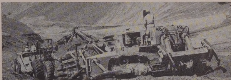
LOADING requires skilled operators. Notice how the D9 operator stands so that he can see arm signal of scraper operator when front scraper is full. Tendency to jack-knife is diminished by loading back scraper first and loading in slight trench.
