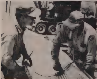
ASSEMBLING the 2-ft. width of sections with bolts to form the self-supporting arches for the 120-ft. span.
