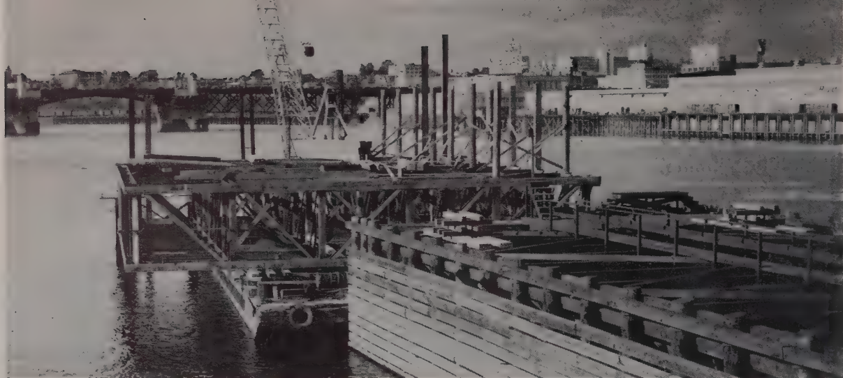
GUIDE PILES are being driven through the cofferdam crib as it rests in position on floating barge. When the crib
