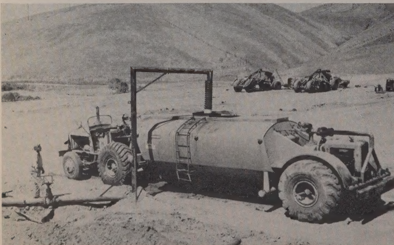
SPRINKLING is done with this water wagon consisting of a 5,000-gal. Southwest tank pulled by a Euclid tractor. Driver is shown filling it with salt water obtained from nearby oil refinery. Salt helps to diminish the dust nuisance on the fill.
