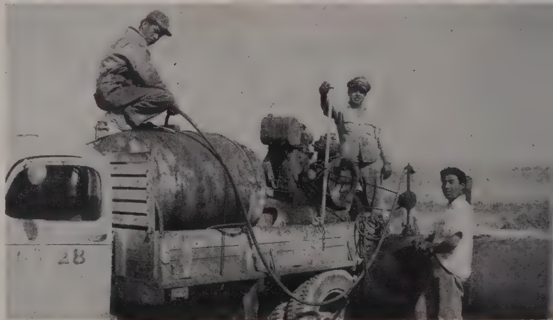
INGENUITY is better than hand pumping. This crew is using one of the drive belts off the compressor to operate the fuel pump out of the stationary tank.
