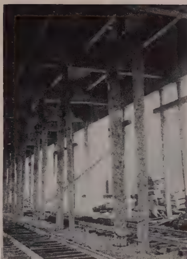
FALSEWORK is supported on temporary timber piles driven to 35-ton capacity and later cut off below ground.
