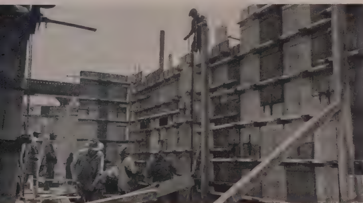
Million ELEMENTARY SCHOOL —Plywood face and rigid locking of forms by Combina- on Clamp insure clean, true surfaces.
