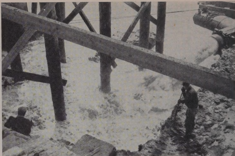
BRIDGE FALSEWORK in the excavation area presented a problem for the dredge. Much of the material was successfully sluiced away during periods of low tide.
