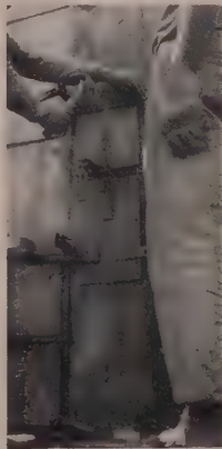
ONE BLOW of hammer locks panel, secures snap tie, holds liner.
