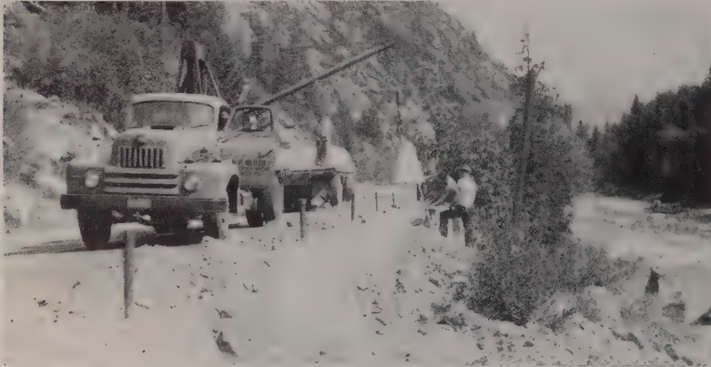
INTERNATIONAL truck on county-road work handling concrete guardrail posts.
