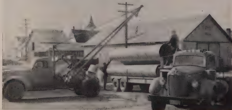
CHEVROLET truck converted to crane unloads culvert pipe from Mack truck.
