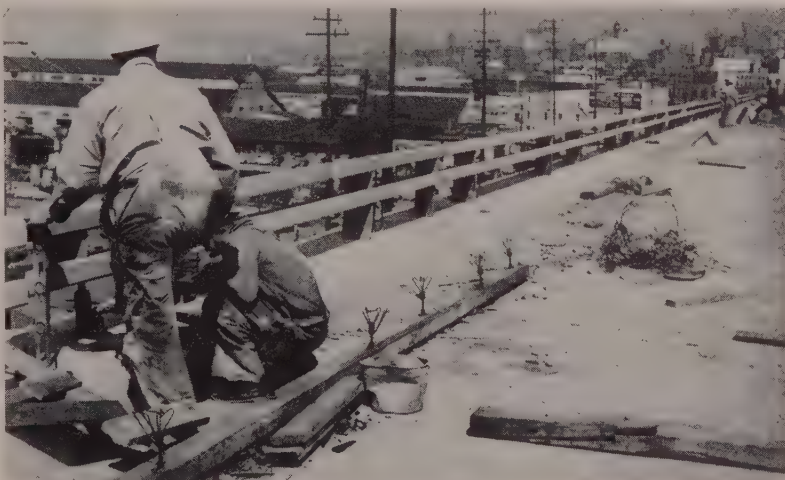
WORKMEN SET guardrails which permit good visibility. Note upturned wooden screed behind men with screed chairs in position.
