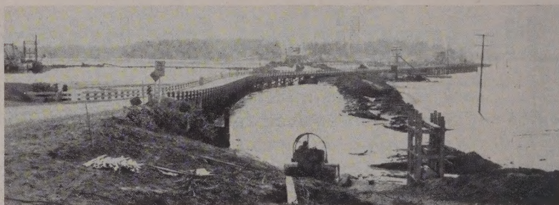
PORTIONS OF EXISTING BRIDGE were removed and traffic was routed over new fill to the old bridge as soon as new fill was up to grade. Cat D8 is building dike.
