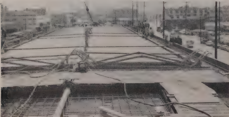
TOP DECK VIEW —Lateral pouring platform mounted on wheels is visible in foreground. Wheels resting on center longitudinal screed can be seen in left center. Concrete pouring progresses without the usual interruptions for repositioning.
