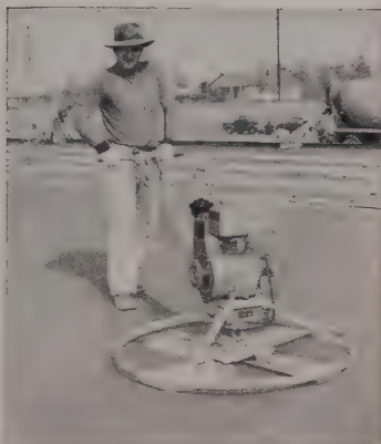
Superior Power Trowel, powered by Wisconsin Engine because "it was the only engine combining light weight plus hp. — a big factor in power trowel design."
