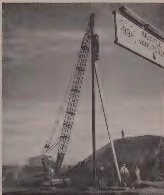
Driving piling for a new interstate bridge near Portland, Ore., is this Bucyrus-Erie 22-B Transit Crane. Consolidated Freightways of Portland owns the machine.
