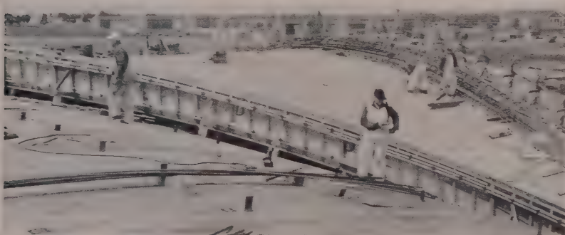
BOLTS THROUGH CONCRETE BLOCKS placed between rib forms and deck form tie forms together. Shell and ribs were poured at same time. C&E Staff Photos.
