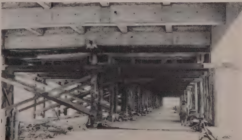
FALSEWORK for upper deck is similar to that for lower deck. Here, too, a passageway is kept clear, in this case for transit trucks bringing concrete to the end of the lower deck. Lateral horizontal beams are 12BP53.
