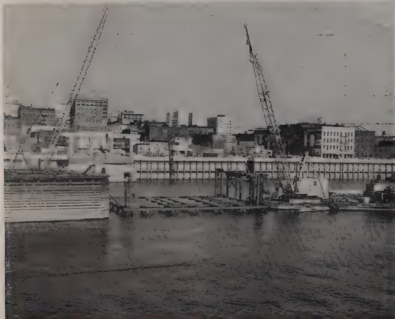
THE BARGE has been floated out of the way and the crib is being lowered by the tackles. When crib is in place near bottom sheet piling is driven around it. Tackles are transferred to the sheet piling and the guide piles are removed.
