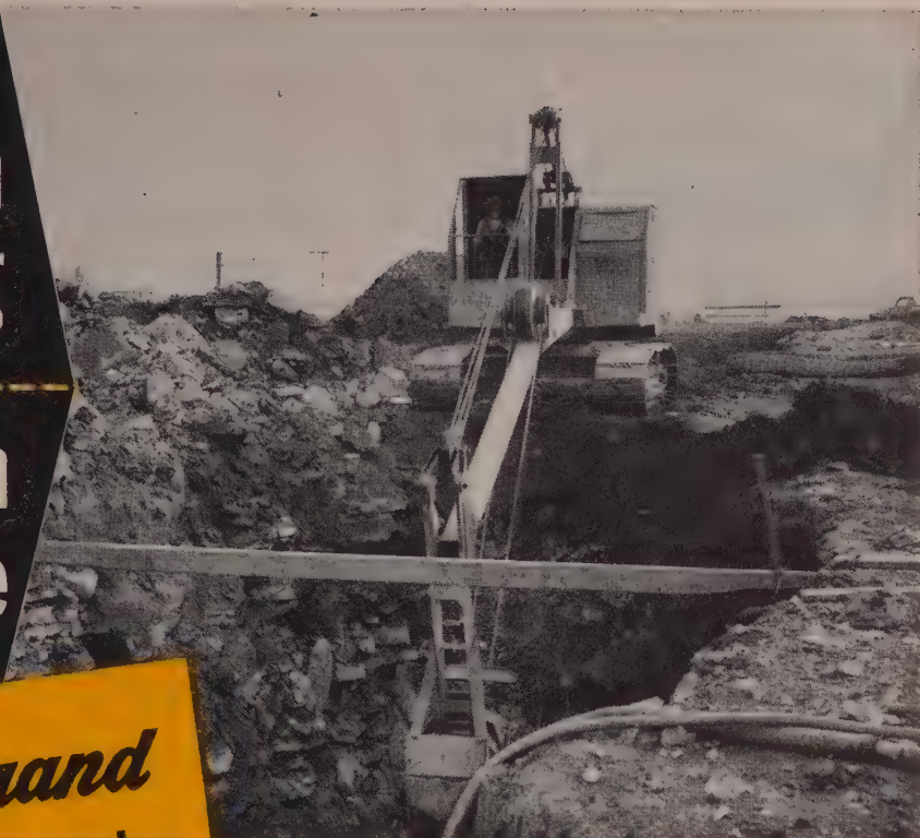
Yellow Strand Flattened Strand is used by Donlon Construction Co., Nashville, Tenn., in this \frac{3}{4} yard backhoe on tough rock cut for sewer line.
