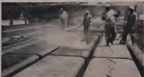
Richfield Form Oil #36 is applied to deck slab form prior to casting. Approximate area of contact is 5370 sq. ft.
