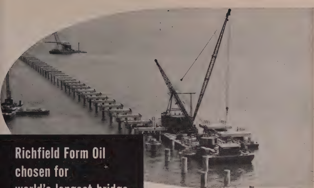
Early phase in construction of 24-mile-long Lake Pontchartrain Bridge, New Orleans.
