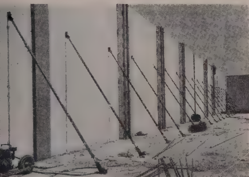
ADJUSTABLE BRACES used for quick and easy alignment of panels
