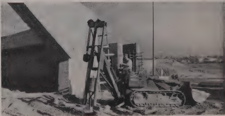
TAMPER ATTACHED TO DROTT SHOVEL USED AROUND STRUCTURES
