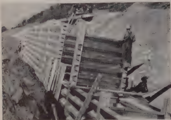
Construction crew assembles 530-foot-long Armco Bin Wall in repairing slide damage on an Illinois highway.
