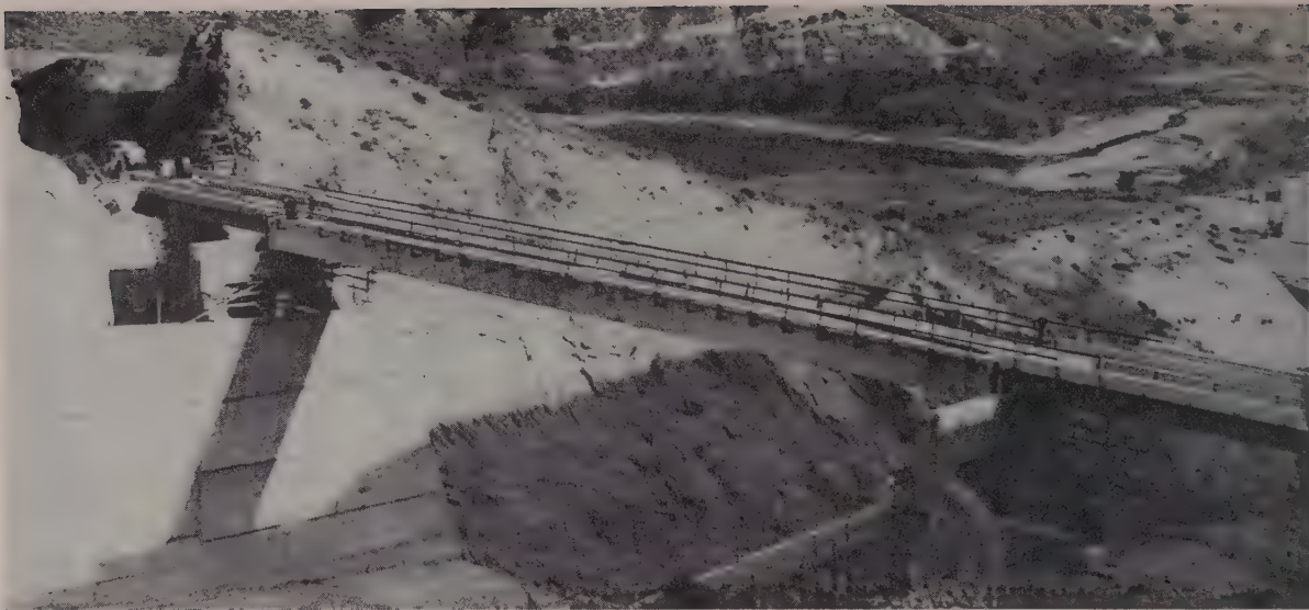
CROSSING the spillway of the Santa Felicia Dam, this single-lane bridge of 31, 51 and 122-ft. spans cost only $11.24 per sq. ft. for the
