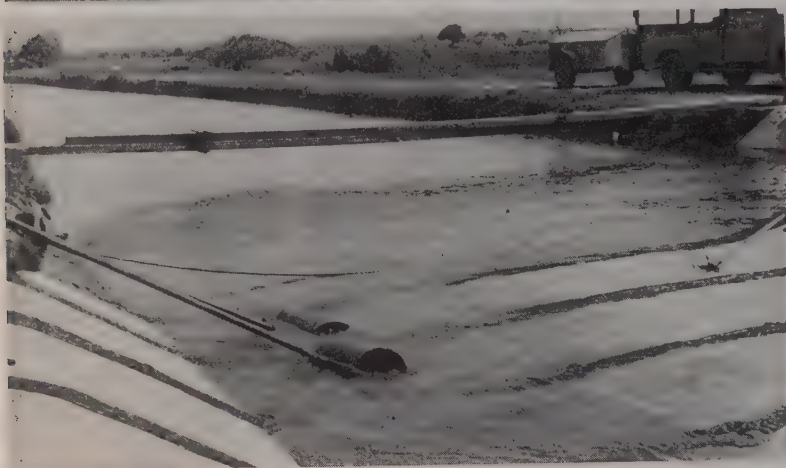
PLACING (above) was done by pulling the barge across the canal, allowing the asphalt panel to sink and conform to the slope and bottom of the canal. At first some difficulty was experienced with the panels tending to float or porpoise with the current. Note the mastic applied to the ends of the panel. This was intended to bond to the end of the opposite panel, when it was placed by the reverse procedure from the opposite bank.
