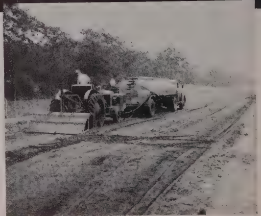
Preparing 8" Bitumuls stabilized base
