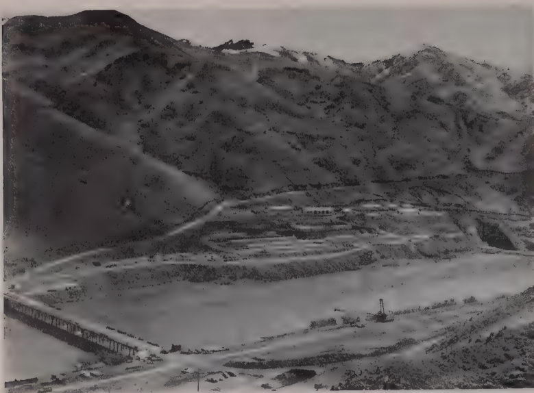
CONSTRUCTION CAMP is on Idaho side of the river built on broad steps made of spoil from the tunnel. There are 20 major buildings, with air-cooling for the bunkhouses, mess hall, and offices. Access bridge at lower left was also built by M-K.
