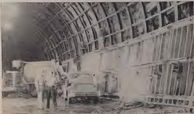
DRIVING CONDITIONS were good but about 400 ft. of the 38-ft. diameter horseshoe had to be lined with concrete. Steel ribs were positioned from the drilling jumbo, panels moved ahead with a truck crane. Concrete at top of arch was placed by Pumpcrete.
