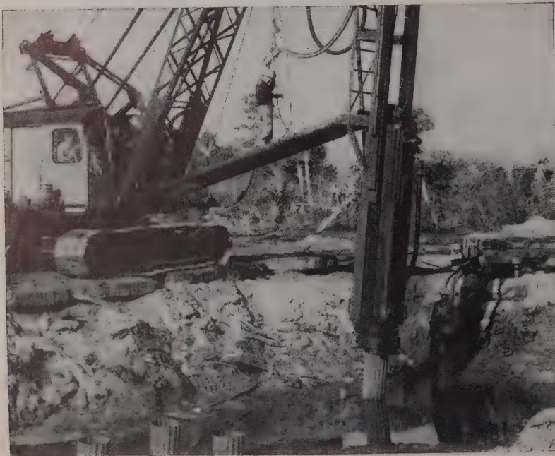
Driving batter pile of trestle for the St. Lucie Canal Bridge in Florida. Schedules called for driving 42,000 lin. ft. of these 33-ft. light wall steel pipe piles in 90 days through a tight saturated formation of seashells, sand and marl underlying the top 6 to 8 ft. of matted vegetable matter and sand. Skillful work by the contractor, Paul Smith Construction Company, and the powerful blows of a McKiernan-Terry S5 Single-Acting Pile Hammer powered by a McKiernan-Clayton Steam Generator completed this difficult task successfully within the time limit, with piles being driven at the rate of 30 ft. in less than 10 min. driving time. McKiernan-Terry Corporation, 24A Mercer Street, Dover, New Jersey.
