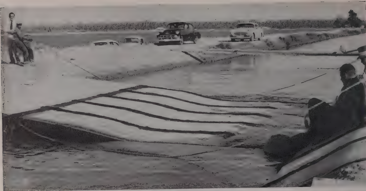
PLACING (above) was done by pulling the barge across the canal, allowing the asphalt panel to sink and conform to the slope and bottom of the canal. At first some difficulty was experienced with the panels tending to float or porpoise with the current. Note the mastic applied to the ends of the panel. This was intended to bond to the end of the opposite panel, when it was placed by the reverse procedure from the opposite bank.
