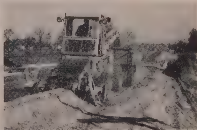
Making clean 8' wide pick-up, Traveloader loads surplus material windrowed on road shoulder, without interference to passing traffic.
