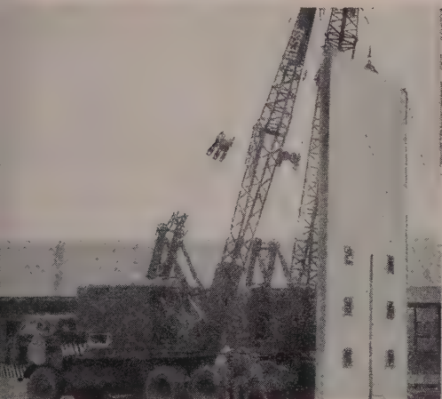
57 TON SLAB being positioned
