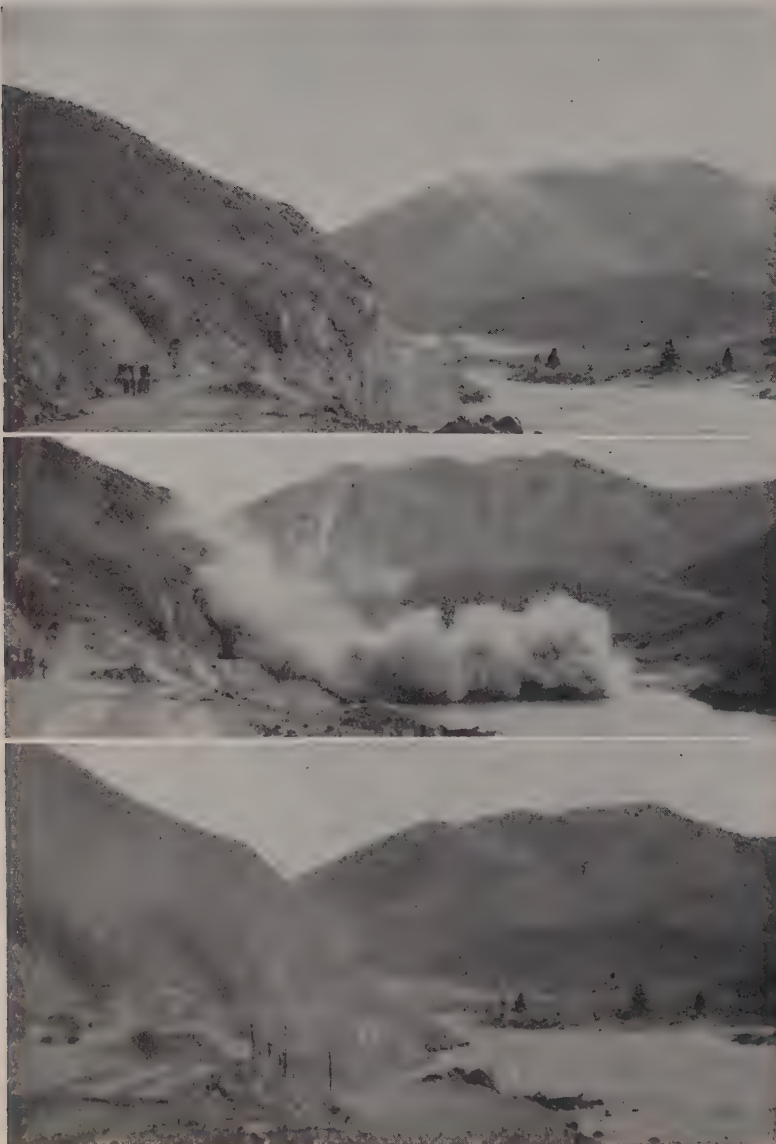
SEQUENCE PHOTOS show blasting 10,000 cu. yd. during improvement of U.S. 95 in central Idaho. Biggest blast so far took out 20,000 cu. yd. Total excavation will be about 510,000 cu. yd., of which 240,000 cu. yd. is rock. Job required round-the-clock traffic control.
