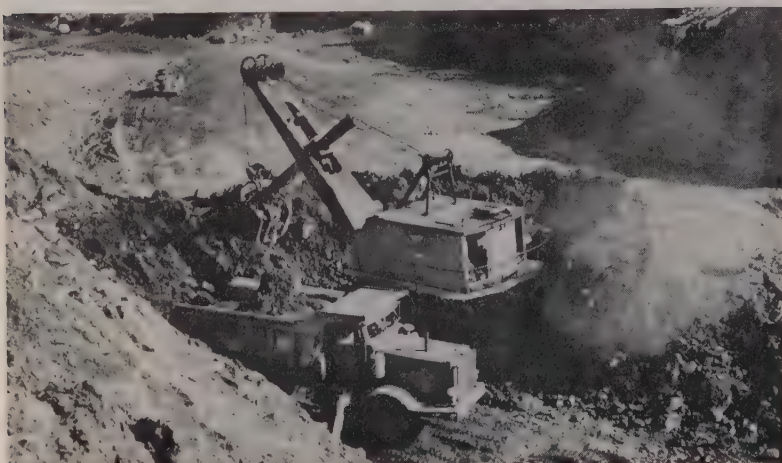
A BUCYRUS-ERIE 71-B, 3-cu. yd. shovel loads one of a fleet of Euclids. The shovel is powered by a Detroit Diesel 6-110 engine with torque converter and tail shaft governor.
