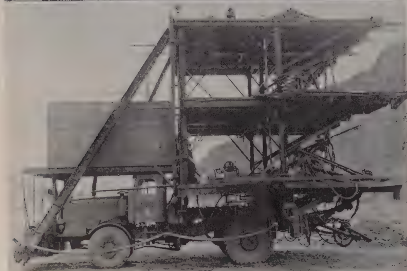
TUNNEL DRILLING JUMBO was designed by Woody Williams, head of M-K's Dam Division. It carries 14 Joy drifters and is built around a 17-yd. Euclid tractor and frame. This gave the rig good mobility, enabled it to move quickly from one heading to another. Tunnel meeting was remarkably smooth, with no visible rock rib. Top photo shows jumbo under construction.
