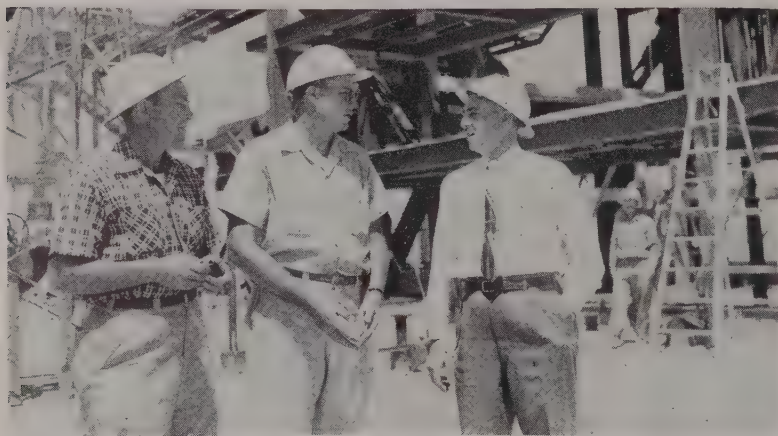
GOING UP on schedule, is the $26,000,000, 200,000-kw. Agua Fria steam power plant of the Salt River Power District, located between Glendale and Peoria, Ariz. The above trio of on-the-job leaders of construction are (l. to r.) Ken Wells , job engineer, Bechtel Corporation; John Dingle , resident engineer for the power district, and K. Haig , project engineer for Bechtel, the builder and designer.
