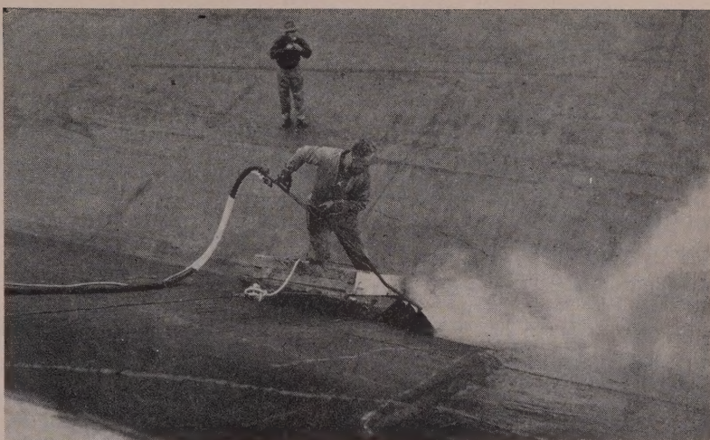
PLATFORM for the operator was mounted on casters and handled by a winch on the canal bank. The recirculating line (1/2-in. metallic covered) did not prove successful and was removed.
