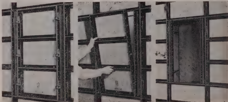
NEW TECHNIQUE FOR POURING POCKETS
