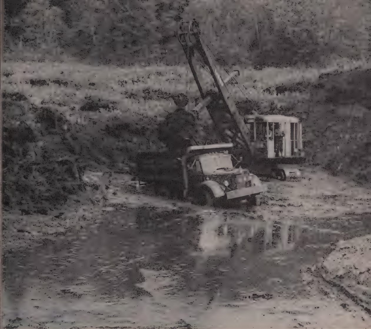
S & M Construction Company, Providence, R. I., uses 12 of these Mack LJSWX diesel dumpers under 2-yard Lorain shovel in excavating peat bog near Atholl, Mass., on a by-pass for U. S. Route 20.
