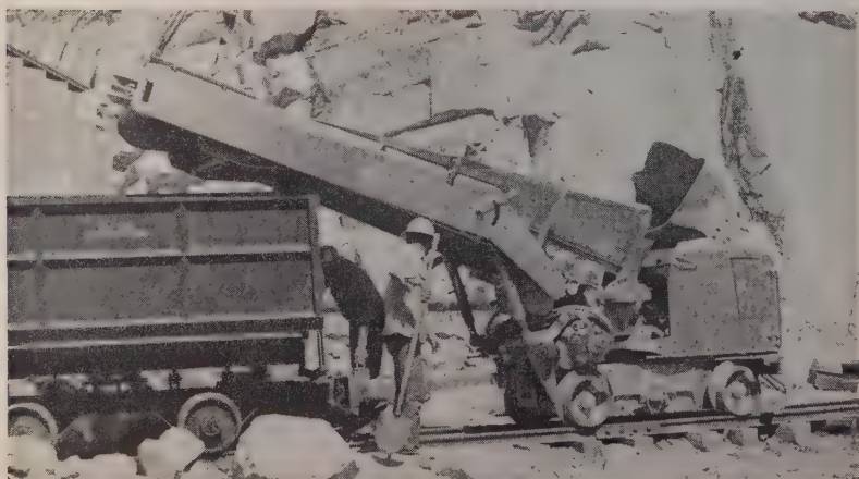
MUCKING is handled by an Eimco mucker loading into cars of 5-yd. capacity made by Century Steel. The usual train of seven cars is hauled by a Goodman 10-ton battery locomotive. A California switch near the face is carried forward about every 10 days to keep it close to the heading.
