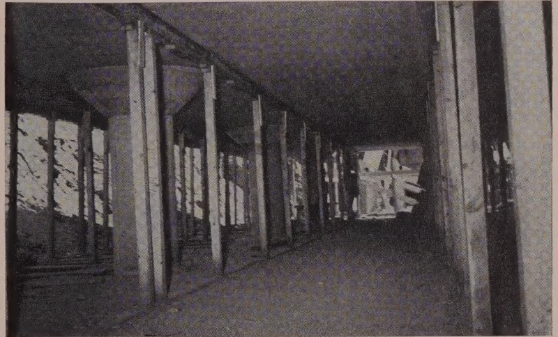
AFTER INITIAL STRIPPING , slab looks like this. Note that every other shore has been removed in the remaining rows. Panels have been dropped, cleaned, and moved to next erection point.
