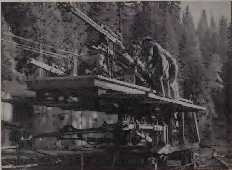
EACH HEADING has a job-built jumbo operating on the 36-in. track. Six Ingersoll-Rand drifter drills operate from the two levels of the jumbo, supported and operated by I-R Hydro booms.
