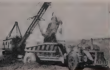
One of PCA's fleet of Wooldridge Terra Cobra wagons equipped with Fuller 4-speed 4-A-112 Transmissions.
