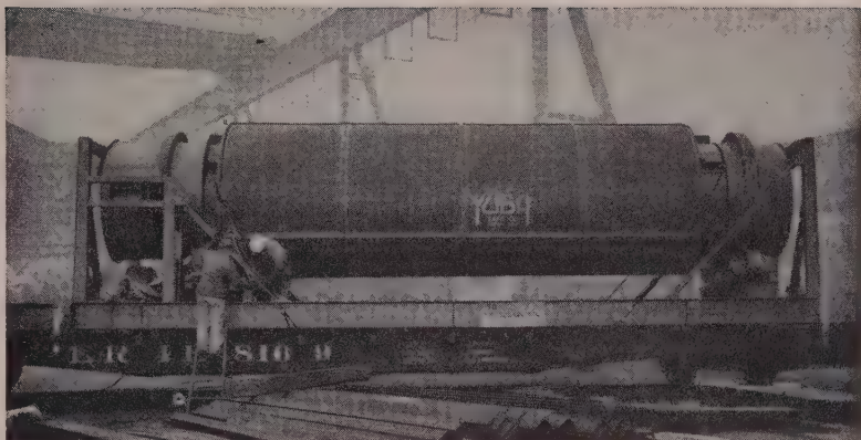
Yuba designed this screen for long life, minimum maintenance. Inner and outer screens easily renewed. Can be lubricated from outside.
