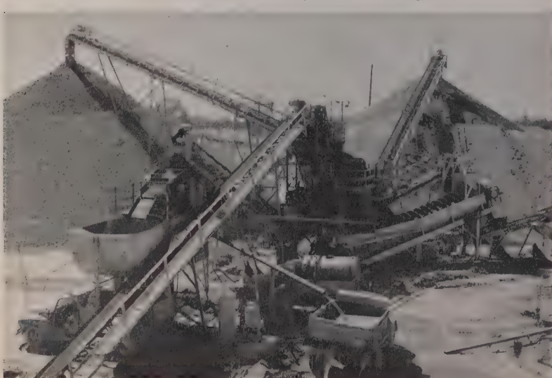
AGGREGATE for the job is being supplied by subcontractor Madison Sand & Gravel Co. at their permanent plant. Most of the 6-in. material is coming from deposits along the American River, north of Sacramento. Trucks haul aggregate to the site from as far away as 50 mi.
