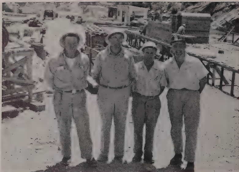
STANDING in the mill yard are (left to right): Joe Hassel, day shift superintendent, Ford Johnson, general superintendent, Shorty Schramm, cleanup and sandblasting foreman, and Doug Baker, project manager.
