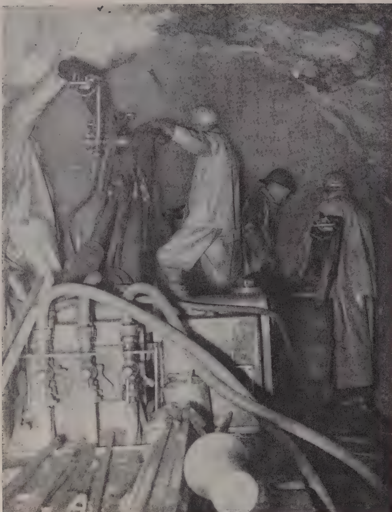
DRILLING CONDITIONS were similar at all headings. Work is progressing at two headings on the last remaining section 13,000 ft. long. The usual drilling pattern calls for 56 to 60 holes per round which are drilled to a depth of about 11 ft. Since the tunnel will not be lined, overbreak, which has been small, is not a serious problem.
