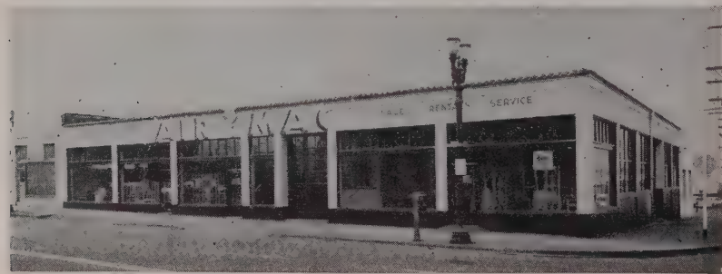
AIR MAC INC. of Oregon's new 10,000-sq. ft. building at 1111 S. E. Grand Ave., Portland. This distributor offers complete sales, service, and parts for both the Towmotor and the Gerlinger fork lift trucks and carriers. Air Mac is also exclusive distributor for many other materials handling lines. Jack W. Emahiser is manager.
