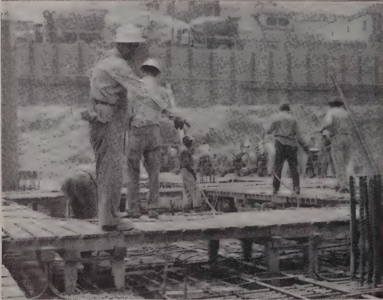
RUNWAY BRACKETS EASY TO ASSEMBLE, DISASSEMBLE
