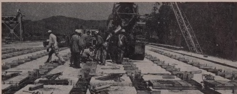
POURING THE SPACE between stringers and pouring the diaphragms were completed last month. Dowel steel of adjoining members interlocks for maximum bond between members.
