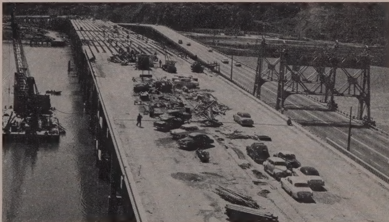
ABOVE —The six-lane structure is almost ready for traffic. Next step for contractor Duncanson-Harrelson Co.-Pacific Bridge Co. (joint venture) is removal of old timber bridge at right.
