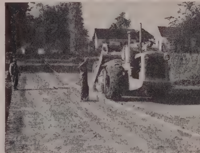
Fine-grade before paving
