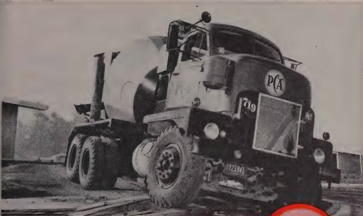
A PCA "Engine-Take-Off" mixer truck—one of 42 IH FC-402-L Trucks with T. L. Smith Integral Mixers and Fuller 5-C-650 Transmissions.
