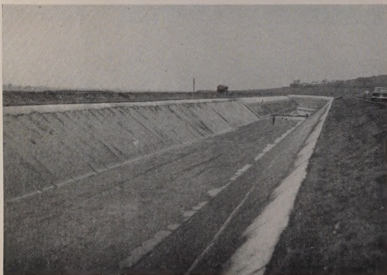
A COATING of asphalt-base aluminum paint covers completed membrane as protection against weathering and to reduce membrane temperature during summer months. 165 gal. of paint were applied and 19.73 tons of "cat-blown" asphalt to cover 3,710 sq. yd. of canal lining surface.
