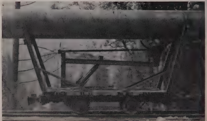
SPECIAL pipe-carrying car greatly speeded handling of large diameter ventilation pipes. Air is supplied by a Roots-Connorsville blower. Compressed air is supplied by two stationary 1,100 cfm. compressors, and is carried to the face in aluminum pipe. Water is also carried in aluminum pipe, and about 50,000 ft. will be used before the job is through.
