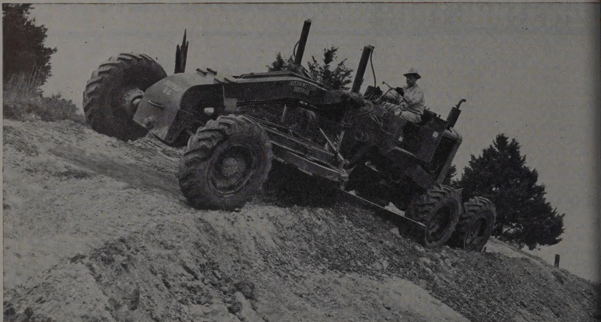
Power in the front drives makes it safe to work along the top of a steep bank.
