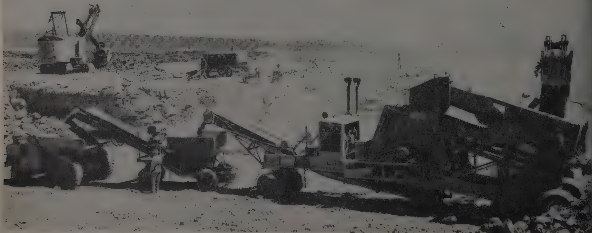
THIS CEDARAPIDS portable primary double impeller impact breaker is producing base-course material. Western jobs are rock jobs.
