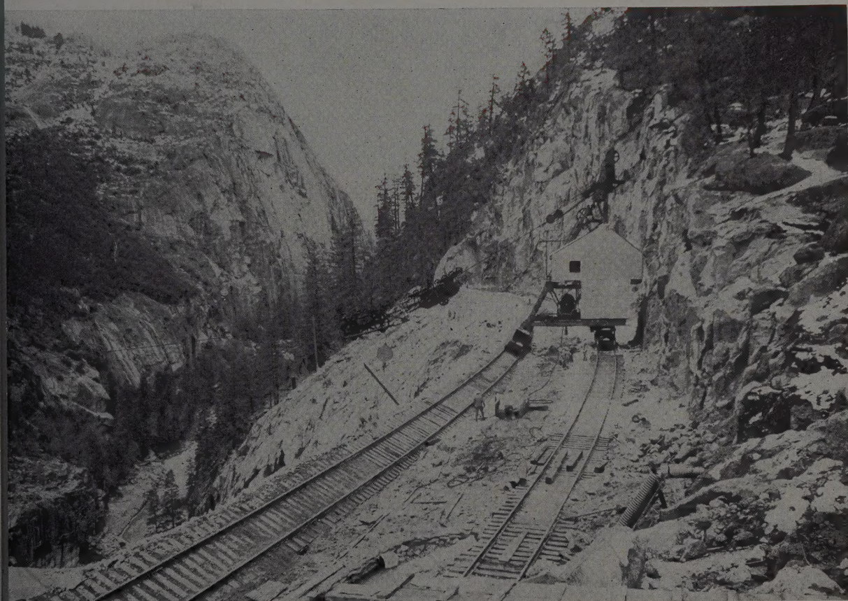
Space for construction plant was a serious problem, but gravity flow at the aggregate plant is a compensation. In the extreme lower left the stream is shown turning into the diversion tunnel.
