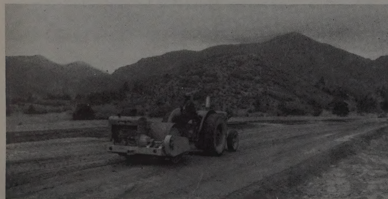
VIBRATORY COMPACTION is being used with excellent results by many of the contractors. Shown is a Vibro-Plus roller pulled by an Allis-Chalmers farm tractor.
