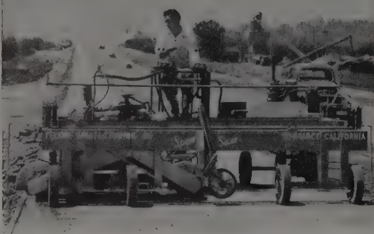
This V-type 4-cylinder model is one of two Wisconsin Engines that operate the Concrete Span-Saw.
