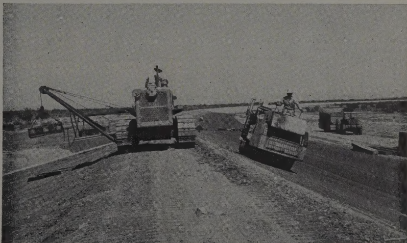
ROLLING on the upper section of the track required rollers with curved drums. The counterweight on the crawler could be varied to keep connecting cable force constant.
