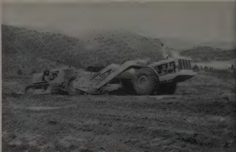
CRAWLER-SCRAPER combination heaps up a load in the excavation for the cadet quarters building. Deepest cut is 47 ft., highest fill, in the parade grounds, is 80 ft.
