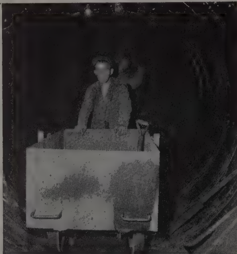
Two-man crew works face of Edmonton tunnel. One operates clay spade; other removes excavated material. Both install Armco Liner Plates.
