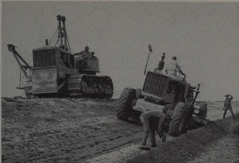
GRADING was handled by Caterpillar No. 12 motor patrols with special blades curved to fit the curved slope. The embankment was built one foot over, then cut back to finished grade.
