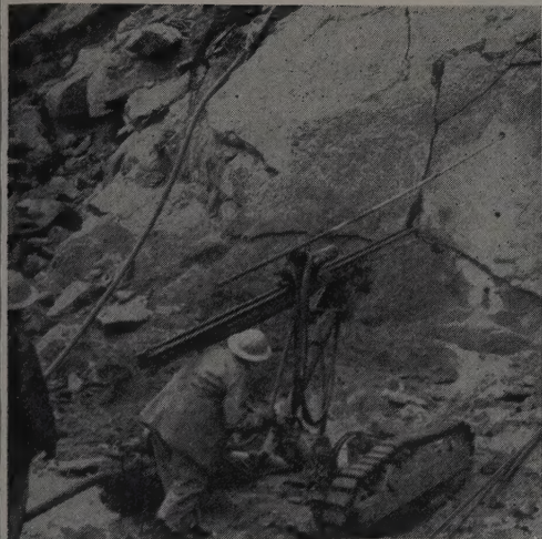
DOWN IN THE BOTTOM of the hole this I-R rig is drilling for excavating to solid rock in the side of the canyon. Aluminum pipe delivers compressed air over the job.
