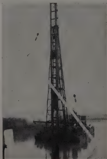
HANDLING a prestressed concrete pile 95 ft. long is easy because you can use a two-point hitch. All piles had hollow cores.
