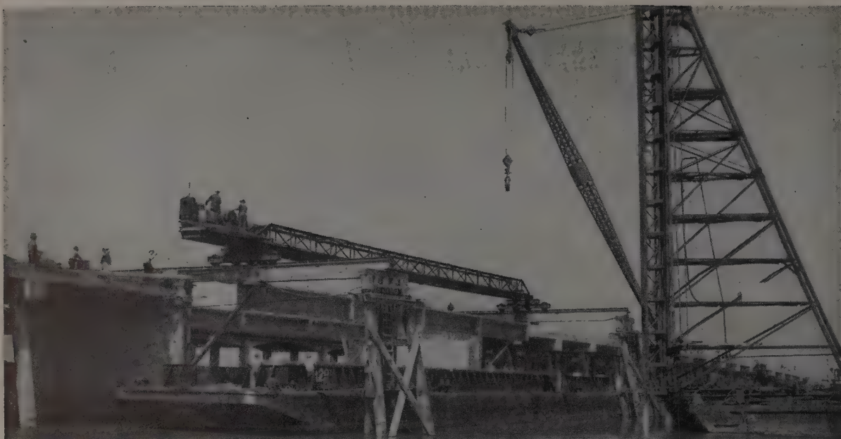
ERECTING the seven 66-ton prestressed concrete girders was done with a temporary gantry crane. The traveling trolley moved on rails
