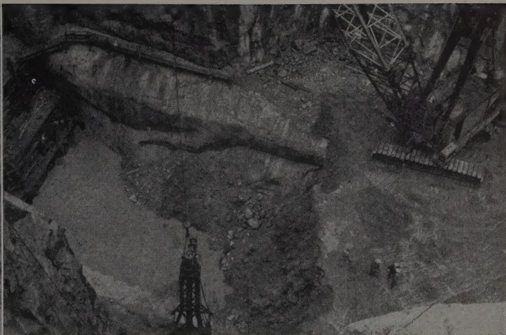
LOOKING DOWN in the foundation area, showing face of upstream cofferdam (see front cover) and the Manitowoc crane used to load out material. From 100 to 150 gpm. of water is handled by pumps mounted on tripods and handled by crane.
