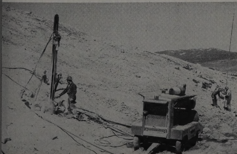
ON GOOD JOBS the loading follows closely behind the drilling, as shown, and the shots are fired promptly. The West is "bag powder country" because it is mostly arid.
