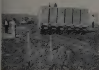
Southwest Model C-15 with D-4 "Cat" on Highway Job.
