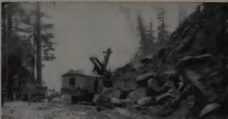
CONTRACTOR Arthur B. Siri loads rock with a Northwest shovel from a slide on Highway 101 south of Garberville during the second flood, which struck in mid-January. Over 31,000 pieces of privately owned equipment were put to work on restoration of the highway system.
