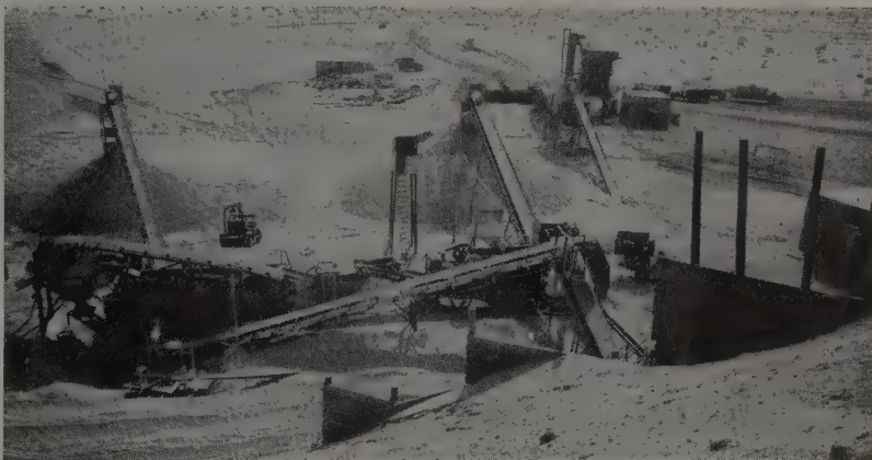
CRUSHERS in the foreground and screening plants turn out two sizes of aggregate delivered into stockpiles. A 200-ft. reclaiming tunnel had feeders operated by remote control.
