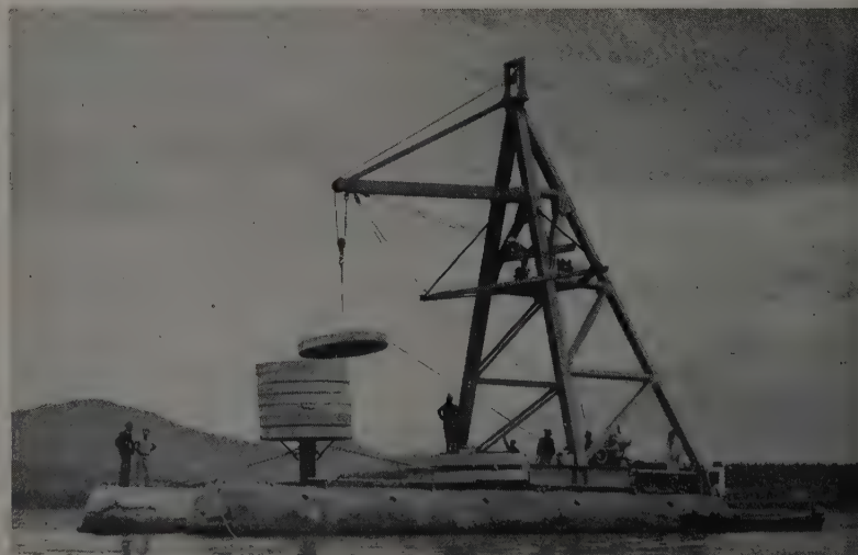
EARLY CONSTRUCTION featured the loading of eight test piles by the floating derrick. Loads ranging from 45 to 55 tons were placed on a pile, guyed in three directions. The derrick was mounted on two 8-ft. diameter by 60-ft. long boat salvage tanks.
