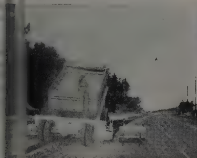
Seaman-Andwall Hercules Spreader applies cement, carefully metered to precise 2½ percent by weight to leveled and graded sub-base material.
