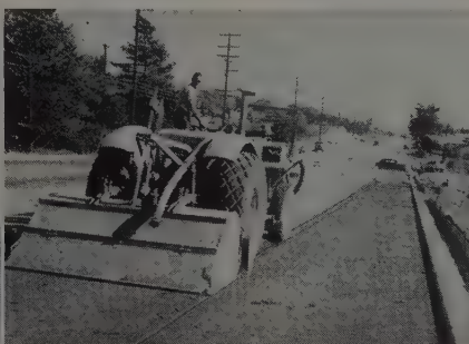
Initial dry-mixing with a TRAV-L-PLANT provides uniform and intimate blend of cement and materials to full 6-inch mixing depth.
