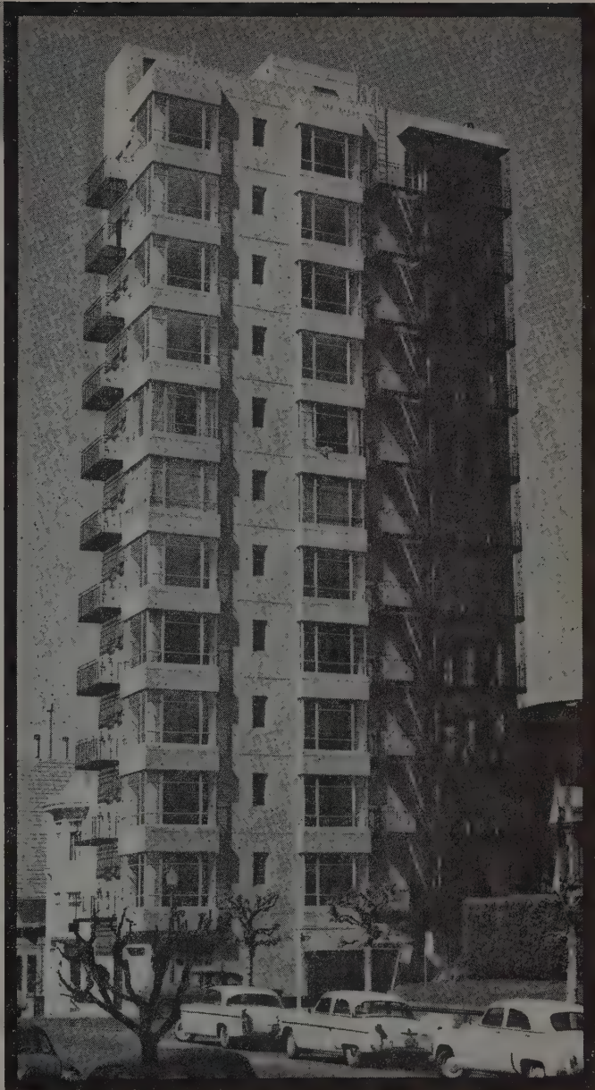
COMMUNITY APARTMENTS, Nob Hill, 1190 Sacramento Street, San Francisco. Note expansive glass areas and cantilever principle for window treatment.
