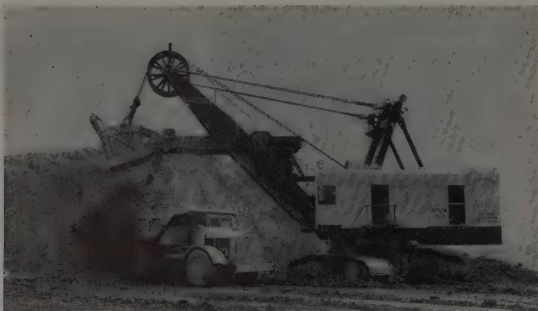
A BIG SHOVEL in the pit—10-yd. Marion—means low cost loading per truck load.
