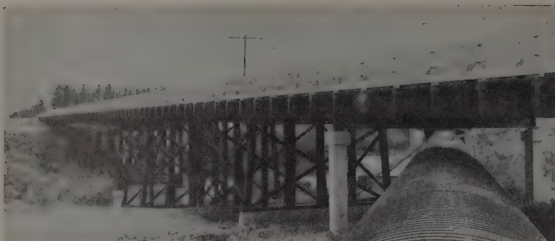
IN IDAHO this 536-ft. timber bridge over the Bear River (main span 161-ft. steel truss) contains 203,700 bd. ft. of pressure creosoted fir.
