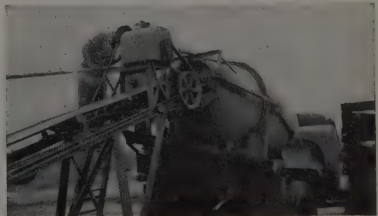
ABOVE: Spreader-box application of Bitumuls Slurry is fast and easy. BELOW: Aggregate and Bitumuls are fed into transit mix truck, then water is added as required.
