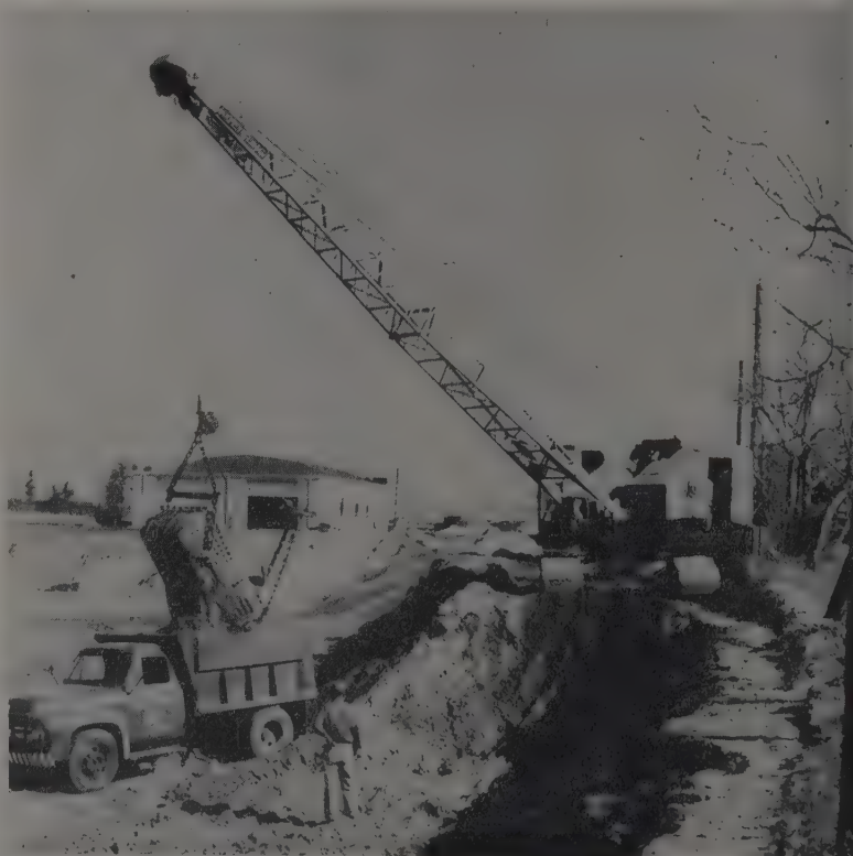
LOADING by crawler-mounted dragline of Koehring Co. calls for operating skill and timing.
