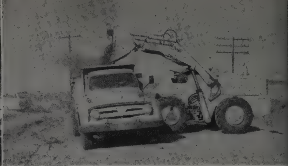
WIND AND PLOWING fill roadside ditches in the wheat growing areas. Farmers are allowed to plow up to the ditch line as a weed control measure, but it means cleaning out the drainage ways.
