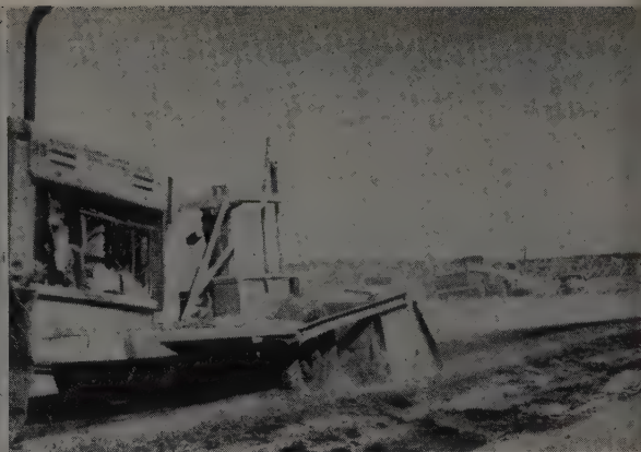
MIXER handles one-third of the asphalt placed in the first pass.
