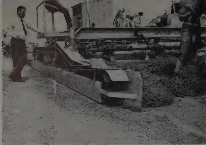
CONCRETE with 1½ to 2-in. slump is deposited ahead of the paver and emerges at the end of the slip-forms as concrete paving without sloughing along the edges of the slab.
