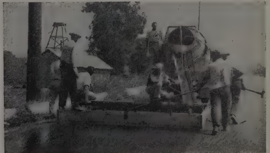
ABOVE: Spreader-box application of Bitumuls Slurry is fast and easy. BELOW: Aggregate and Bitumuls are fed into transit mix truck, then water is added as required.
