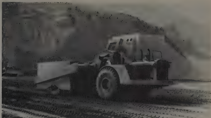
Southwest Model C-75 with DW-21 "Cat" on Dam Project in the West.
