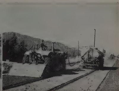
TRAV-L-PLANT working with tank truck, pumps, meters and sprays water as it mixes, for completed cement-treated sub-base, ready for final compaction.
