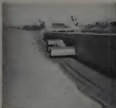
Southwest Model C-25 with D-6 "Cat" in Structural Backfill on Southern California Freeway Construction.
