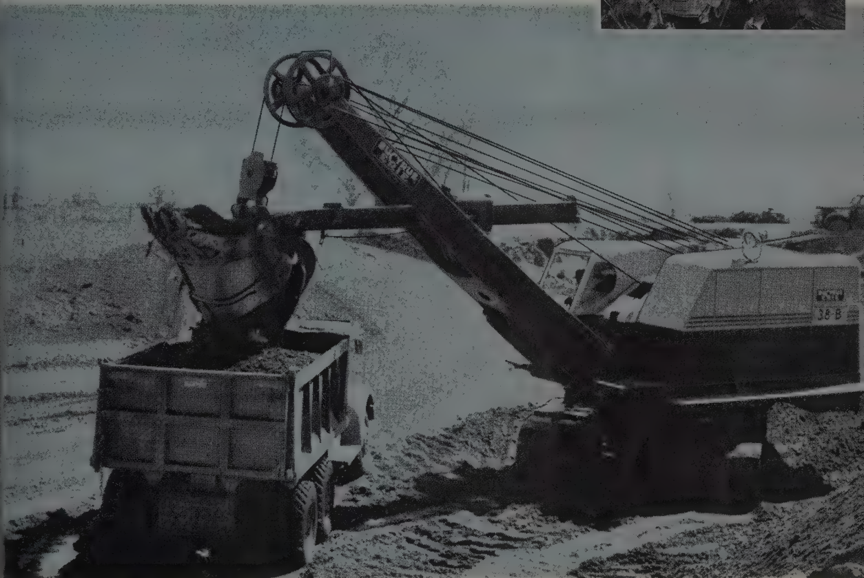
There are many years of heavy service ahead for this 38-B 1 1/2-yd. shovel. Owned by the Pioneer Construction Co., Pueblo, Colorado, it is loading granular base material for the State Highway Department on a construction job near Monte Vista, Colorado.
