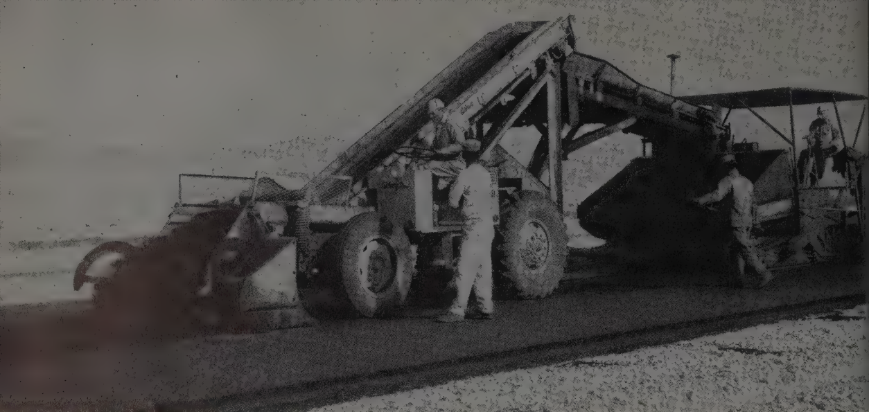
UNUSUAL METHOD of feeding the Barber-Greene paver was developed by the contractor. The mix was deposited in a windrow by bottom-dump trucks and then picked up by Athey loader. This operation moved 14.4 mi. across the desert near Palm Springs, Calif., on a $2,341,000 contract.
