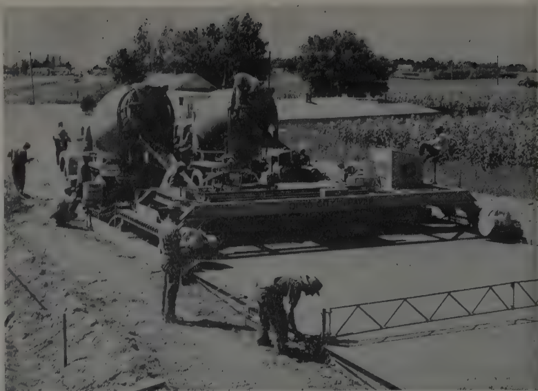
TRANSIT MIXERS were used to feed the slip-form because the 2,800-ft. length of the test section did not justify a paving mixer. This procedure did not prove completely successful since it required too much starting and stopping of the paver.
