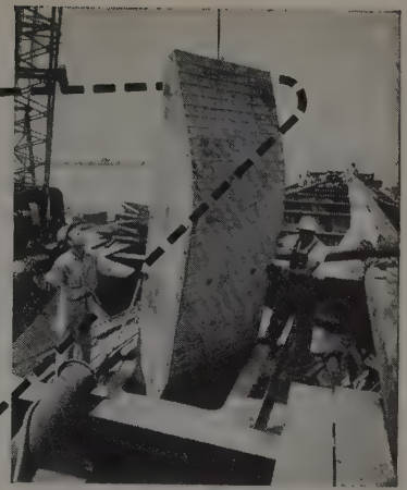
Above—Blaw-Knox sidewall form passes through 6 x 4-ft. hatch diagonally, to clear sides.
