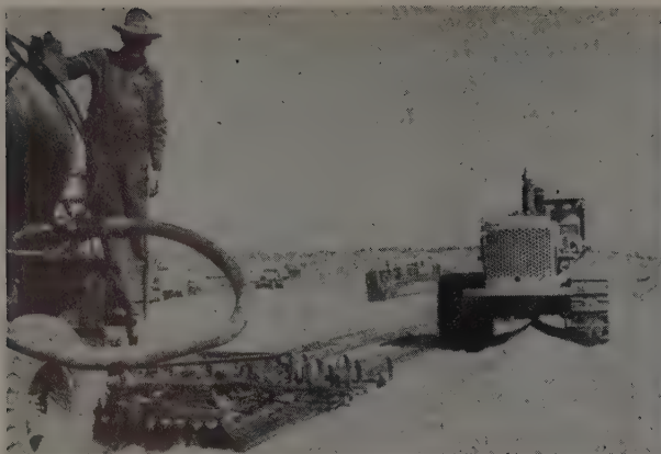
ASPHALT DISTRIBUTOR must be hauled through sand by tractor.
