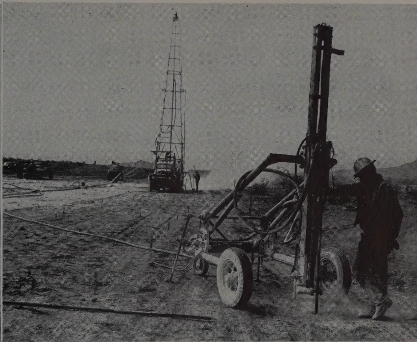
FLAT drilling conditions such as this are uncommon in the West. Superintendent on this job found an economical solution by doing slope holes with a wagon drill, deeper ones with a Joy rotary.
