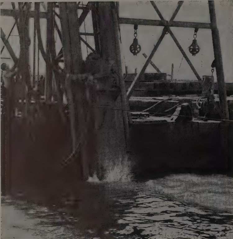
A McKiernan-Terry S10 Single-Acting Pile Hammer starts underwater to drive 195-foot 14-inch H-beam 70 feet below water for Richmond-San Rafael bridge foundation on the West Coast. McKiernan-Terry Corporation, 24A Mercer St., Dover, New Jersey.
