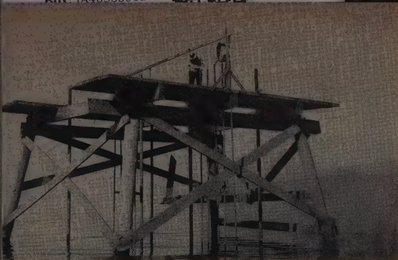
FIVE WOODEN ISLANDS were built last year in Great Salt Lake by SP in early phases of the railroad's construction of 13-mi. rock fill. While fill took shape at ends of present wooden trestle, tests of lake bottom were made from these platforms. Survey showed 15,000,000 cu. yd. of soft mud must be dredged away before mid-lake part of fill can be dumped. In distance is Promontory Point where new fill material will be quarried.
