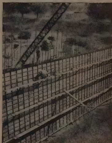
Section of exterior battered wall 31' high, showing Uni-Forming nearly complete. Uni-Form Scaffold Brackets replaced costly conventional scaffolding systems.
