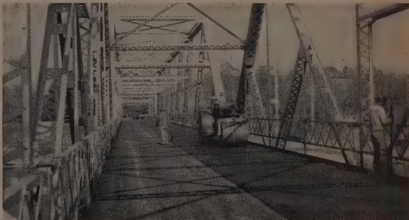
Contractor is compacting the second course of asphaltic concrete over Armco Bridge Plank installed on this old bridge.
