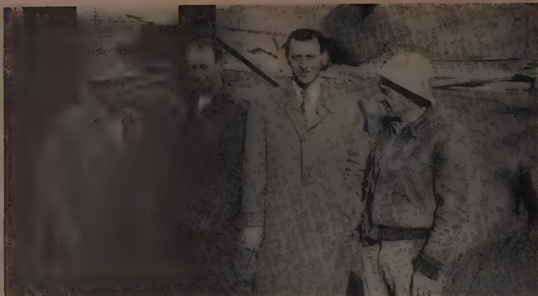
PERSONNEL on the bell caisson job described on pages 36 and 37 include (l. to r.) J. Brozman , inspector for the University of California; J. Mahaffey , superintendent; Don Mahaffey , contractor, and A. Austin , underground superintendent.
