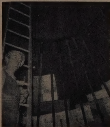
AT THE BOTTOM of one of the largest caissons the shoring technique can be seen clearly. The pipe lagging forms the contour of the bell and rests against the casing at the top. As the pieces of sheet metal are placed behind the lagging dirt is tamped behind them to keep the original soil in place. As concrete is poured the casing is withdrawn.
