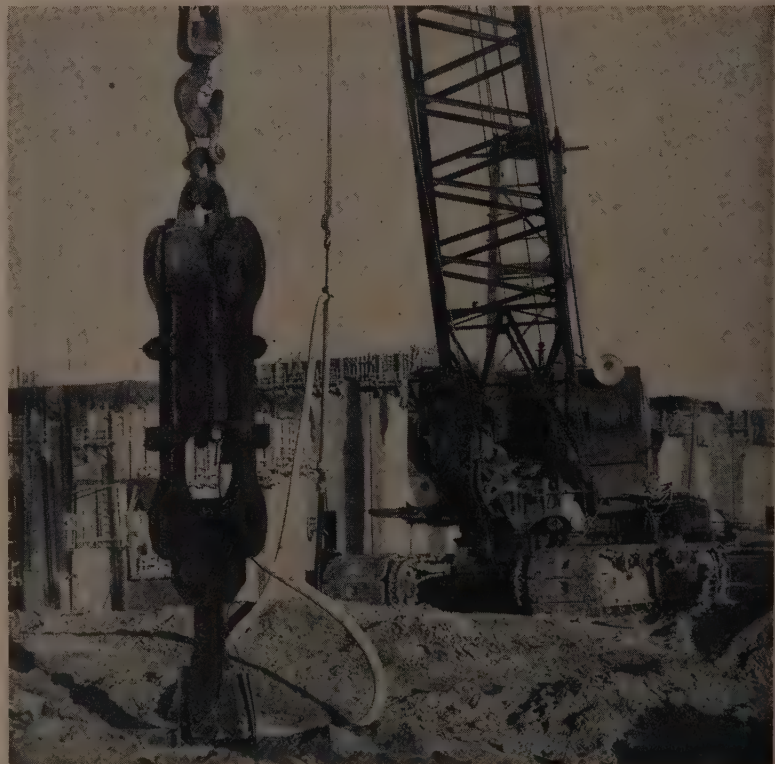
Steel sheet pile stubbornly set in hard rock in constructing the Buggs Island Dam across the Roanoke River in southern Virginia breaks loose under the blows of a McKiernan-Terry E4 Double-Acting Pile Extractor. McKiernan-Terry Corporation, 24-A Mercer St., Dover, New Jersey.
