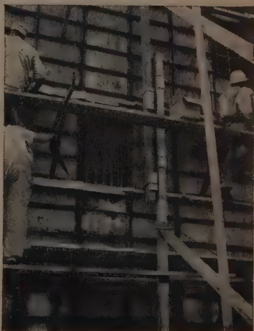
Pouring pockets permitted specified control of concrete placement.
