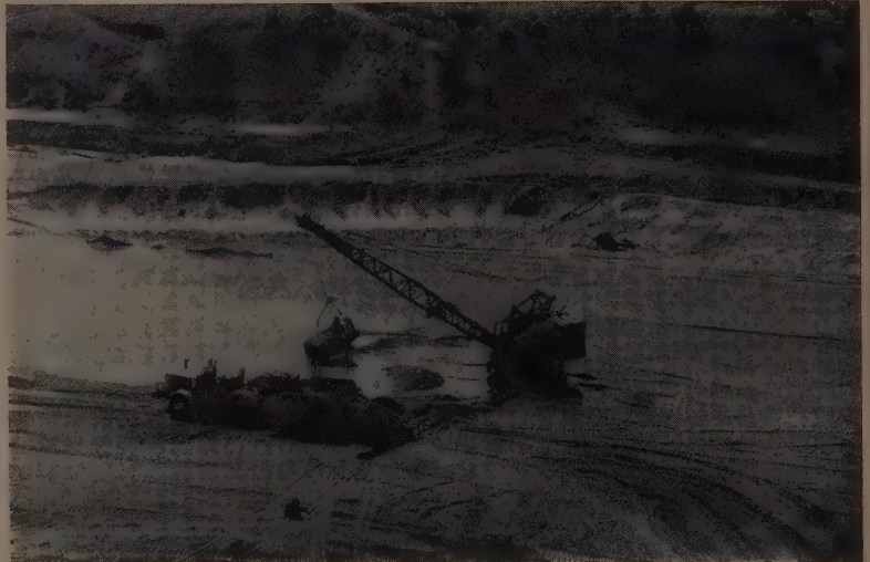
A NORTHWEST DRAGLINE loads scrapers with pervious material from upstream river bed while a Cat D8 in the background heaps up material in preparation for easy scraper loading.
