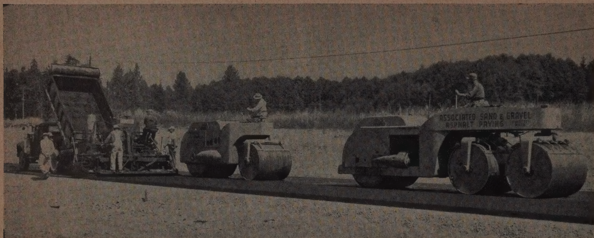
ROLLING longitudinal joint immediately behind paver to eliminate joint ridge. On all types of asphalt surfacing the combination of transverse
