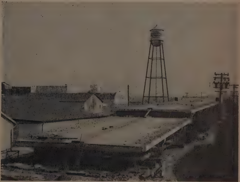
AFTER: One section is in place with one more section remaining to be lifted. The edge nearest the camera will be raised 13 ft. The entire low section is on rollers as it was necessary to move it back about 6 in. to disengage an expansion joint.
