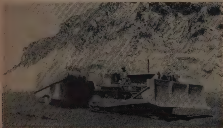
A CAT D8 pulls a Southwest 50-ton pneumatic compactor over the fill in the upstream pervious zone. Other compaction equipment includes a Southwest sheepsfoot and a Le Tourneau-Westinghouse sheepsfoot. Most of the pervious material is being taken from the upstream river bed. The impervious borrow area is on the south bank of the river.
