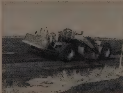
Cuts drainage ditches
