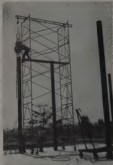
ROLLING TOWER is effective aid in mounting jacks on the column tops. Projection on jack base provides moment connection.
