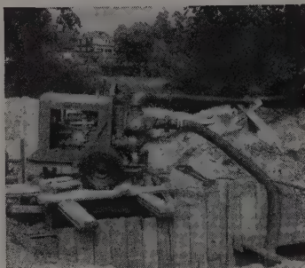
Model 36A-JF, on above project, has an A. G. C. rating of 90,000 G. P. H. at 25' TDH.
