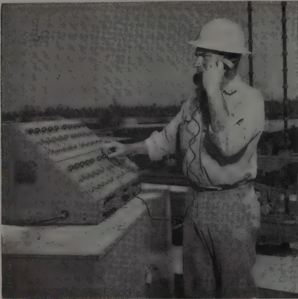
CONTROL of lifting is through the electronic panel (above, left) which automatically maintains slab level during jacking. One flip of the switch raises or lowers the slab 1/64 in. Jack (above, right) mounted on the column top includes an air-actuated hydraulic pumping unit.
