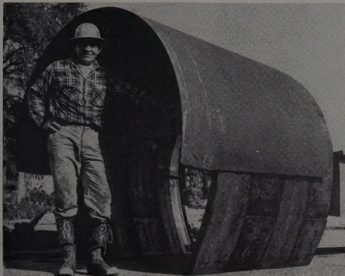
HANK EWART, general foreman, stands before the partial shield which was jacked forward into the sandy soil in unique driving operation. Shield is made of 3/16-in. plate rolled to shape of tunnel.
