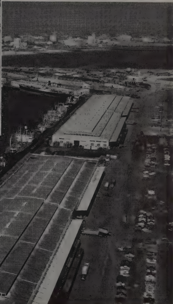
This is Pier "A," the world's longest. First to design and construct gigantic clear-span transit sheds, the port management also developed the use of 62-ft diameter circular steel cells formed with Bethlehem Sheet Piling to retain hundreds of acres of filled areas and to support its steel and concrete wharves.
