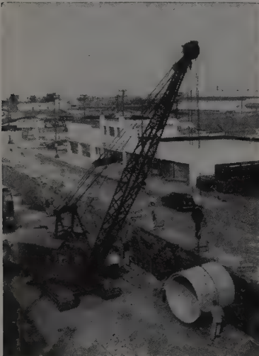
THE 84-in. pipe sections are placed with a Northwest Model 6—an average of eight are placed and covered each day.
