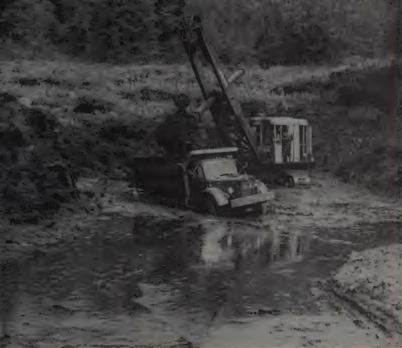
S & M Construction Company, Providence, R. I., uses 12 of these Mack LJSWX diesel dumpers under 2-yard Lorain shovel in excavating peat bog near Atholl, Mass., on a by-pass for U. S. Route 20.
