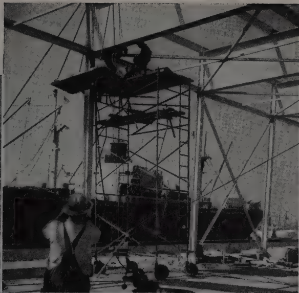
Another new clear-span transit shed takes shape on Pier 1 as Bethlehem Pacific crews speed the erection of structural steel. Support for the new building is provided by Bethlehem H-piling. Pre-cast concrete walls are reinforced by Bethlehem Pacific bars. General Contractor: J. C. Boespflug Construction Co. Designer: George F. Nicholson, Engineer.
