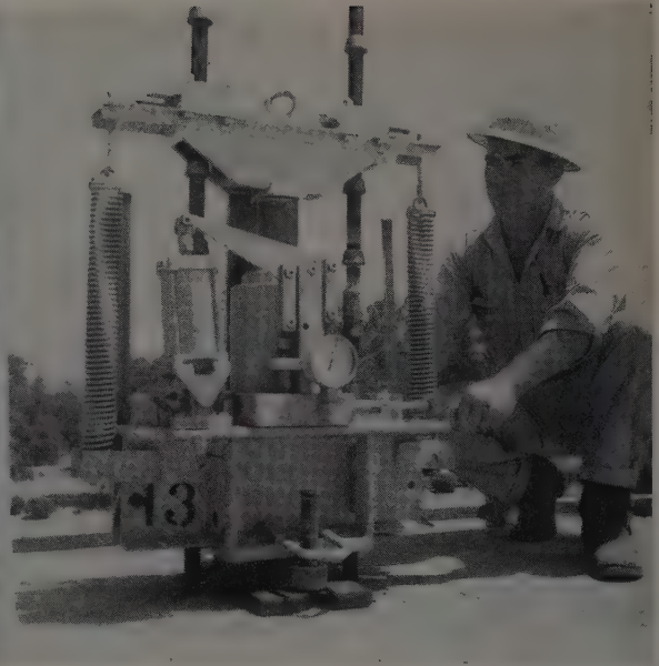
CONTROL of lifting is through the electronic panel (above, left) which automatically maintains slab level during jacking. One flip of the switch raises or lowers the slab 1/64 in. Jack (above, right) mounted on the column top includes an air-actuated hydraulic pumping unit.
