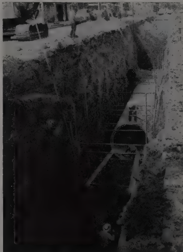
FIRM SOIL requires little shoring. Trench at this point is 28 ft. deep, 9 ft. wide at top, 18 ft. wide at the bottom.
