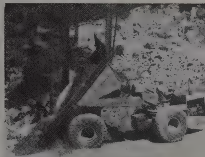
Tournapull dumps in ½ minute, including time maneuvering to edge of bank. "They're fast dumpers" says Operator Gordon D. Wood. Working a 58-hour week, Tournapulls hauled 75% of the material in this road relocation. Balance was moved by 2 crawler-scraper combinations and 2 crawler-dozers.
