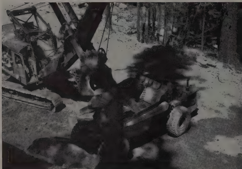
MOST ROCK along the new 9,600-ft. high Sonora Pass road was found in solid cliffs which had to be drilled and blasted. Only a few of the boulders were small enough to be hooked in the angle of the shovel bucket and hoisted into the rear dumps.
