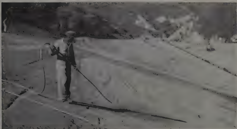
AIR JETS are used to remove loose material from the subgrade prior to laying the 3-in. asphaltic concrete lining. This is the first project on which a mechanical spreader was used on a slope as steep as 2:1. A spreader increases quality and quantity of work and provides compaction.
