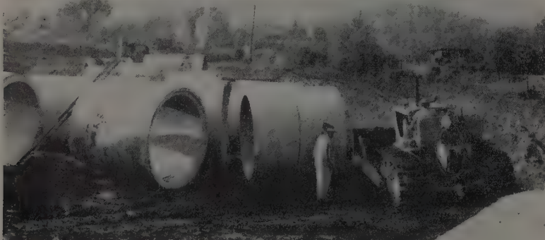
A CATERPILLAR D8 'dozes out a bench for the Lorain crane which will place the pipe. The sections shown are 90 in. in diameter, weigh over 10 tons. Specs call for 576 ft. of this size.
