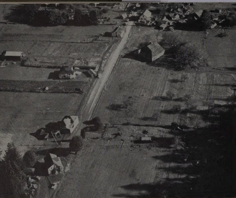
ABOVE —Houses on the roadway were a problem at Pepperwood, Weott, and Klamath. Some were remarkably intact and were moved to one side on rollers or dollies. Over 300 homes were completely destroyed in Humboldt County.
