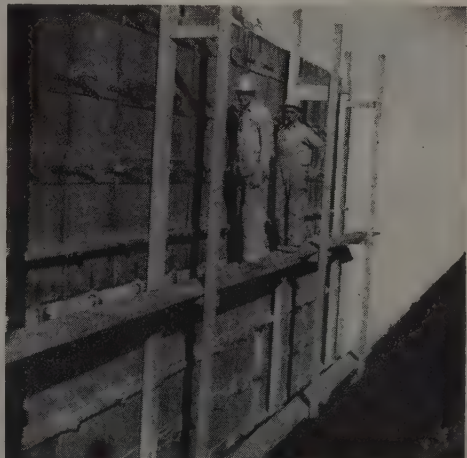
30 FT. SECTION IS STRIPPED and reset in one day for an every-other-day pouring schedule.
