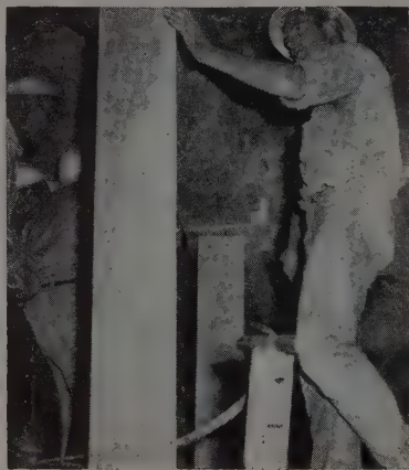
WORKING back from the face of the drifts this arch timbering was held with stulls against the core material until the nine segments were in place, making the arch self supporting. Stulls were then knocked out and the process repeated out toward the portal.
