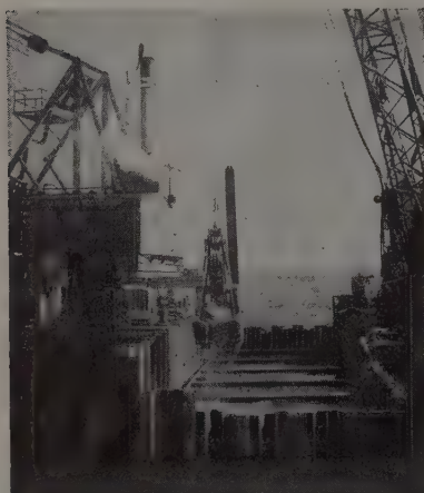
Foster Rental Piling forms cofferdams used in construction of the piers for the MULLICA RIVER BRIDGE Garden State Parkway
