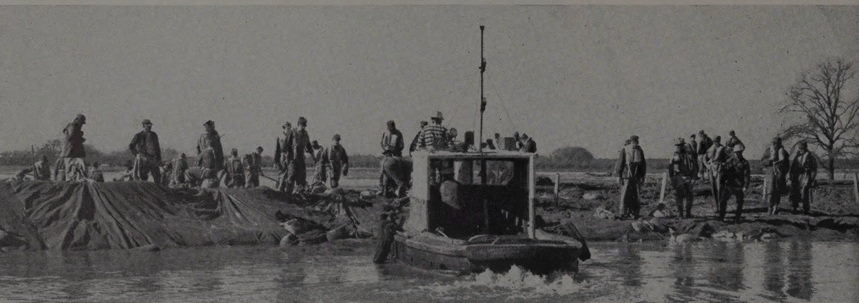
WHEN it became too muddy for equipment to move the work had to be carried on by hand. A detachment of men from Beale Air Force Base
