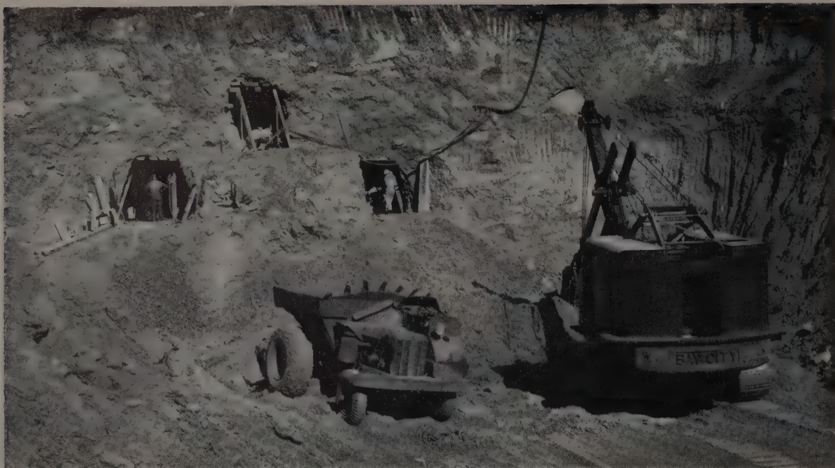
Three 7 x 7-ft. drifts, one at the arch crown and two at the location of the wall plates, were used by Colorado Constructors, Inc., to start
