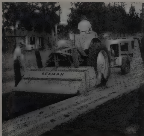
Above — Seaman Self-Propelled TRAV-L-PLANT in bituminous parkway construction, Jacksonville, Fla. Binder is pumped from transport ahead of the Seaman.
