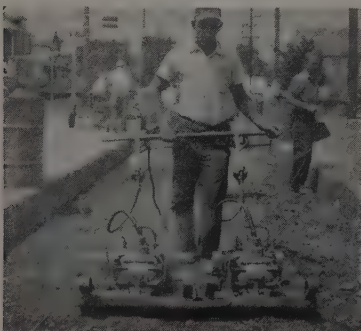
Above: a Jackson Multiple (6 units) on 7 mile sub-grade. Below: 2 units equipped with operating handle, self-propelling and easily operated by one man.
