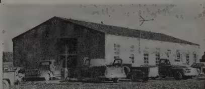
This 40-ft.-wide Armco Building was used by the Cook Construction Company, Jackson, Miss., as a repair shop on Ohio Turnpike.
