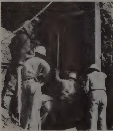
WORKING in from the portal, these 12 x 12-in. plumb posts were set to support the wall plates as excavation advanced. The picture shows one of the many elements of tunneling where mechanization will never replace human skill and plain, old muscle.
