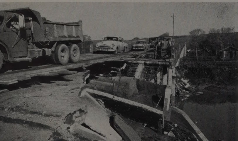
BELOW —Timber planking keeps a bridge open until permanent repairs can be made. The Humboldt County road system had 38 bridges knocked out—about 19 to be replaced.
