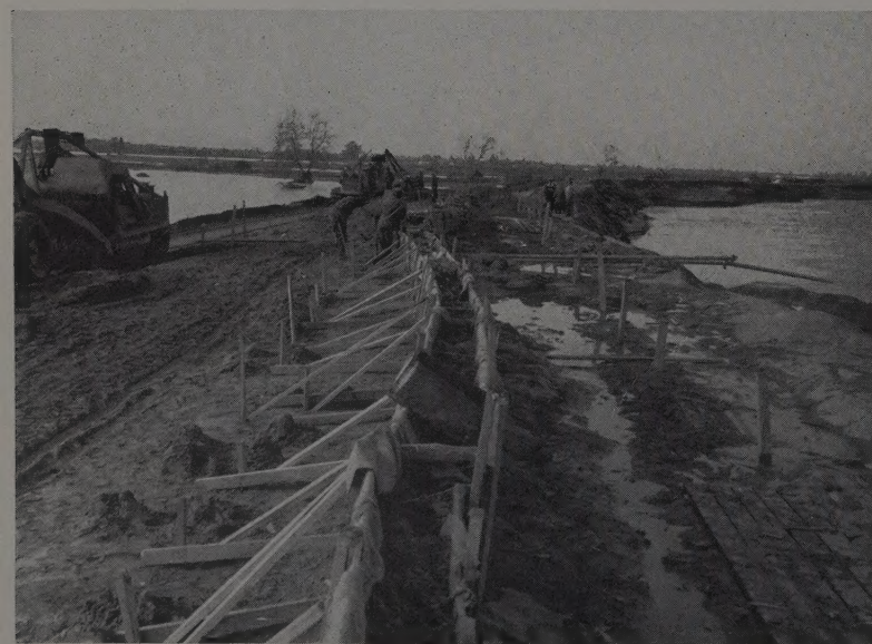
AT LOW spots on the levee 3-ft. high wooden walls were thrown up and filled with soil—to hold back the Feather River. Men and machines worked day and night for three weeks.
