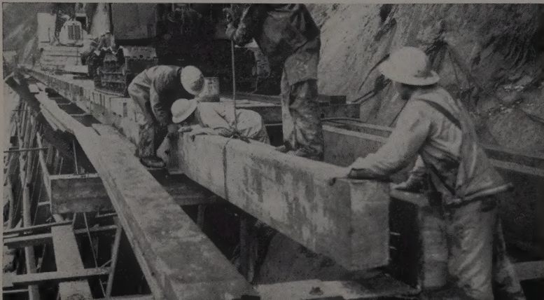
GOING INTO place is an 8x18-in. fir stringer to close the gap. Trains were running here a few days later. But on January 27 about 135 ft. was taken out again by a landslide.
