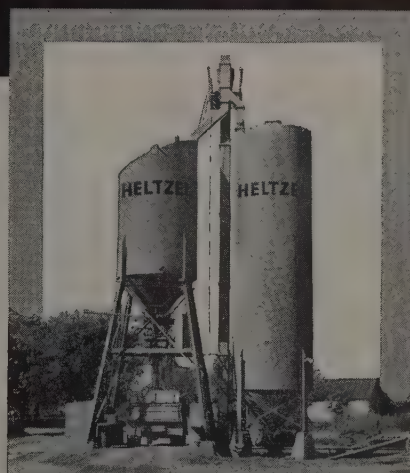
Heltzel's Advanced Flare-Legged E-3 Cement Batching Plant with high speed recirculatory system in use on midwest paving project.
