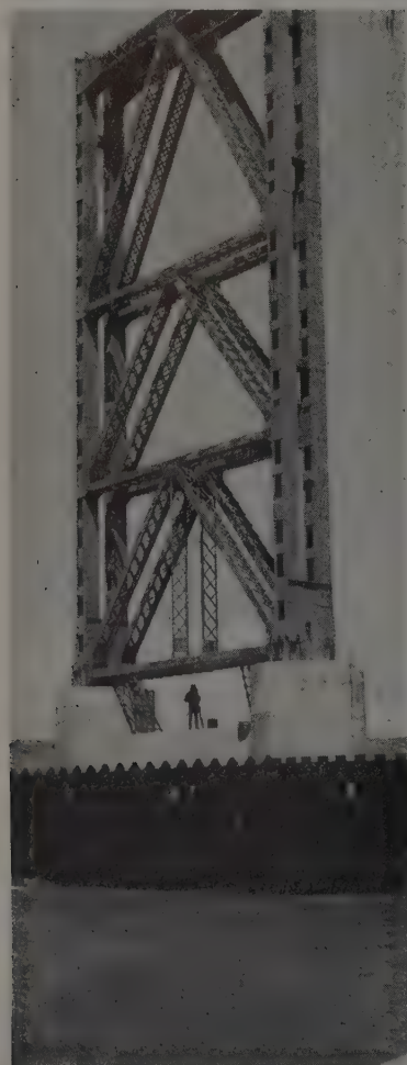
COMPLETED timber fender is of flexible design to reduce possible damage to ships. About 1,450 spliced piles were required for the piers of the Richmond-San Rafael bridge.
