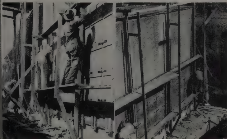
STRIPPING OPERATION IS FAST and the concrete surface is smooth. The absence of spreaders speeds-up form setting and makes finishing the concrete after stripping easier.
