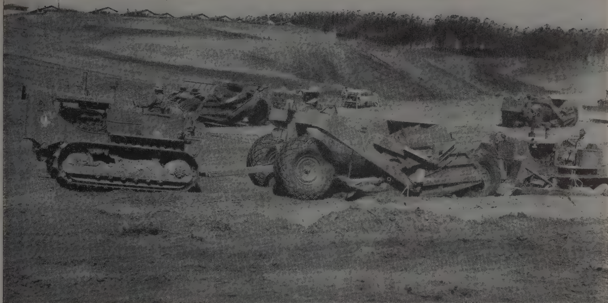
These two Allis-Chalmers HD-16 Crawler Tractors, one pulling and one pushing a scraper, are both equipped with A-C Torque Converter Drive — which incorporates Twin Disc Torque Converter components.
