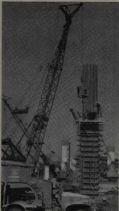
WORKMEN stand on shelves supported by steel brackets attached to forms to assist pour. Concrete lifts were usually about 25 ft.
