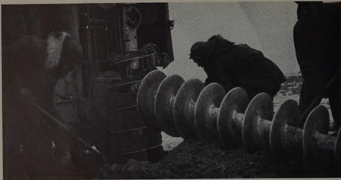
DRILLING an 18-in. hole for a timber pile that will be frozen into the permafrost. Refrigerating pipes are attached to the pile, the hole filled
