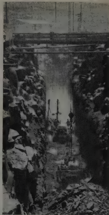
TOUGHEST JOB was the excavation of this slot for the south fishway channel. With no access at either end it called for ingenious selection and use of equipment.
