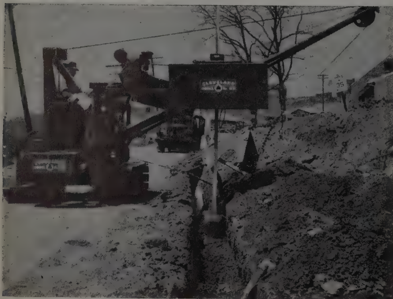
Same job—same day—same "80W"—backfilling and tamping.
