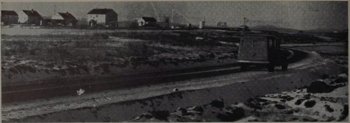
FIVE MILES of access road had to be built across the tundra to reach the job site. The 3-ft. depth of sand fill placed as a base kept the heavy
