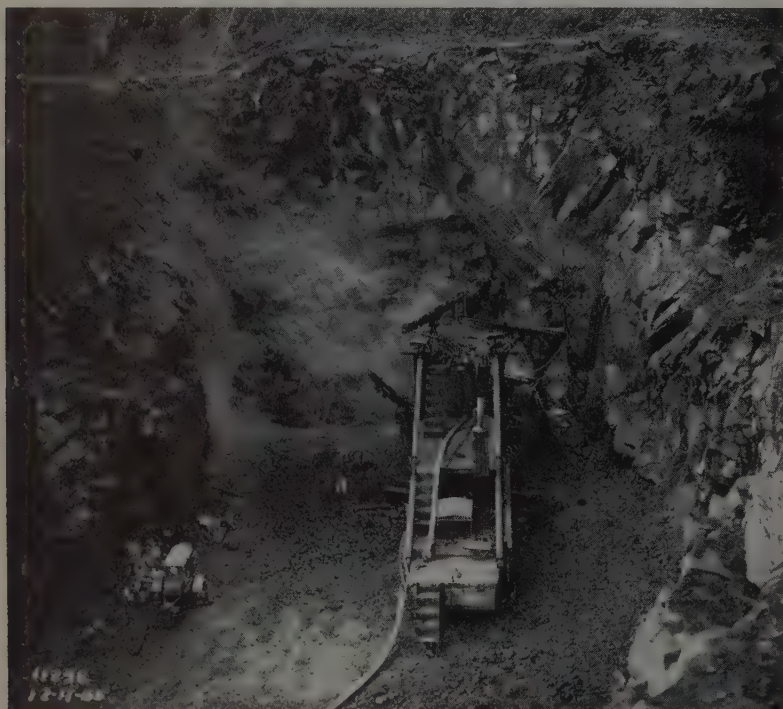
Photo from Tacoma Dept. of Public Utilities
