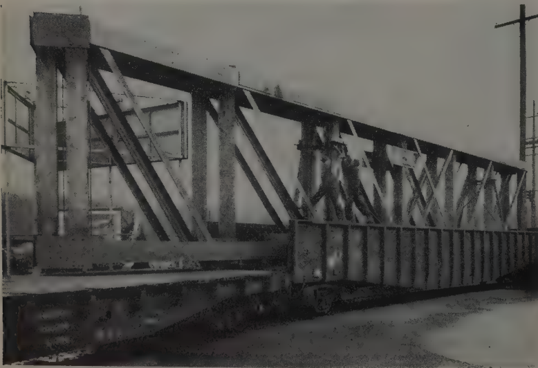
FIRST STEEL FOR PORTLAND BRIDGE
