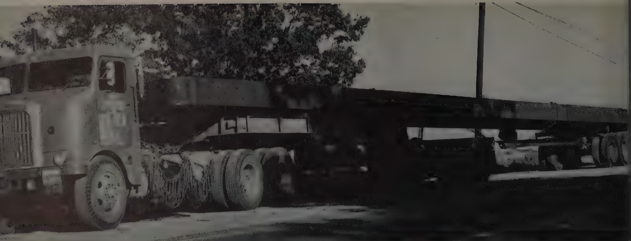
WEIGHING 35 tons, this 90-ft. plate girder was trucked to an overpass job near Ashland, Oregon. Because of its length a dual axle pole dolly
