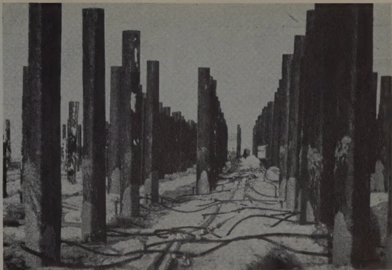
TIMBER PILES frozen by refrigeration into sockets drilled into permafrost. This view is of an installation similar to the one now under way at Bethel. The piping for the refrigerant leads to pipes fastened to the pile before it is placed in the hole.
