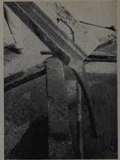
SLURRY from the transit-mix truck is poured in as the screed is towed forward by the same truck. Note the consistency and the uniformity of the mix. Sand used for aggregate will all pass the No. 8 sieve.
