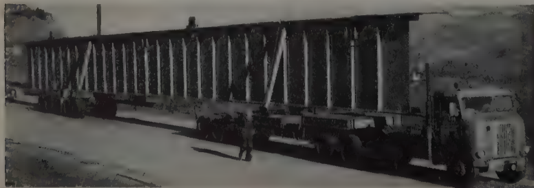
ON A HIGHWAY bridge job in Washington this 122-ft. long girder was one of two weighing 49 tons each that were moved from railroad siding to site. For this haul the second dolly had a tongue extending to the rear, and steering was done by a following vehicle.
