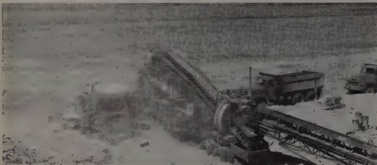
THROUGH THE PLANT the key is control to meet ever-tighter engineering specifications and flexibility to change from one type of product to another. For example, this plant had to switch fast from building a stockpile of graded material for plant mix surfacing to producing sub-base material. Finishing one job, a rapid move to the next is a characteristic of the modern plant.
