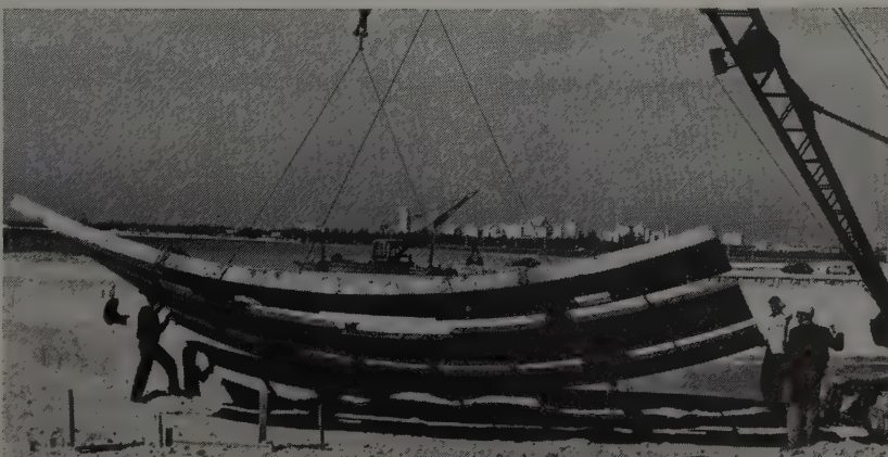
Prefabricated welded segment of tank goes into position on concrete base
