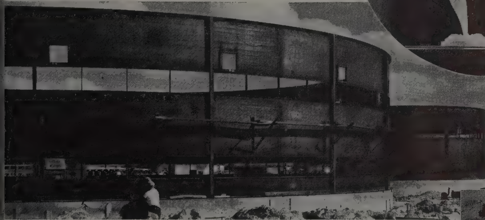
The steel aquaria under construction. 80 ft, 565,200-gallon tank in foreground, with 50 ft, 260,252-gallon tank in rear. Acclimating flume connects both tanks
