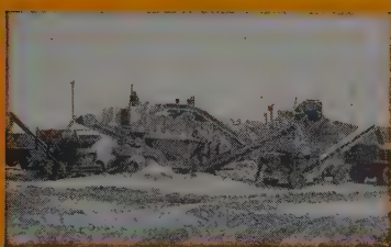
Hammermill Secondary Plant , a complete gravel crushing and screening plant, produces roadrock or aglime or a percentage of both at the same time.
