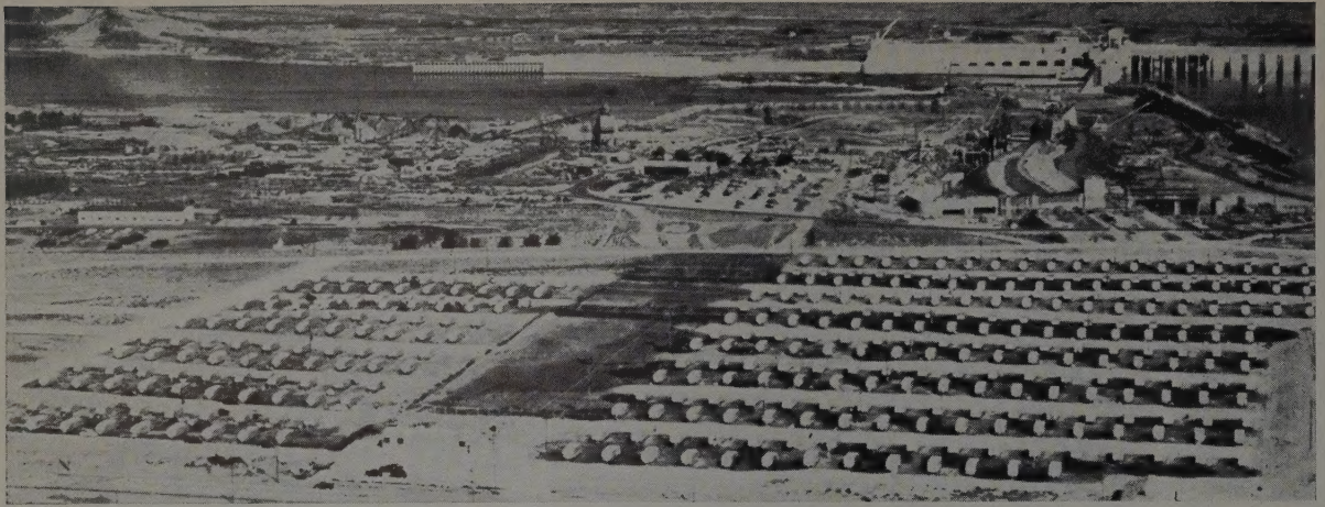
AT THE McNARY DAM project this orderly layout of about 600 mobile homes houses a part of the construction force. It has been estimated
