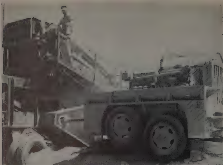
MOUNTED on its own rubber, this Cat D364 power plant was used by Jack Parson of Smithfield, Utah, to drive this Pioneer 35-S plant. This type of hook-up eliminates use of flat-belt drives which can be troublesome during the summer showers common to the Western mountain country.
