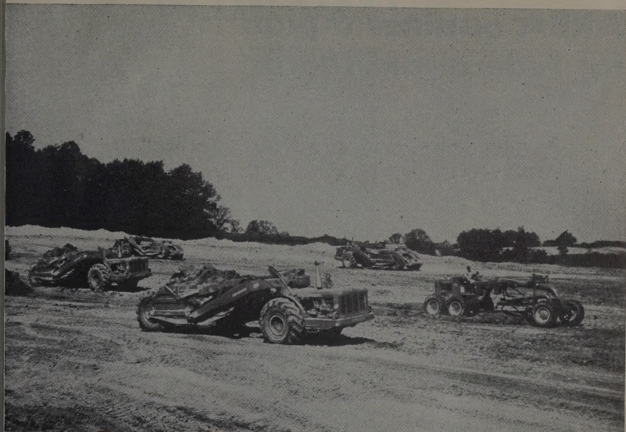
A new toll road takes shape in northern Indiana
