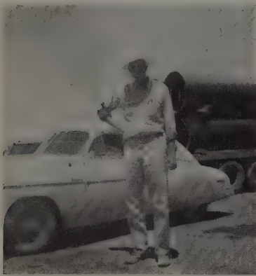
JAMES W. SCHELL , superintendent on the Bear Creek flood control dam near Merced, Calif. Ferry Brothers was the contractor on the Corps of Engineers project.
