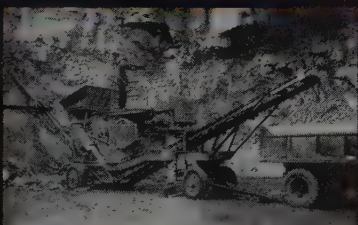
Single Pass Plants for low-cost crushing units where material does not have to be accurately graded, and for jobs where portability and fast set-up are important.
