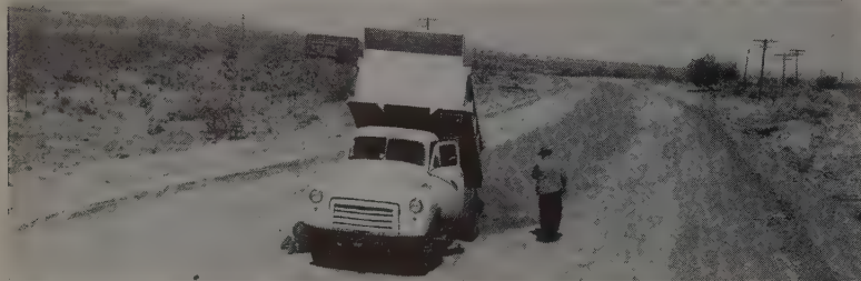
ON THE ROAD goes thousands of tons of base course to support the new and rebuilt highways of the West. This may be specified as minus 2\frac{1}{2} or 3 in. and the volume of output holds the key to success on the job. But the same specifications may hold rock chips within narrow limits of tolerance. Flexibility must extend to producing concrete aggregates.
