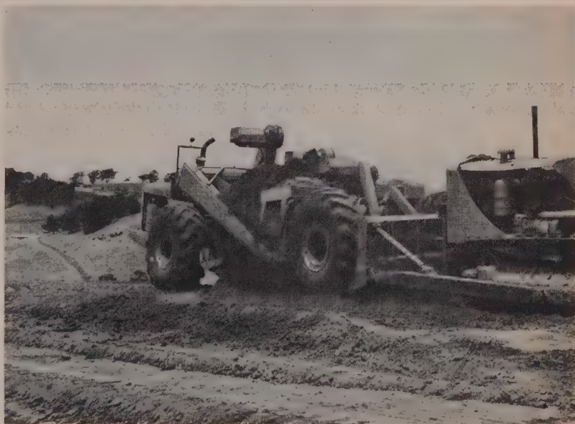
R. A. Farish, San Francisco, coupled his 2 "C" prime-movers to scrapers for subdivision grading in Belmont, California. Units moved 286 pay yards of clay and common earth hourly over 1125' cycles. Changeover takes only a few hours.
