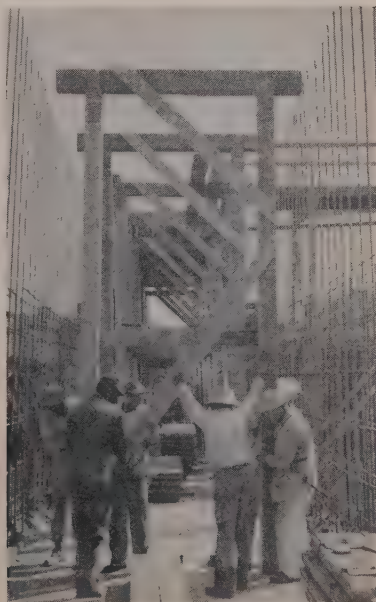
FALSEWORK for the roof, shown going into place, will also support scaffolding for erecting inside plywood panels.
