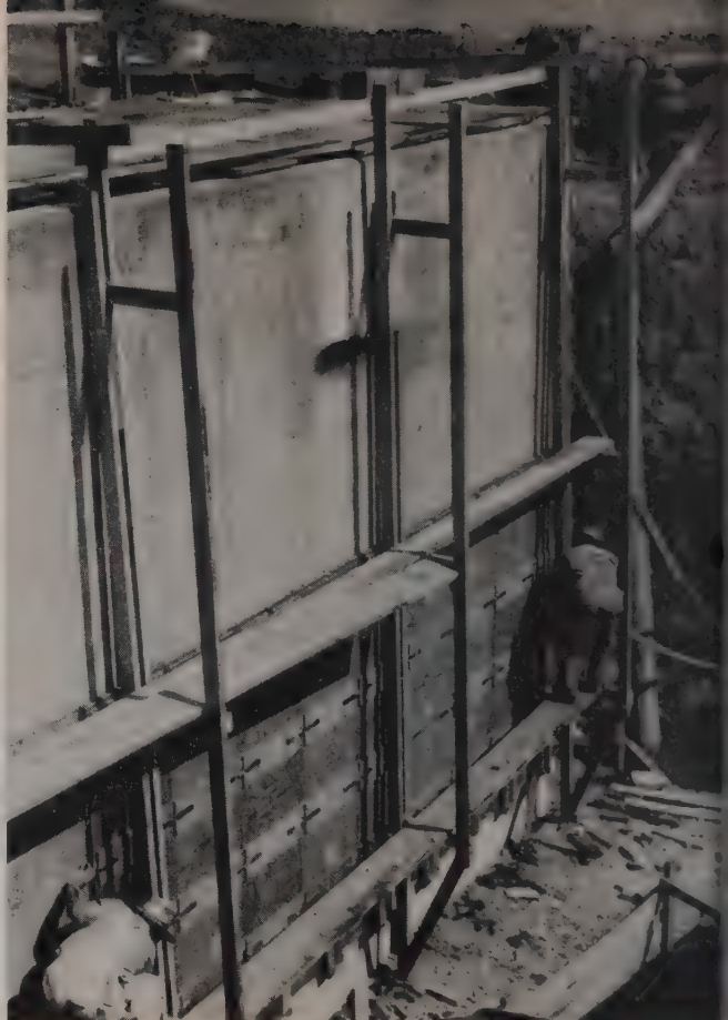
STRIPPING the panels is fast and the concrete surface is smooth. A 30-ft. long section is stripped and reset in one day for an every-other-day pouring schedule.
