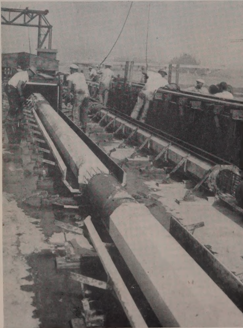
FORM STRIPPERS are close behind as the end of the 500-ft. line is reached. Next step will be to cut the strands between the piles with a torch and load the piles on a barge for trip to job.
