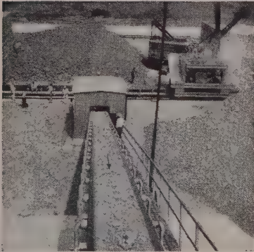
Sulphur is weighed "on-the-run" as it rides slope conveyor to loading tower.
