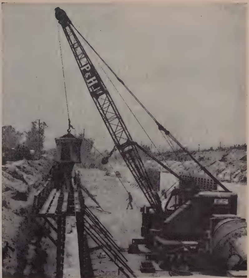
CONCRETE WAS HANDLED by this P & H crane with a 1-cu. yd. Gar-Bro bucket. In the right background are two of the 11-ft. high, 54-ft. long panels used to form the walls.
