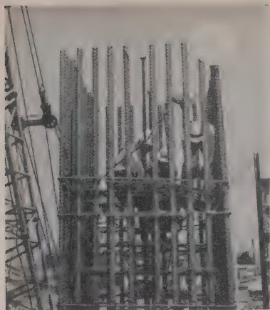
THE REINFORCING bars are 2\frac{3}{8} in. in diameter—800 tons were used. Inside the column grout pipes are being positioned.
