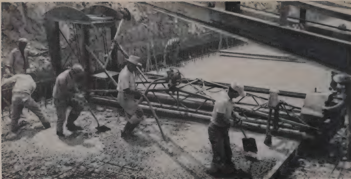
THE PAVER OPERATOR gets this view of the slab pouring operation. The 6-ft. high offset on the left end of the finisher enables the finisher
