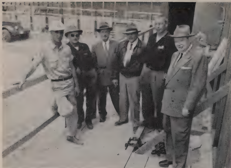
CHIEF PERSONNEL in charge of construction on Webb & Knapp's $35,000,000 Court House Square development in Denver, Colo., are, l. to r.: G. E. Lapham , assistant general superintendent; F. G. Chaisson , general superintendent; J. J. Wetzel , business manager; J. E. Smith , assistant project manager; A. J. Magee , resident engineer, and T. J. Smith , project manager. The names of other key men appeared last month.
