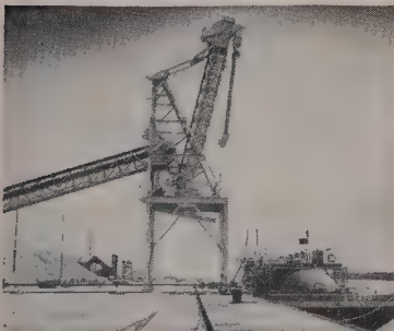
Ship loading boom conveyor in raised position to clear ship superstructure.
