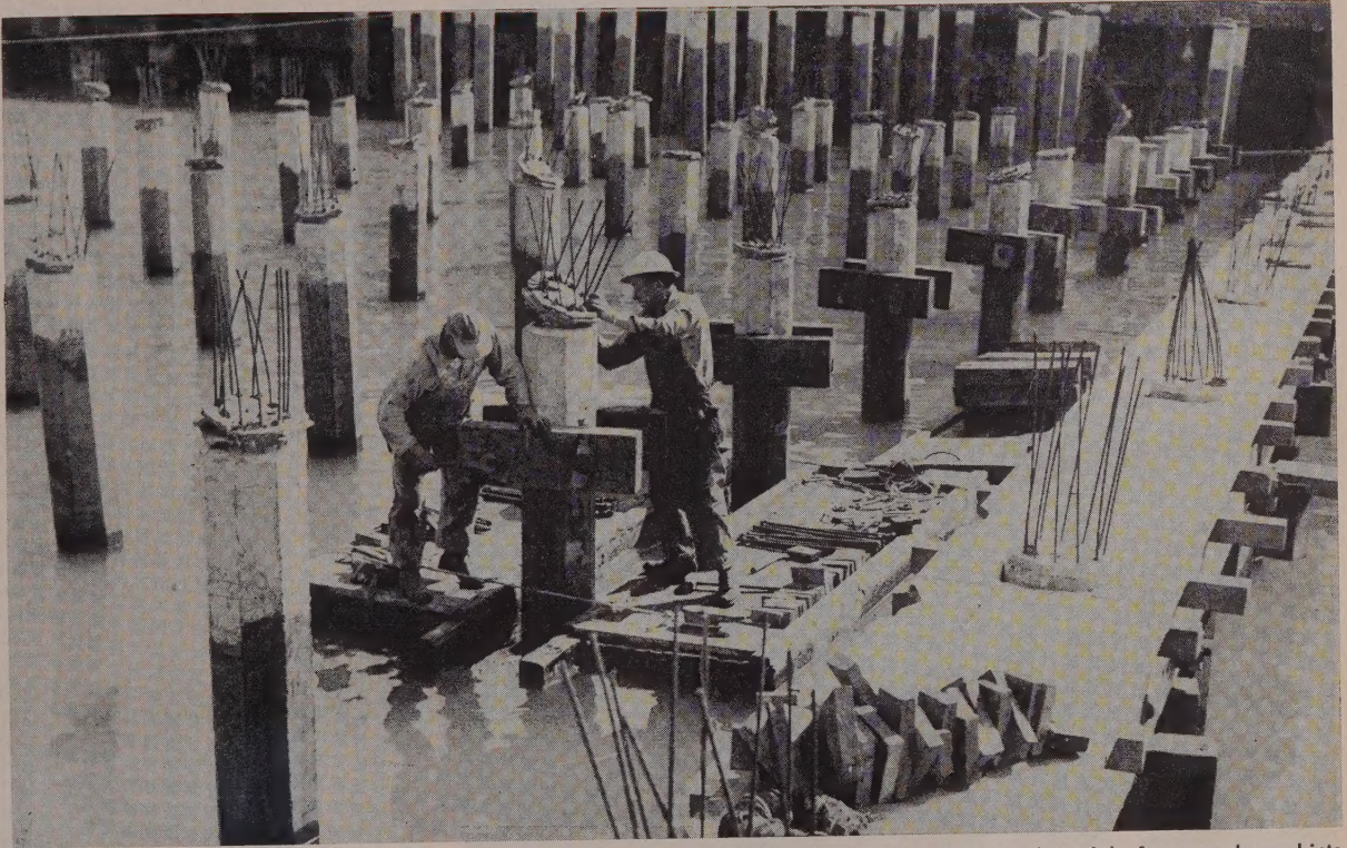
FLOATING ON RAFTS, workmen fasten 6x12-in. blocks to the piles by tightening 1-in. bolts. All formwork is supported by the blocks.
