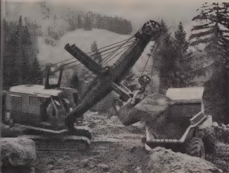
Babler Brothers, Eugene, Oregon, used "C's" with rear-dump bodies on this 160,000-yd. 7-mile relocation of U.S. 99 near Anlauf. All-steel body easily withstood shocks of loading big-chunk rock. Short 14'4" turn radius speeded positioning at both shovel and dump.
