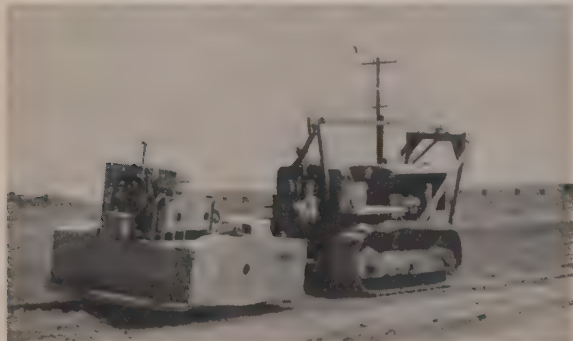
MODEL 25 on a California highway job produced 90% density with two coverages on a 4-in. lift after the contractor had been taking sixteen passes of a sheepfoot roller to secure this density on an 8-in. lift. Soil was decomposed granite, moisture averaged 7.2% and forward speed was 2.5 mph.
