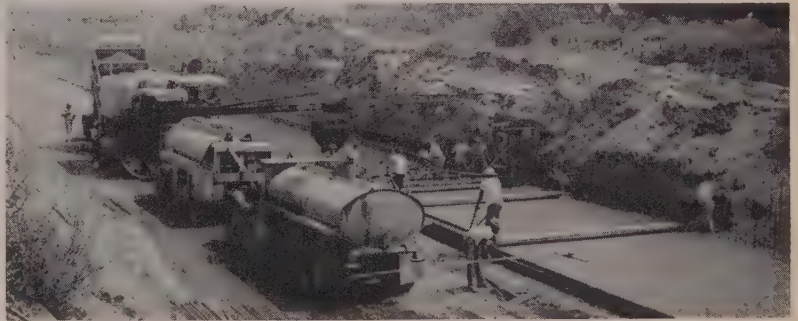
A COMPARTMENTED dump truck is depositing its load into the Rex paver. The paver tows generator trailer with the water truck bringing up the rear.
