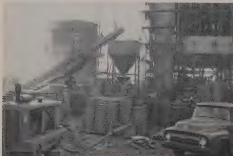
BATCHING grout took place at foot of structure with aid of conveyor and hopper shown here. In the background one of the steel vessels is being fabricated which later will be lifted into place.
