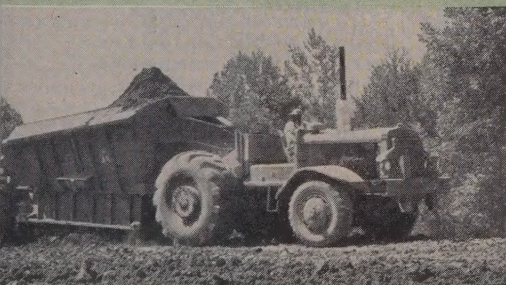
Dumping their big loads on the fly, Bottom-Dump "Eucs" made fast cycle time from borrow pit to fill and back again. They were loaded by 2½ yd. draglines and a Euclid Loader.
