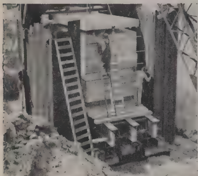
Checking Foundations with 120-Ton Load on H-Bearing Frames Anchored to Foster Piling Hotel - Department Store - Parking Facility THE DENVER COLORADO PROJECT
