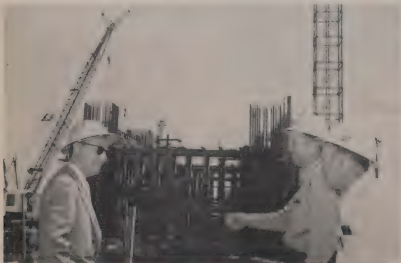
ON THE JOB during the first pour were R. C. Richardson of Gilmore Fabricators, Inc., steel suppliers and Bechtel's George Wilcox, superintendent, and Bill Shellhase, senior field engineer.
