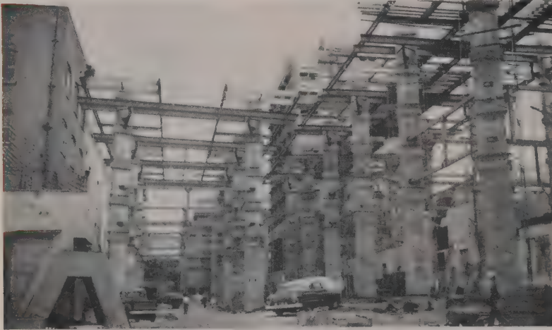
PRECAST COLUMNS, 40 in all, in place with first part of form framework at the top floor. The timber frames at middle of the columns stiffen the structure until top two floors are poured.
