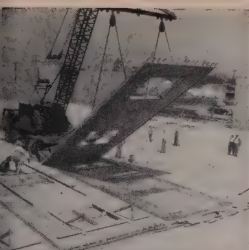
PRECAST PANEL 32' high, 18½' wide with two large window areas.
