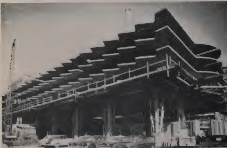
FORM LOWERING is under way. The top three slabs have set up and the forms are being positioned for the fourth pour. Two hand-operated winches at each column handle the lowering.
