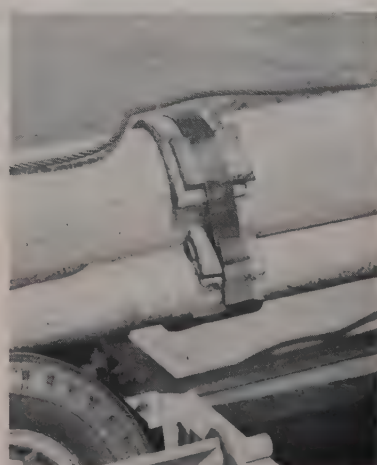
READY FOR PULLING , the band is shown with the padding of Panelcraft to protect and cushion the pipe coatings.
