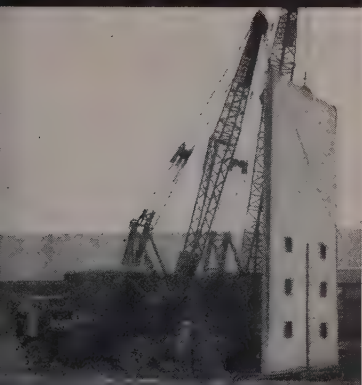
114,000 LB. SLAB being positioned
