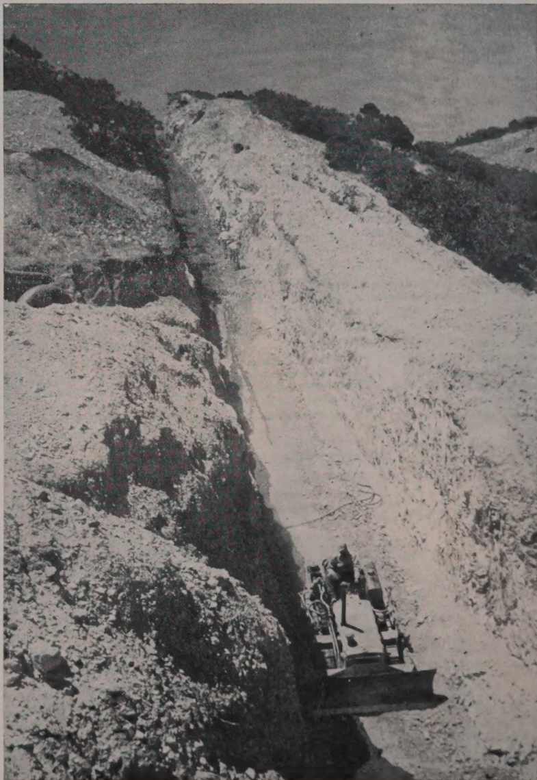
A CAT D4 fine grades a 52% slope before placement of the 48-in. diameter concrete pipe. Benches in the hillside to the left is where crane will be positioned to place pipe.
