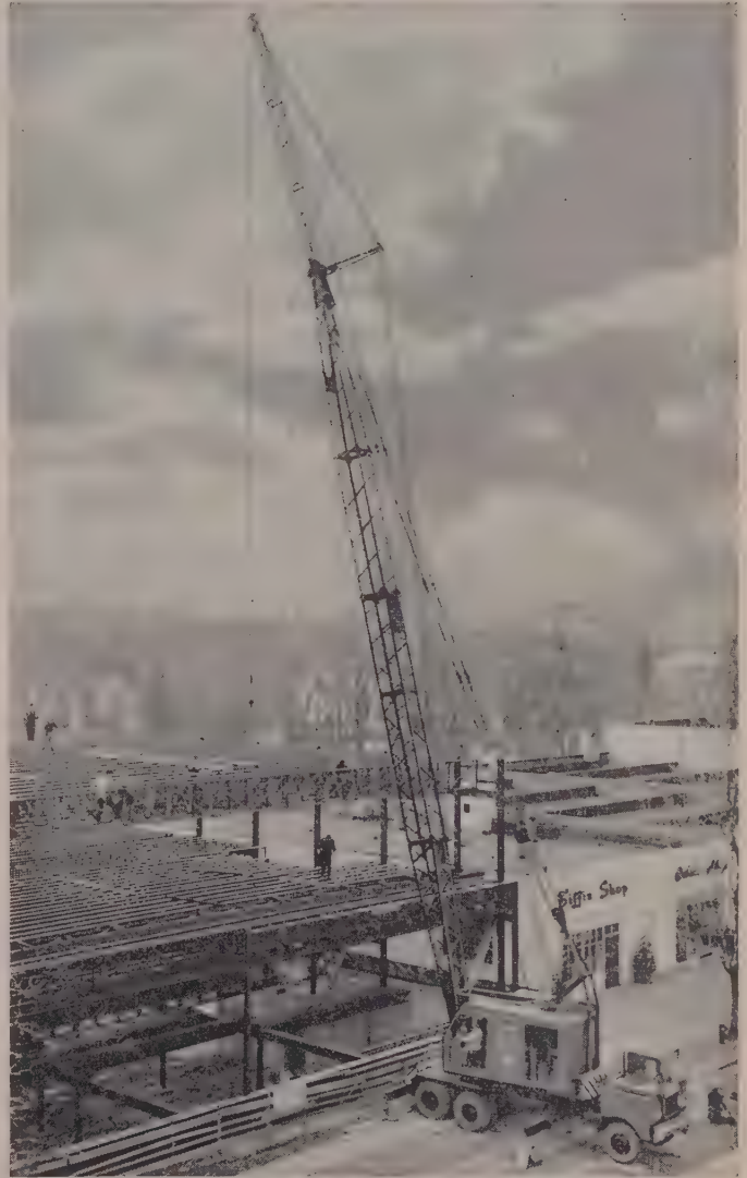
HC-98 Zephyrcrane with 80' boom and 20' jib works quickly, spots loads gently, accurately. Operator has clear, up-front visibility.
