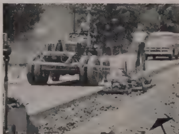
The MULTIPLE on base course of a widening job 36" wide, 9" thick. One of the compacting units fitted with operating handle and used individually.
