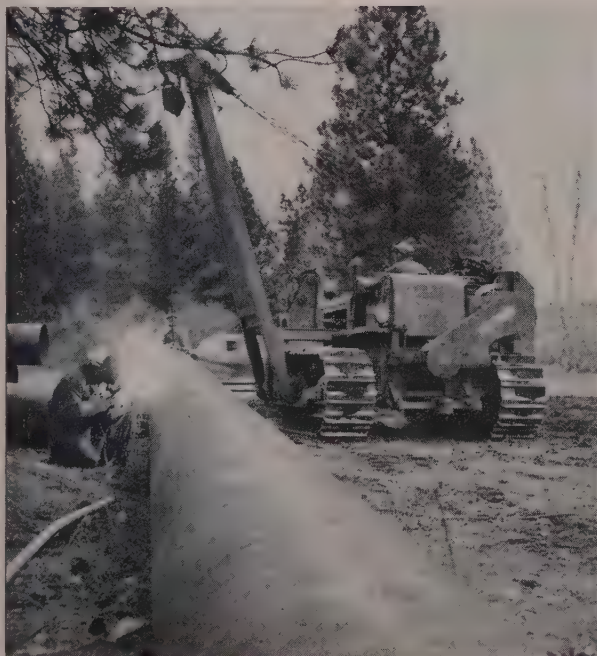
WELDERS double joint 24-in. pipe to save installation time.
