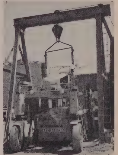
FULL CONTAINER has been hoisted, as carrier backs away. Truck is shown moving under container and will take on box in its truck body. Containers are attached by chains to the bed of the truck so that with end gates of box and truck down the load can be dumped without delay.
