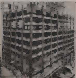
Erection of the Equitable Life Assurance building in San Francisco showing tapered continuously welded columns and "butterfly" spandrel beams which are welded to the columns.
