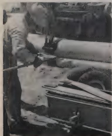
BANDING was carried out with standard tools using a 2-in. steel band. Spacing was at about 10-ft. intervals.
