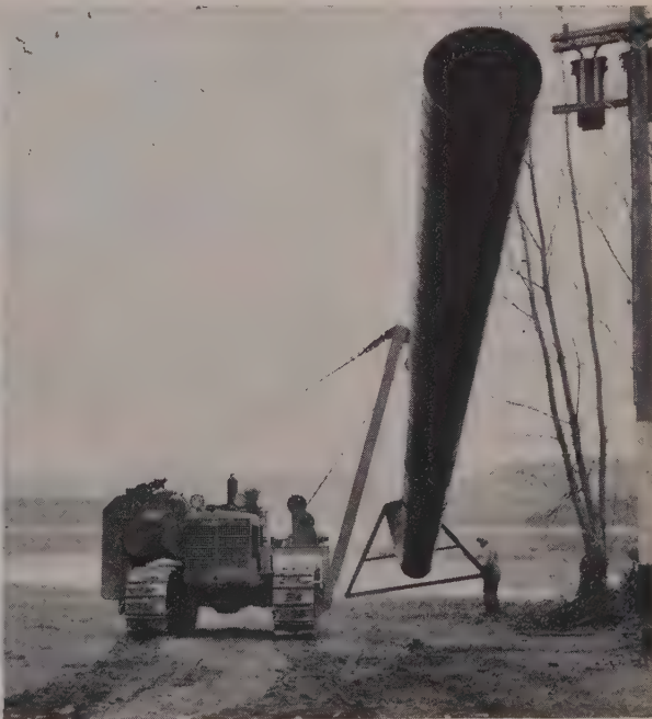
INTAKE pipe into lake is placed with TD-14S and sideboom.
