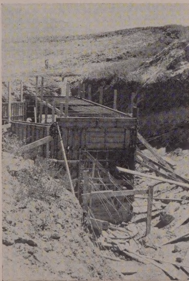
ECONOMY STEEL FORMS outline a structure that will serve as combination vent, turnout and wasteway. Form assembly went rapidly.
