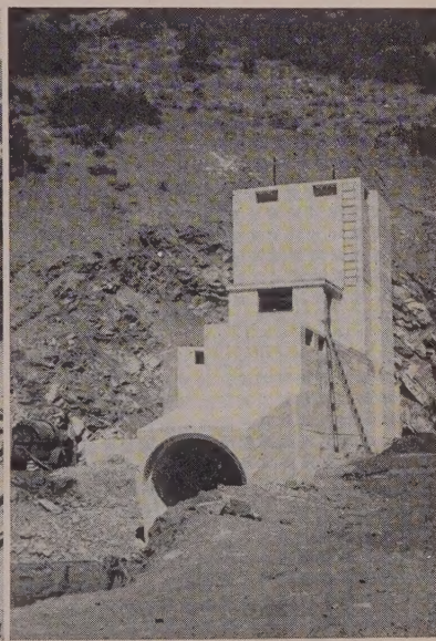
BIFURCATION STRUCTURE at lower end of tunnel splits water. Part goes to Weber Aqueduct, part to Davis Aqueduct.
