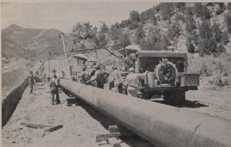
WELDING the sections together is a fast moving operation. For the stringer pass and the hot pass, welders are located on both sides of the pipe. Lincoln welding machines furnish 300 amp.
