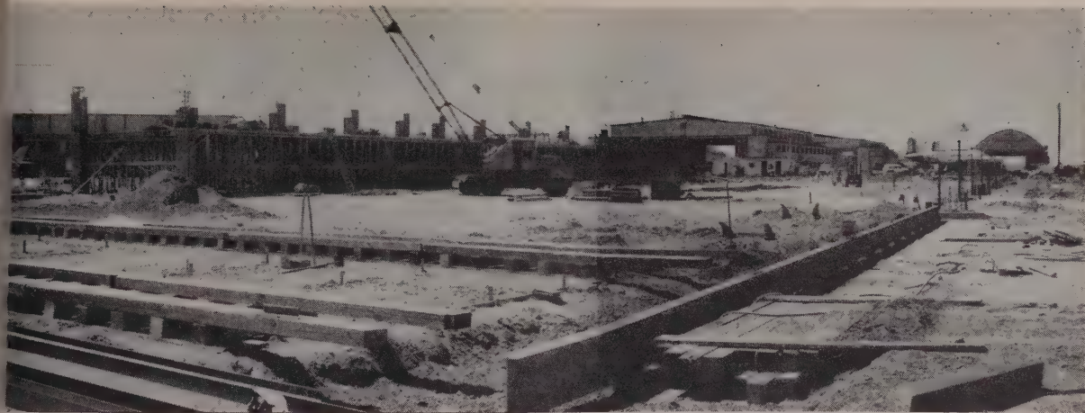
PRESTRESSED GIRDERS 136 ft. long will be formed and poured in a yard at the left edge of the picture. They then will be rolled on rail-
