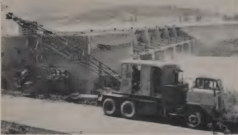
FINISHING UP AT DEXTER DAM
