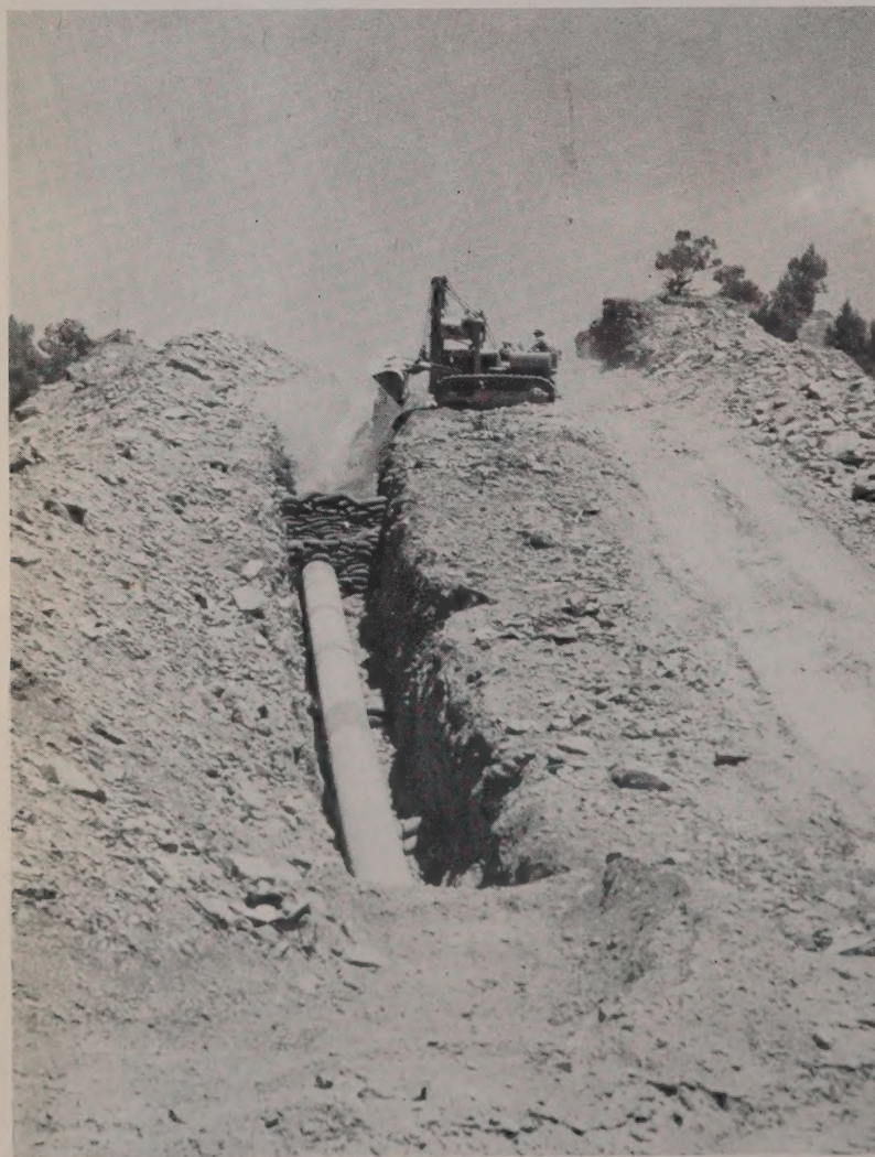
BACKFILLING with fine material in rocky stretches is a job for this front-end loader. He makes his haul with material from the foreground.
