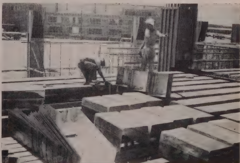
PAN-TYPE JOIST construction with 2-ft. 3-in. spacing was used to span the 31-ft. distance between girders on the two-story section of the building. These sheet metal pans are 1 ft. 8 in. wide and leave a 3-in. thickness of slab between joists. Rapid erection of formwork was typical of this system and procedure.
