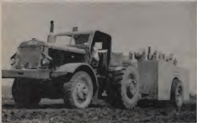
COMPACTION of lifts is handled by Ferguson and Southwest 50-tonners. First pass is the toughest, and wheels slip if already loose material is a little too wet.
