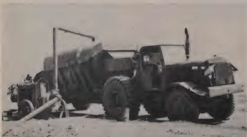
WATER is supplied in 5,800-gal. loads from this odd rig, converted by Lefever from a bottom-dump Euclid. Big capacity means more time on the fill, keeps work going smoothly.
