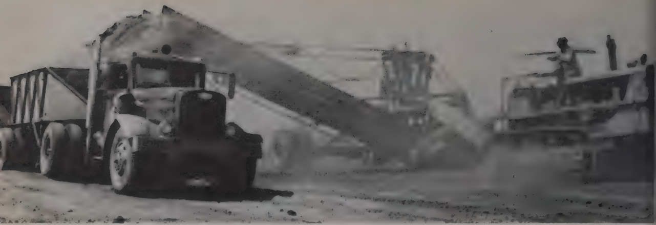
NATIVE SOIL breaks out easily for Morrison-Knudsen and Westbrook at March Air Force Base. The big thing is putting it back, 6 in. at a
