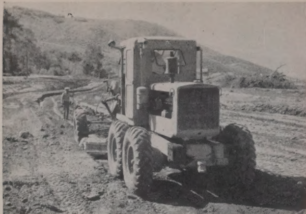
CANAL SECTION is developed by a series of steps shown on this page. Leading off is a grader to define the 4-ft. wide berms.
