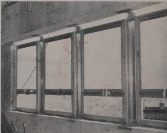
Over 7,500 studs were installed to secure the clip angles that in turn hold the panel units. First panels were given extensive testing to determine vibration and waterproof characteristics.
