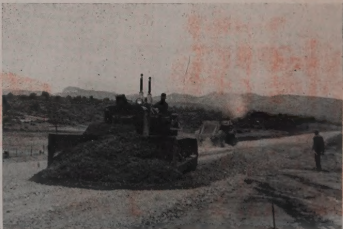
ON THE GRADE the material was spread and rolled in 6-in. lifts to make up the 11 to 19-in. thickness of base.
