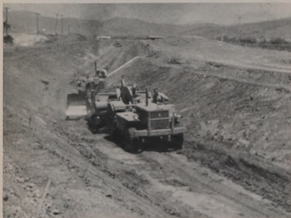
BOTTOM 10-ft. width is reached and the smaller Cat DW 10s are used rather than the bigger Wooldridge scrapers used at first.
