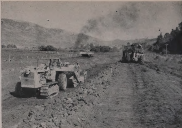
SCRAPERS MOVE in to rough excavate for the 9-ft. depth and 1\frac{1}{2} to 1 side slopes. Roadways are built up on each side.
