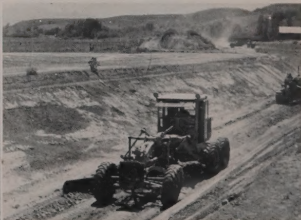
TRIMMING THE SLOPES and the bottom to accurate line and grade is the next important step prior to using slip form paver.
