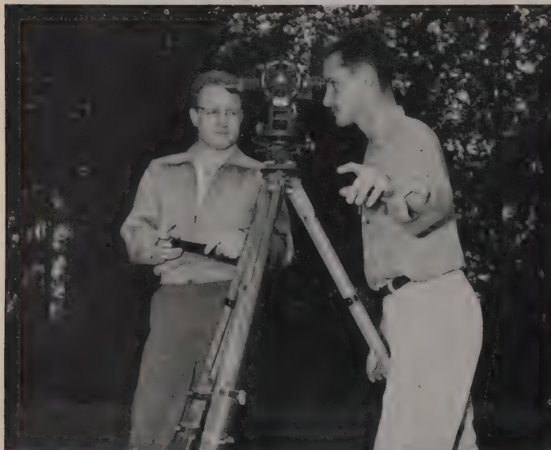
STUDENT ENGINEERS from the nation's colleges have summertime jobs with the Alaska District, Corps of Engineers, on defense construction jobs throughout the Territory. Here, one of them, Ted Spittler (on the transit) signals his directions to the chainman, as Burt Rochefort of the Corps stands by to record the readings.
