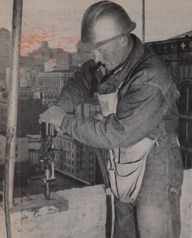
Nelson MG threaded studs are here end welded to steel inserts cast in the concrete. Using a battery unit for power gave operators maximum freedom of movement. Template was used to locate studs first.
