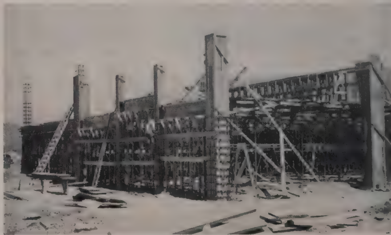
TWO-TYPE SHORING is shown in this general view, with the 13-ft. pipeframe topped with the wooden supporting system for the concrete girders. Concrete pouring will be in 40-ft. sections to provide contraction joints at that spacing.
