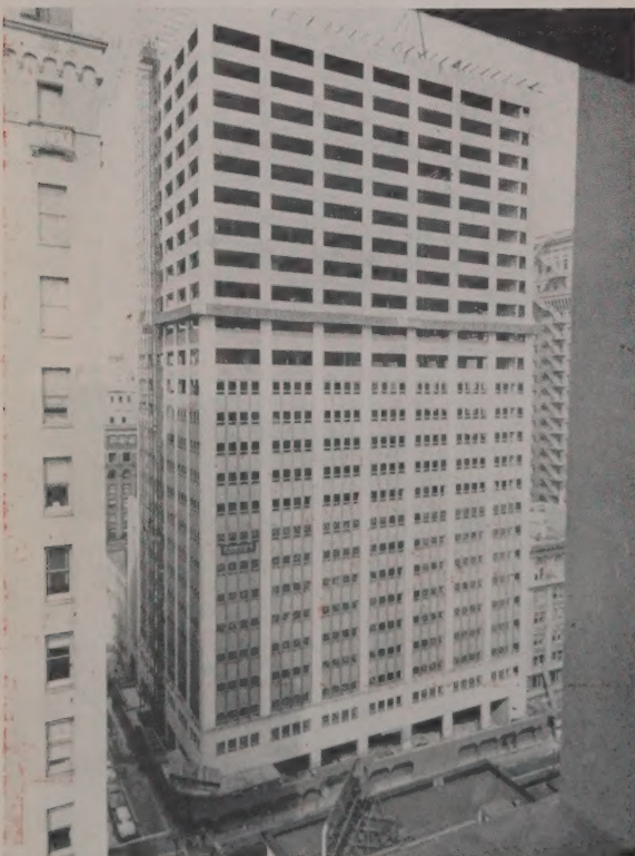
Two sides of the Equitable Life Assurance Building had the aluminum preassembled window wall panel installed, and to lesser extent on another side. A total of 23 floors was involved.
