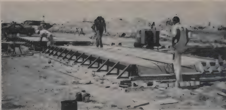
TWO CASTING PADS for the 100 precast roof slabs 28 ft. 8 in. long feature steel headers for accuracy of length, steam curing pipes on top and bottom and a compressed air system for blowing the slabs loose from its forms. Sequence calls for pouring at noon one day and removal the following morning.
