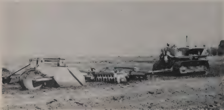
PROCESSING material on the fill includes disc and drag that leaves uniform moisture content and a fairly easy chore for the blade operator. Most of the time, compactors can follow up directly.
