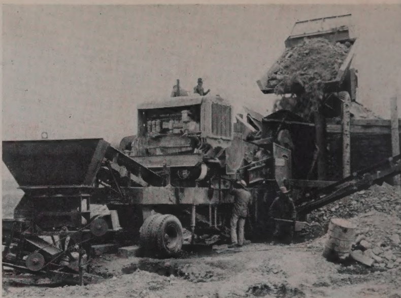
PRIMARY UNIT to cope with unfavorable pit conditions consisted of a 20 x 36 jaw crusher and a 4 x 6-ft. two-deck Pioneer vibrating screen. If necessary this screen can reject objectionable fines.
