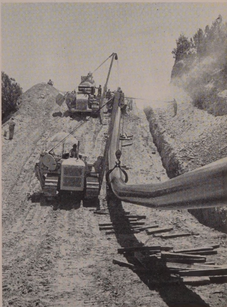
DOWN THE HILL comes the doping operation, the pipe receiving a 3/32-in. protective layer of dope, fiberglass, and paper. Blocking is replaced under the pipe after machine passes.
