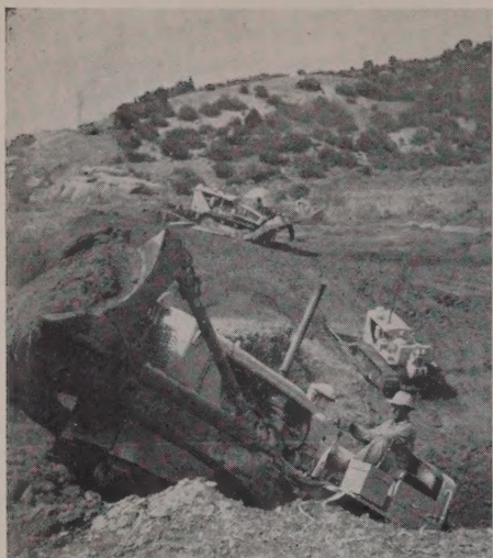
LEVELING the way goes a pioneer team of Cat D8's, some equipped with rippers.
