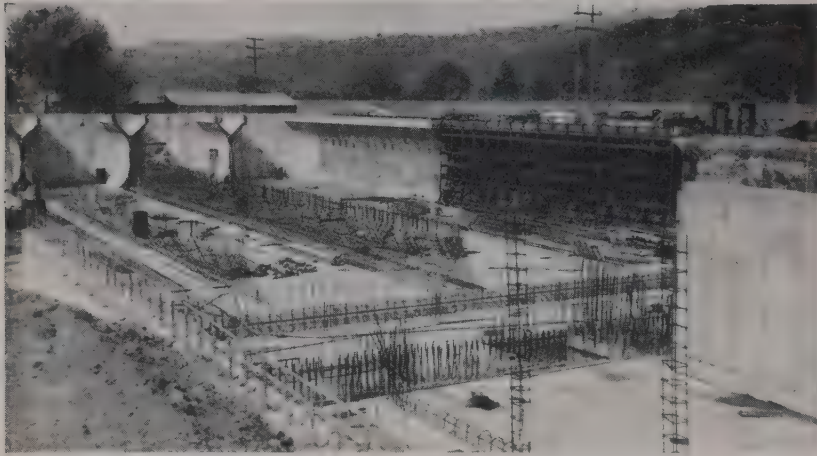
MECHANIZED FORMING with new "Y" wall trusses and UNI-FORM Panels speeds construction, saves labor and material
