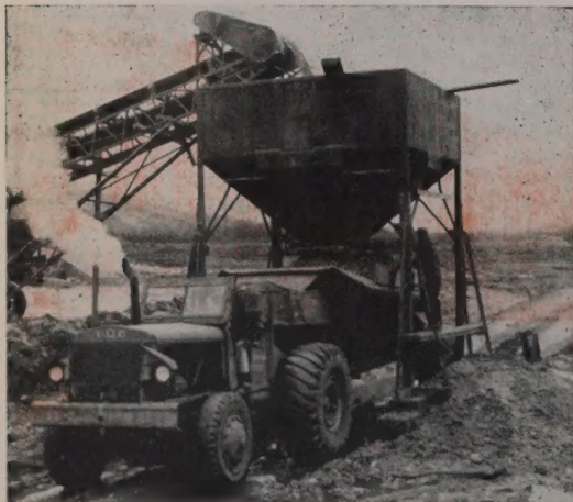
SURGE BIN of 45-yd. capacity loaded the Eucs as the plant turned out its 200 tons per hr.
