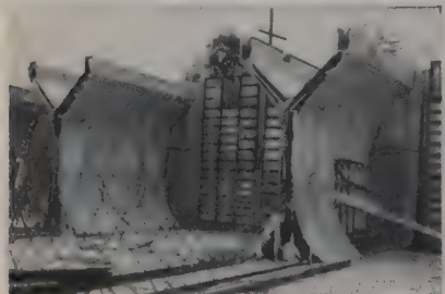
ASSEMBLED SECTION of "Y" wall truss with UNI-FORM Panels
