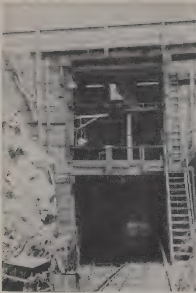
PORTAL is framed to carry project road overhead. At left is simple retaining wall, while crib at right holds 200 yd. of drain rock for easy chuting to mine cars below.
