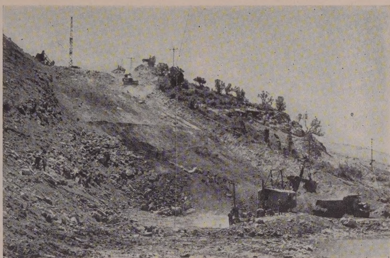
LOOSE SANDSTONE and dirt is dozed down the 42 % spillway slope by a Cat D8. At the bottom a Northwest 80D loads it into Eucs for placement as the zone 3 toe rock of the dam.
