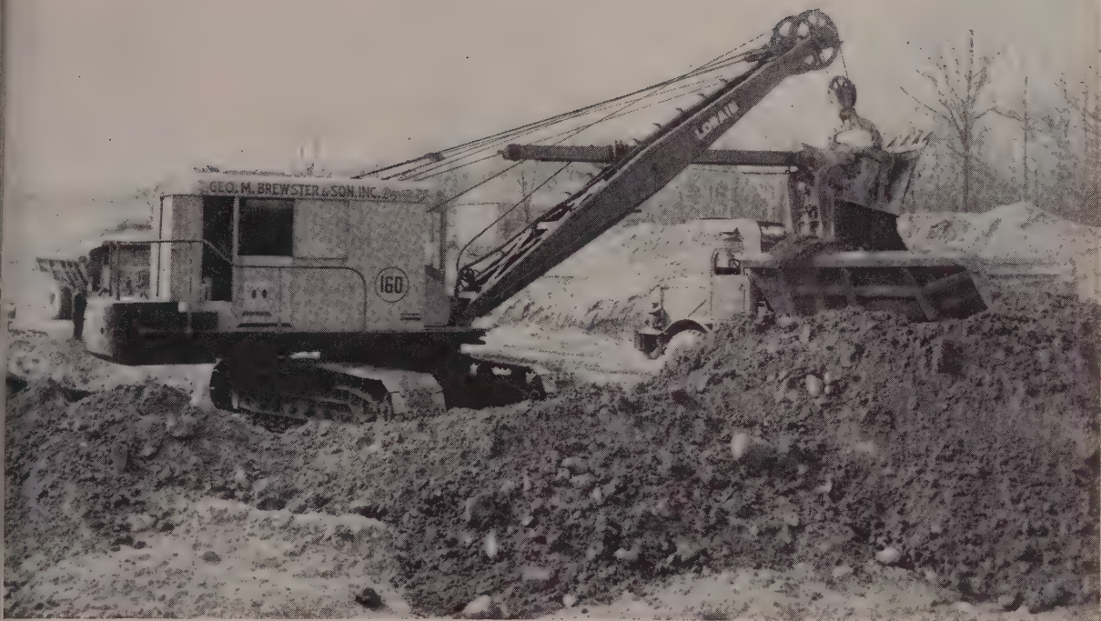
Owned by George M. Brewster and Son, Inc.—this new Lorain 85, with a 2½-yd. dipper and a 26-ft. boom, is working on the New York Thruway, where contract called for 2½-million yards of grading on a 4.7 mile stretch near Nyack.
