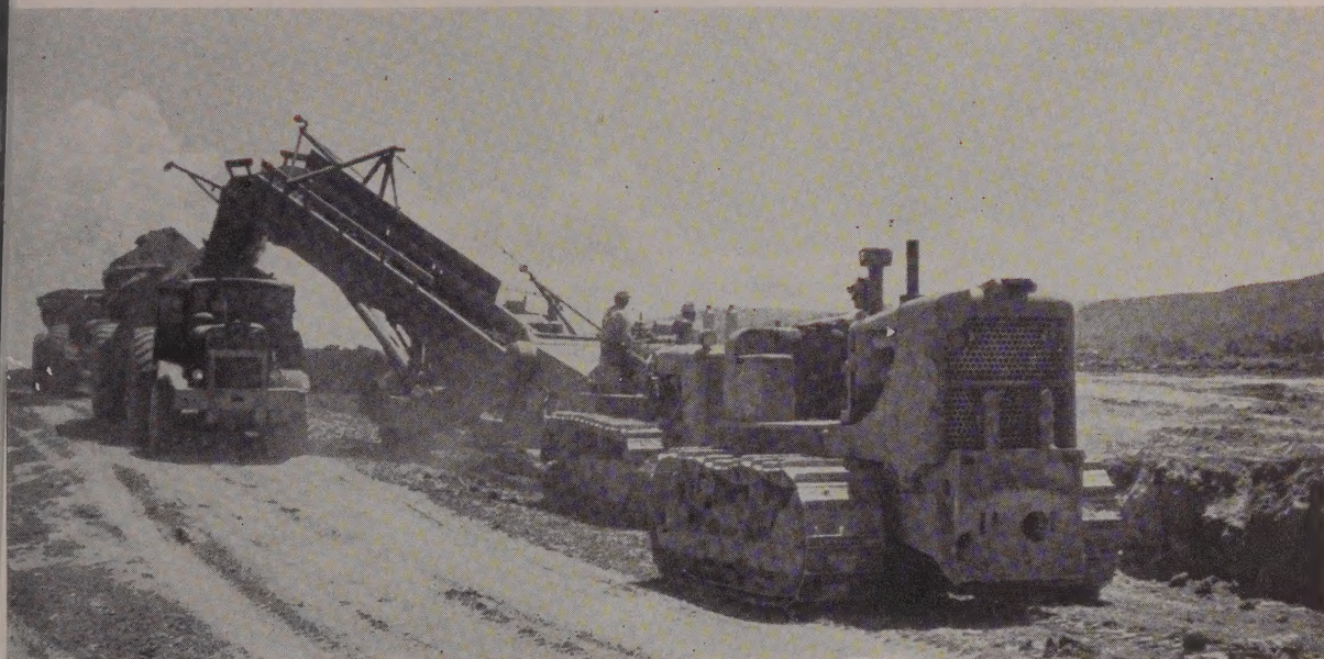
IT'S A BIG equipment operation in the impervious zone 1 borrow pit of heavy clay. Here a Euclid sidecutter elevating loader is being pulled
