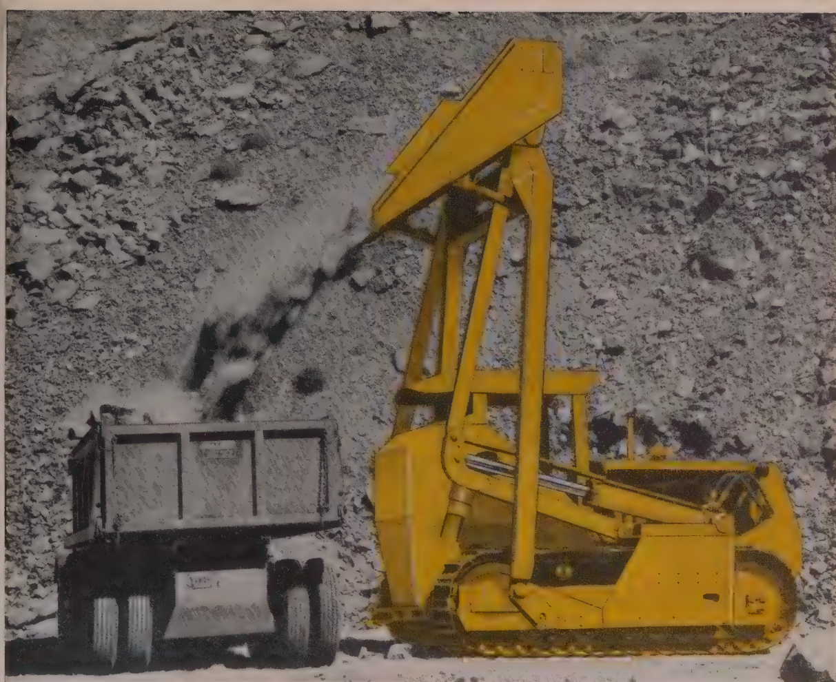
Model 8-C Austin Overshot Loader loading rock in Colorado quarry.
