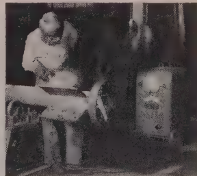
Welding wing plate to solid round tower leg with Lincoln Jetweld and Lincoln AC welders.
