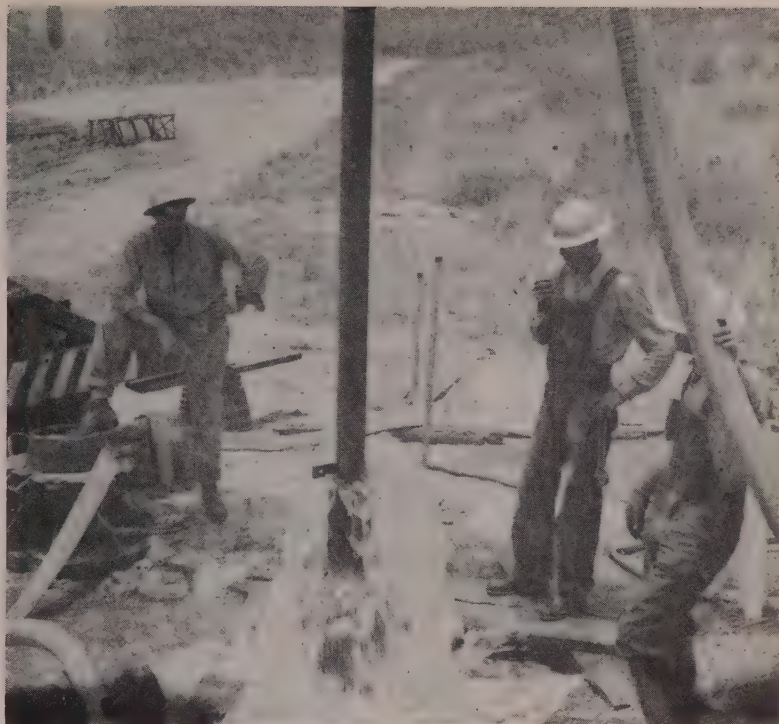
WATER DOES THE WORK , while Raymond crew under drill foreman Emil Geist takes a break. A 25-ton Bay City handled the leads and the pipe. River water was pumped at 500 gpm.
