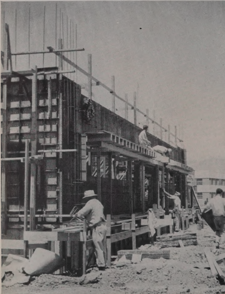
BLOCKOUTS for windows, doors, canopies are no problem to construct with basic panel sizes. Filler panels can be easily made to fill in gaps and connected to the others.
