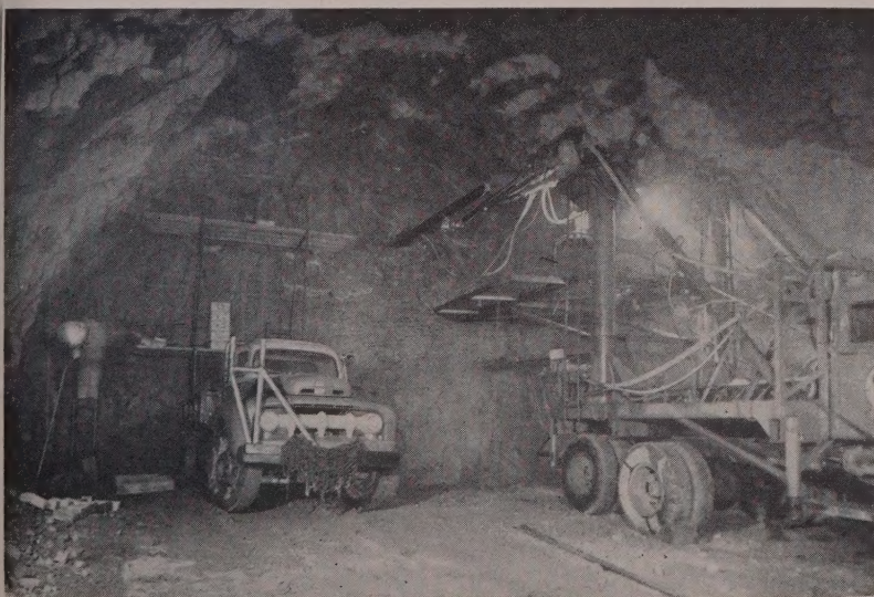
HERE IS ONE of the large drill jumbos and a loading platform used by Gibson & Roberts working in a heading of the Heart of the Hills tunnel, Olympic National Park, Wash.
