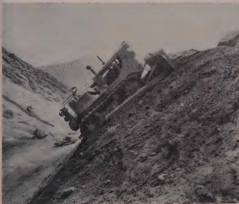
TRIMMING THE SLOPE AT SANTA FELICIA DAM
