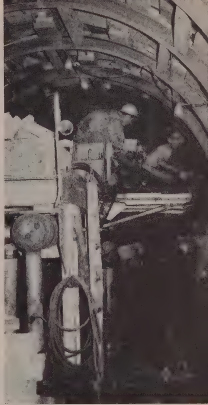
FULL SUPPORT frames crew in soft shale. The ground is strongly deformed, with thin beds of siltstone, limestone, and sandstone.
