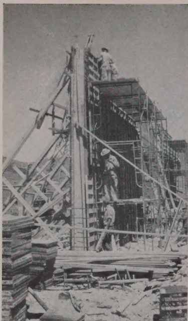
23-FT. HIGH wing walls are formed using Universal Uni-Form panel sections and pipe-frame scaffolding for fast erection.
