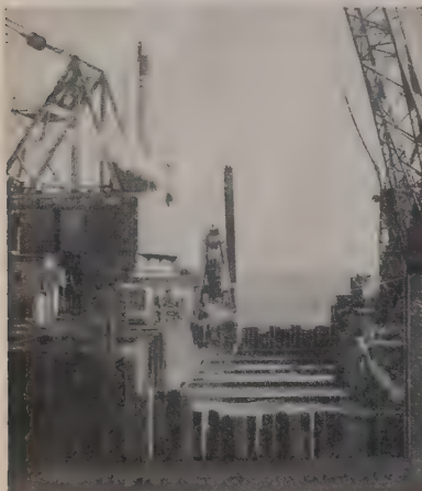
Foster Rental Piling forms cofferdams used in construction of the piers for the MULICA RIVER BRIDGE Garden State Parkway
