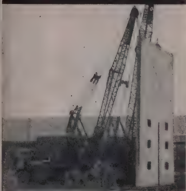
114,000 LB. SLAB being positioned
