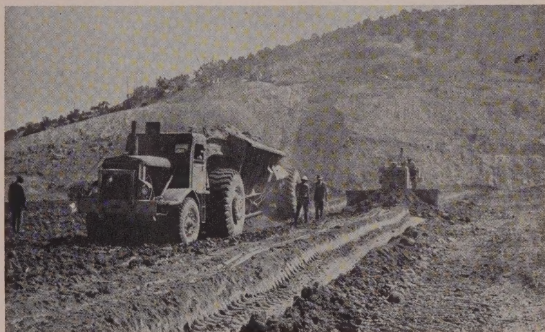
EVEN SPACING of windrows, spread by the bottom-dumps across the full length of the dam, gives a consistent 6-in. layer when spread out by the dozer. Going is boggy at 17 % moisture.
