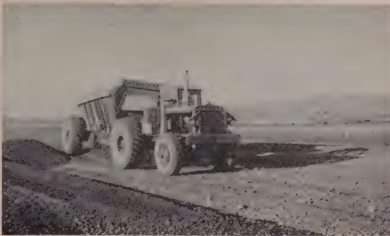
SPREADING on the run was done with the large bottom-dump units, while the smaller trucks were spotted and end-dumped. Lift thickness was 6 in. for select base being placed here.
