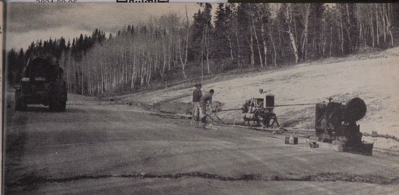
HALTING A LANDSLIDE which caused the pavement upheaval in the foreground was accomplished on the south approach road in Yellow-
