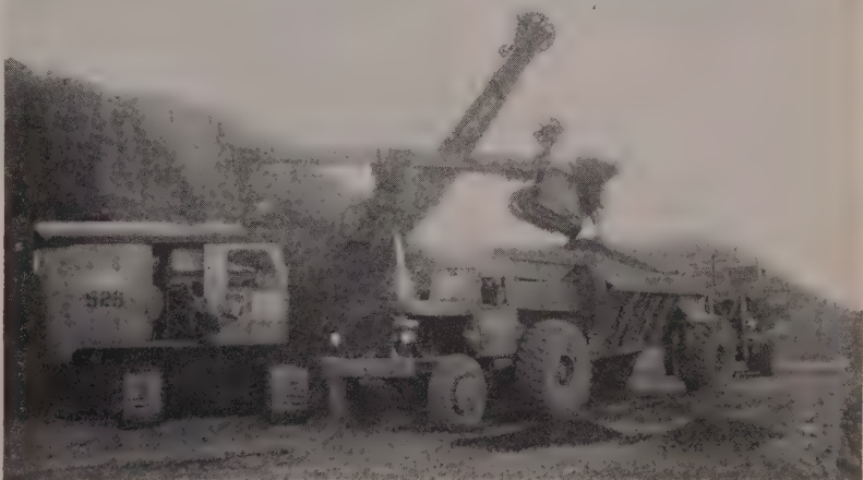
LOADING select base material at Isbell Construction Co.'s pit was done with a Northwest shovel with 2½-yd. dipper. Hauling units were all Euclid and varied in capacity from 20 to 50 tons.
