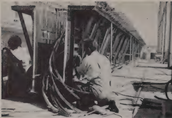
ECONOMY STEEL FORMS are used to good advantage in forming the intricate girder section and will be reused about 90 times.
