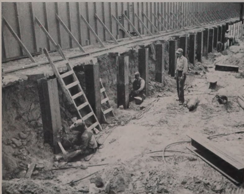
SOLDIER BEAMS, supplied by the L. B. Foster Co., were driven at 6-ft. intervals around the perimeter of the job site and will be left permanently. Penetration was about 50 ft. A crew follows up installing breast boards which will serve as the exterior foundation wall forms.
