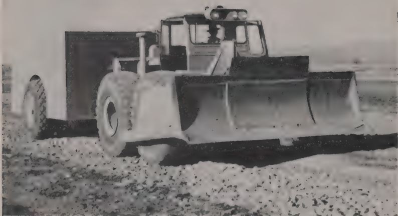
FINAL COMPACTION was given with this 50-ton Southwest pneumatic roller pulled by a Tournatractor. For 100 % modified AASHO density, four passes were usually enough.
