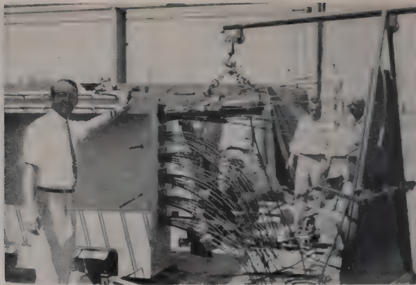
FREYSSINET SYSTEM of prestressing is used. New features on this job include twelve 7-wire strands per unit and steel female cones.
