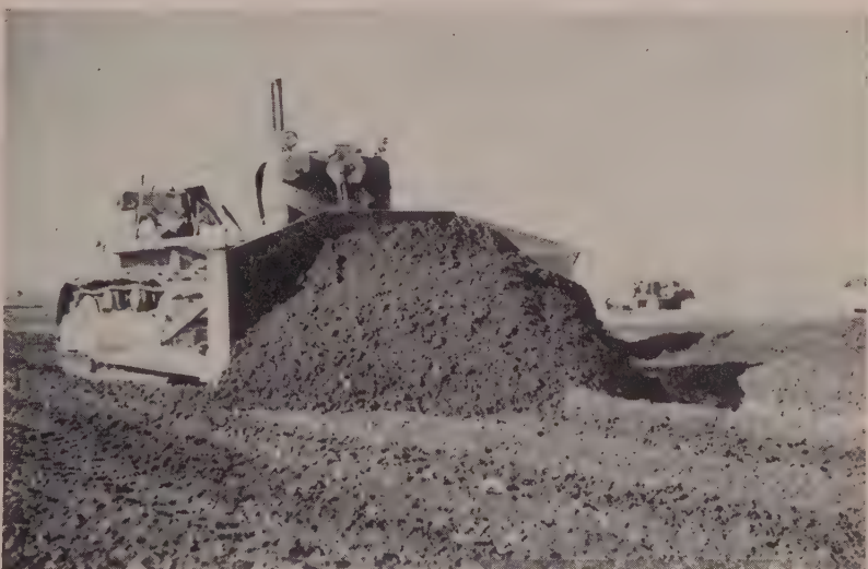
LEVELING out the windrows and spotted loads was done by this Cat D8 equipped with U-dozer. In background is maintenance truck that kept downtime of equipment to a minimum.
