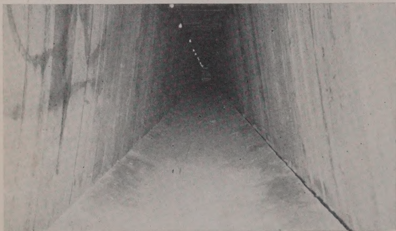
DRIVING PILOT tunnel first was secret to the success of the operation. It was followed up with a concrete paved invert that served as an accurate, greased skid for the pipe to slide on.
