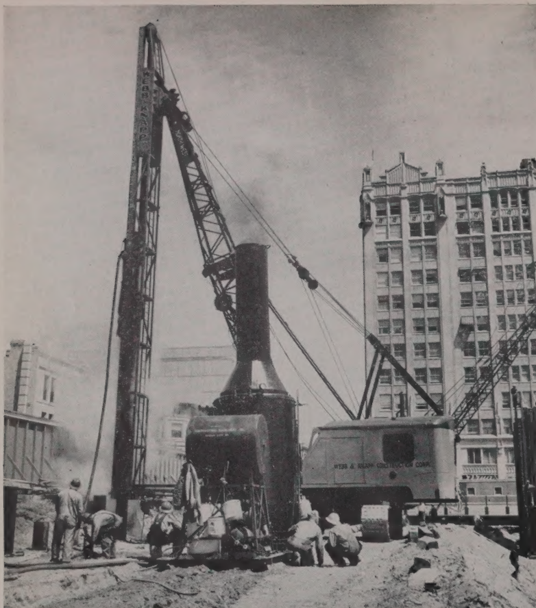
PILEDIVING was done by this Northwest 80D with 50-ft. boom and 60-ft. leads. McKiernan-Terry 11B3 hammer developed 19,200-ft. lb. blow. Steam was supplied by skid-mounted 90-hp. oil-fired Hamburg boiler.
