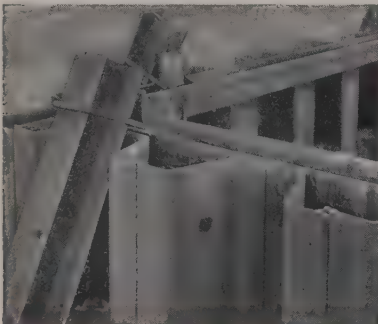
Foster Piling waled and braced with H-Bearing Pile for the foundation of the GEORGE HUBBARD CLAPP SCIENCE HALL UNIVERSITY OF PITTSBURGH
