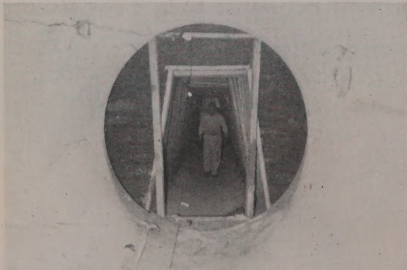
EXTENT OF the material to be removed between the pilot tunnel and the pipe can be seen here. At this stage, 160 ft. of culvert had been shoved forward and operations would now move to far heading.
