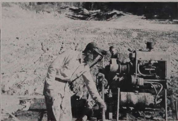
JOY 12-B core drill has 4-cylinder Waukesha engine and drill head that rotates 360 deg. It is also used for other foundation work.
