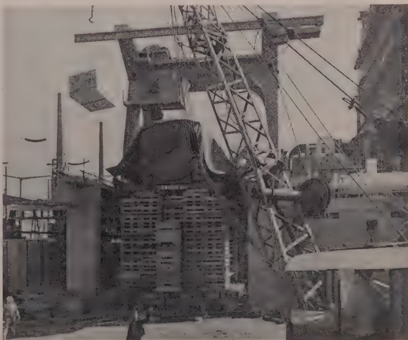
THE GENERATOR is being jacked into place. This was done with the use of special hydraulic jacks of 50-ton capacity each which lifted the stator 6 in. at a step.
