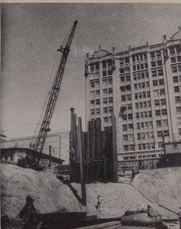
ESTABLISHING a sump, steel sheet piles are set around a pipe-frame "bandstand" with aid of Bucyrus-Erie 38B with 70-ft. boom and jib.
