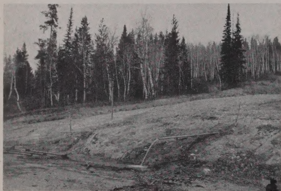
FLOW OF 22,000 gpd. came from one of four drain pipes, each about 200 ft. long, driven into the slide area.
