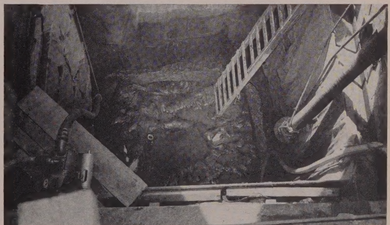
DRAINAGE SUMP bottomed out in shale formation has burlap strips hung to keep seepage off the footing while load tests are conducted. Footing is also covered with canvas in the view. Pump at lower left is a 3-in. Homelite.
