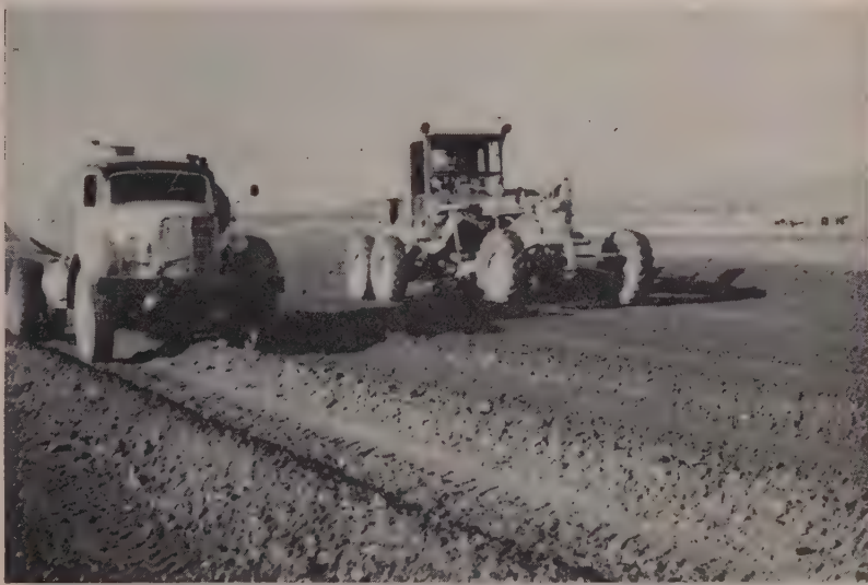
WATERING to get optimum moisture content and then blading with a Cat 12 to get uniform distribution of the moisture was necessary in the arid climate. Total depth of base was 28 in.
