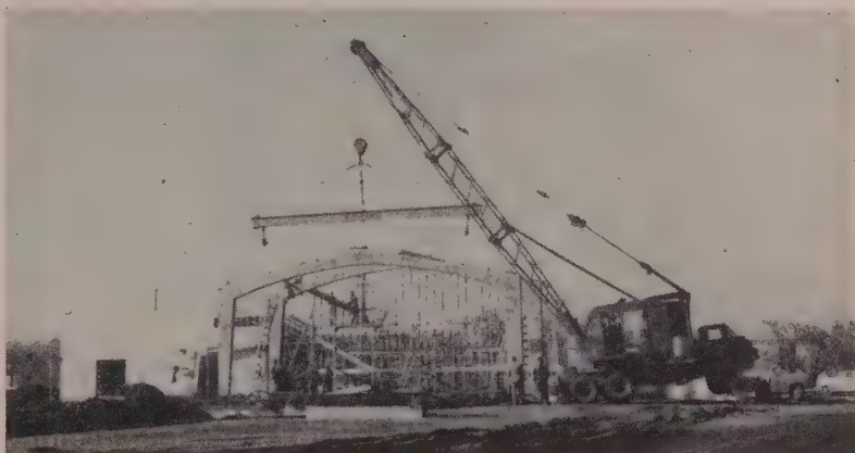
LINK BELT CRANE with 55-ft. boom had a long reach from paved road to place the frames. Recent rains made the center area of the structure muddy and unstable for lifting the 10-ton weights involved.
