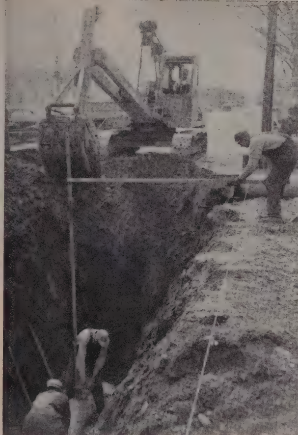
HILTON & CARR Construction Co. used a \frac{1}{2} -yd. Unit backhoe with sufficient room in the street to dump material. Grade for concrete sewer pipe set by ordinary grade rod. Pumps were required to keep bottom of trench dry with gravel backfill placed for pipe bedding.
