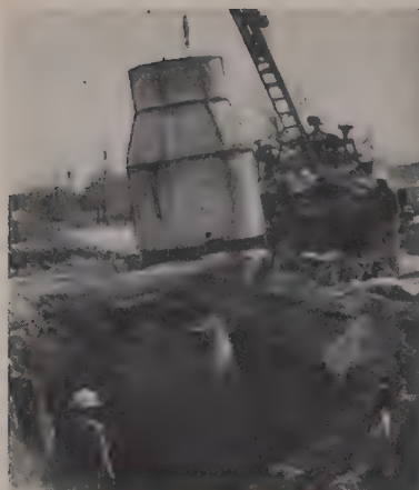
MOST MANHOLES were constructed using metal forms inside and outside. Ease of stripping entire outside form is evidenced here.
