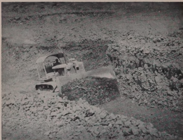
WESTERN CRUSHING is a rugged industry. Here is a Cat D8 with U-dozer working a quarry near Coulee City, Wash. This is typical of the shot rock pits in central Washington.
