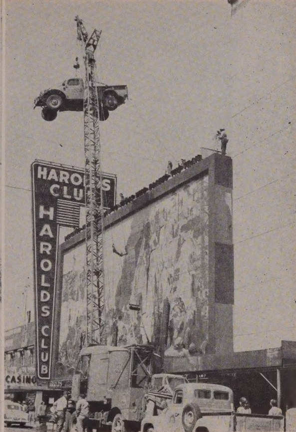
SECOND STEP required this Link Belt truck crane with 60-ft. boom to then pick it up and further lower it to street level.
