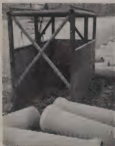
THIS PIPEFRAME box with heavy sheet metal sides was used occasionally by Hilton & Carr to protect workmen while laying pipe in caving ground. Dimensions are about 3x8 ft. by 6 ft. tall.
