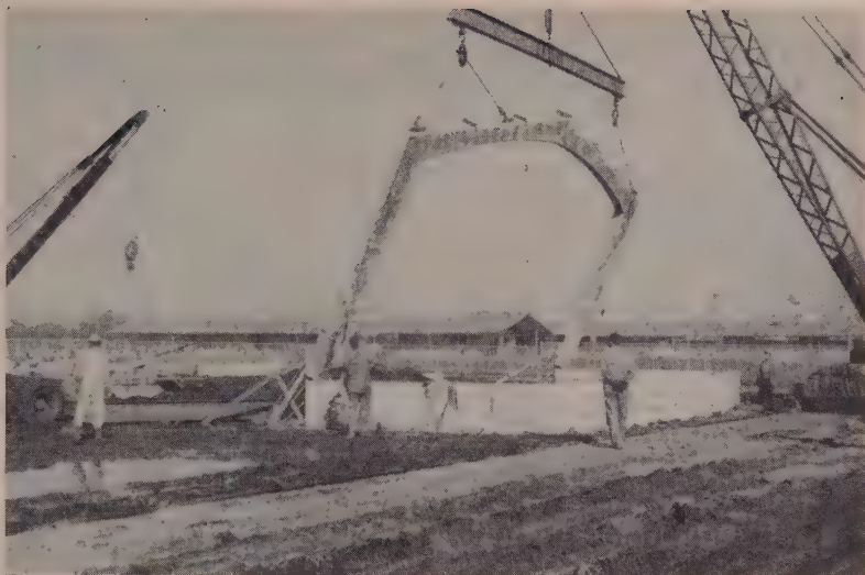
FIVE RIGID FRAMES, with a span of 44 ft. each, were cast one on top of the other using Techcote Antibond 200 applied between layers. Kickers against base of frames made pickup by crane foolproof.
