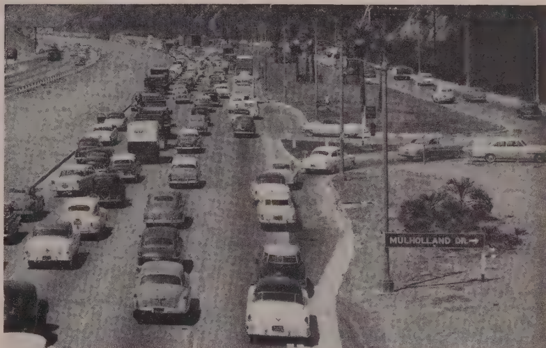
EARLY FREEWAY design for on and off ramps had lane at right for autos to use before making turn. Drivers didn't behave as figured and stayed in the main lane before turning with the result that rear-end collisions were frequent.
