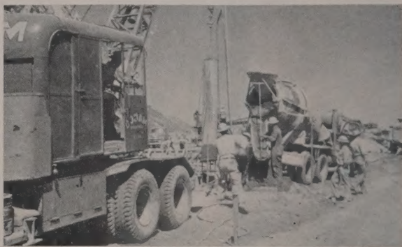
HIGH-STRENGTH tremie concrete was poured in each of the bell-bottomed holes with casing being pulled as concrete was brought up.
