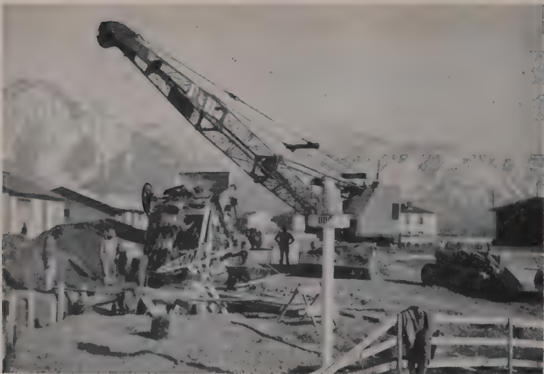
MGR CONSTRUCTION CO. made good time with cuts to 20 ft. with this Parsons 310 trencher where ground conditions allowed. P&H truck crane handled pipe sections, and Allis-Chalmers HD-5 placed gravel pipe bedding.
