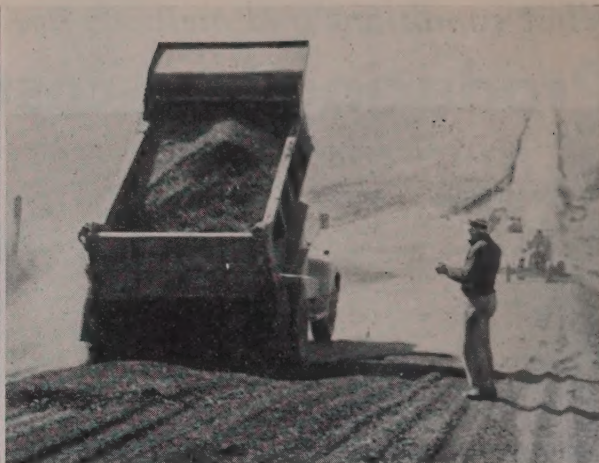
FEW FINES were required for the 1-in. minus crusher-run rock being placed upon this Douglas County haul road. Binder material came from the roadside. Road will not be surfaced in foreseeable future.
