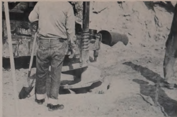
AUGER DRILLED 3-ft. diameter holes at 20 ft. per day rate. The rig, largest in the West, is capable of drilling 8-ft. diameter holes.
