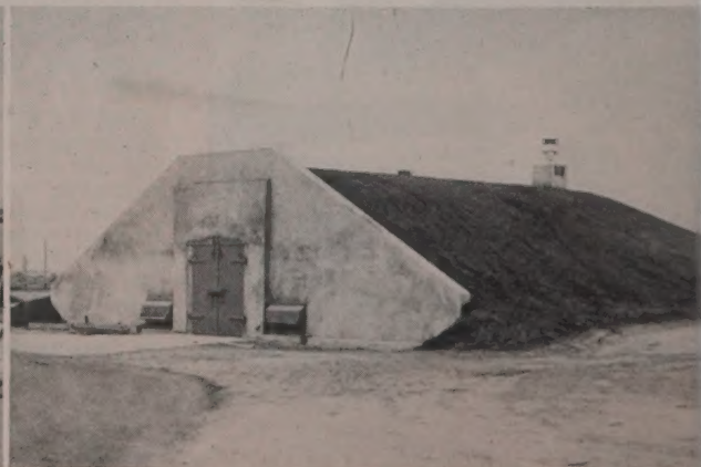
COMPLETED STRUCTURE has 4-ft. thick dirt fill over the crown section tapering off on three sides on a 2:1 slope.
