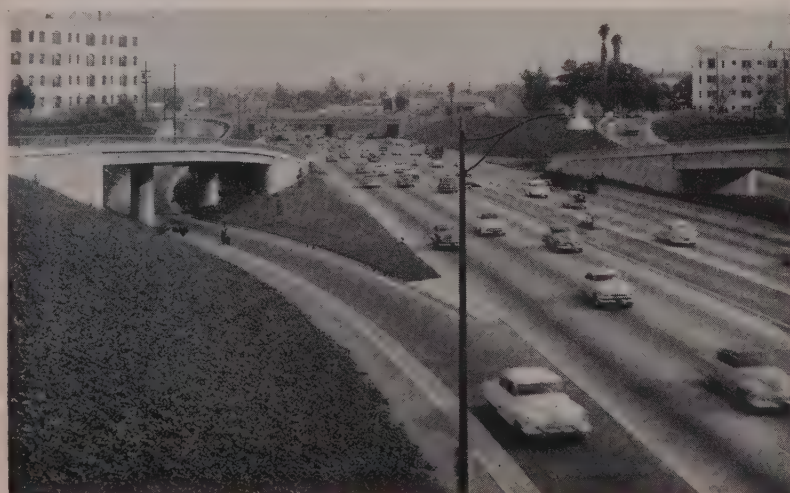
MODERN FREEWAY has full speed take-offs and merging lanes that have successfully done away with the rear-end collision type of accident. More time has been spent in developing freeway connection designs than all other design features combined.
