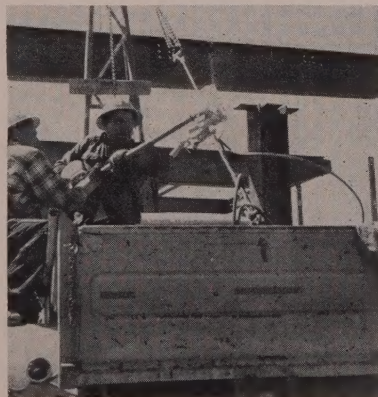
TIRFOR GRIPHOIST jacks ordinary wire rope in either direction and came in handy for booming the A-frame up and down for setting steel in cramped quarters.
