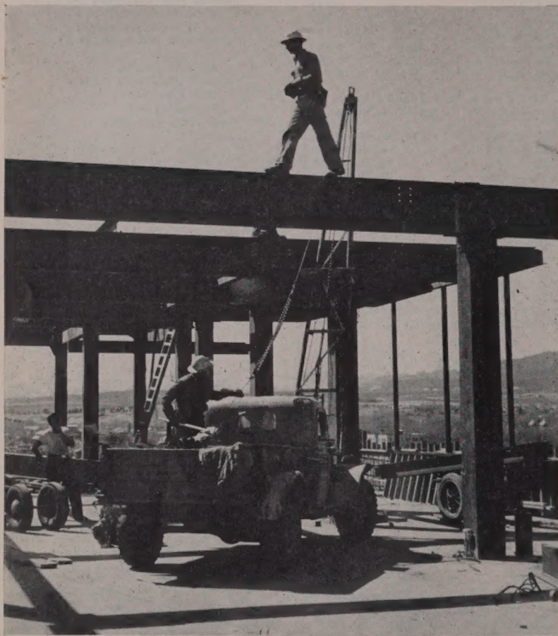
ERECTING HEAVY structural steel on the 7th floor was handled by this Dodge powerwagon having a 20-ft. A-frame on front and a Tirfor Griphoist to allow booming up and down. Beginning with the 4th floor erection, the truck was raised from floor to floor through the elevator shaft.
