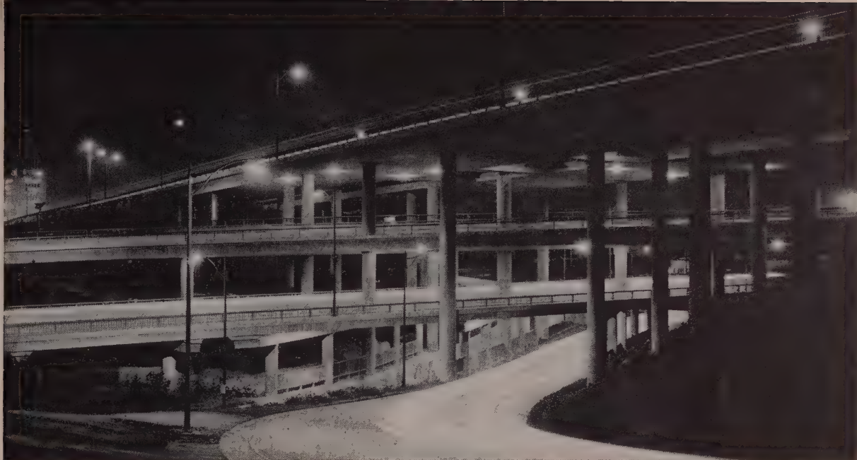
COMPLEX TO LOOK AT, BUT SIMPLE TO DRIVE: Four traffic levels in a single bridge structure makes a lot of sense to Los Angeles motorists. It enables the traffic of two crossing Freeways to interchange with a simple turn in the desired direction and provides a right-hand take-off and junction, and minimum travel distance, at all times. California Division of Highways Official Photos.
