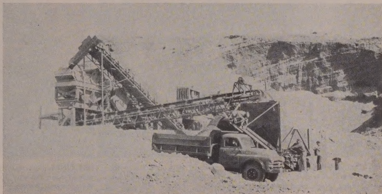
ROAD CONSTRUCTION in isolated areas calls for portable plants such as contractor Frank Baulne's outfit producing 2,200 tons per shift in the Moses Coulee area of Douglas County. Another important factor for low-cost aggregates is awarding stockpile contracts in off-season.
