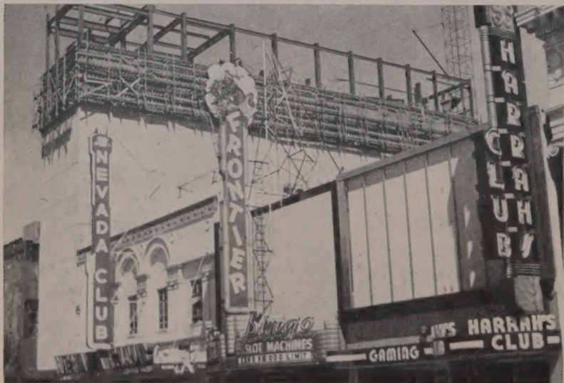
IN RENO, NEVADA, where everything is unusual, this building expansion by Harolds Club fitted in with the spirit by having steel erected and concrete poured floor at a time.
