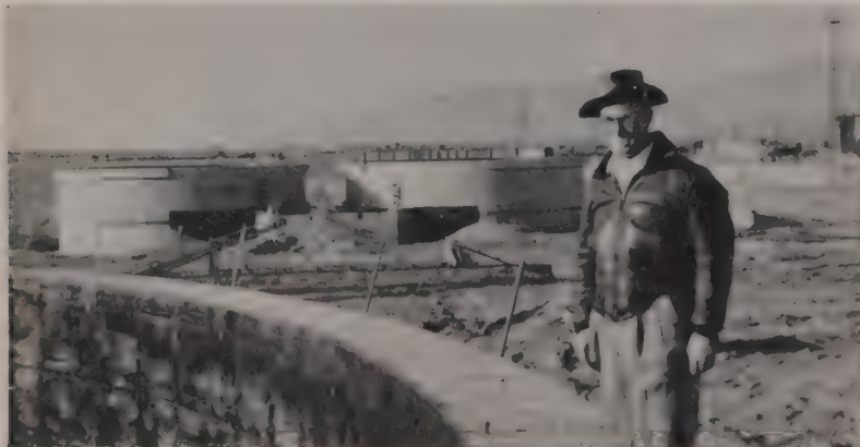
"CHUCK" KELLEY is resident engineer for this $8,000,000 project. In the background are digester tanks built for cold weather conditions at the treatment plant being constructed by Tolboe & Harlin. Walls of tanks will have insulating mats attached to them and then have dirt backfill to the top.
