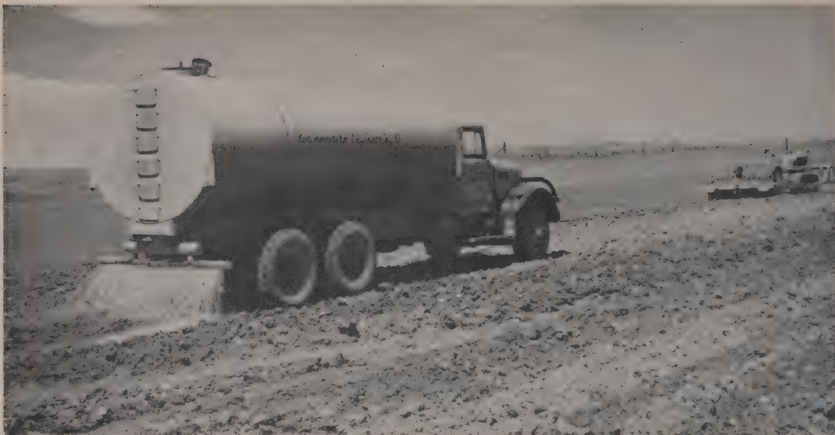
MOISTURE CONTROL on heavy clay soil—typical throughout the project—was a key factor. Typical A-7-6 soil (Highway Research Board
