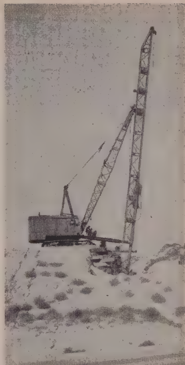
ABUTMENT PILES up to 94 ft. long were driven from top of approach fill built the previous year to allow for predicted settlement.
