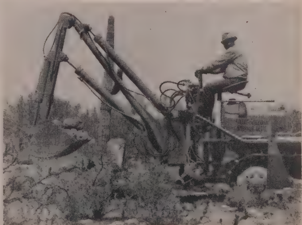
FOR EXPLORING sand and gravel deposits, and for deep digging on pavement patching, Arizona Highway Department uses a Hopto backhoe on a D4. Machine like this encourages getting clear to the bottom of weakened base, and then some, for replacement with greater thickness of 1955-specification base material.
