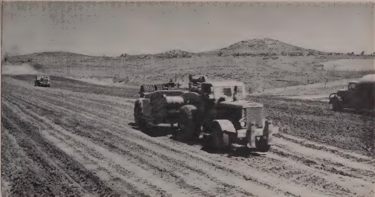
ROUTING EQUIPMENT over the full width of the embankment as loads are spread is an important factor in getting the most economical re-
