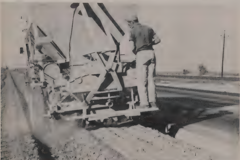
METERING cement into notched windrow can be tricky. Some trucks plow their own notch. Problem is maintaining even rate of flow despite level of cement in truck bin.
