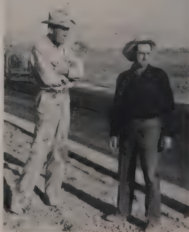
WORKING as a team, resident engineer John Smith (left) and Joe Knight figured they had a job to do instead of a battle to fight.
