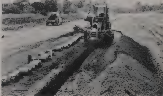
↑ Herkner Construction Co.'s CLEVELAND cuts underdrain trench adjacent to a catch basin at Route 21—Turnpike Interchange.
