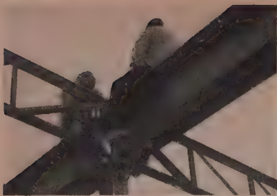
Fig. 1. Tacking roof joints in position on 440' x 440' all welded frame work.
