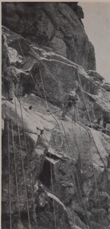
DIFFICULT-TO-GET-AT places on snow-covered rocks were a jackhammer drill specialty. At such places, special 2-ft. long sticks of DuPont dynamite cut loading time by a third.
