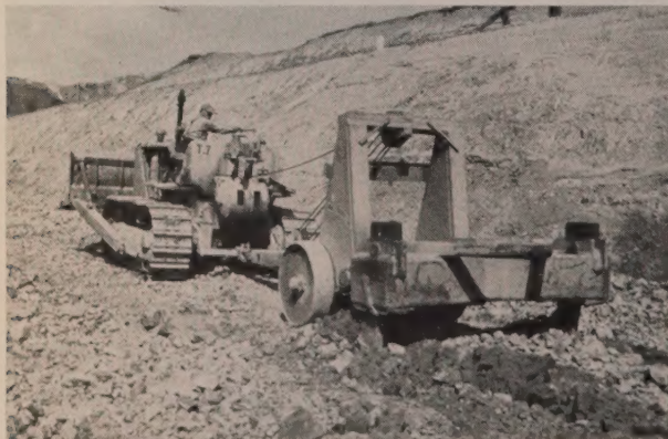
HARD SANDSTONE gives up under attack of LeTourneau ripper pulled by Cat D8. Several passes were required for rock breakup.
