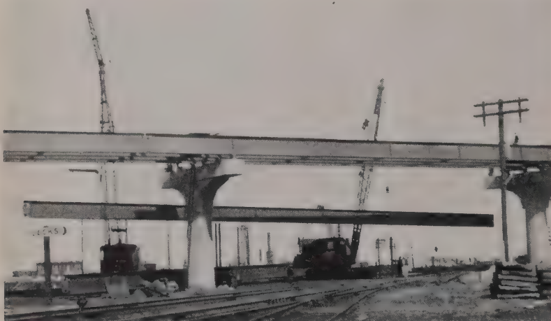
STEEL GIRDERS 4 ft. deep and up to 125 ft. long were walked into position over the railroad tracks by two cranes. Tight schedule was necessary on erection because of passing trains.
