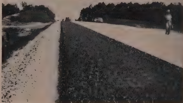
Completed Penetration Macadam before Surface Treatment.
