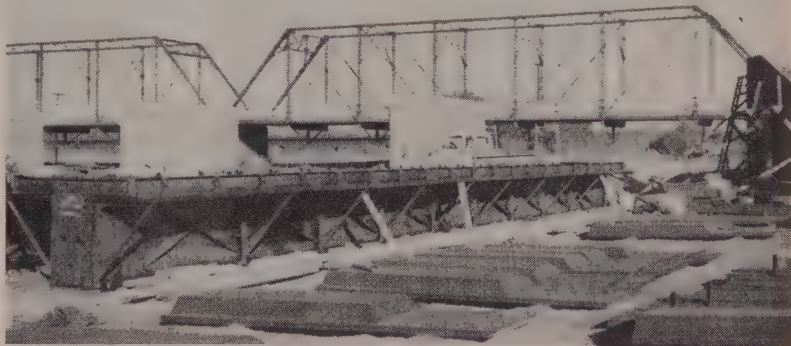
"... forms must be able to withstand multiple uses and be easily erected, stripped, and cleaned. They must be light enough for handling, and strong enough to withstand stress . . ."
