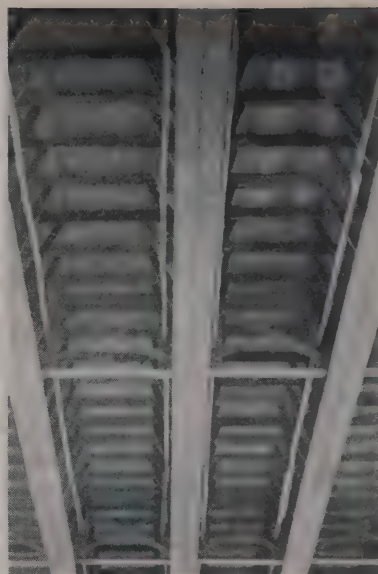
ERECTION and stripping of deck forms was done without scaffolding. Four-foot depth of girders allowed room for workmen and kickers.
