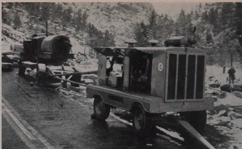
GARDNER-DENVER was the compressor and drilling show here. An older, reliable 900-cfm. unit is mounted on a lowboy and joined with a new 6-cfm. unit. Air pipe leads off to the right where more Gardner-Denver jackhammers were used in drilling large boulders lying in the future roadbed.
