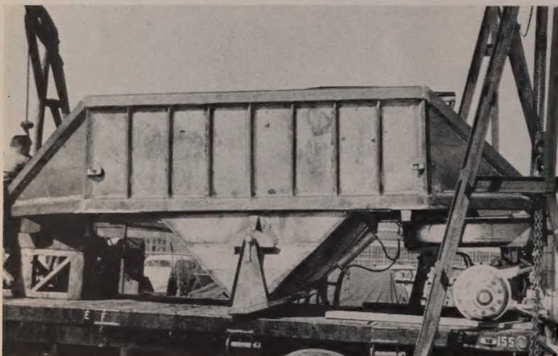
SPECIAL BODIES of Cor-Ten make for light weight, permit big payload within legal limits. They'll be pulled singly for short hauls on soft grade early in season, then in doubles later on when grade is firm and haul longer.
