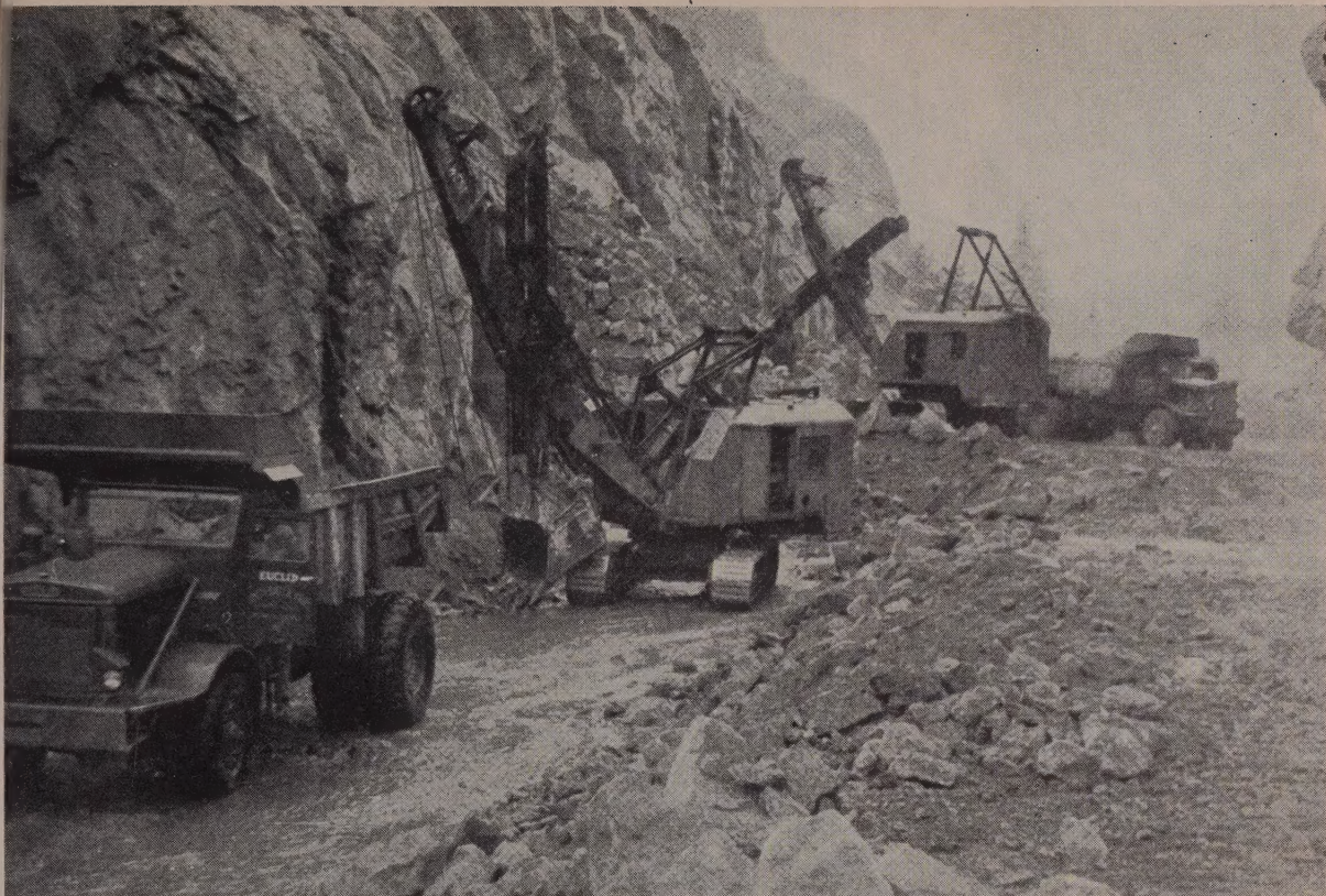
SHOVELING FROM THE STREAM BED, these two Northwest shovels are handling some tough rose granite. Rugged Euclids haul the rock up and downstream to fill in areas (on the right) for the new road location.
