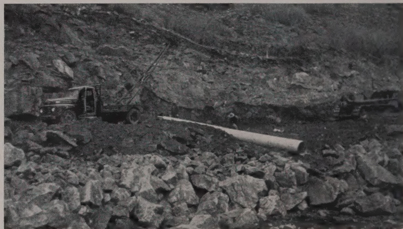
CULVERT PLACEMENT occurred an average of every 300 ft. on the 4-mi. long job and had to be closely scheduled with filling operations. Cat D8 bulldozed trench for culvert. Culvert lengths of about 20 ft. were then picked up, delivered, and lowered into trench by use of A-frame on truck.
