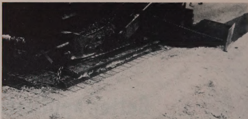
HOT-MIX PAVER passes over welded wire fabric in test resurfacing of U.S. 40 near Vallejo. Steel rail suspended from front of paver irons out fabric for laydown. Attachment at right rear of machine catches spill-over hot mix and distributes it as edging.
