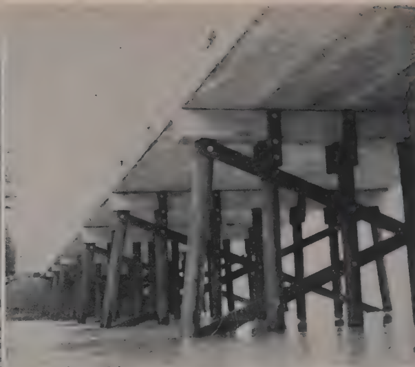
TREATED TIMBER piles, concrete caps, and prestressed slab units make up the bridge which has seven 30-ft. spans and one 45-ft. span. Six slab units make up full bridge width.
