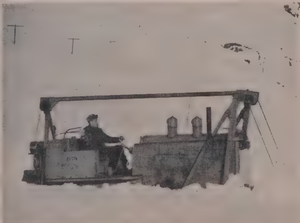
WINTER OR SUMMER, if the maintenance forces can't buy it, they rig it up themselves. For plowing snow on the Richardson Highway, the Alaska Road Commission enclosed the engine and air-intake breathers on this HD-19. Machine works on warmer air now, and doesn't get stalled by snow clogging breathers.
