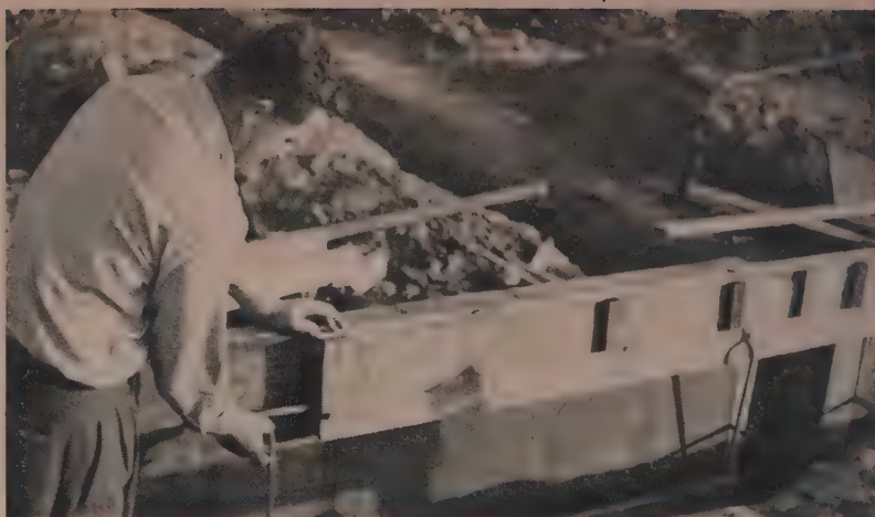
TWICE-BENT dowel slides into place in the blockout in this view showing inside of form. Notch on end of blockout permits snug fit for next section.
