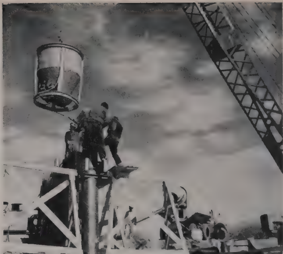
POURING CONCRETE in steel shell piles was easy with transit-mix trucks able to use access road for close approach to work.
