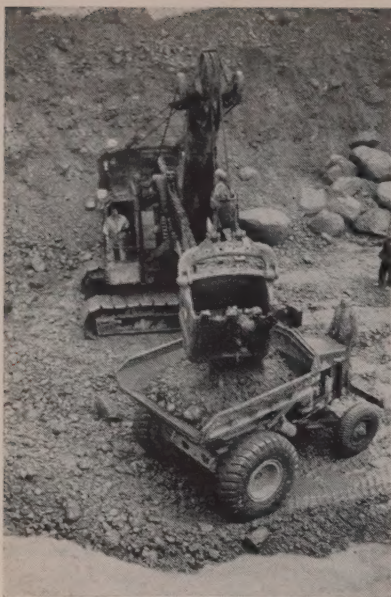
SLICK AND UNSTABLE material digs easily, will make good base after having "bath."
