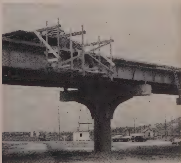
SCAFFOLD HANGING from truck and suitably counterbalanced made it easy to strip forms from the cantilever section of the deck.
