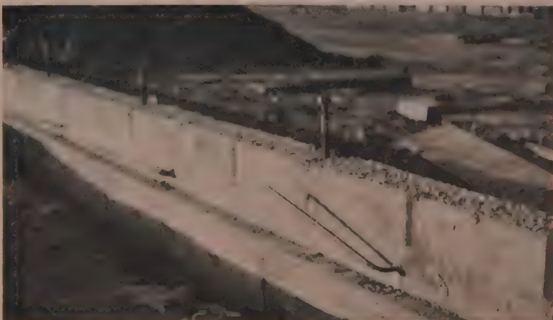
FORMS COME OFF by sliding them parallel to wall. The bars in this position do not interfere with backfilling or other operations. Before pouring slab the bars are straightened.
