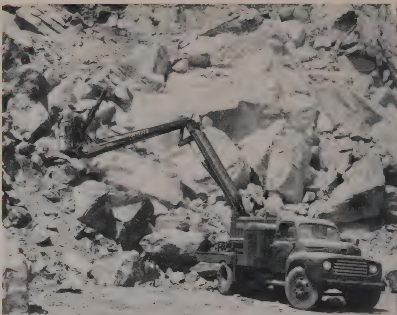
VERSATILE EQUIPMENT still gives good old contractor ingenuity a chance to pay off. Here's a serious secondary drilling problem, solved by shop building: a platform on the end of a Pitman Giraffe boom and mounting a Gardner-Denver wagon drill, for sinking holes from any angle. Giraffe's 38-ft. reach was the big boost.
