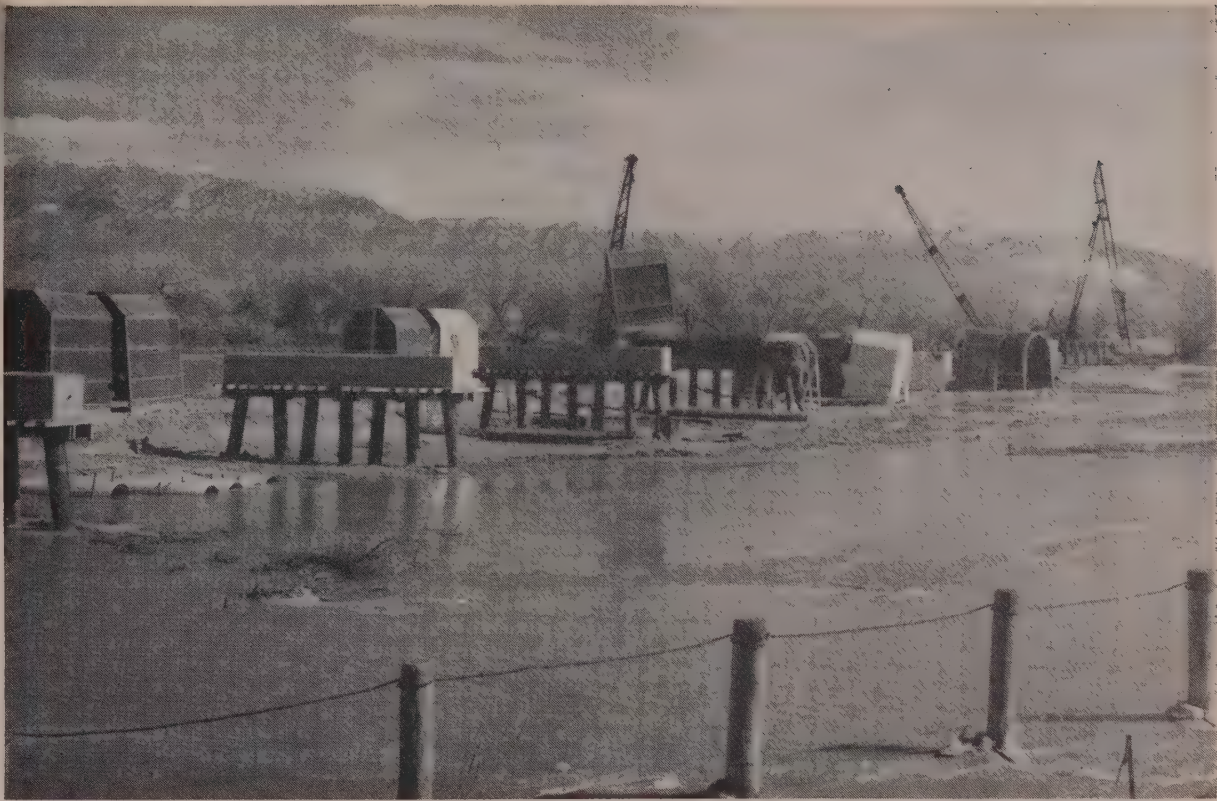
COLD ENOUGH for ice to form on the river, so wood frame and canvas igloos were necessary over freshly poured bents to allow heating.
