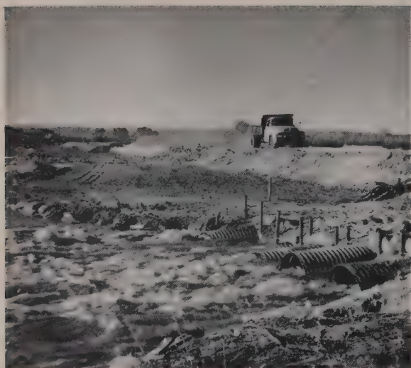
CORRUGATED METAL culverts placed under access embankment handled entire winter stream flow of the Rio Grande. View is looking west.
