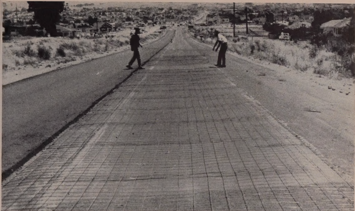
WORKERS PLACE sheets of welded wire fabric on two 600-ft. sections of the mile long project. Hog rings fasten longitudinal wire together to join individual sheets. Expanded metal mesh of various weights and
