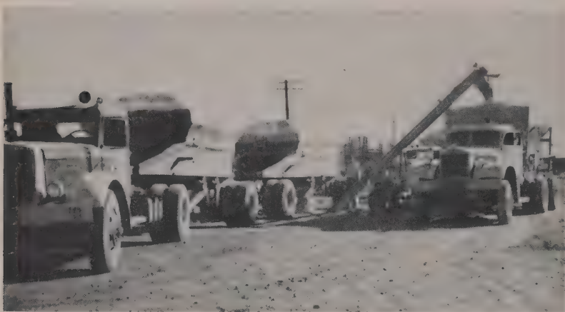
BULK CEMENT is cheaper, even with necessity for handling into smaller distributor trucks on job. Economical and effective materials handling is key to success with cement treating.
