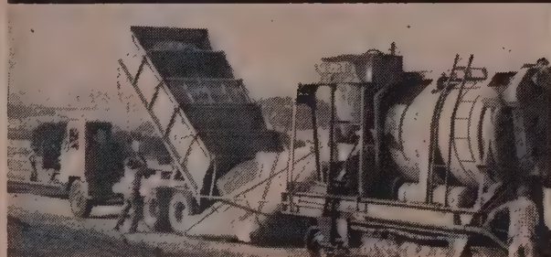
C-B "M-310" BATCH TRUCKS each carry five 1½ yard batches per load. This single passenger, cab-beside-engine truck with regular dump body has a 15 ton legal payload capacity in many states. Heavy duty front axle and shorter wheelbase permits easier handling and greater maneuverability on or off the highway.
