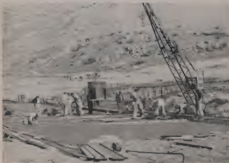
TWO CONCRETE POURS a week were easily handled with up to 125 cu. yd. per pour. Northwest crane with 80-ft. boom allowed swinging 1-yd. Insley bucket to all parts of 36-ft. wide deck.
