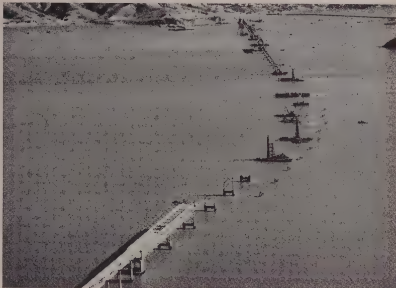
RICHMOND-SAN RAFAEL BRIDGE (4 mi. long) had low trusses in the foreground placed by floating in. Erection is underway in center section using aluminum falsework trusses. Cantilever span nearest the far shore is also underway using the balance method of erection.
