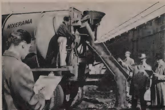
A HI-UP TRUCK MIXER manufactured at Worthington Corporation's Plainfield Works, being demonstrated at an actual job site. The Mixerama is part of the company's concentrated program of selling through on-the-job product demonstrations.
