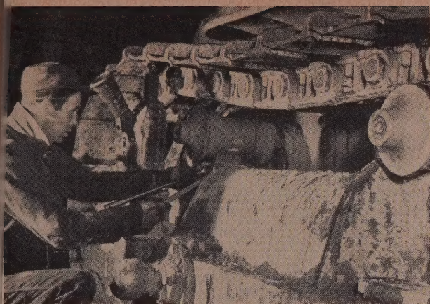
TRACK REPAIR: Art Debroux again, this time replacing a top carrier roller on an HD-20—one of 16 on the job.
