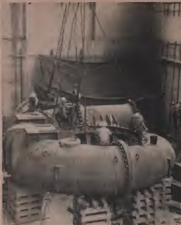
SCROLL CASE is just about ready for the big lift into position. At this early stage of installation, there was plenty of room to work.
