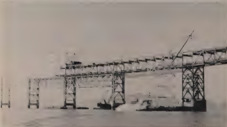
DOUBLE-BOOM TRAVELING DERRICK erects steel panel truss parts in continuing operation on top of the two aluminum trusses. Falswork trusses are leapfrogged ahead. Judy Ann is to the right placing secondary steel truss sections.
