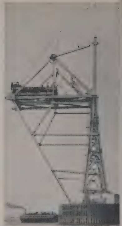
A 55-TON stiff-leg derrick has been placed on the anchor arm of the cantilever span and will be accompanied soon by another traveling derrick working in an opposite direction.
