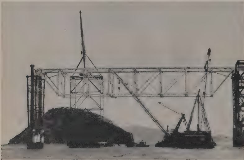
FIRST ALUMINUM FALSEWORK TRUSS going into position. Temporary timber bents setting on the piers support the truss. Total length of truss is 280 ft. and it weighs 120 tons.
