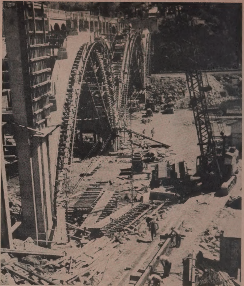
BOWSTRING TRUSSES , in which the upper curved chords were glued laminated timbers, were used by Charles MacClosky Co. on the Dunsmuir bridge in place of ordinary falsework. Clear spans of 102, 180, and 114 ft. were involved. Two trusses hinged at the top completed one span.
