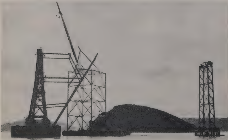
JUDY ANN AGAIN. Here the derrick barge places the inclined strut and tie-in pieces to tower No. 47. Relative size of tower can be seen by comparison to men standing on horizontal members. This view shows all the falsework indicated in the upper diagram.
