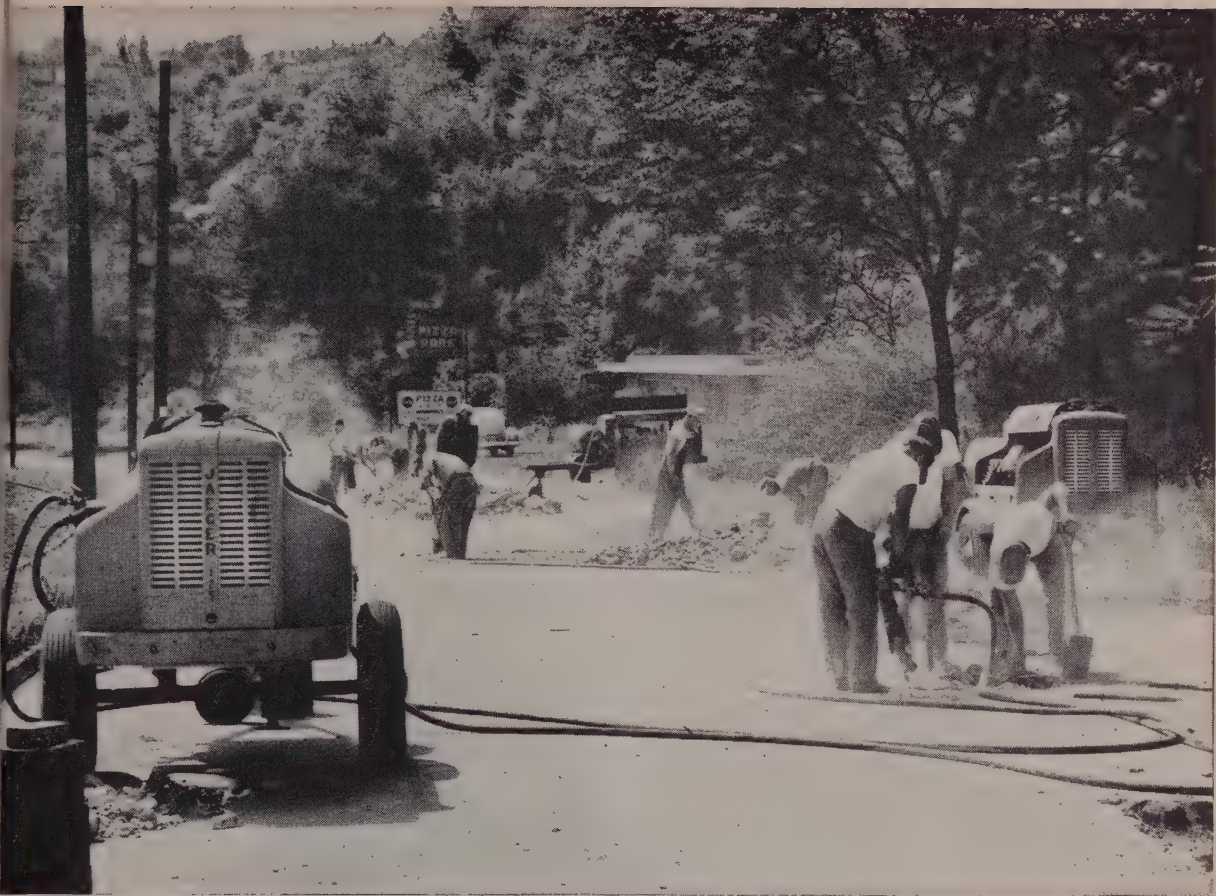
Three 4-man crews, each with a "125" compressor and two heavy breakers, formed fast-moving team.
