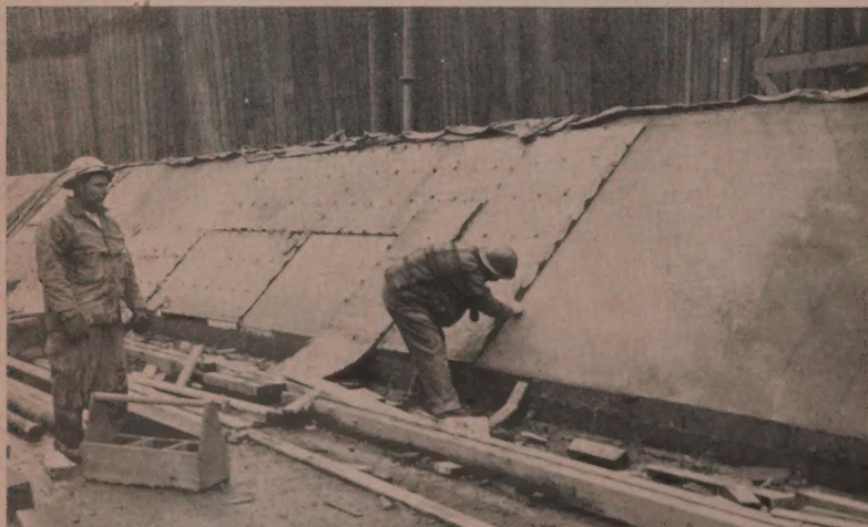
FANCY FORMWORK included absorbent liners to assure very dry concrete at surface of new end sill. Applications like this are laboratory for concrete durability.
