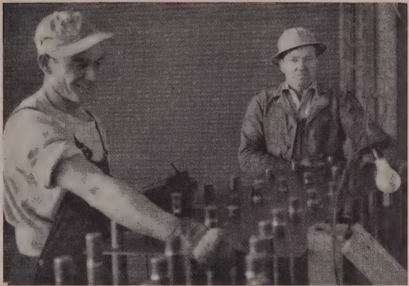
FIVE THOUSAND rotor punchings for each unit had to be cleaned and assembled. A steam cleaner, a roller conveyor, and an electric sander made it a production line job, and the millwrights had enough energy left to smile when doing the final hand stacking.
