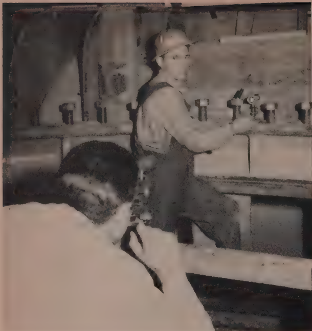
ILLUMINATED TARGET makes scroll case leveling easier. So does independently supported instrument at dead center of circle.
