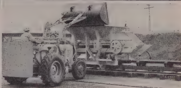
Filling portable reclaiming hopper. Pan conveyor under hopper delivers to the main belt conveyor.
