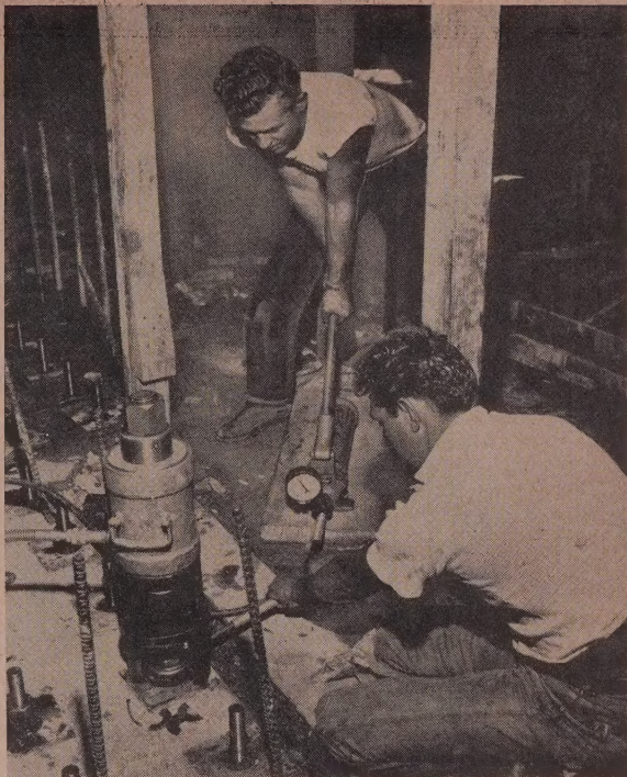
TENSIONING CREW in action. Elongation is taken up with pin wrench after hydraulic jacking. Split washers are at hand to slip into place when proper elongation has been obtained.
