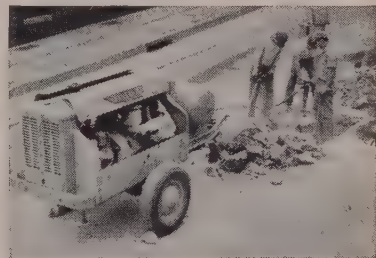
Each "125" had the air volume to hold 2 heavy-duty breakers at full pressure operation.
