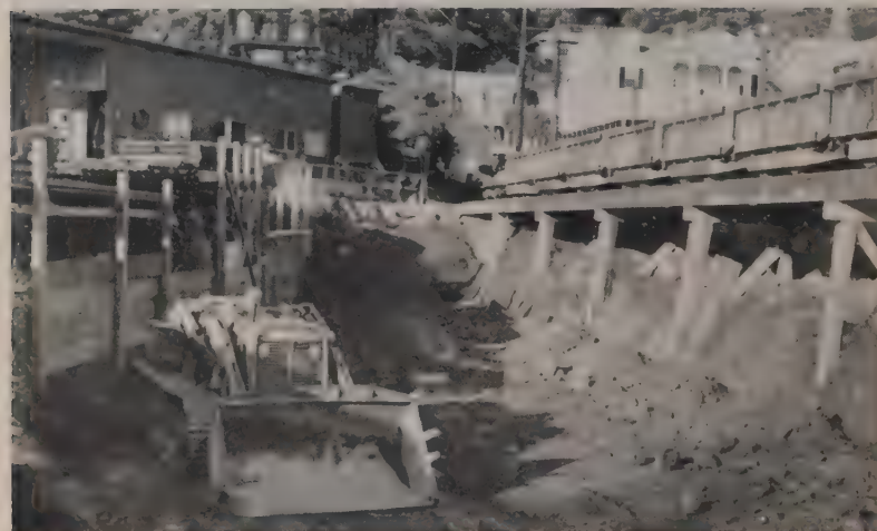
MUCK DISPOSAL at south heading. Cars are side dumped by an air-operated gantry hoist with further removal of the muck by trucks which are filled by front-end tractor loader.
