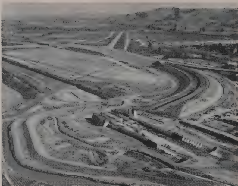
OUTLET STRUCTURE for Rio Hondo is under construction in center while earthfill is built up on either side. Similar work for the San Gabriel River in the background is near completion.
