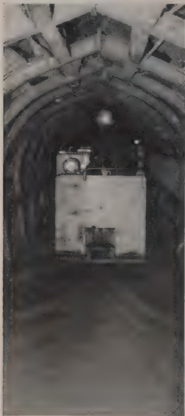
LOCOMOTIVE APPEARS to float in some places where water accumulated in 6-in. depths.
