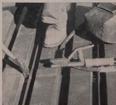
CROWN BEAD, 3/4-in. diameter, is tested. It anchors corners of four sheets to purlin.
