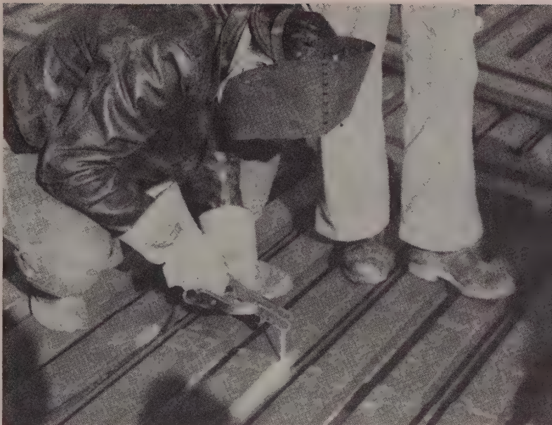
WELDING of the metal roofing to the purlins went along at a fast clip. Two welders were required, using Fleetwood L-70 rod with power supplied by Lincoln welding machines.
