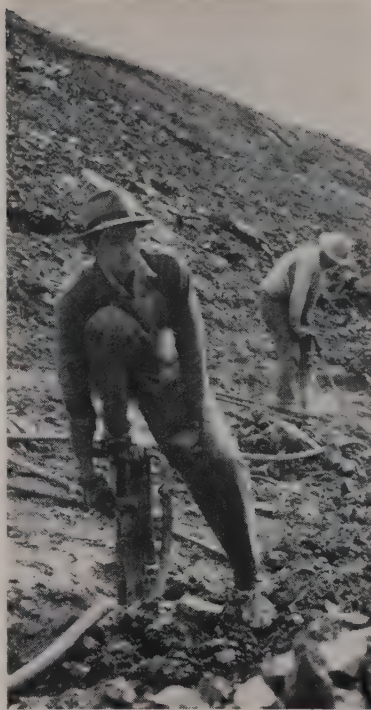
CHARLIE costs money. Said Ingersoll-Rand when providing pictures: "We're concerned with this method of operation since it puts uneven wear on the chuck and causes premature replacement."
