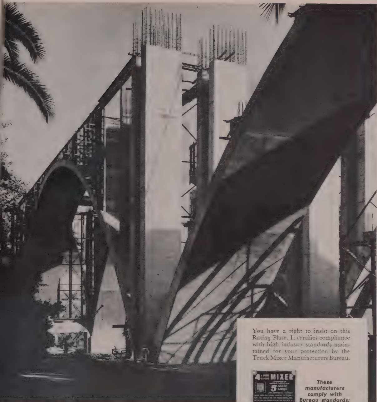
Pasadena Pioneers Bridge. California Department of Public Works, Division of Highways. Guy F. Atkinson Company, Builders.
