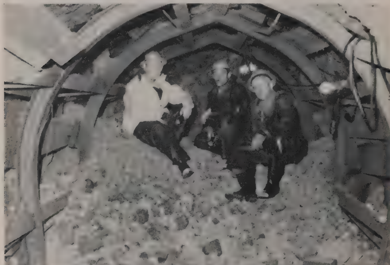
RESTRICTED CLEARANCE is evident at rear end of 120-ft. long conveyor belt where muck is loaded in successive cars of a 9-car string. Last car is being loaded here.
