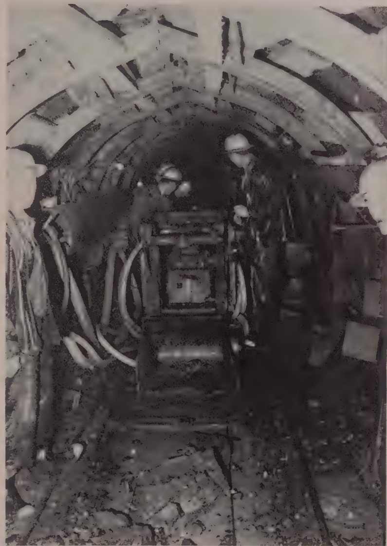
AIR LINES ARE ATTACHED to the Eimco No. 12 mucker and the cleanup begins after firing of a round. Steel sets and timber bracing can be seen against right wall of tunnel ready to be used. Extra 2 in. of working clearance was gained by making air line to left oval-shaped.
