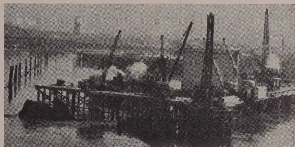
ONE BIG LIFT, with 5 truck cranes and a derrick, pulls stiff-leg out of the drink. Collapsed sheets in foreground match position shown in sketch detail at left. Pile driver bangs away on new trestle piling.
