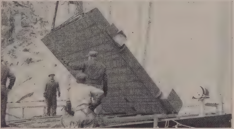
BULKHEADS, 12x14 ft. in size, were constructed of 12-in. wide-flange sections welded together to form airtight compartments. Each compartment was pumped to 100-psi. pressure from air bottles to counteract water pressure of 86 psi. at depth of opening.
