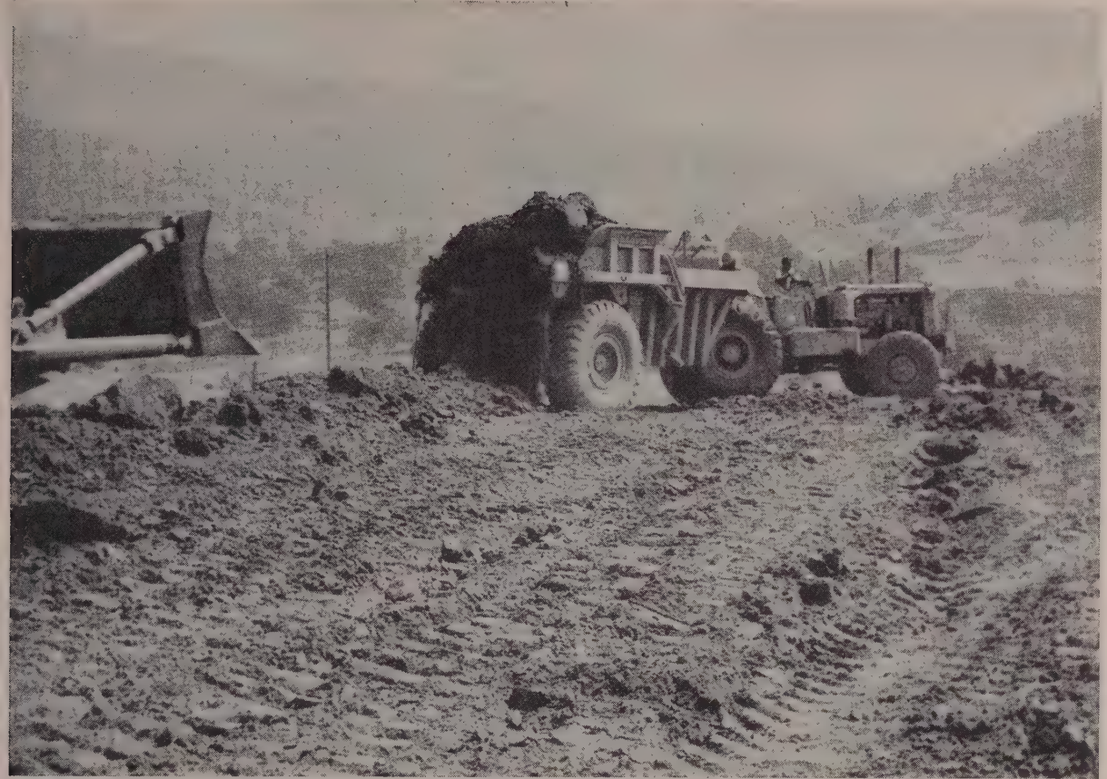
DUMPING CLAY & SHOT ROCK "ON THE GO," two MOVALLS on 1,000 foot haul keep 3 yard Manitowoc shovel busy on this highway job near Roseburg, Oregon. MOVALLS dumped their sticky loads clean as they turned at end of fill without stopping. Specifications required dumping on top, dozing over edge as shown. D & H Construction Co. and M. H. Hasler Construction Co., contractors.
