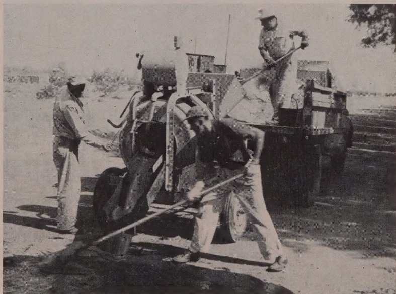
PATCHING small deteriorated road areas can be done with hand squeegees and small mixer—equipment normally available to any city. Traffic can be allowed over patch in about 1 hr.
