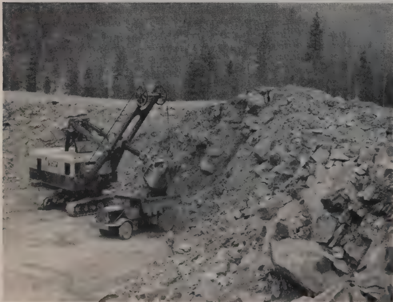
RAPID HANDLING OF LARGE BLASTED ROCK
