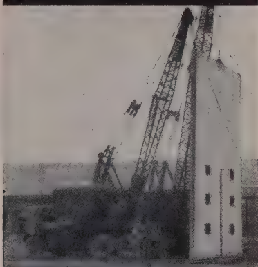
114,000 LB. SLAB being positioned
