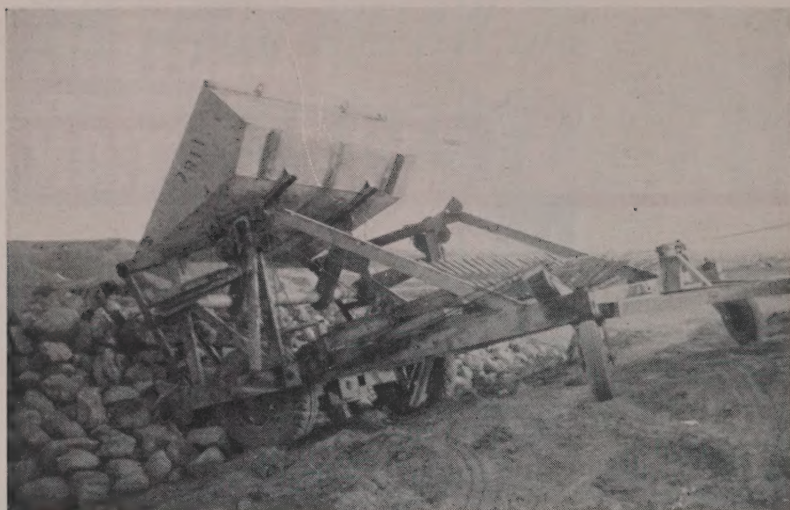
UP SHE GOES . . . and 6 tons of rock lands in stockpile at edge of fill. It can be dozed off the edge later on, or put to constructive use where the opportunity presents itself.
