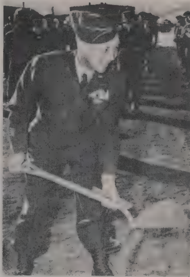
MAJ. GEN. JOHN G. VAN HOUTEN, Commander of Fort Carson, Colorado Springs, breaking ground which signaled the start of a $2,777,308 construction program which will add six new permanent barracks to the Fort by June 1956. Supervising construction of the new barracks is Lt. Col. Robert W. Dalrymple of the Corps of Engineers' Denver area office. All construction activities of the Corps in the Rocky Mountain area are headed by Col. Thomas J. Hayes, Omaha District Engineer.
