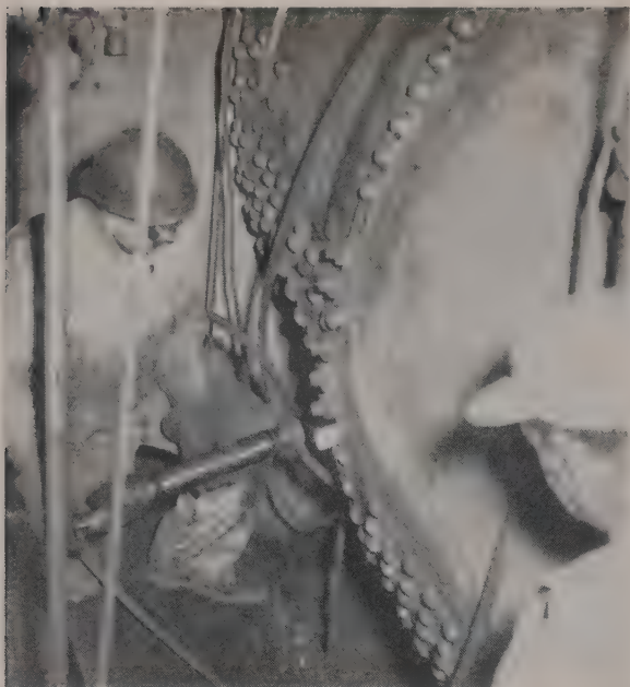
HOT RIVET is going in to replace one of the old faulty ones. Original construction misalignment of penstock plates caused the water leakage problem that necessitated the entire repair program.
