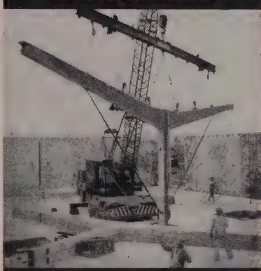
TRUSS has 60' span at top.
