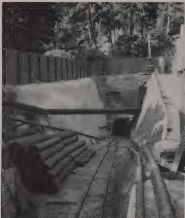
SOUTH PORTAL has gunited slopes to prevent bank cave-ins. Pipes to right (4- and 6-in. diameter) carry seepage water. Other pipelines to left carry air for ventilation and to run equipment.
