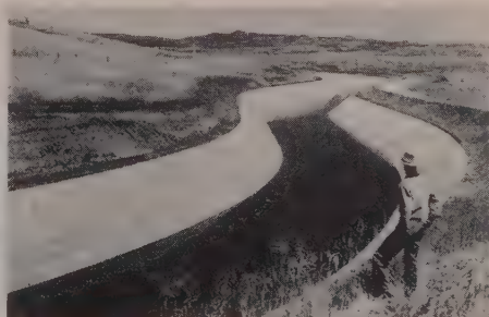
California's Delta Mendota Canal. Alkaline soil required Permanente Type 2, Low Alkali cement throughout.
