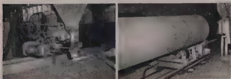
Automatic welding Steel grit blasting
