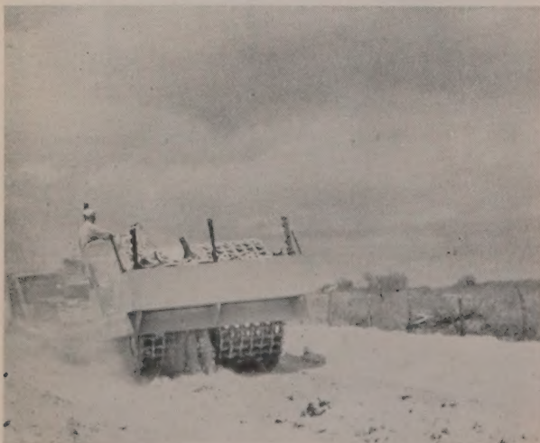
3 HYSTER grid roller with 18,000 lb. of concrete ballast is towed by Cat D6 tractor operating in third gear.
