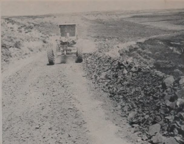
2 CAT 12 motor grader spreads part of windrow over road for next step which is size reduction by grid roller.
