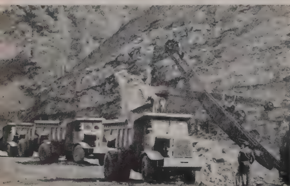
WEST VIRGINIA TURNPIKE —probably the most rugged test of equipment on all turnpikes to date because of the rocky, mountainous country. Of 275 off-highway rear-dump trucks used on the job, 260 of them were "Eucs".
