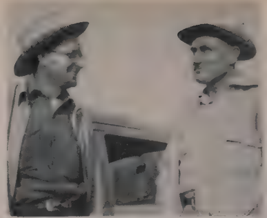
H. L. (RED) DAVIS (right), general superintendent of Alaska Division of Williams Bros., chats with Dick Hamilton , trenching superintendent.
