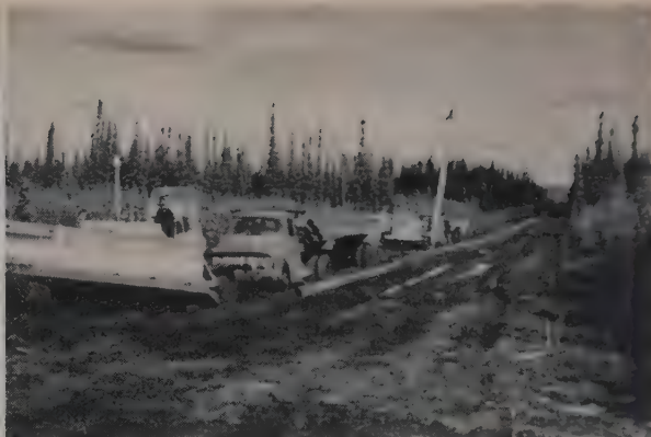
PIPE STRINGING crew out in front of spread near Fairbanks. Two spreads laid pipe — one out of Fairbanks working southeast to Canadian border, one from there on along the Alcan highway.
