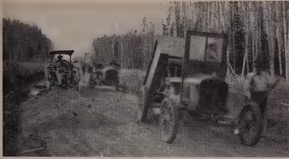
HEAVY EQUIPMENT—1929. Reconstruction of a portion of the Richardson Highway by government forces. Since then this section has been reconstructed to Alaska Road Commission "Through Road Standards."
