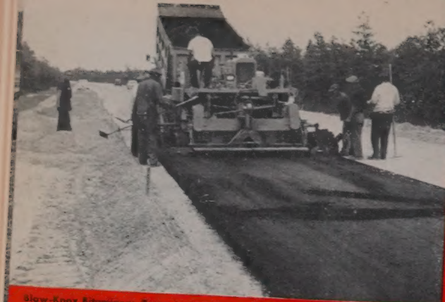
Blaw-Knox Bituminous Paver laying base course on the Garden State Parkway in New Jersey.
