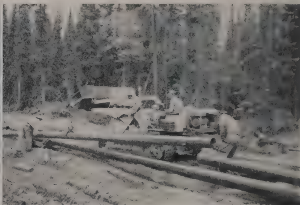
CAT HT 4 SHOVEL was used for picking up pipe for buffing on pipeline construction near Dot Lake, Alaska. Portable power units and special pipe pickup were necessary job innovations.
