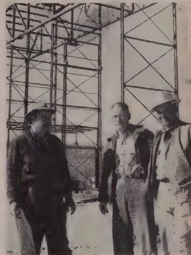
KEY MEN for Vinnell at Edwards Air Force Base near Los Angeles: (l. to r.) Schyler Walker, general superintendent for all operations; Neal Lange, general superintendent in charge of steel erection; and Robert Walling, job superintendent on erection of the hangar. (For description of job, see page 53.)
