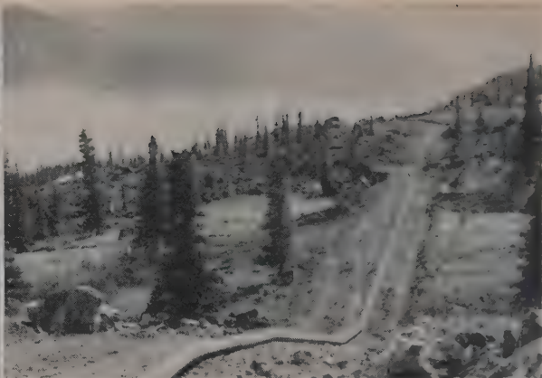
FINISHED PIPELINE lies unrestrained and in the open for 500 mi. of its total length. Only 120 mi. is buried. Rugged scene here is near shoreline of Klwane Lake in Canada.
