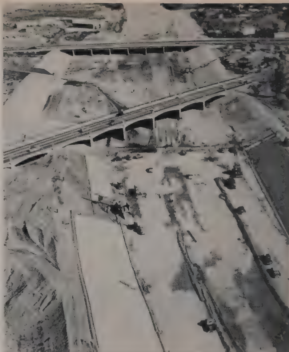
ONE-HALF of slope paving had been completed by early December before rains began. Crane in background is placing cobbles in normal flood control bank protection. New method is almost as cheap and may be used again in future work.
