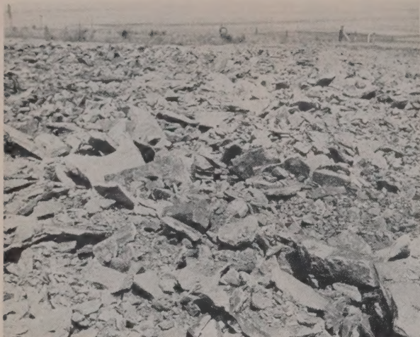
1 SHALE and sandstone deposit near road was ripped up and then hauled to nearby road and dumped in windrow.
