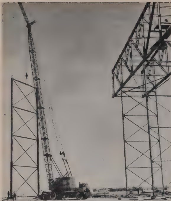
P & H TRUCK CRANE is shown carrying 75-ft. high falsework bent to position at end of trusses. An American truck crane could alternate on this work. Maximum height of lift was 115 ft. to top of trusses.
