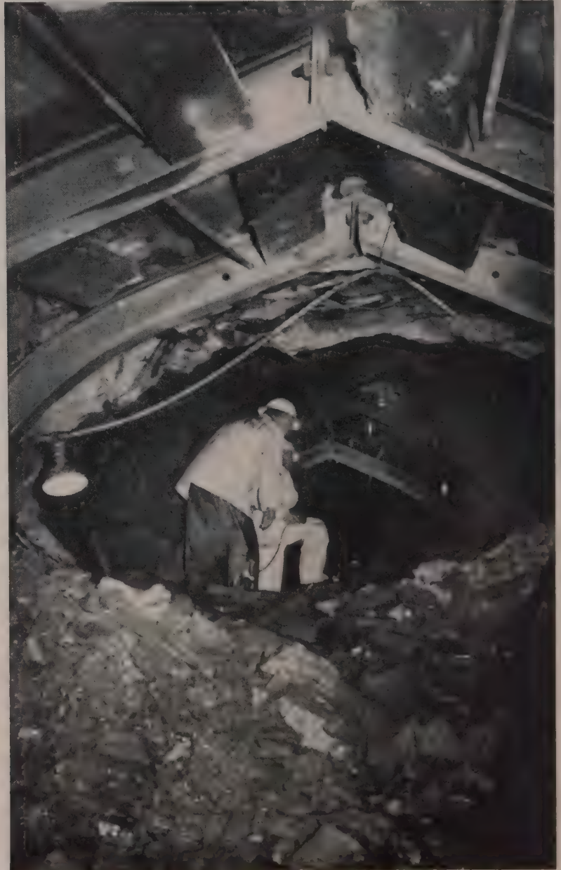
SCENE OF VICTORY shows good alignment for line and grade, and good breakage. Heat and water left behind, this work was done in the dry, with daily progress of 40 ft. toward end.
