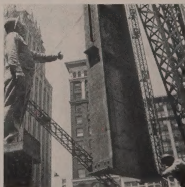
BOOM-UP signal for first steel column was given last June by Vernon Rutledge, foreman.
