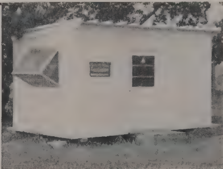
This 175-square foot Armco Steel Building serves as a "portable" field office for the Perry McGlone Construction Company, Kansas City, Missouri.
