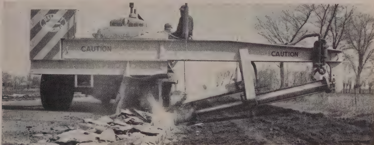
Machine is run entirely by air—even pneumatically-propelled. Shoulder is first sloped to facilitate its operation.
