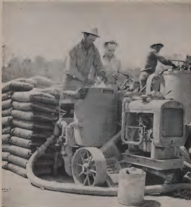
MIXING GROUT for grouting of the foundation rock of Mormon Island auxiliary dam. Ray Heffington (center) is checking the mixing time of the Colcrete Mark III double drum mixer.
