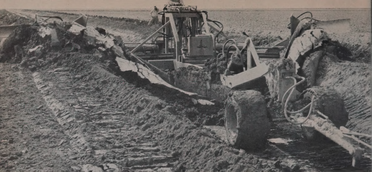
MOIST BLACK LOAM curls off the moldboards and spoil wings of the latest thing for heavy-duty canal excavation. In this test last year the
