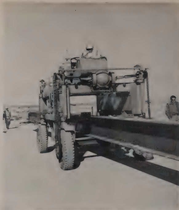
RAPID SORTING of structural steel was aided by Ross carrier. Versatility is shown here by its handling a 100-ft. long column weighing 10 tons. Sorting of steel required about 6 acres.
