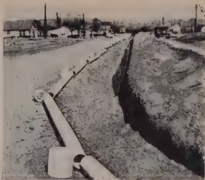
"Century" Pipe, 4" Class 150, ready for laying in trench in Oakland, Oklahoma.
