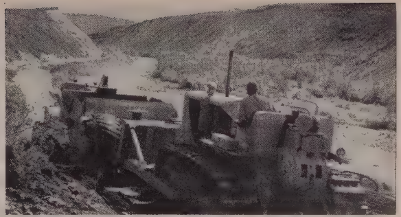
HEAVY EQUIPMENT—1955. Reconstruction of another section of the Richardson Highway by Morrison-Knudsen Co., Inc. Modern equipment such as Cat D8 bulldozer and DW20 make possible today's roads.
