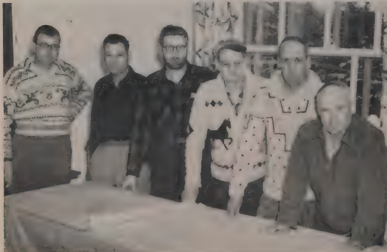
AT THE HAINES END of the Alcango Project (l. to r.): B. D. Edwards , representing the prime contracting combine; D. S. Nease and G. T. White , Corps of Engineers, inspectors; E. A. Groves and A. E. Johns , clearing sub-contractors, and J. L. McNamara , Corps of Engineers, project engineer at Haines.
