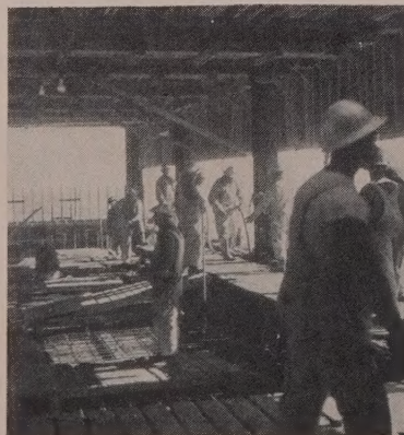
RAMP enabled contractor to pour spandrel beams same day that floor was poured.
