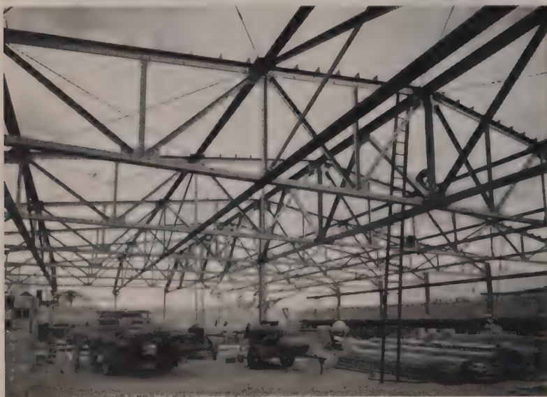
ONLY ONE COLUMN IN THE CENTER OF THE BUILDING
