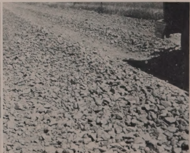
4 REDUCED MATERIAL is shoved to opposite shoulder and process repeated. Final result is maximum 2½-in. oversize.
