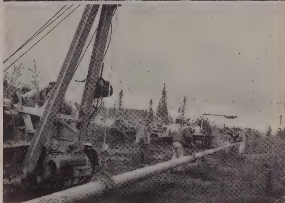
TWO LINCOLN welders were mounted on D6 tractor. Welding team consisted of three stringer bead welders followed by three filler welders. Three more cover men completed the welds. Other tractors with sidebooms prepared pipe for welding.
