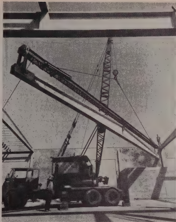
ROOF BEAMS, 66 ft. long, span one-half width of building and are spaced at 20-ft. centers. Rafters, 2x10, rest in joist hangers and have solid \frac{3}{8} -in. plywood sheathing over.
