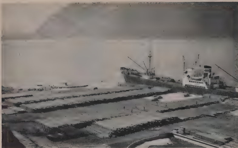
8,500 TONS OF PIPE , slated for use in the 281-mi. Canadian portion of the project, was stockpiled at the port of Haines after shipment from England. British firms manufactured pipe for the Canadian portion, and American firms for the Alaskan stretches.
