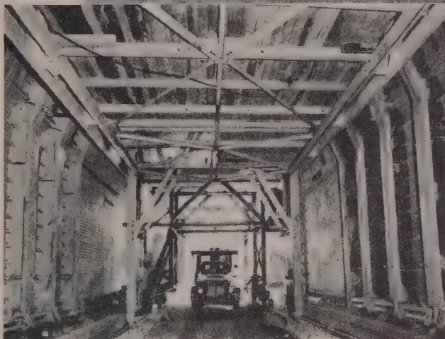
Blaw-Knox telescopic combined sidewall and arch forms (shown above) and telescopic ceiling forms were used on this West Virginia Turnpike Tunnel. Sidewall forms are provided with scoring wires.
