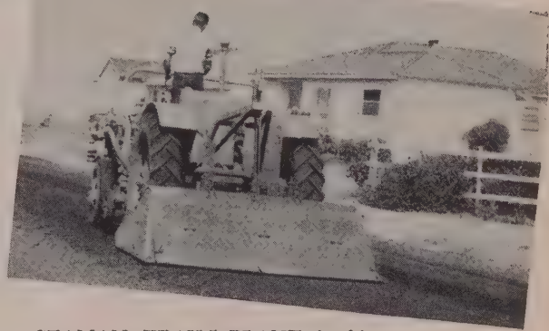
SEAMAN TRAV-L-PLANT in bituminous city street construction.
