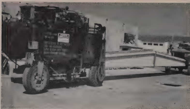
ALL 66-FT. prestressed roof girders were transported two at a time on lumber carriers from a casting yard 5 mi. distant from the job location. Good trick for getting around corners.
