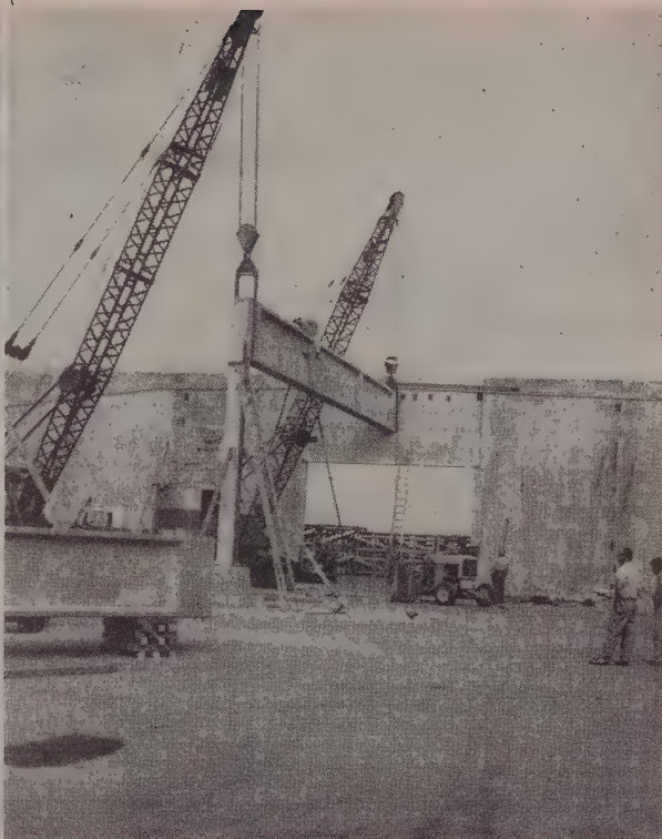
ONE ROW of prestressed girders runs down centerline of shed on 40-ft. centers. Provision was made for doweling beams and girders to their supports. Columns and walls are precast units.
