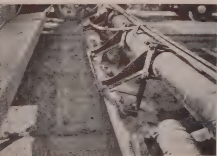
BLACKTOP WIDENING & PATCHING. The same machine operated from power plant on auto-trailer with pickup for Compactor is most efficient means of blacktop pavement patching, paving walks, drives, etc. Will compact up to 2000 sq. ft. per hr. close to maximum density.
