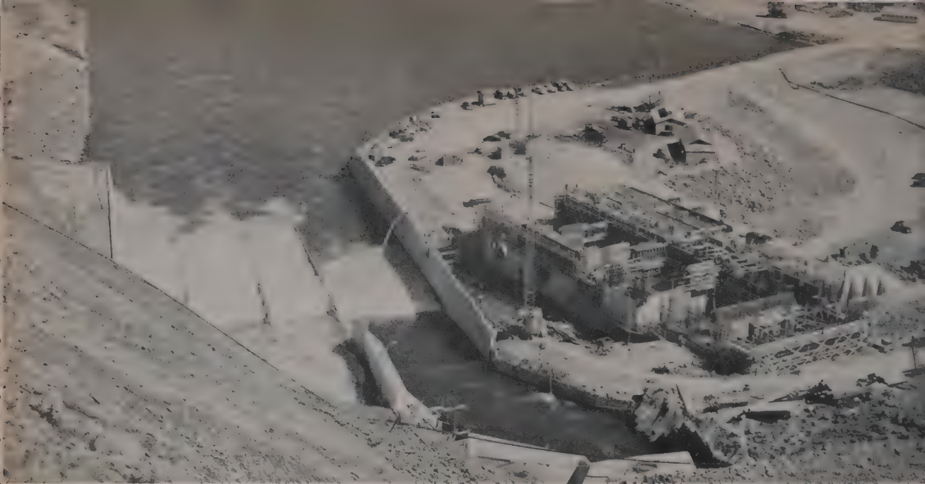
COMPLETION of outlet and power tunnels, and stilling basin at Palisades Dam permitted first use of these facilities for river diversion during 1954. Functional completion is
