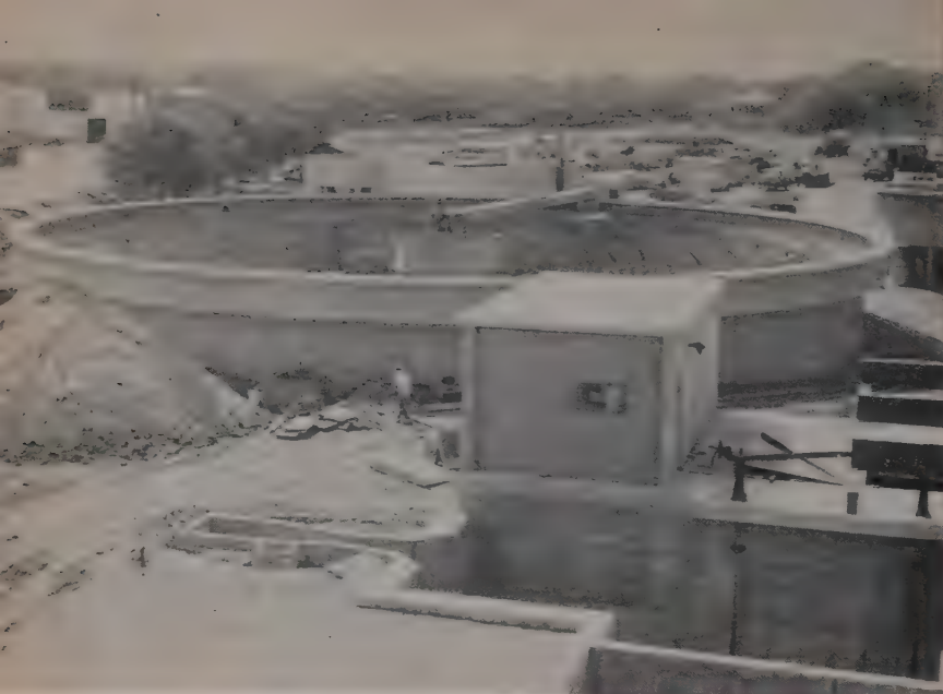
BOOMING ALBUQUERQUE turned to bond issue to finance much needed expansion of waterworks and sewage facilities. Clarifier pictured is a 1954 improvement to the city's sewage treatment plant, built by C. H. Leavell & Co.
