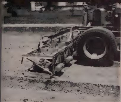
MACADAM DENSIFICATION. Usually just one pass of the Jackson Multiple Compactor is required to key 12" of rock to final density — one pass to completely fill voids with fines.
