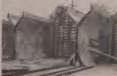
ASSEMBLED SECTION of "Y" wall truss with UNI-FORM Panels
