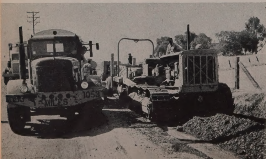
STABILIZING in-place road materials in Contra Costa County utilized such equipment as this Wood mixer. About 3 mi. of two-lane roadway was reconstructed under a $233,000 contract and completed late in 1954.
