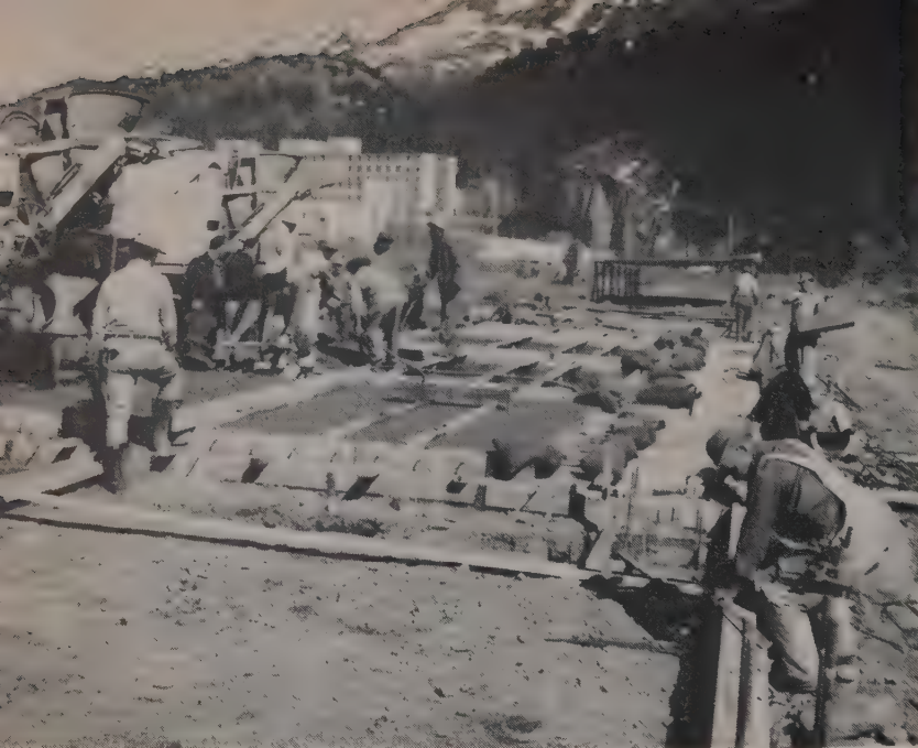
TILT-UP shaves costs in Alaska, too. This is J. H. Pomeroy's $1,236,000 contract for composite shops at Whittier, now 80% complete. Tilt-up came north only 3 yr. ago.
