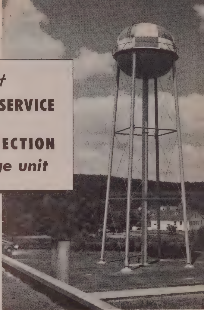
100,000-gallon P-DM dual service elevated steel tank at Hartford Special Machinery Co., Simsbury, Conn.
