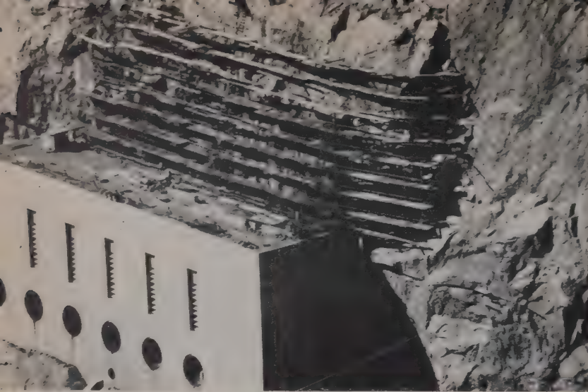
ANCHOR BARS UNDER TENSION were feature of preventive maintenance above Nevada valve house at Hoover Dam, Selby Drilling Co. secured a slab 19 ft. thick, 120x180 ft. in area, and grouted the bars in for good measure.
