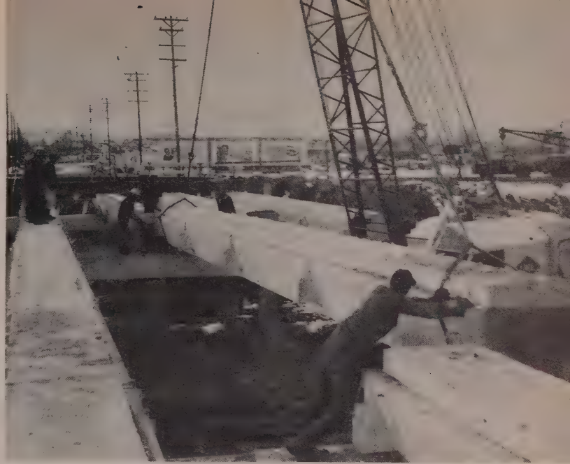
PRESTRESSED CONCRETE is on its way for Denver city structures. Here's one of 24 girders making up the Mississippi Avenue bridge. C. M. Hanes held the $127,450 general contract.
