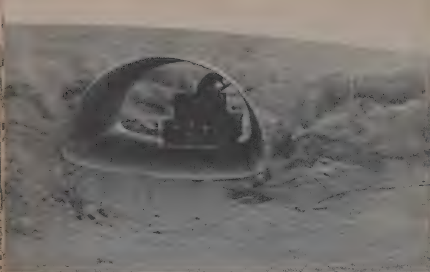
TRUCK BED beats scaffold for bolting culvert plate. Installation is typical of Umatilla County work aimed at replacing old wood structures.
