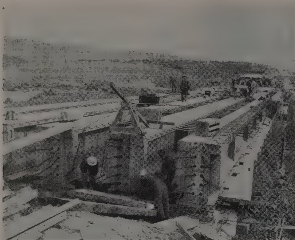
JUST STARTING the stressing operation on one of the beams, the men are removing the formwork beneath the beam end to free it from any possible stresses resulting from beam camber prestressing.
