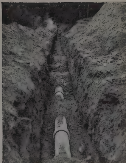
Part of a 13-mile installation of "Century" Pipe, Lakewood Water District, near Tacoma, Wash.
