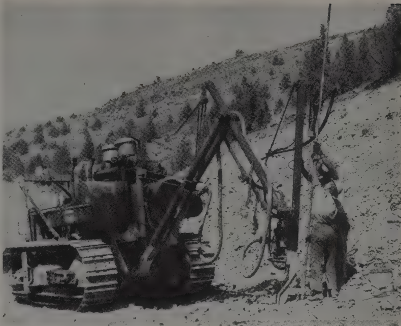
VERSATILE RIG is composed of HD-18 crawler and Ingersoll-Rand drill, with shop-made flexible linkage in between. Two men sink a 13-ft. hole every 15 min.
