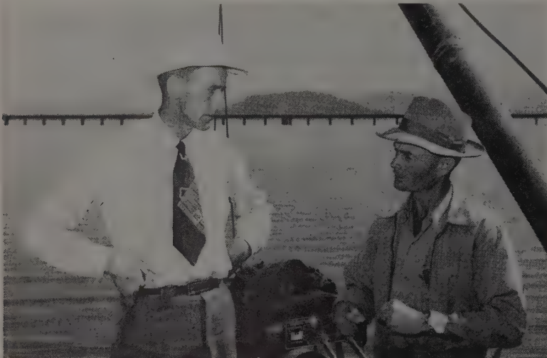
RESIDENT ENGINEER at Sandpoint, Idaho, is Al Sachse (left) of the state highway department. Here he listens to a report from Clyde Wood , pile inspector.
