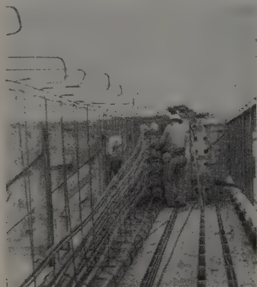
CABLES are in place followed by workmen placing steel on the support frames. Side forms will be fastened next to the near side.
