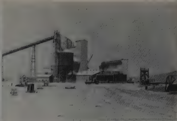
CONVEYOR LEADS in from left to top of tower and 1,100-ton aggregate storage. Two silos this side of tower hold 14,000 bbl. of cement while low building to right houses extensive refrigeration plant.
