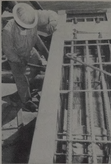
TAKING A STRAIN , workman forces pile into exact position under cap form. Note anchor bolt assembly, adjustable plywood panels in bottom of form.
