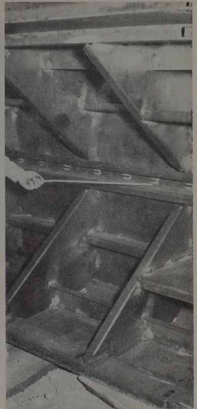
SOFFIT FORMS for precast deck units "break" in the middle. Steel shores make forms rigid for concrete placement.
