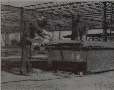
Fig. 1. 440' x 440' all welded framework for American Sterilizer Company, Erie, Pa. On-the-site fabrication cuts steel handling costs, saving an estimated, $15 to $20 a ton.
