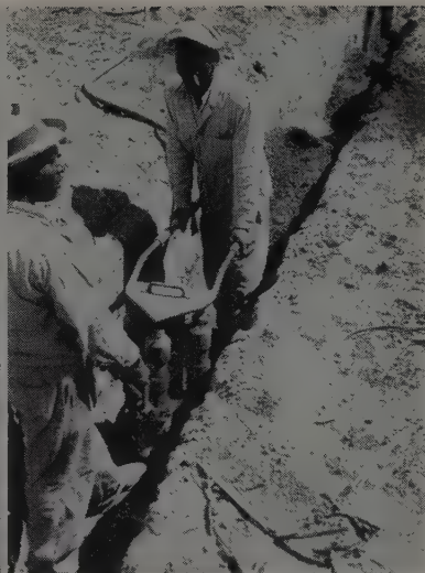
PNEUMATIC COMPACTION of 1-ft. layers was necessary for most backfilling of trenches. Water jetting was used in good soils.
