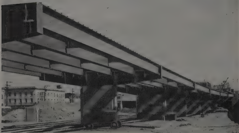
ERECTION OF THE STEEL superstructure for the Freeway approach to the San Francisco Bay Bridge has been completed by Bethlehem Pacific crews. This unit recently won an American Institute of Steel Construction award for aesthetic design. The $897,090 contract for the superstructure and decking is held by Eaton & Smith.
