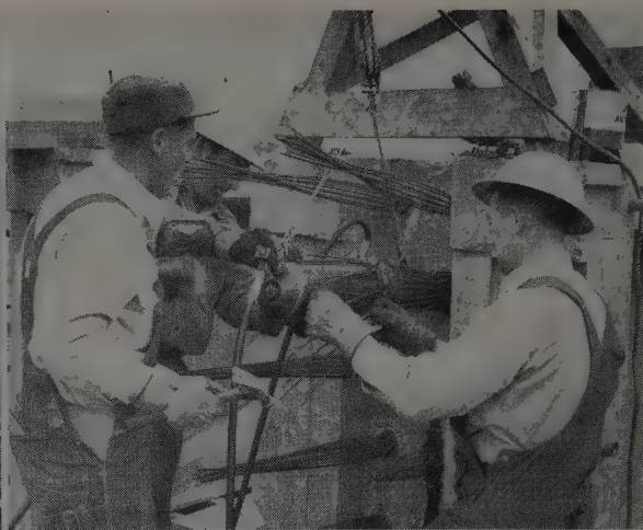
WITH MANY HANDS in the same place at the same time, teamwork pays off on wedging the wires. Time is nearly constant on actual stressing, thus speed on setting up jack determines rate that work goes.
