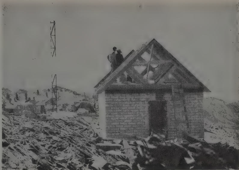
REMOTE STATION construction was essential to hurdle California's Sierra Nevada, linking east and west. Here is radio vault on White Mountain, el. 11,000, near Bishop.
