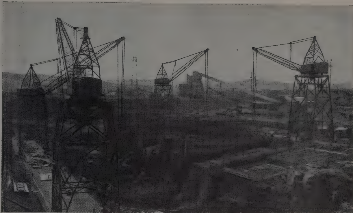
These four Washington Whirley cranes work 'round the clock on The Dalles Dam being built by The Dalles Powerhouse Constructors on the Columbia River. Tiger Brand ropes on these cranes are all in good condition after several months of hard service.
