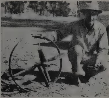
FOR EQUIPMENT in action at right, pilot hole is drilled with small drill. Larger 24-in. auger is pulled through pilot hole. Holding pieces is G. Mitchell, foreman.
