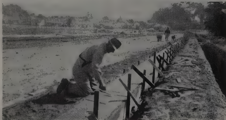
HAAS CONTRACT called for 2 mi. of curb and gutter such as is being finished here. Techkote membrane curing was used. Ditch to right is for underground electrolier conduit.
