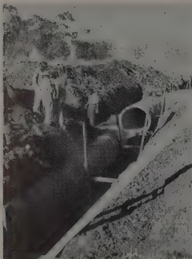
SHORING IS NECESSARY to hold large storm drain in place while small sewer pipe is laid in trench next to it.
