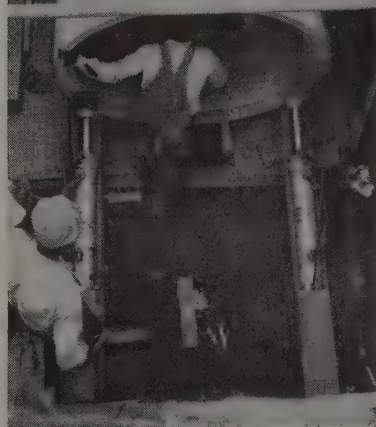
TWO 100-ton RODGERS hydraulic jacks press against first two sections of 60-in. drain to go under highway. Heavy timber is placed between jacks and pipe at later stages.
