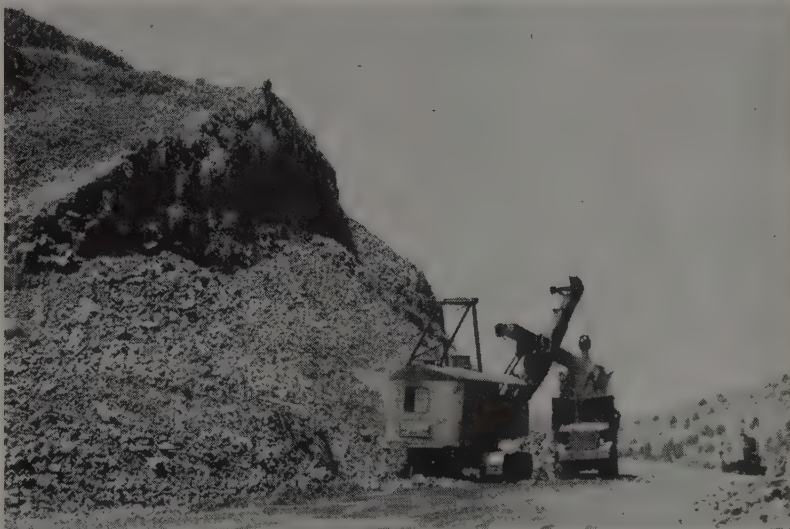
SHOT BANK is easy loading for Northwest, but a bumpy proposition for traffic. This is almost the only spot on the 7-mi. job where old and new alignments interfere.
