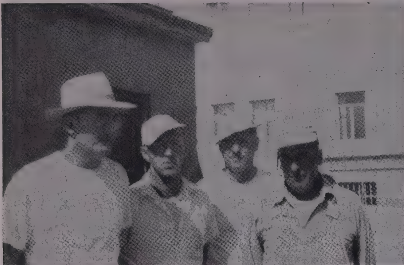
LOWE CONSTRUCTION CO. has a $1,000,000 contract to erect a bank building for Security Trust & Savings Bank at Billings, Mont. Shown above, left to right, are: James O. Kimble , job superintendent; Leonard Koski , carpenter foreman; Vern Hendershot , labor foreman; Bob Senitte , carpenter foreman. Not shown are Bill Green , general superintendent, and Claude Wiesener , steel foreman.
