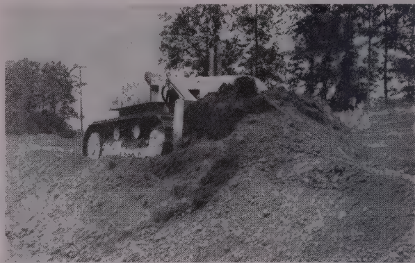
DOZING LOADS like this seems light work for Euclid's new TC-12. Twin engines totaling 380 hp. make it tops in speed and strength.
