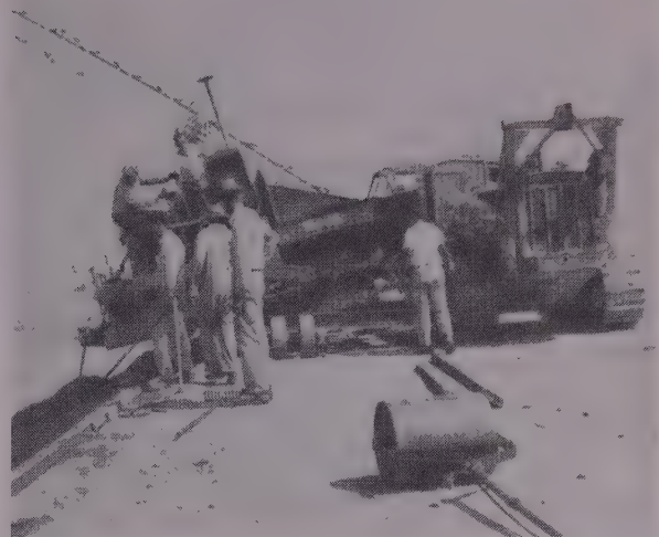
SPECIAL RAMP attached to tractor allowed spreader to complete its run to the top of the slope. The ramp then tilted clear of the ground and was moved forward 12 ft. ready for a new pass.
