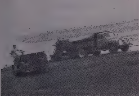
THREE PIECES of equipment—truck, mechanical spreader, and 4½-ton roller—are held individually on the slope by cables attached to two tractors and a crane located at the crest.
