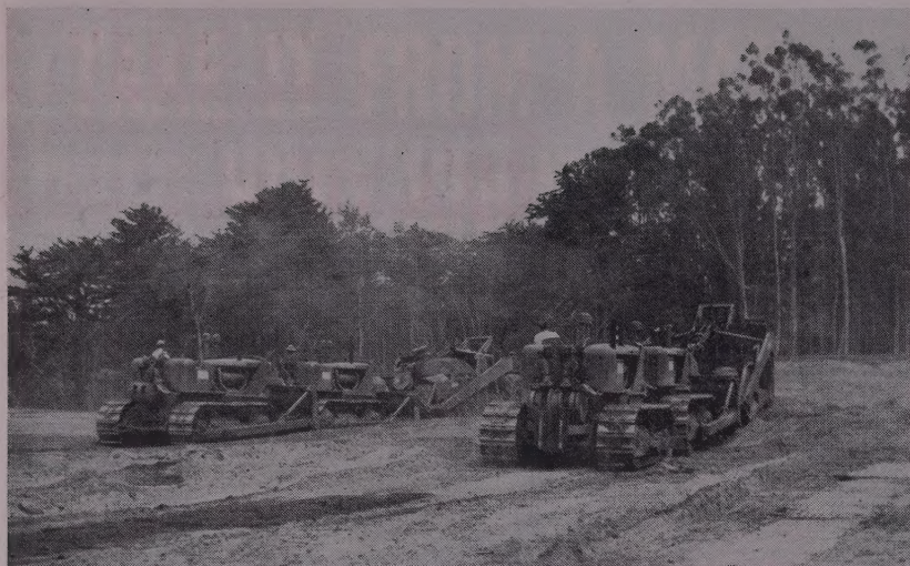
DIRT IS FLYING as each of these Wooldridge Terra Cobras is push-loaded by two Allis-Chalmers HD20's. The rapid loading time is only 15 to 20 sec. in a distance of 100 to 150 ft.
