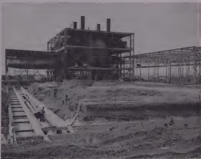
ANOTHER METHOD for insulating steam lines is the use of utilidoras as in the foreground. Utilidor walls are reinforced concrete and the lids precast. In the center background is the heat and power plant proper with coal storage building to the right.
