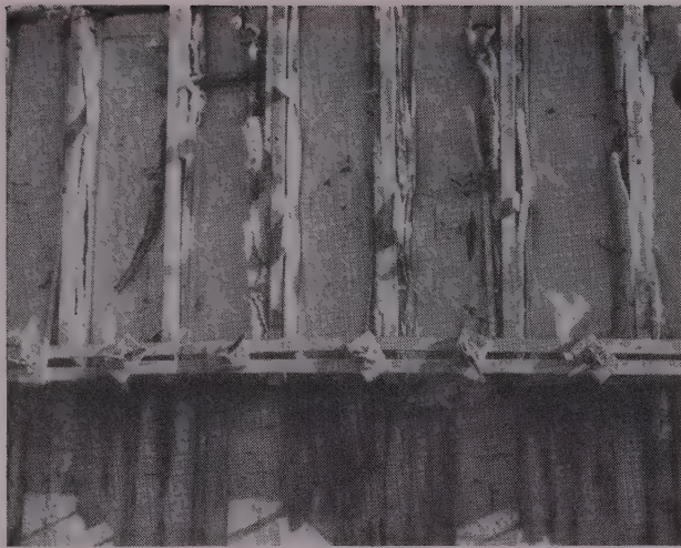
FIBER GLASS insulation blankets were cut to stud spacing and fastened to outside of sheathing by 1x2-in. wood strips nailed to the forms. The form shown here had been used 7 times previously.
