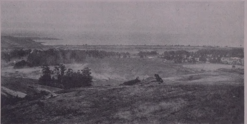
FULL 1,000 AC. OF DEVELOPMENT can be seen here. Trees have been cleared from the hills in the foreground with burning still in the process. Borrow pit is located at left center of photo with material being hauled to the flat area in far background.
