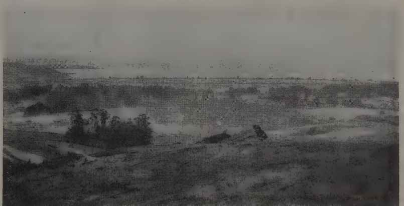
FULL 1,000 AC. OF DEVELOPMENT can be seen here. Trees have been cleared from the hills in the foreground with burning still in the process. Borrow pit is located at left center of photo with material being hauled to the flat area in far background.
