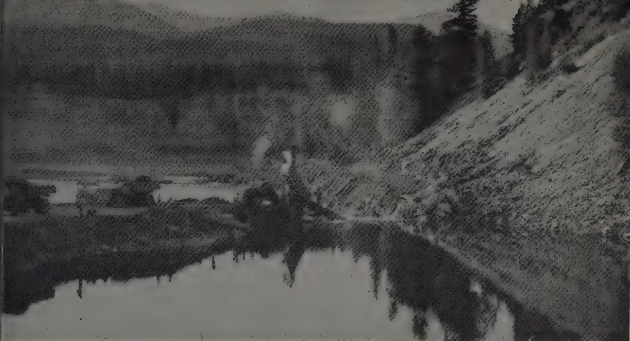
END OF THE BATTLE was in sight as twilight came over Box Canyon. This was 6:07 p.m., and the cofferdam was closed just 28 minutes later. A day's work is well illustrated by comparison of this picture and the one on page 64.
