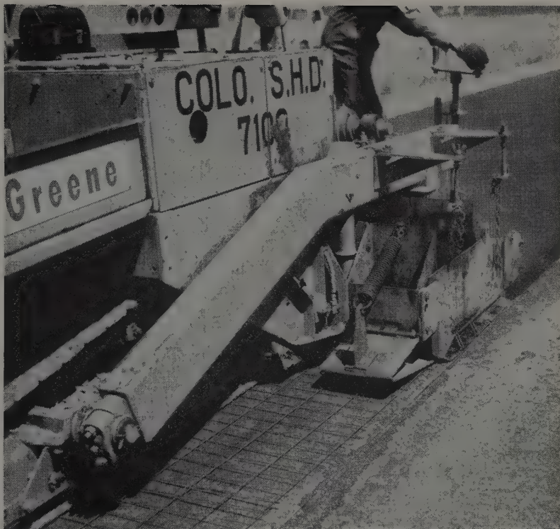
AS HOT-MIX PAVER SPREADS 2-in. course over steel welded wire fabric reinforcement, the fabric is prevented from entangling the conveyor screw by job-devised hold-down shoes at each outside track. A 10-ft. long T-plate between tracks completes the hold-down device.
