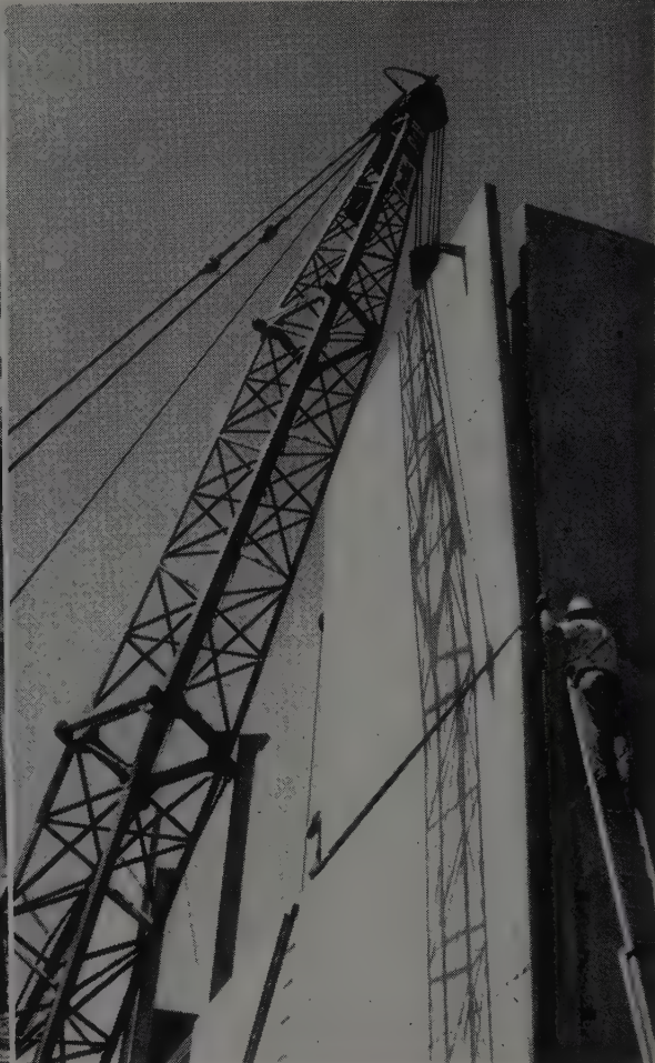
TWO TIERS of 20-ft. wide wall panels make up the 46-ft. wall height. Lower tier is 27 ft. high and upper tier 19 ft. high.
