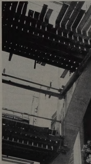
STEEL HANGERS from 8x16-in. cross timbers solve problem of supporting joists and forms for struts between arch ribs.
