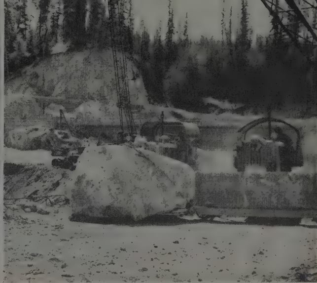
THIS ONE DIDN'T. Sling snapped and crane boom whipped. Result: 2 hr. downtime for fouled rigging while Cats and Eucs took over.
