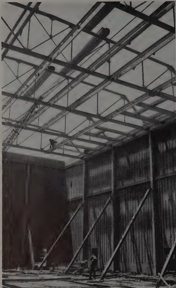
TRUSS framing in the main 90x140-ft. color studio. Temporary shores were required for tilt-up walls erected prior to trusses.
