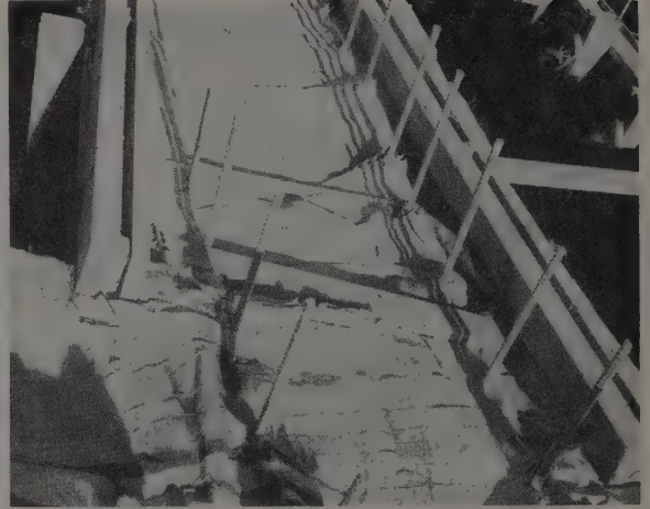
SPECIAL SHAPES such as this sluice pier at Kirwin Dam can be covered with little difficulty. Reinforcing steel bars will fit snugly in holes punched through the blankets.
