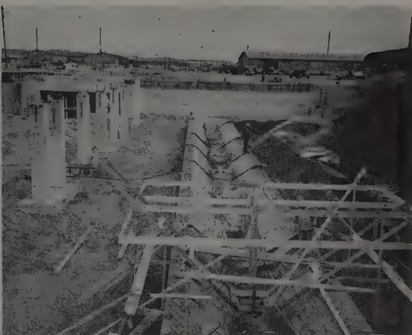
CARPENTERS INSTALL template prior to installation of reinforcing steel for concrete bin in power plant's coal storage building. In background, backfill is sluiced for consolidation.
