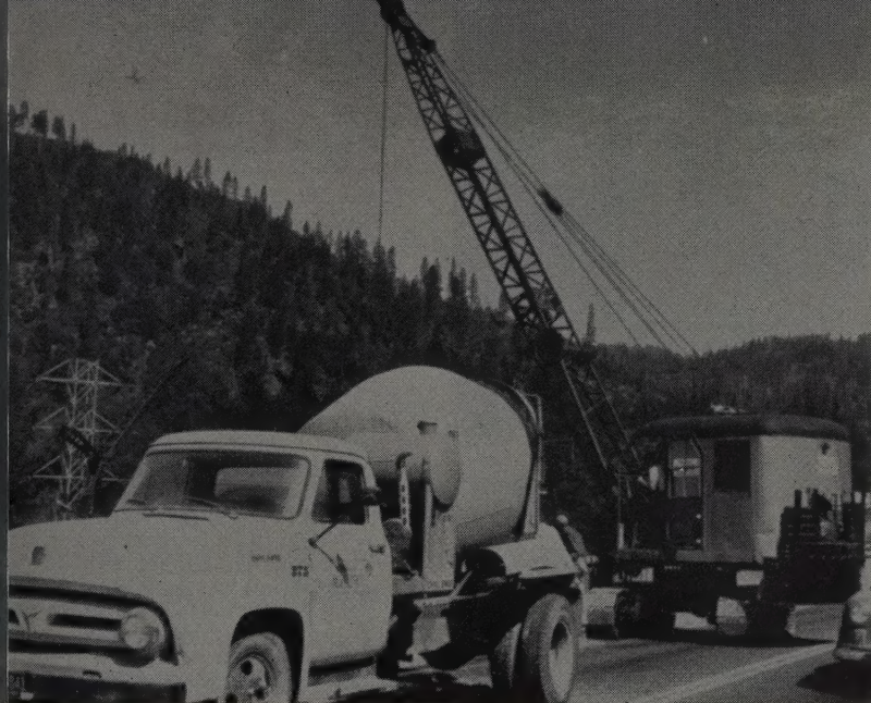
"BOBTAIL" OSGOOD crane handles concrete work from top side. Putting most of counterweight under cab assured one clear traffic lane on existing bridge.
