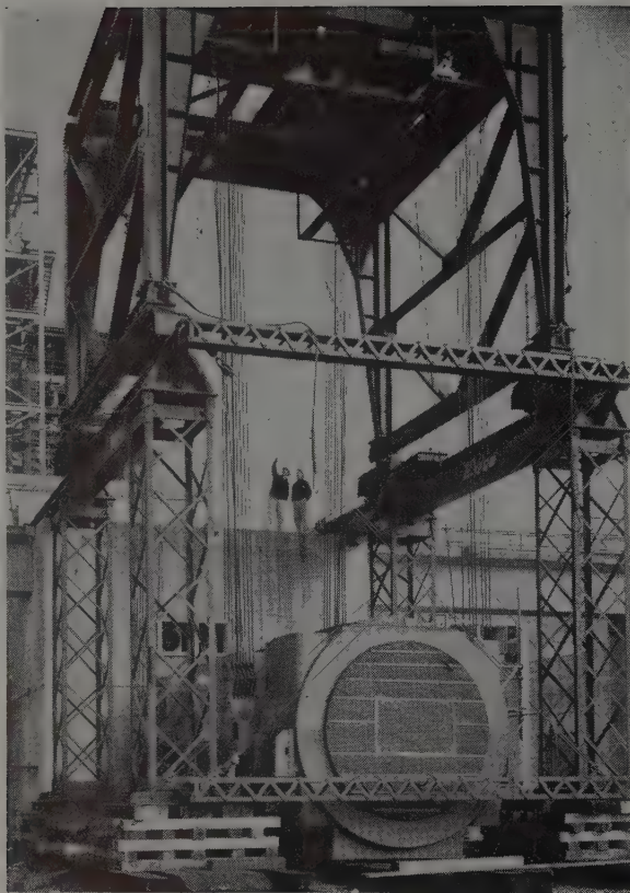
TOWERS of angle iron construction were first erected over the stator, then the portable gantry on top of heavy beams spanning between towers. Connections have been made and the lift is ready.
