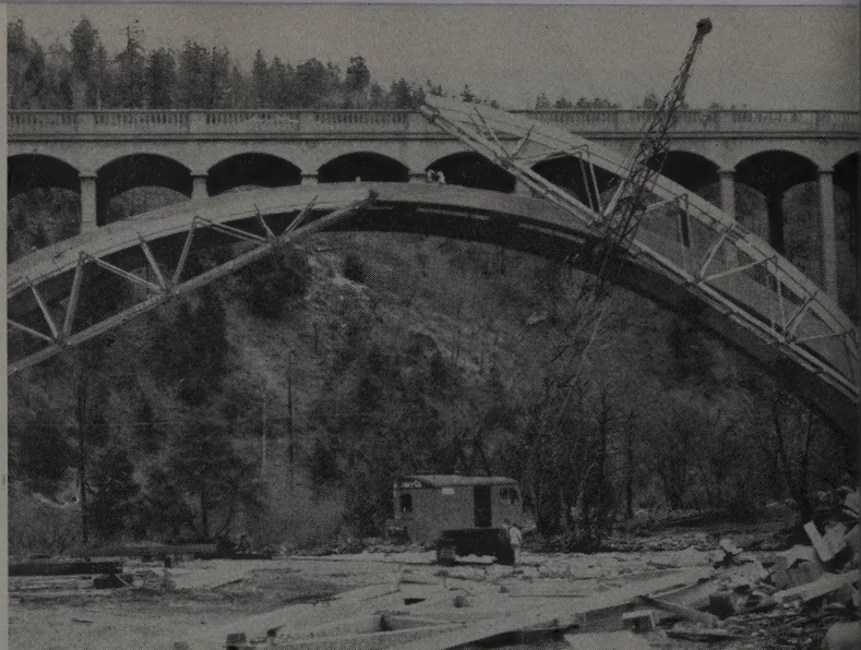
PIN AT CROWN comes next. Trusses at left are a little high, can be lowered as necessary to make connection easier. Workmen on old bridge arch will set struts and cables for lateral support of completed arch assembly.
