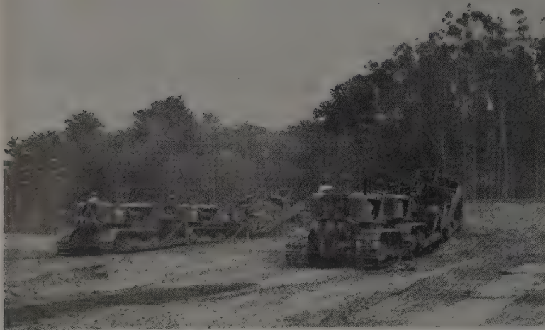
DIRT IS FLYING as each of these Wooldridge Terra Cobras is push-loaded by two Allis-Chalmers HD20's. The rapid loading time is only 15 to 20 sec. in a distance of 100 to 150 ft.
