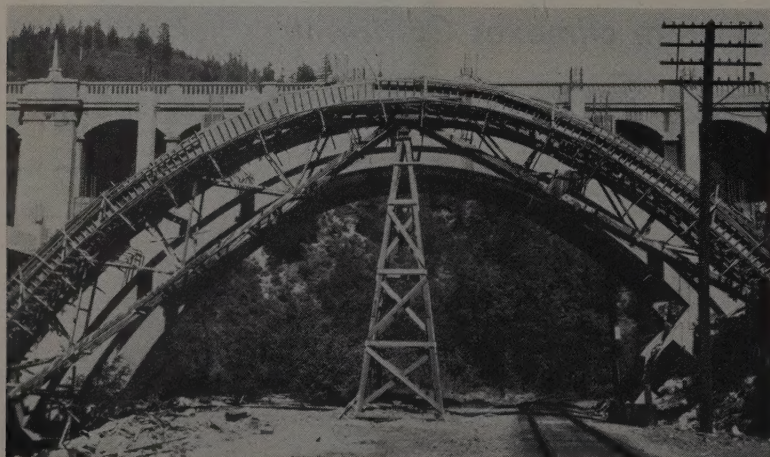
SPECIAL SOLUTION met clearance requirements over railroad main line. Support under central tower included sand jacks for decentering.
