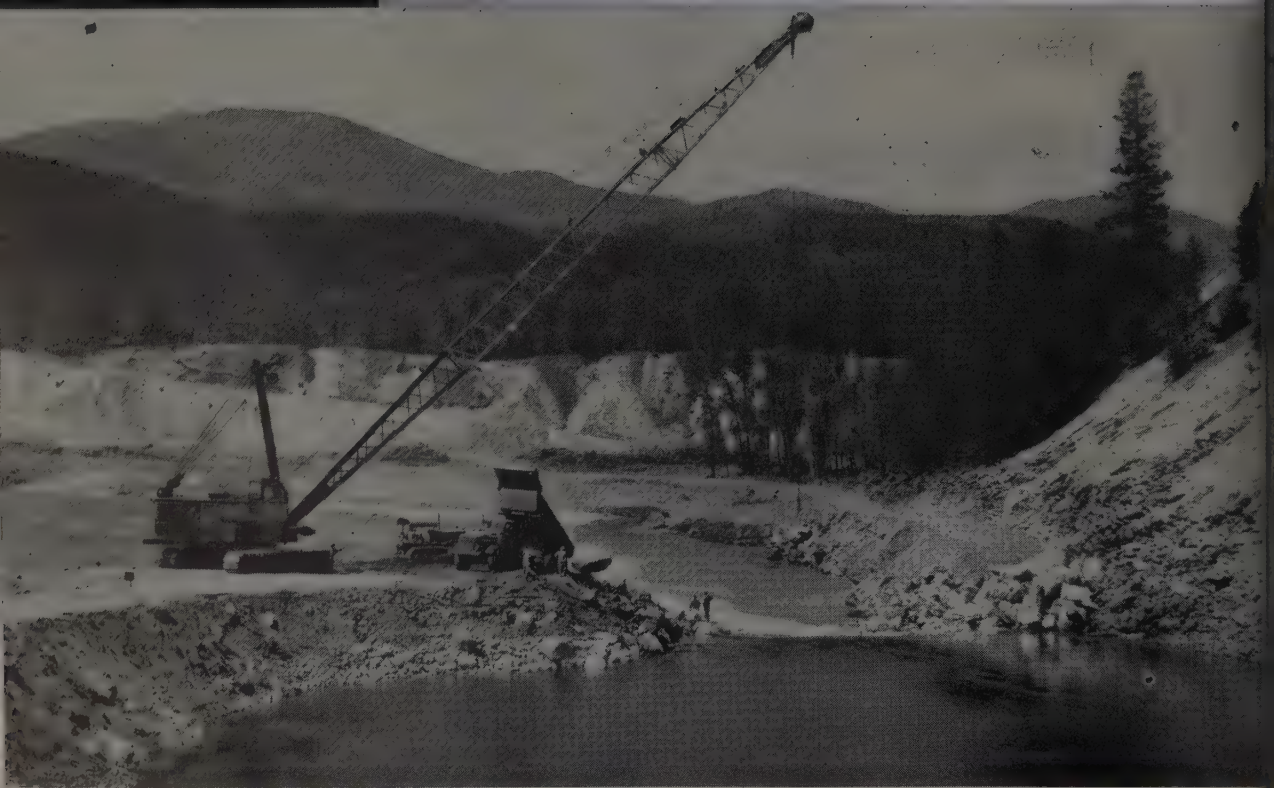
SCENE OF BATTLE was well defined as final day's work got under way. Here's teamwork—a boulder leaving the Euc while the crane spots out over the white water. Trucks had to get their beds down fast so as not to hit the crane boom when leaving cofferdam.
