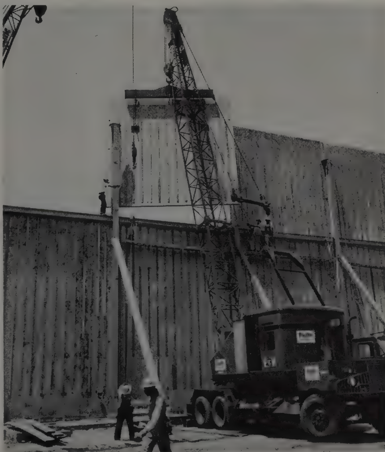
LOWER PANELS were tilted up by use of four pick-up points. Upper panel now going into place uses only two. Truck-mounted cranes were able to place all main structural elements.
