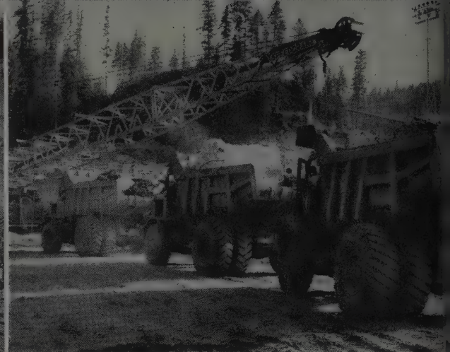
ON THE FILL Eucls pushed the crane into the background as the work moved to a climax. Here's nice distribution: one load of rock, two of loose fill.
