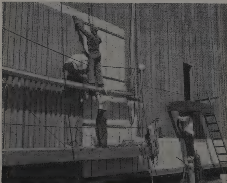
WINTER TEMPERATURES of 30 deg. below zero make insulated metal siding a necessity. Federal Roofing is placing over 88,000 sq. ft. Welder to the right is tack-welding siding to girt.
