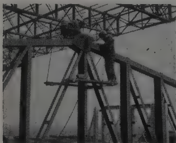
Fig. 2. Erecting shop-fabricated half-sections to form 134' trusses by arc welding.
