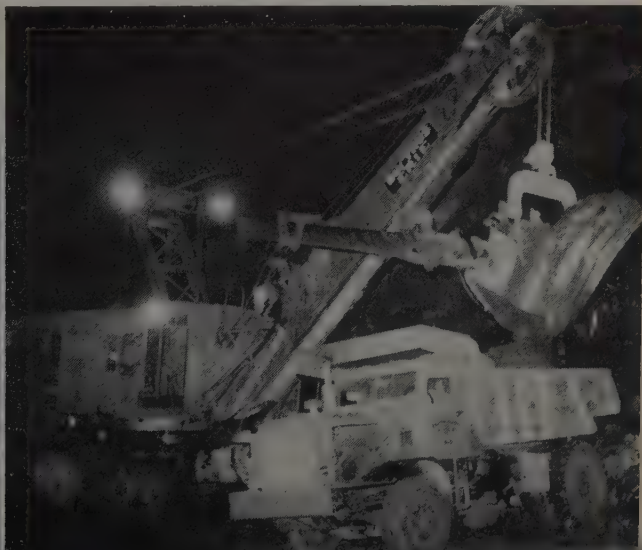
ON INTO THE NIGHT , machines worked to top out new fill, speeding the day of upstream cofferdam completion and unwatering.
