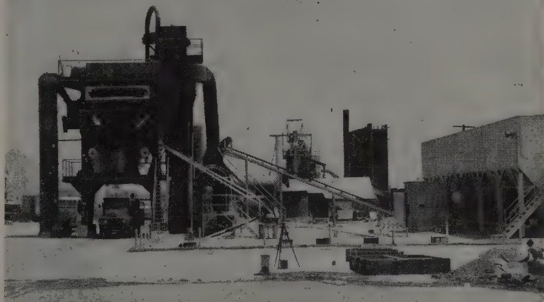
ENTIRE PLANT LAYOUT and function is shown here. Aggregates from the bunkers on the right are combined on the conveyor belt and carried to the drier. Hot aggregates from the tower go up the elevator to the right of the tower and the dust up the elevator on the left. From the top of the tower down are the gradation control unit, the bins, the weigh box, and the pug with discharge into the truck below. Heated storage tanks furnish asphalt to the tower.
