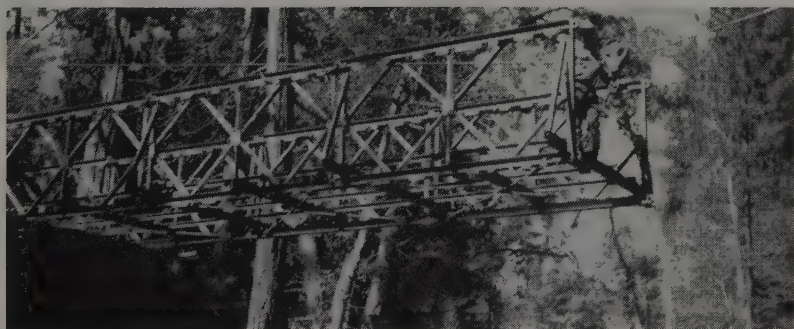
COMPLETED STRUCTURE at the left is composed of an 80-ft. and a 60-ft. span. Erection shown above was by means of a high line "floating" the outboard end, while 10-ft. panels were added at the opposite end. Completed cost is only half that of a comparable log structure.
