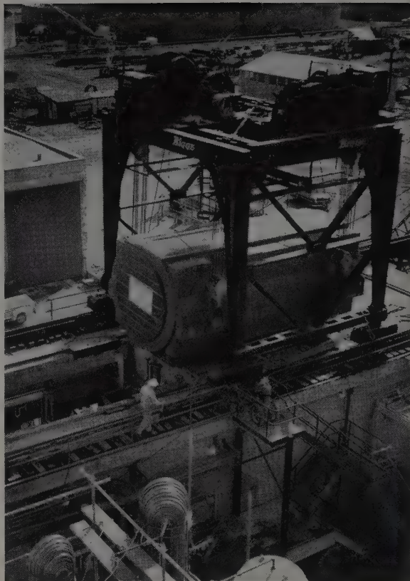
AFTER LIFTING the 236-ton stator approximately 30 ft. vertically between the towers, the portable gantry then travels horizontally along temporary rails to set the stator on its foundation.
