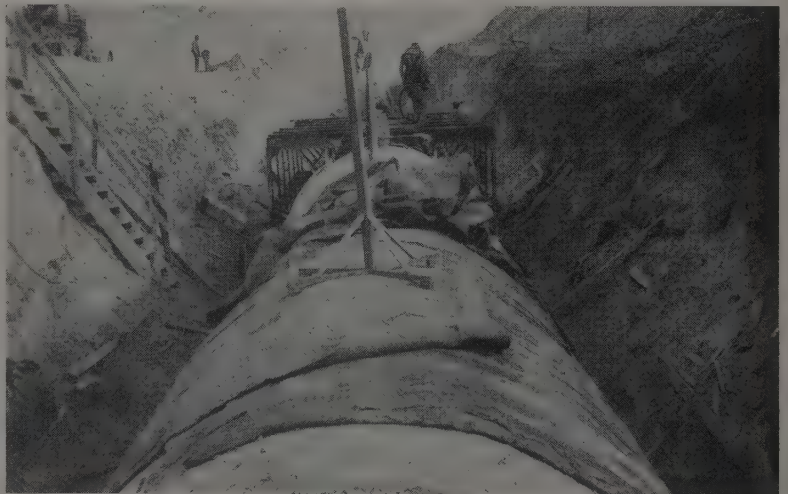
ROCK WOOL INSULATION blankets were placed directly on the exterior concrete surface of Courtland Canal siphon barrels. Metal slip forms were covered for 12 hr. prior to stripping while the concrete hardened.
