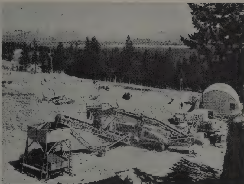
COMPLETELY PORTABLE , all electric Pioneer 46-VE crushing plant was set up in 6 hr. and ready for production. This plant produced 4,000 cu. yd. of ¾-in. minus gravel in the first three days.
