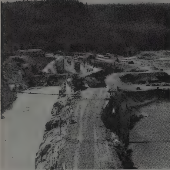
Long forebay channel hugs left bank below dam. White water from the diversion tunnel is stopped short of the powerhouse and turned out to the right just beyond boulders stockpiled for river channel cofferdam closure.
