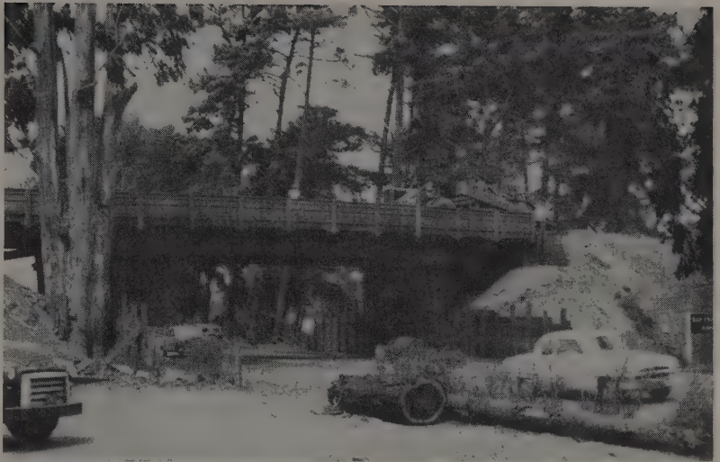
TWO LAMINATED WOOD BRIDGES with spans up to 60 ft. were manufactured by Timber Structures, Inc., to solve the problem of earthmoving over a four-lane highway and over railroad tracks. All timber parts will have excellent salvage value.
