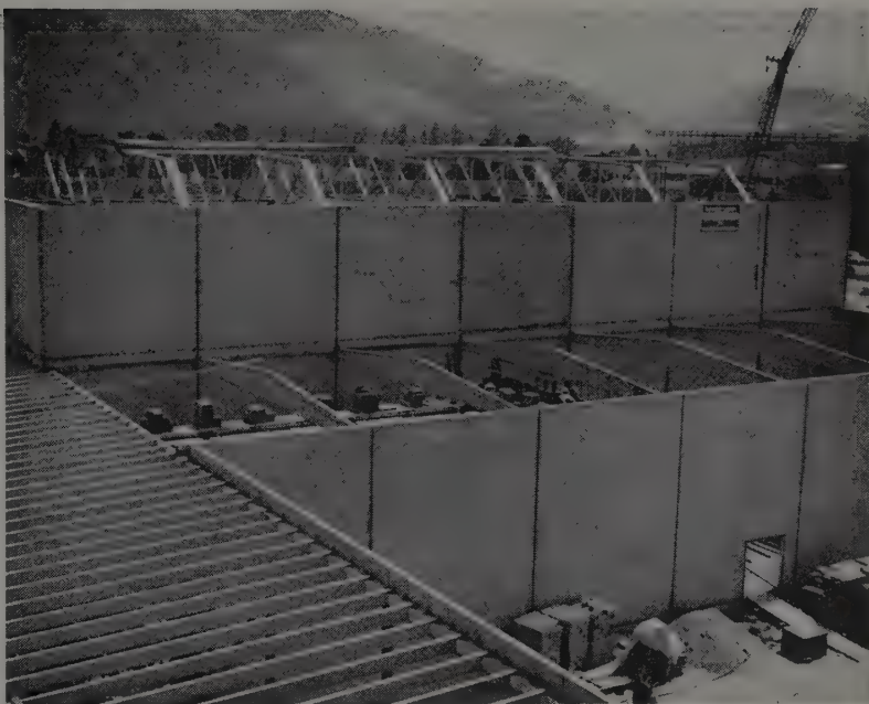
SERVICE CORRIDOR in the foreground connects old studios to new construction. Near structure has 27-ft. high walls and clear-span 50-ft. long steel beams. Color studio is next.
