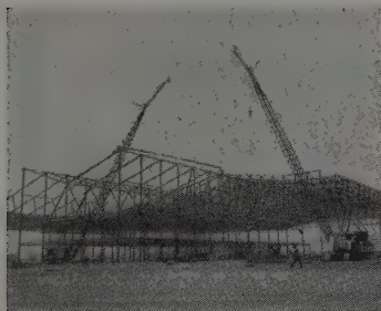
Fig. 1. 347-ton welded framework at Idlewild Airport. Designed to house 5 large and 3 small transports. Designed by Port of New York Authority. Fabricators and Erectors, Lehigh Structural Steel Company.
